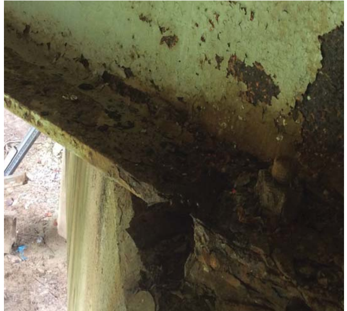
PHOTO 15 Description 02872 10-01-2015 Span 2 Girder 2 over bent 2 bottom flange.
