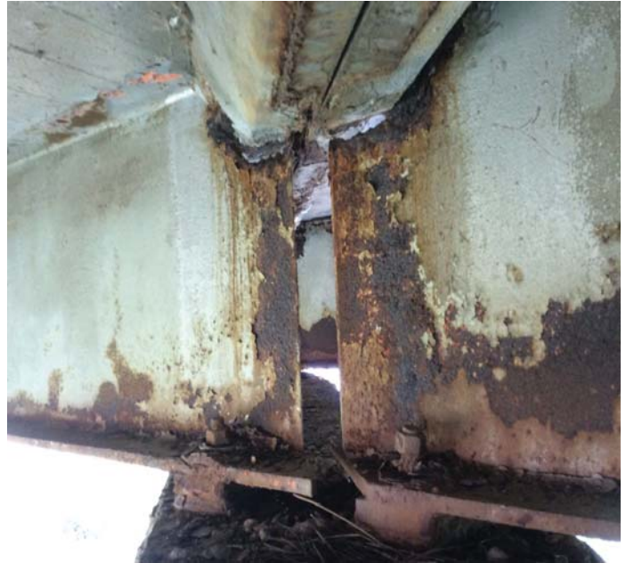
PHOTO 19 Description 02872 10-01-2015 Span 3 & 4 Girder 4 over Bent 4.
