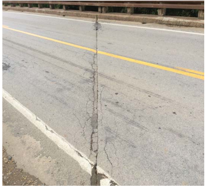
PHOTO 2 Description 02872 10-01-2015 Bent 3 joint spalls.
