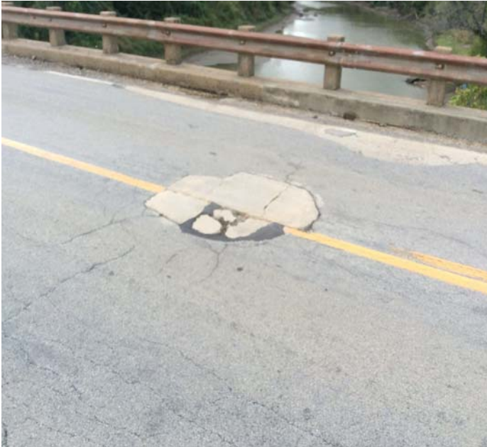
PHOTO 3 Description 02871 10-01-2015 Span 2 centerline repair.
