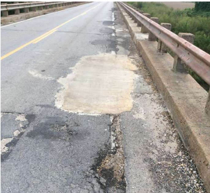
PHOTO 4 Description 02871 10-01-2015 Span 3 Right lane repair.
