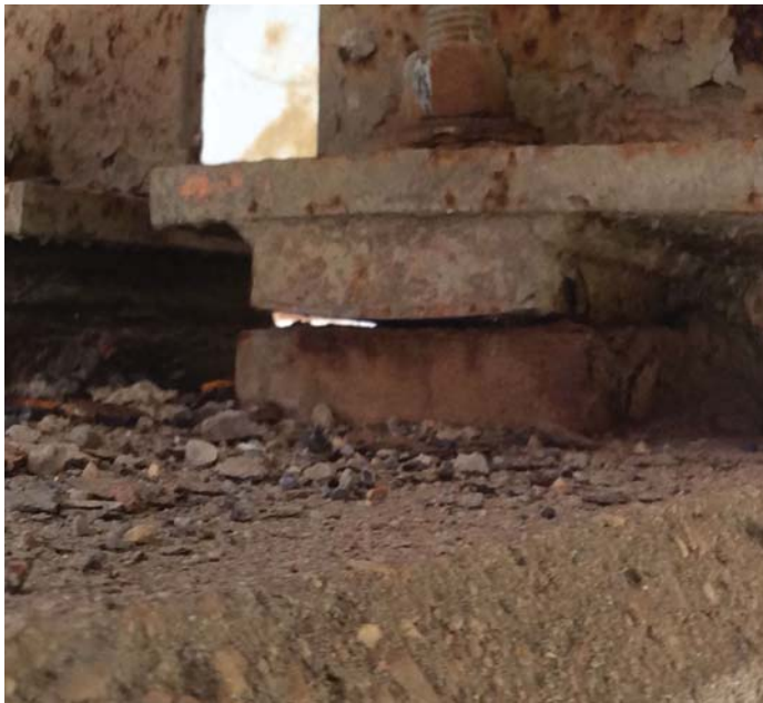
PHOTO 1 Description 02871 10-01-2015 Span 2 Girder 2 over Bent 3 Movement under traffic.
