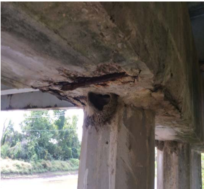
PHOTO 4 Description 02871 10-01-2015 Bottom of Bent 2 Cap near Pile 3.
