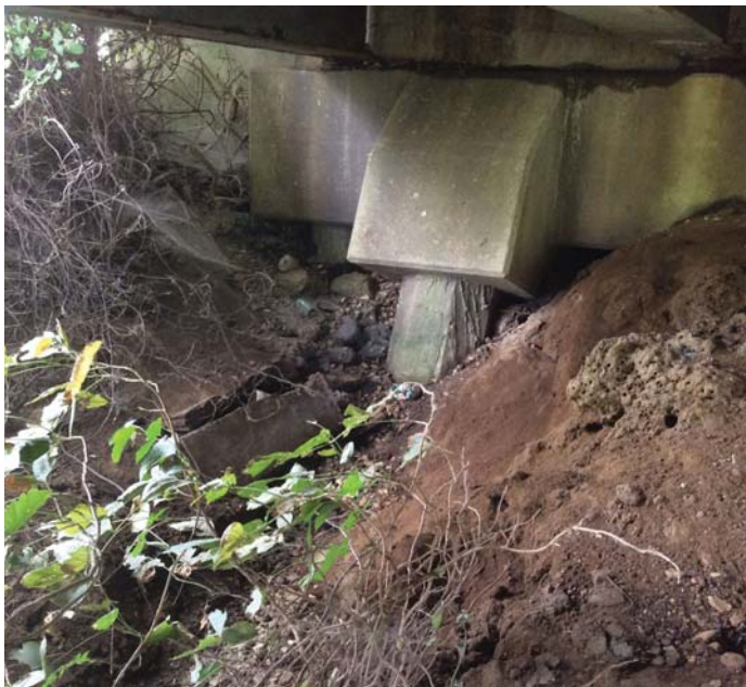
PHOTO 1 Description 02871 10-01-2015 Bent 9 left end of abutment erosion.
