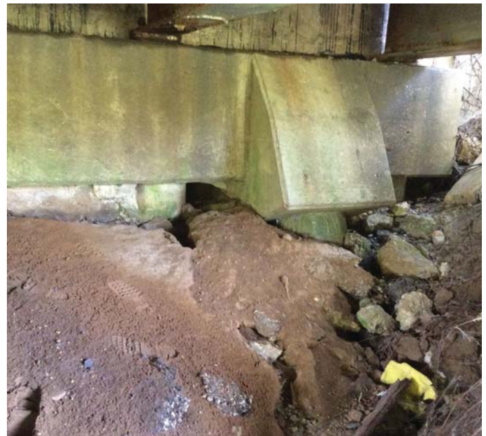
PHOTO 2 Description 02871 10-01-2015 Bent 9 right end of abutment erosion.
