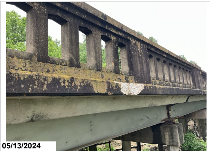
Span 1 Rt overhang has 2' spall near mid span cs3
