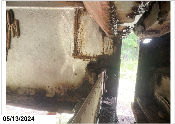
Span 2 bent 2 girder 4 has a welded web splice at haunch.
