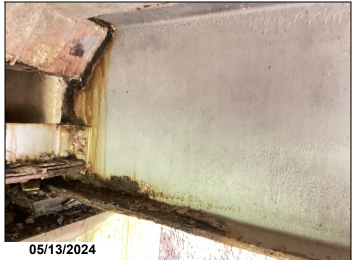
Span 5 bent 6 girder 4 has 2' of moderate section loss (up to 3/16") at web below haunch, diaphragm connection and along bottom of web.
