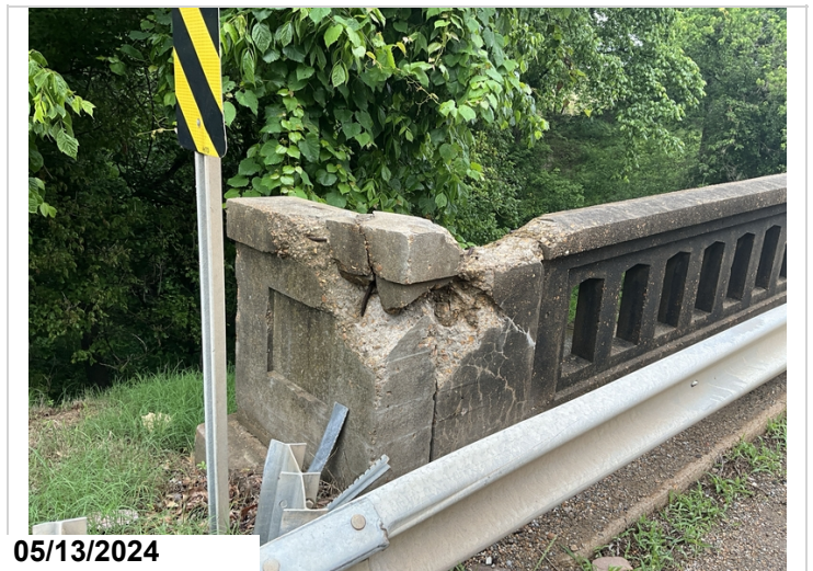
Bent 6, Right side: collision damage at bridge rail end post with exposed rebar cs2
