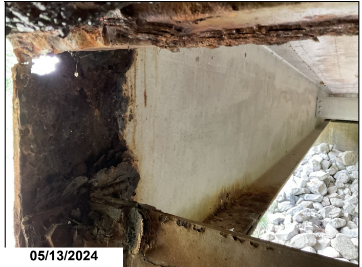
Span 1 bent 2 girder 4 has a 2" x 1" hole at web below haunch.
