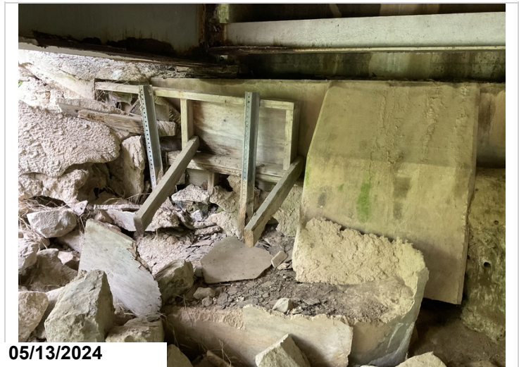
Bent 6 Lt scour repair
