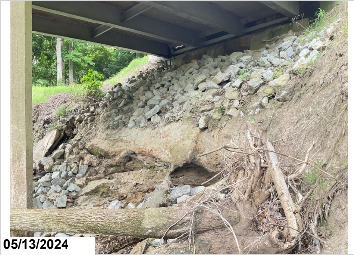
Embankment under span 5 has scour at toe of slope with rip rap displacement
