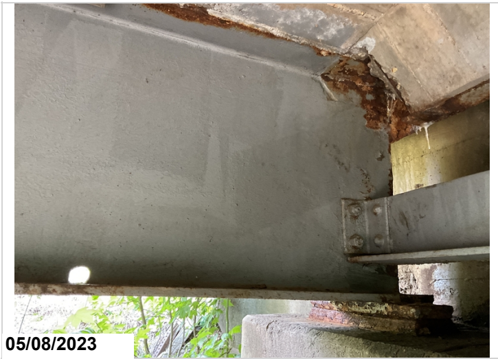
Span 1 bent 1 girder 4 - typ girder repair
