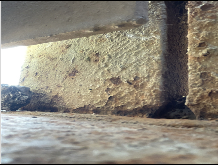
L1 Lt section loss to 1 angle of vertical
