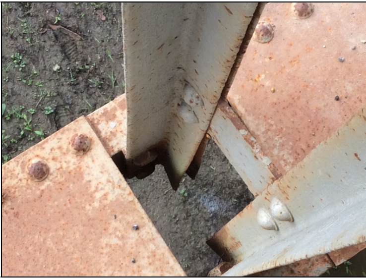
Left truss unit L3 connection pack rust.
