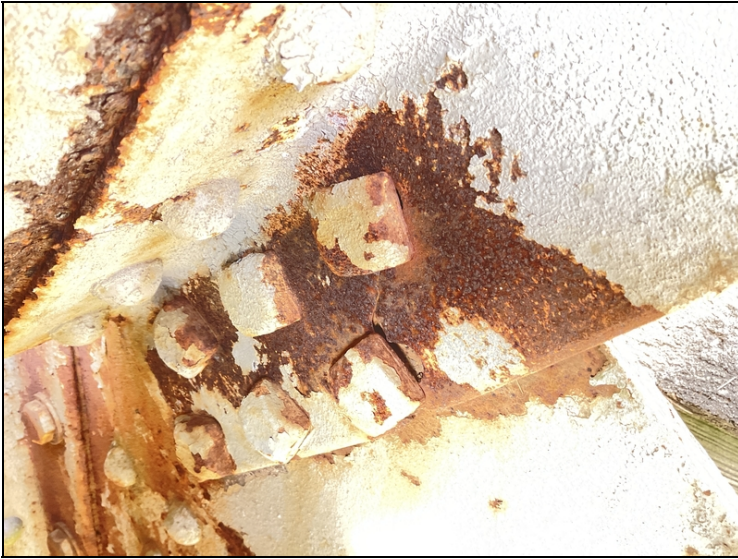
2021 - Interior angle of U5 - L6 diagonal Lt bottom
