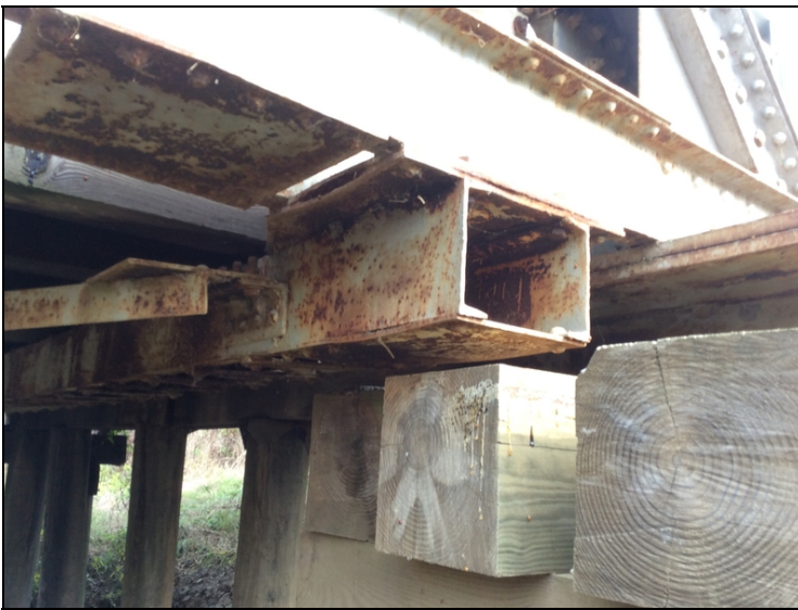
Left end of lower lateral brace bent 3.
