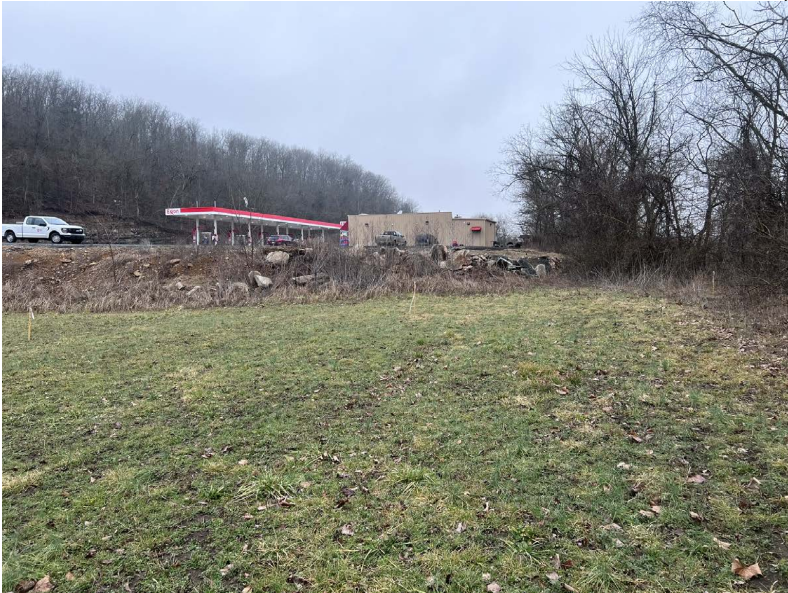
Looking north from proposed location of west bridge end with boring locations marked (February 2025)
