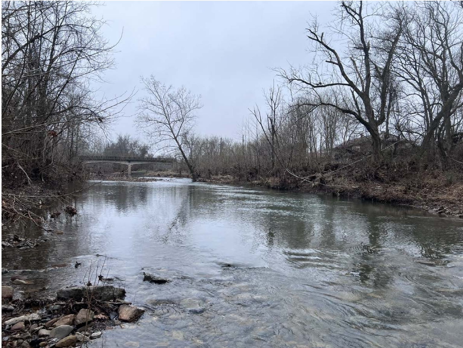
Proposed bridge location looking upstream towards existing bridge (February 2025)
