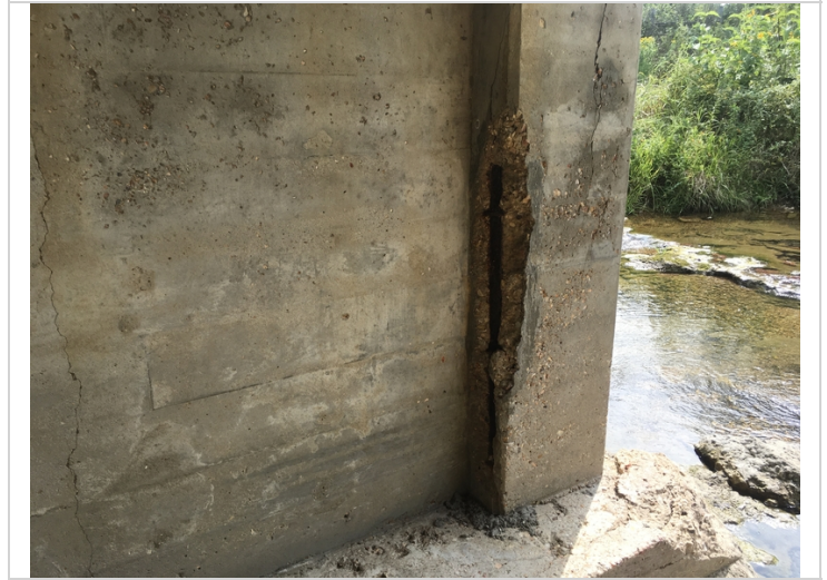
Right column of bent #1 has a spall with exposed rebar.
