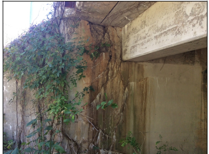
Abutment #2, Left side, Concrete deterioration with mapcracking and spalling.
