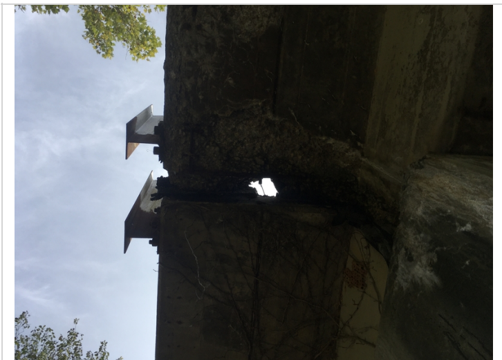
The pourable joint seal has Cs4 leakage at the bent #1 left deck edge.
