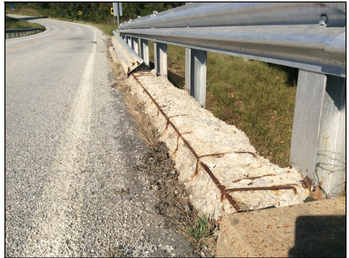
Span #1 concrete curb, Left side, concrete deterioration with exposed reinforcing steel to curb.
