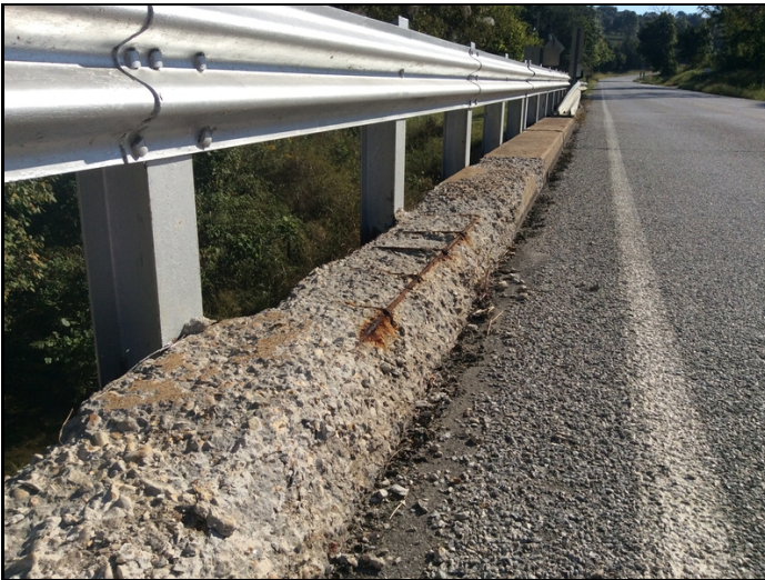
Span #2, Left side, concrete deterioration / spalling with exposed reinforcing steel to curb.
