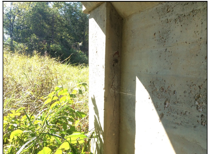
Bent #3, Right column, large delaminated area.
