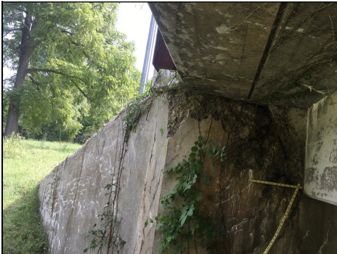
Abutment #2 has a large area of deteriorated concrete with efflorescence map cracking next to beam #1. The left wing wall has heavy map cracking with concrete deterioration and spalling along the top of the wing wall.
