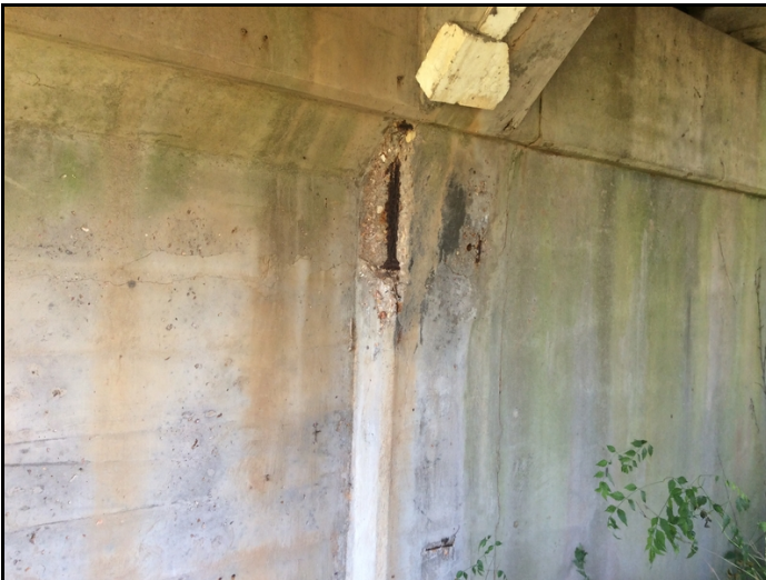
Bent #3, column #1 has a 14" spall with exposed primary reinforcing steel below bent cap.
