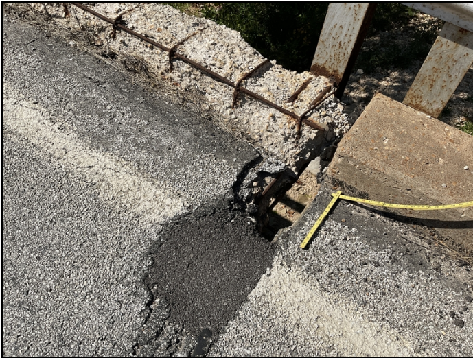
Spalling in the left lane at the end of span #1.
