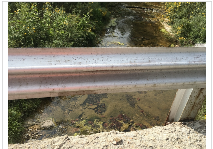
Freckled rust beginning to form on front side of railing.
