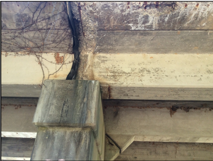
Girder #1 of span #1 over bent #2 has an area of spalling.
