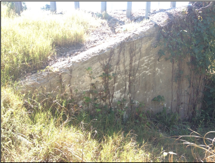
Northwest wing wall, Concrete deterioration and spalling
