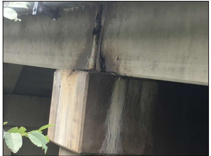
Vertical delamination on beam #4 at the beginning of span #5 over bent #4.
