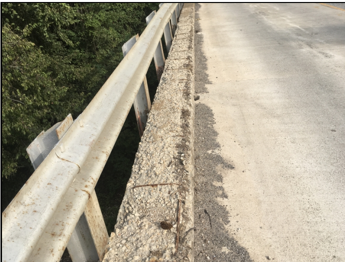
View of deterioration with exposed rebar in the left and right curb sections.
