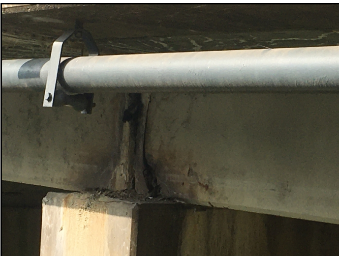
Vertical delamination on tee beam #4 over bent #4.
