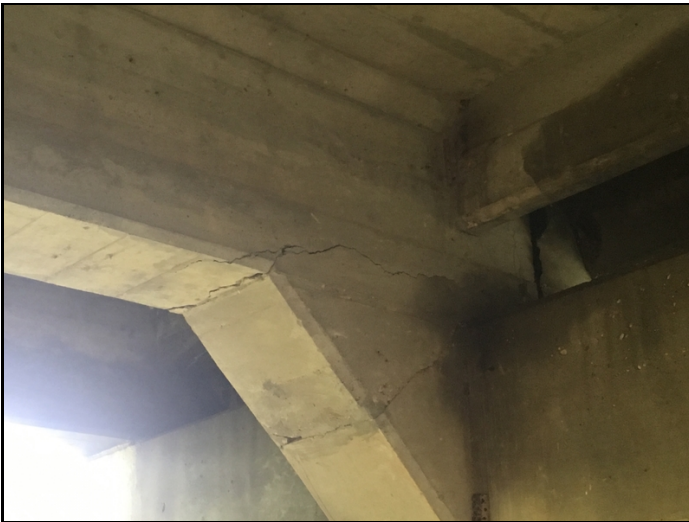
3' long horizontal crack at the beginning of span #5 in beam #3. Beam #2 also has the same crack at the same location.
