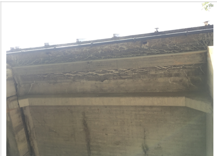
Typical view of efflorescence cracking in the left and right deck edges.
