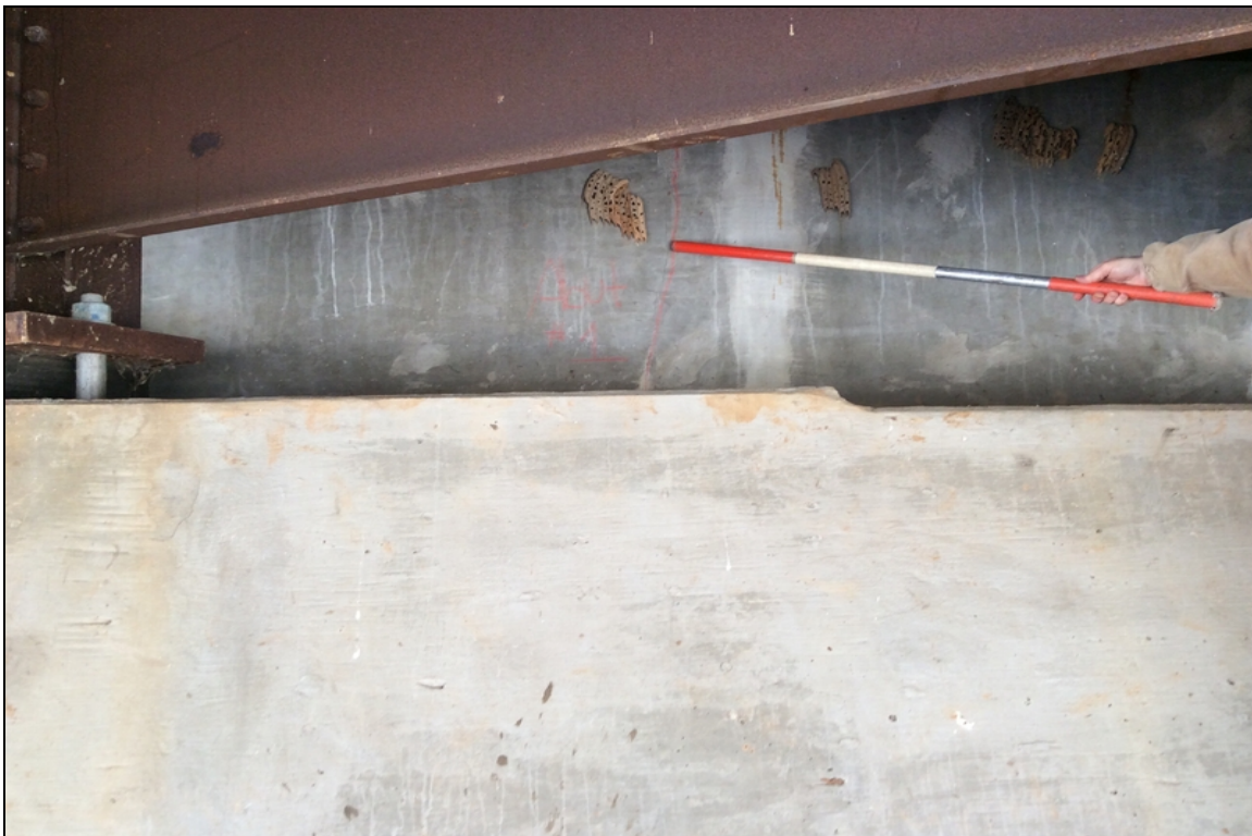
Vertical cracking in backwall.
