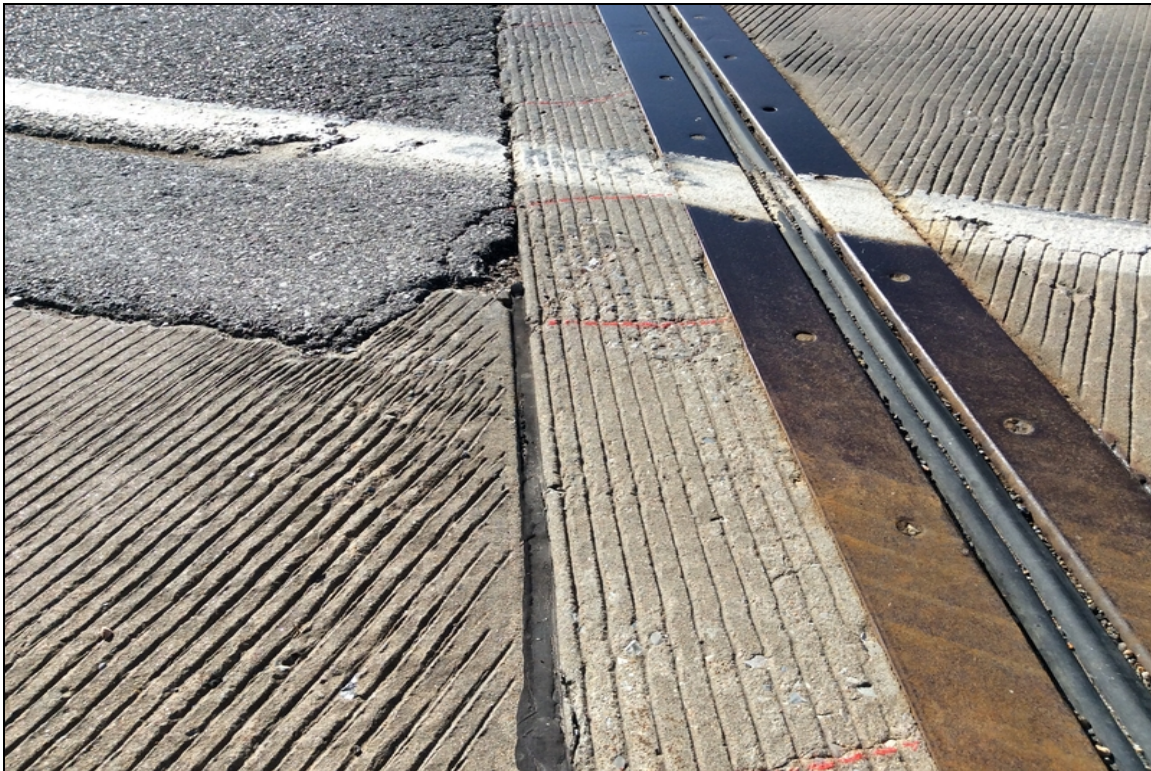
Transverse cracking in the backwall.
