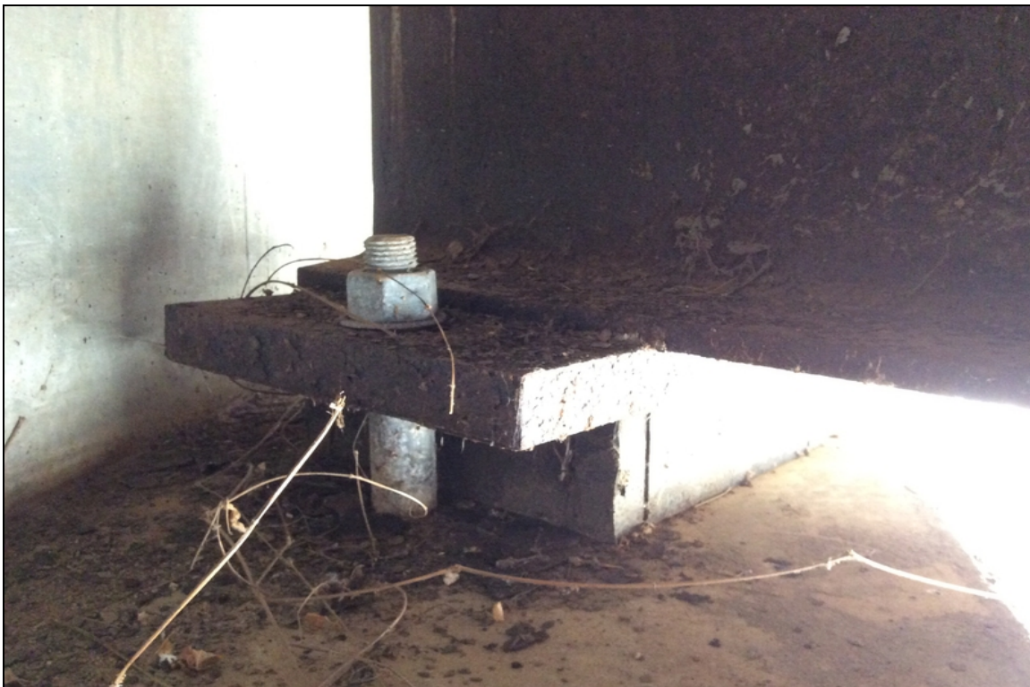
Abutment #2, bearing #4-Abnormal weathering.
