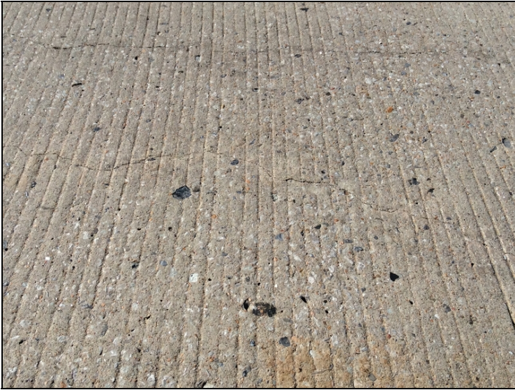
Longitudinal deck cracking.
