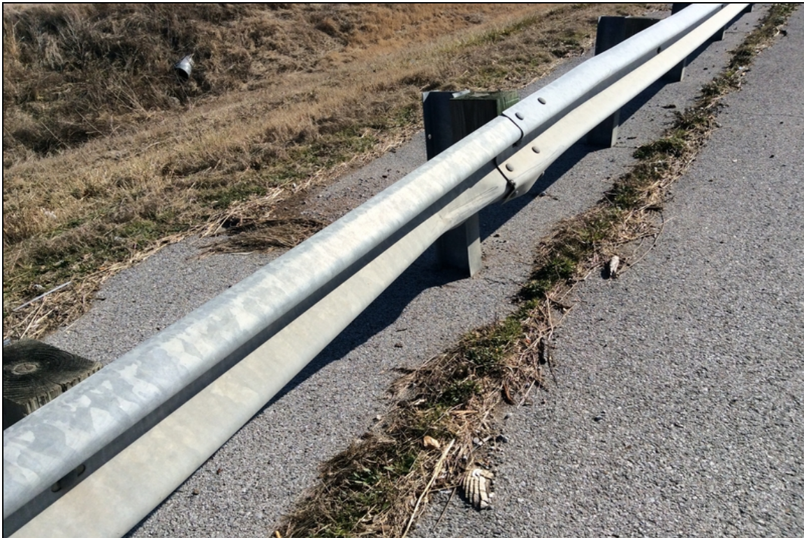
Collision damage at guardrail approximately 40 feet from bridge end. Southeast railing.
