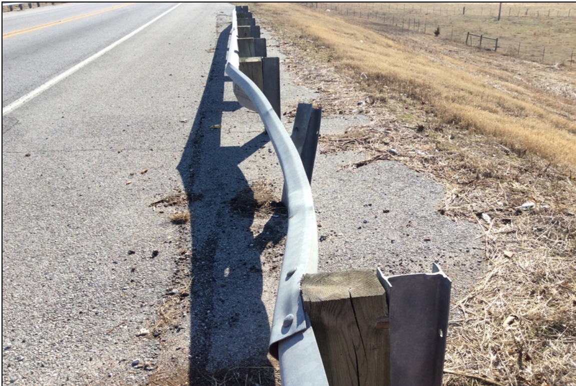
Collision damage at guardrail approximately 20 feet from bridge end. Southwest railing.
