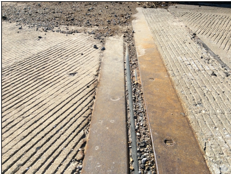
Abutment #1-Debris impactation in compression joint.
