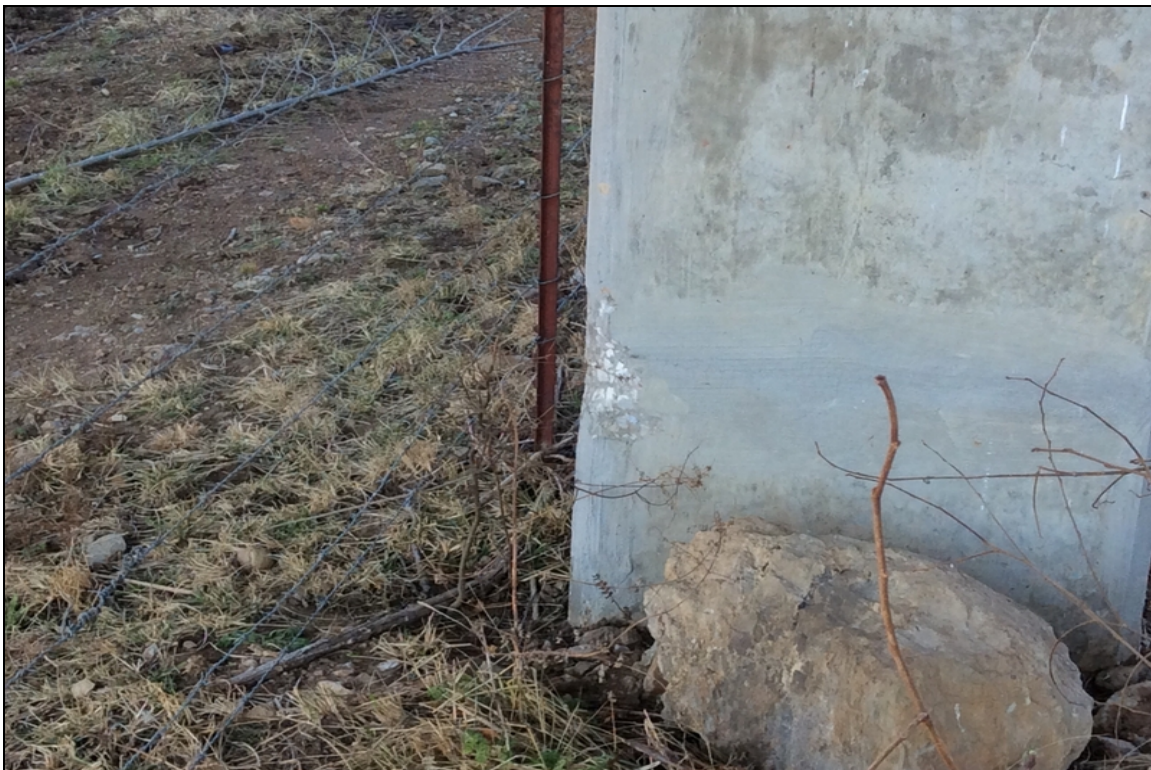
Bent 2 column 1 softball sized shallow spall
