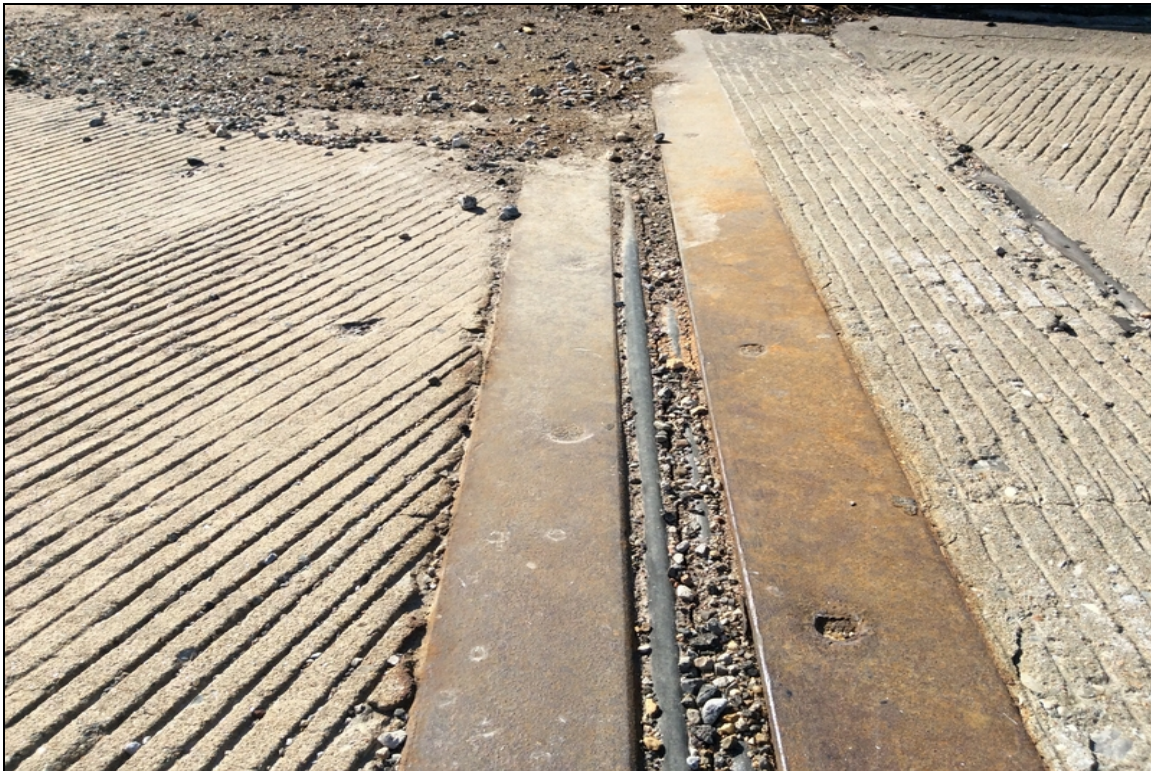
Abutment #1-Debris impact in compression joint.
