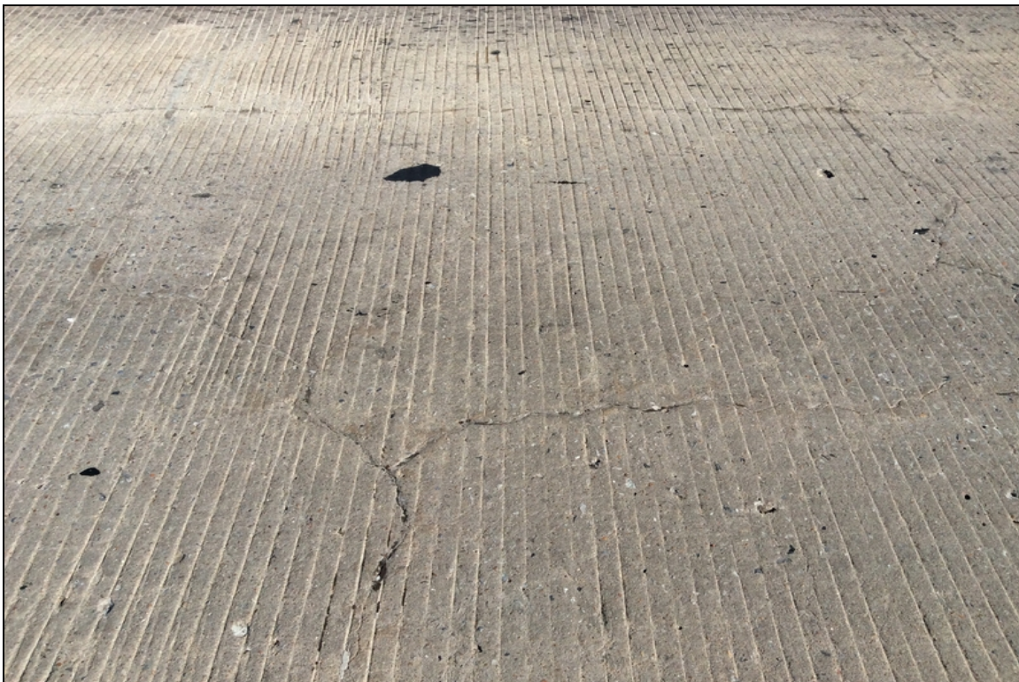
Cracking span 1 right side near mid span.
