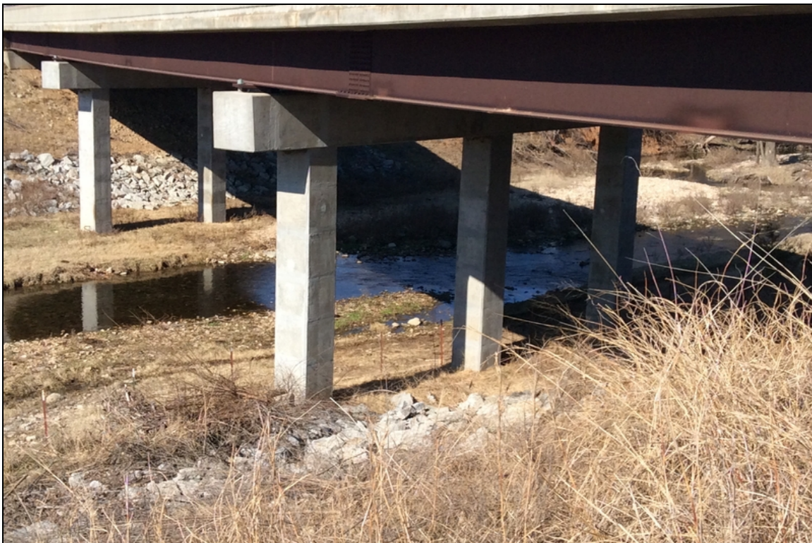
Substructure footings have cover.
