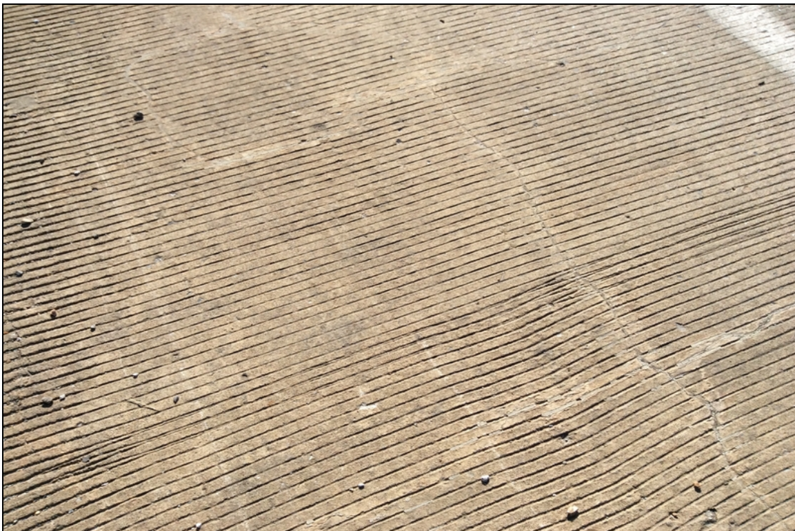
Cracking in deck span 2 near bent 1.
