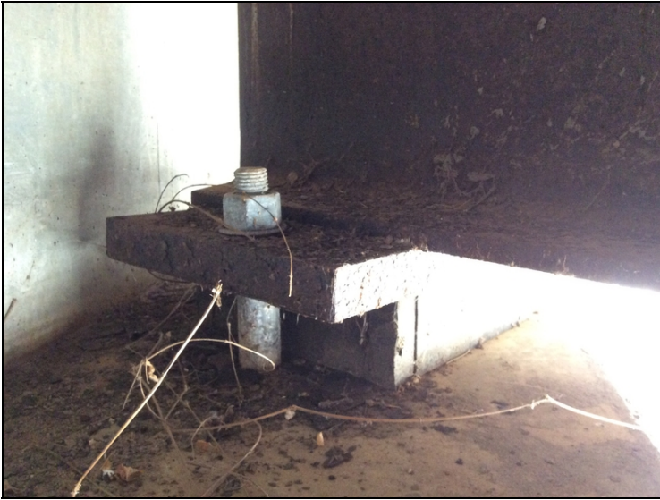
abnormal weathering to girder end and bearing device.
