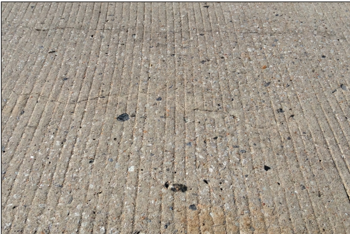
Cracking span 1 Left side near bent1
