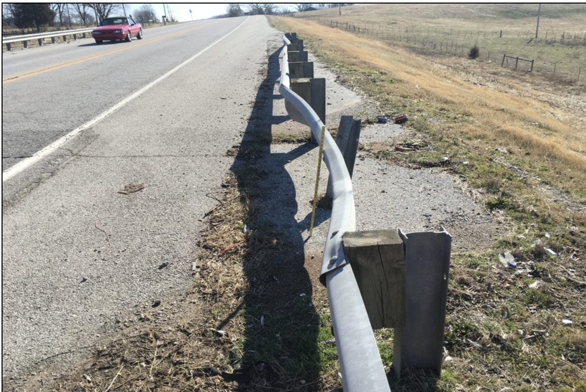
Approach rail damage at the right end of the structure.
