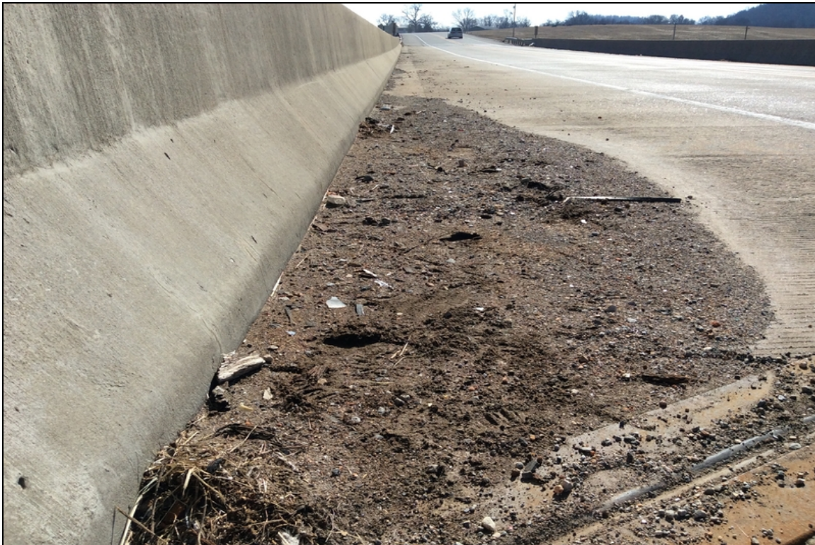
The gutters in span #1 have dirt and debris accumulation near abutment #1.
