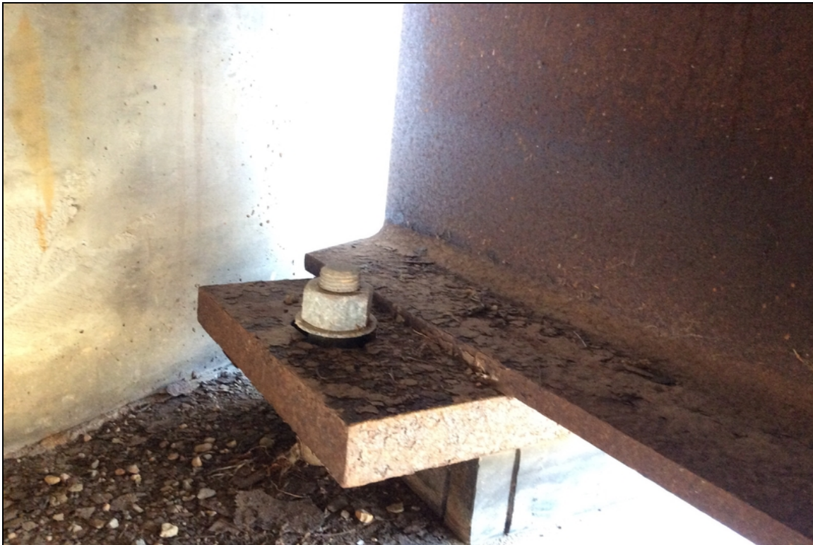
Corrosion with flaking rust.
