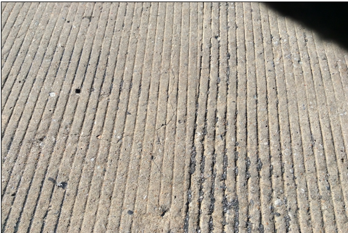
Cracking in span 1 Left side near abutment 1.
