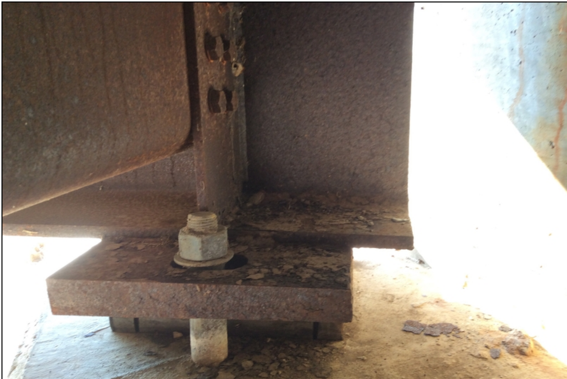
Corrosion with flaking rust
