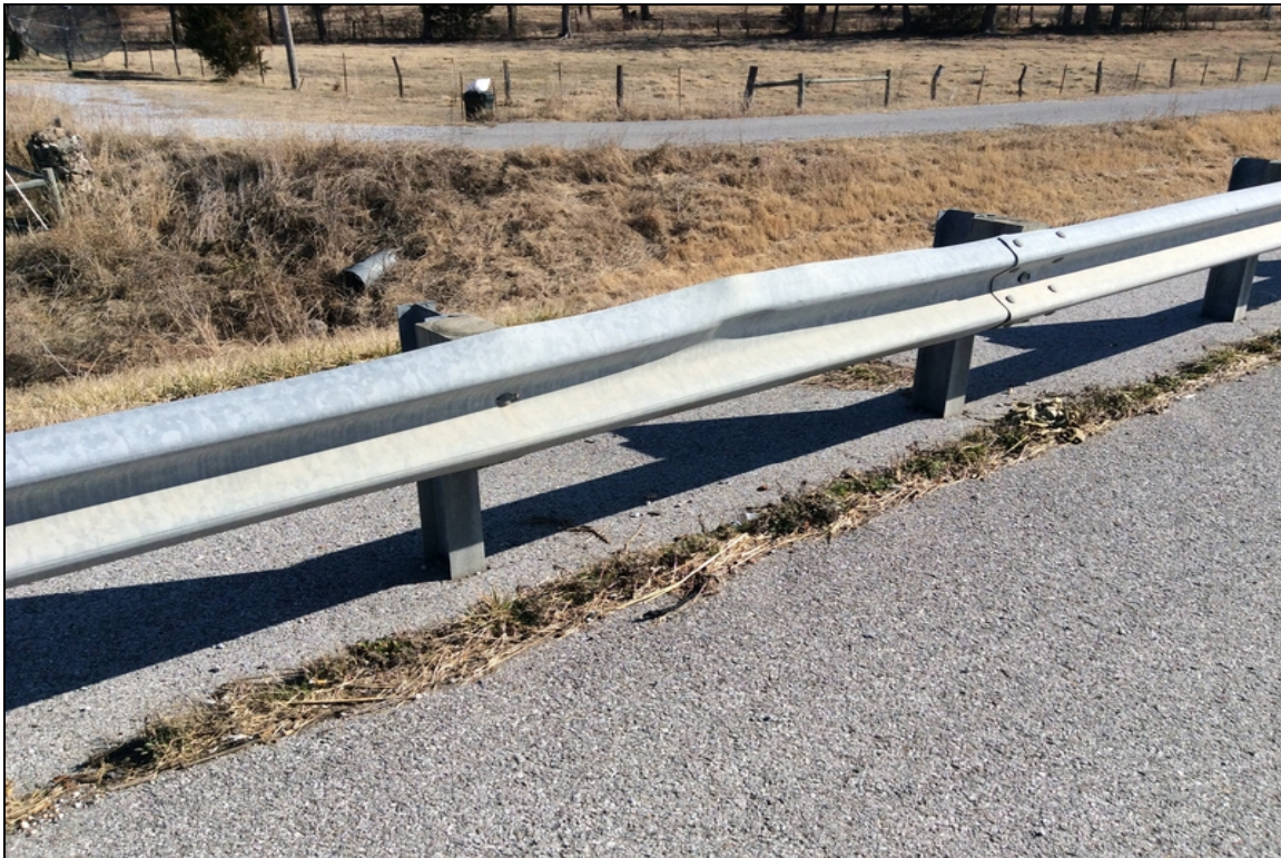
Collision damage at guardrail approximately 60 feet from bridge end. Southeast railing.
