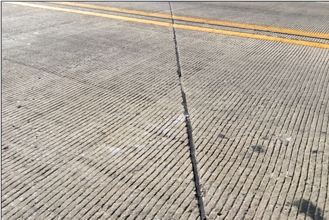
Bent 2 joint seal missing.
