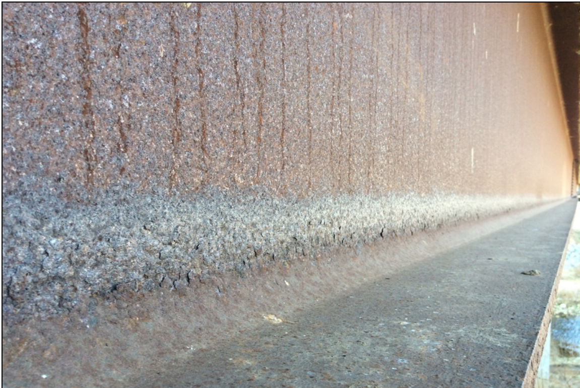
Girder #1-Abnormal weathering to exterior side.
