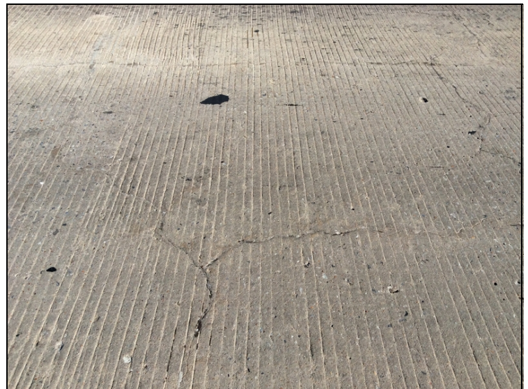
Deck cracking.
