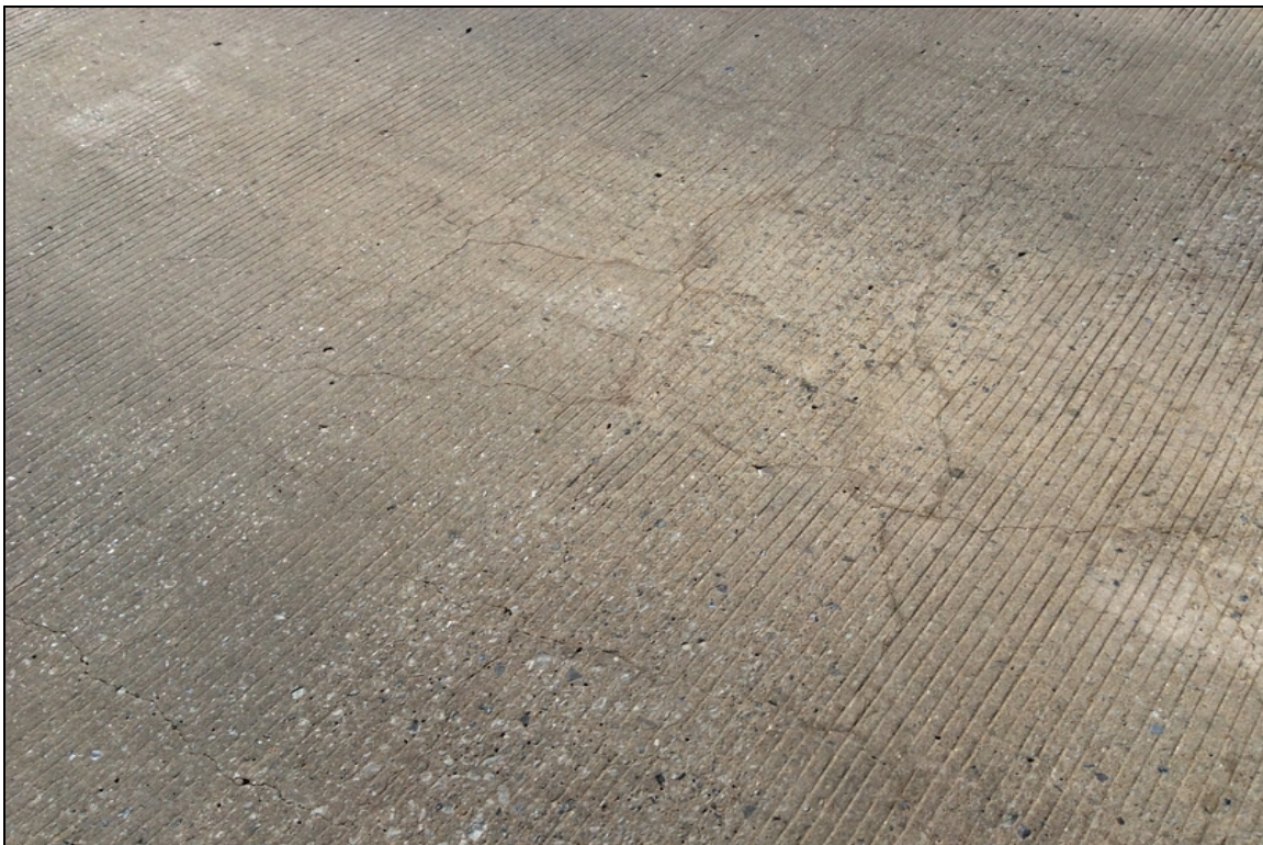
Map cracking in span 3 Left side center of north bound lane.
