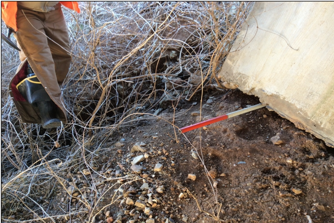
Abutment 2 Left side has minor earth settlement.
