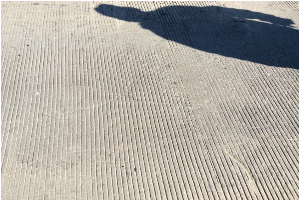
Cracking span 1 right side near mid span.
