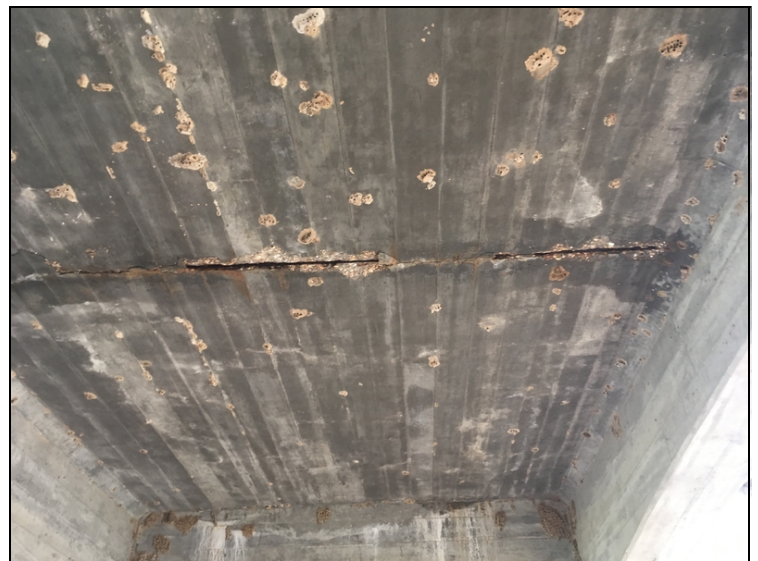
Spalling with exposed reinforcing steel in spans #2, 7, and 9.
