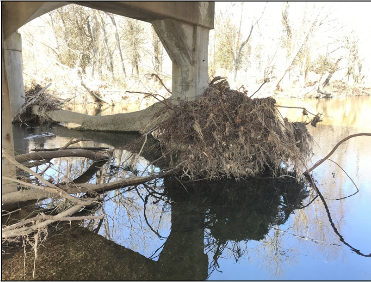
Bents #2 and #3 have Large trees and drift accumulation causing localized scour.
