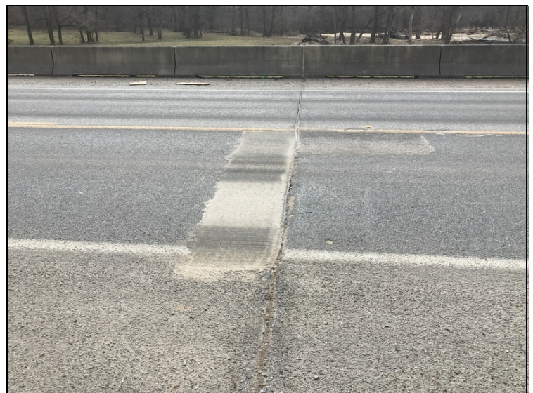
Span #8 Failed patched area in the approach span has been repaired since las inspection.
