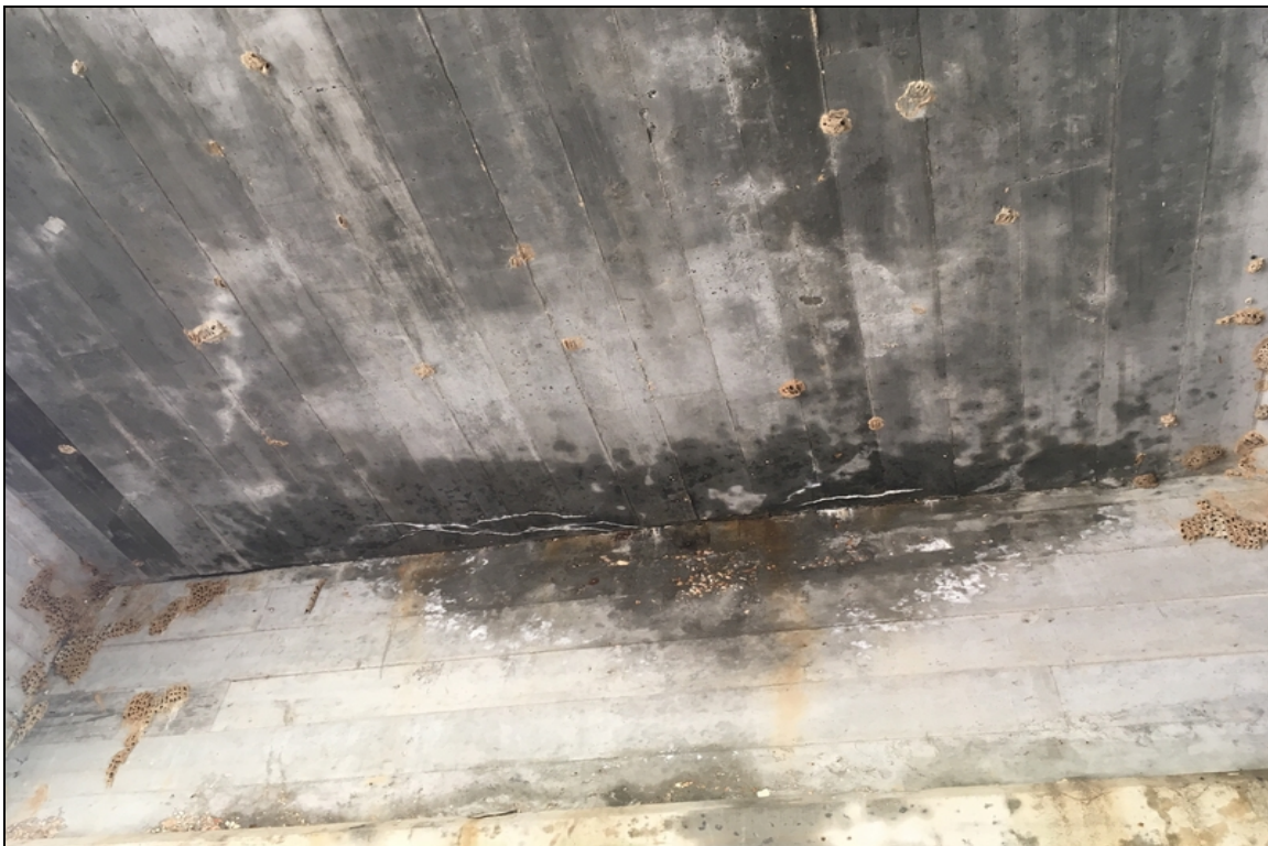
Span 10 has cracking with efflorescence
