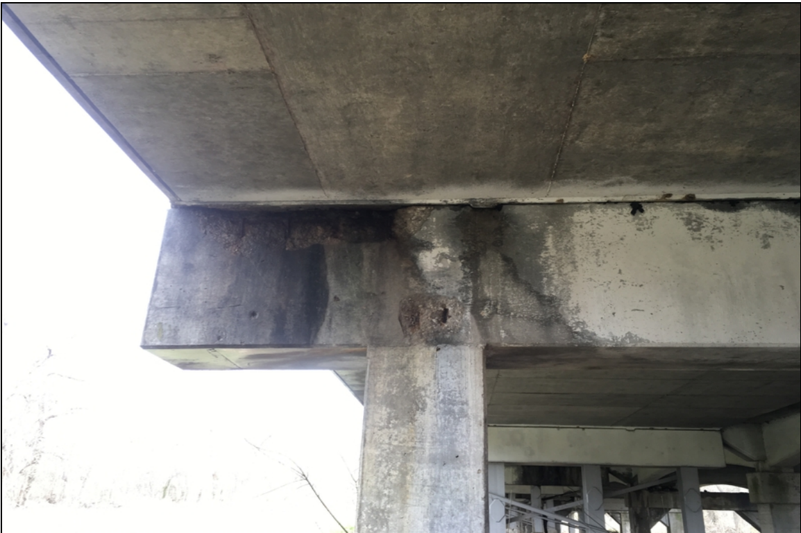
Bent 9 has spalling with exposed reinforcing steel
