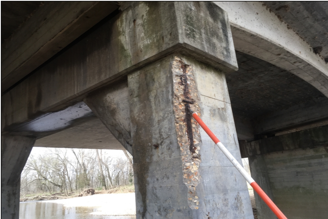
Bent 3 Column 1 has Spalling with exposed reinforcing steel
