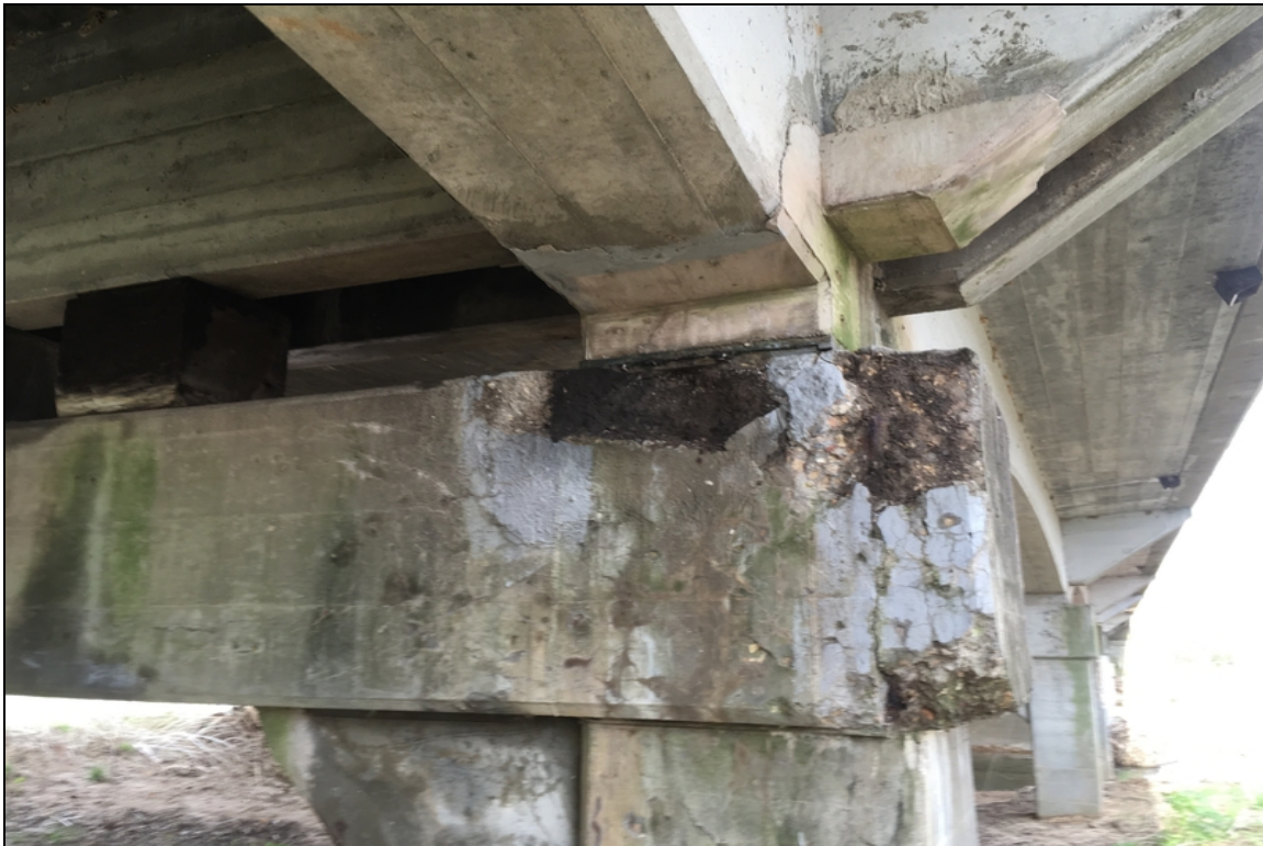
Bent 5 has Spalling with exposed reinforcing steel
