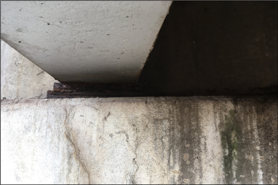
Bearings have Active corrosion with flaking rust
