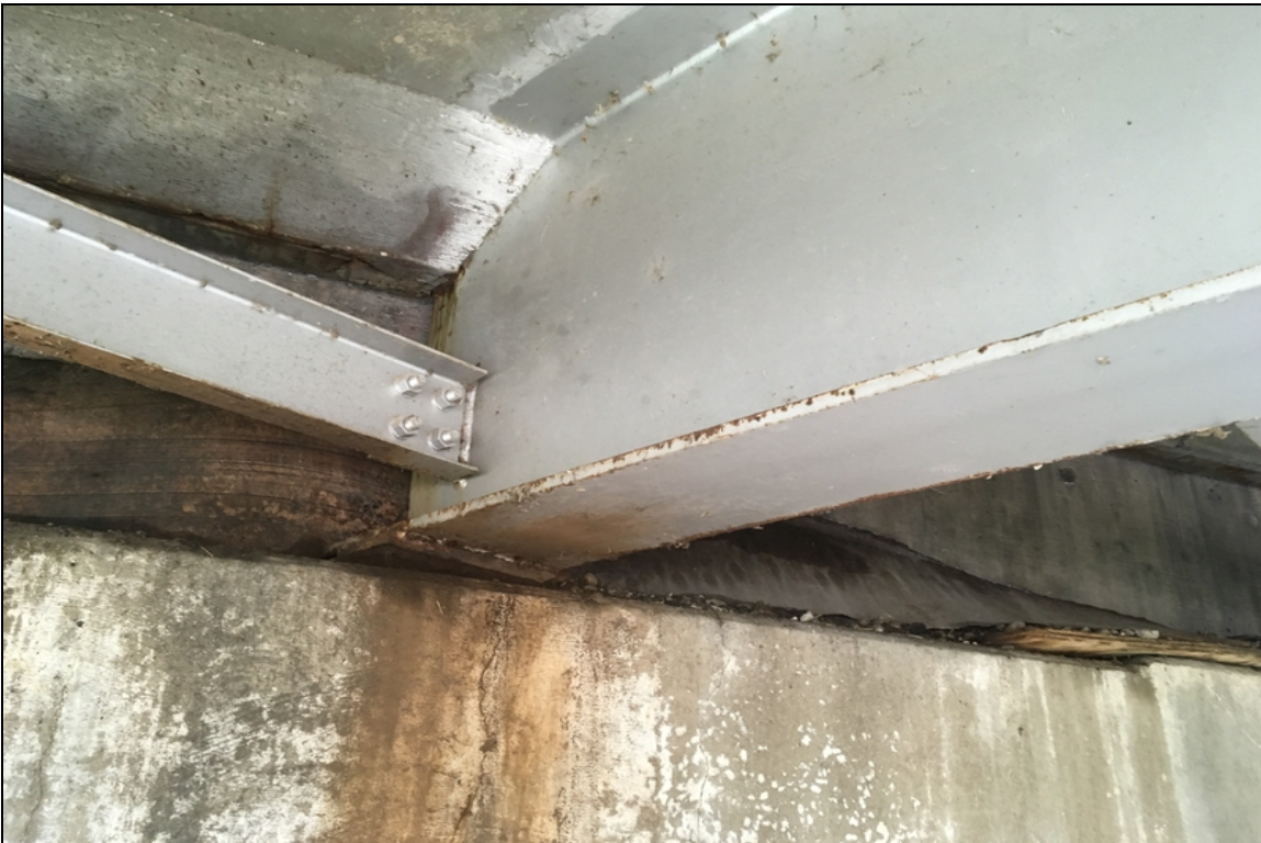
Beam ends have paint failure with active corrosion
