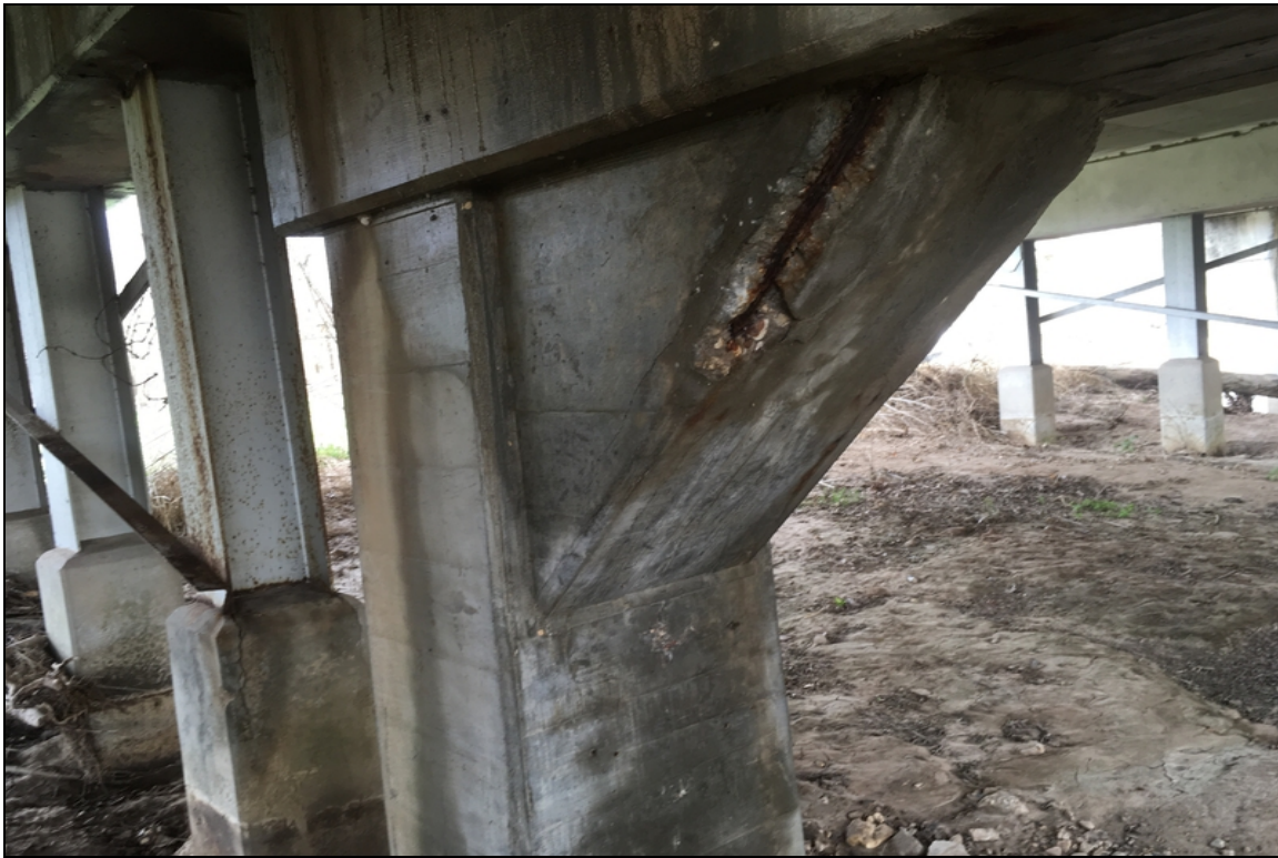
Haunches have exposed reinforcing steel
