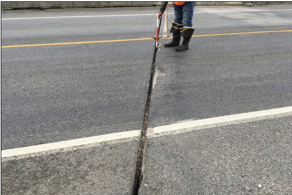
Abutment 1 pourable joint Seal is missing allowing dirt and debris on top of bridge seat
