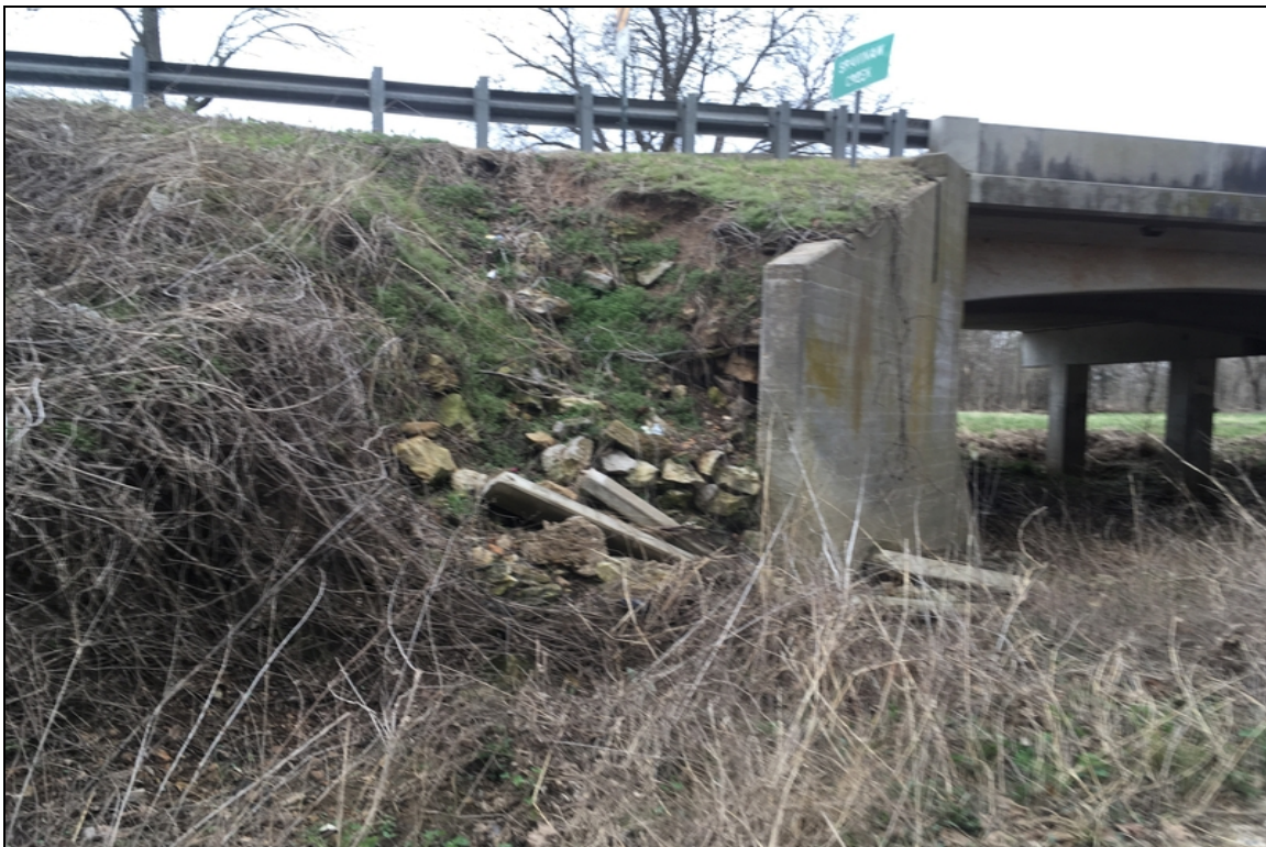
Erosion behind left wing wall at Abutment 2
