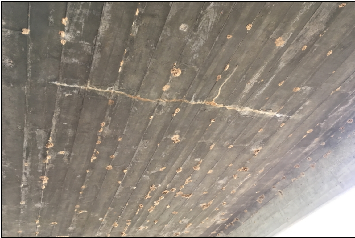
Span 7 has transverse cracking with efflorescence
