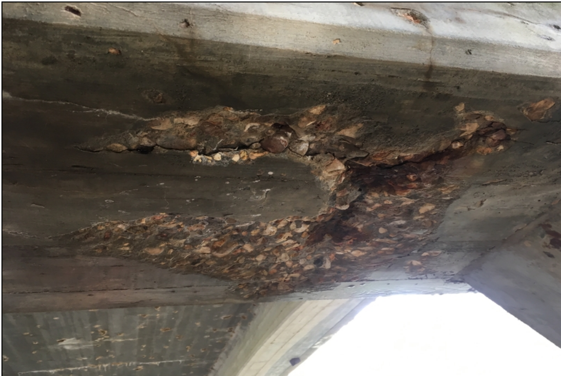
Bent 7 has exposed reinforcing steel on the under surface of cap
