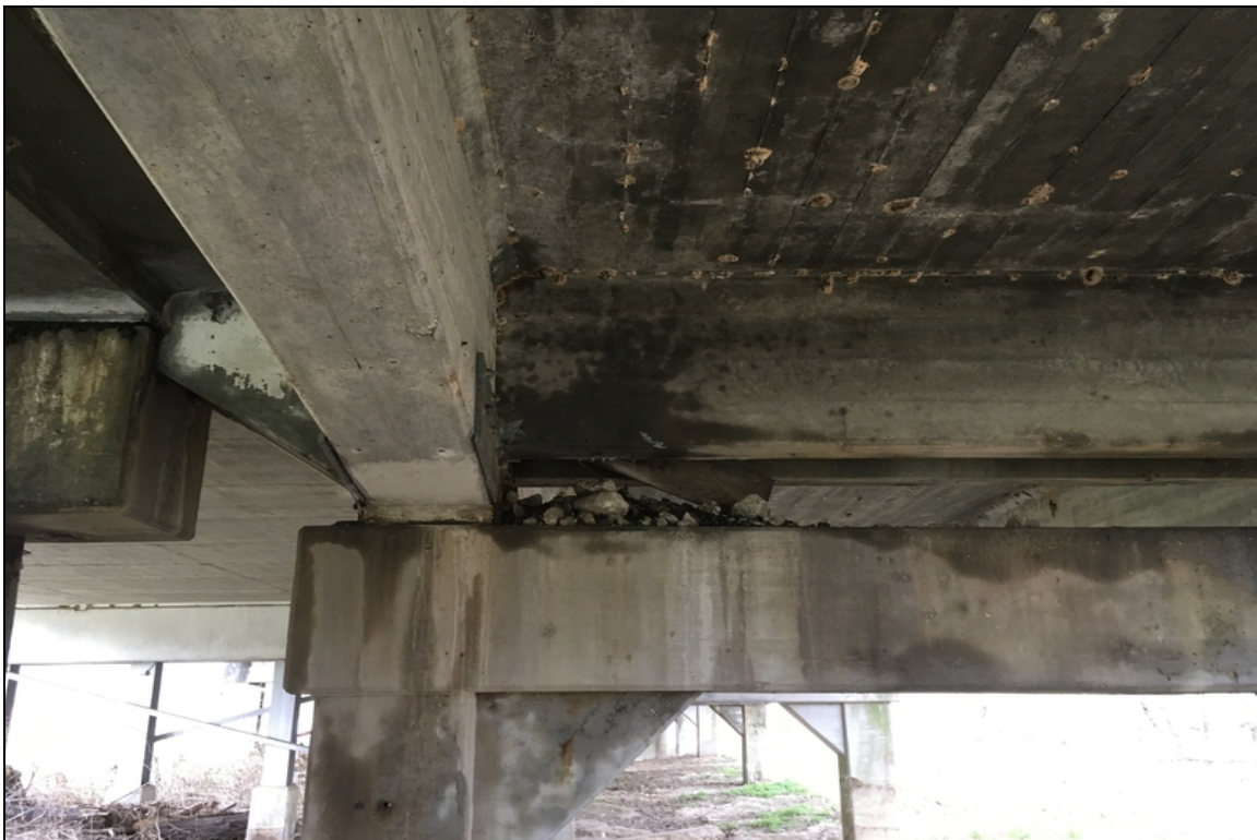
Bent 7 Cap has dirt and debris accumulation
