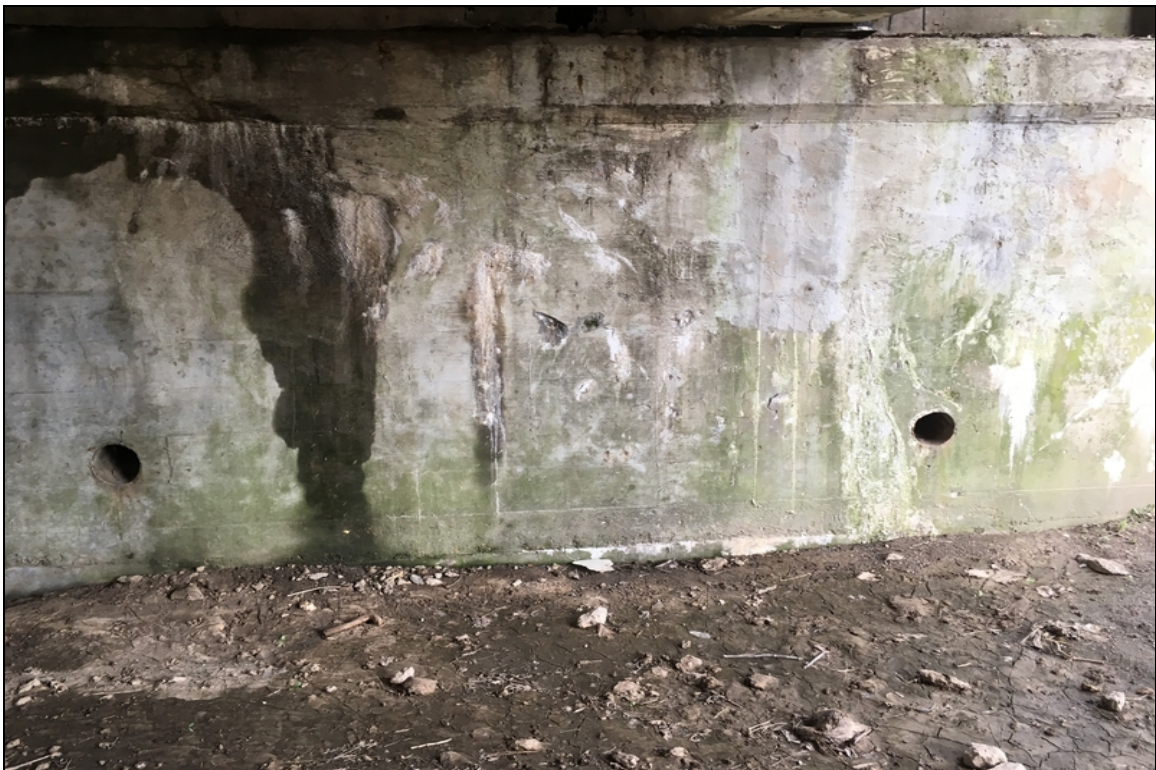
Abutment 1 has efflorescence build up
