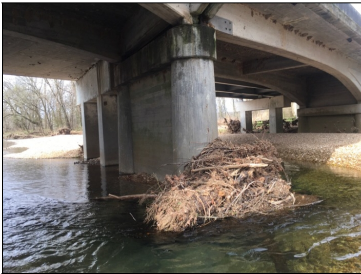
Minor drift accumulation at bent 2.
