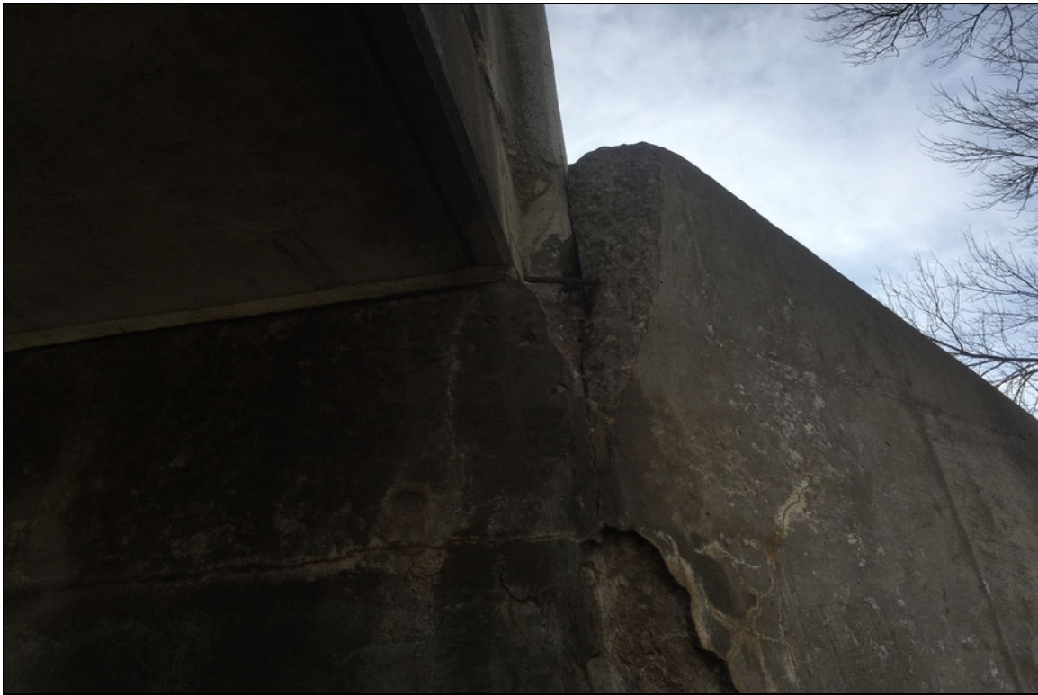
Abutment 2 right wingwall juncture has spalling that exposes the reinforcing steel with initial section loss.
