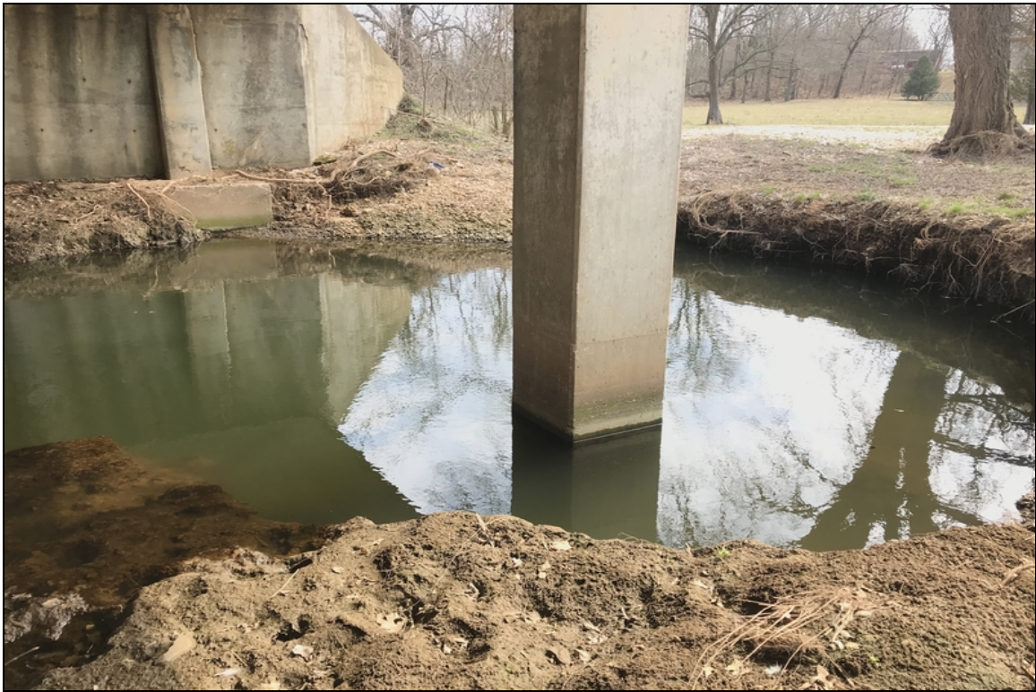
Channel at bent #10 right has a localized scour since last inspection due to high water event.
