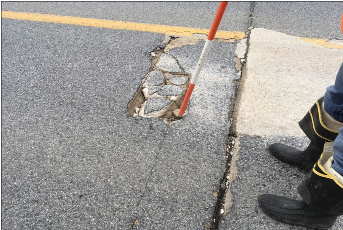
Failed patched area in the approach spans
