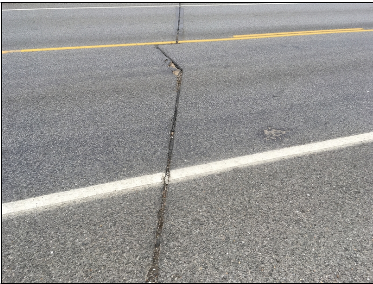
Adhesion failure
