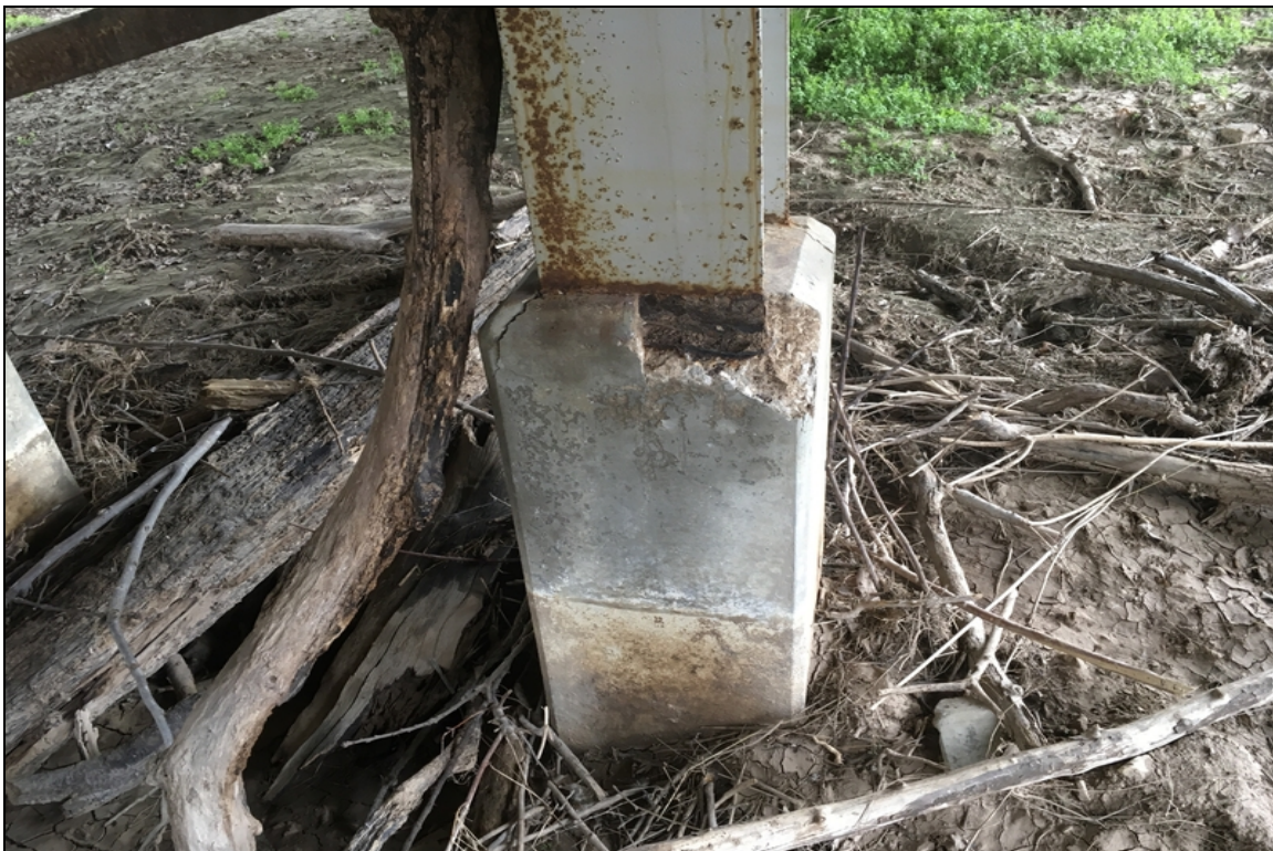
The reinforced concrete is Spalling and cracking at the base of the steel piles
