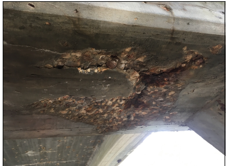
Bents #1, 2, 3, 5, 6, 7, & 9 has concrete delaminations and spalling that exposes the reinforcing steel with measurable section loss.
