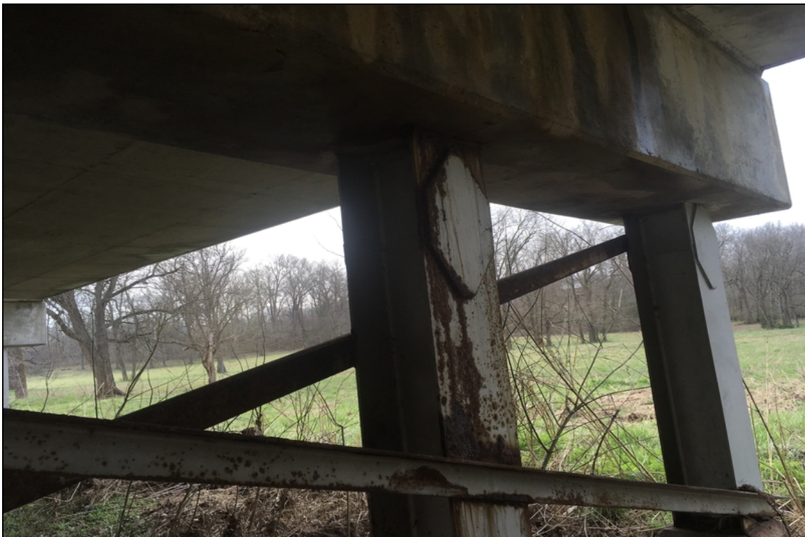
Steel piles have Active corrosion with Section loss
