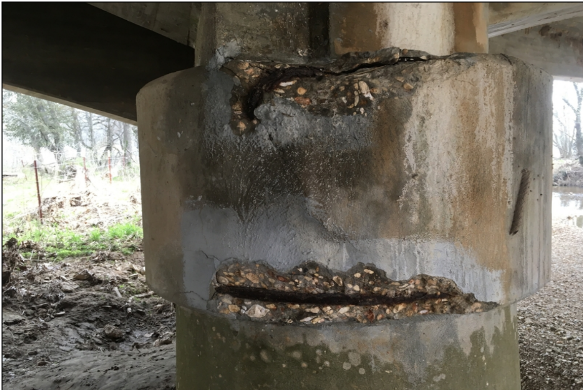
Bent 2 Column 2 has Spalling with exposed reinforcing steel
