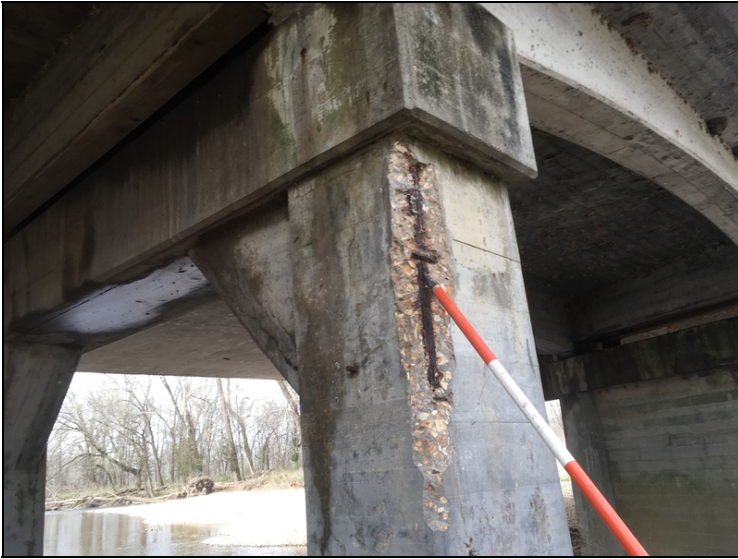
Bent 9 (column 2), bent 2 (column 2), bent 3 (column 1), has concrete delaminations and spalling that is exposing the reinforcing steel with measurable section loss.
