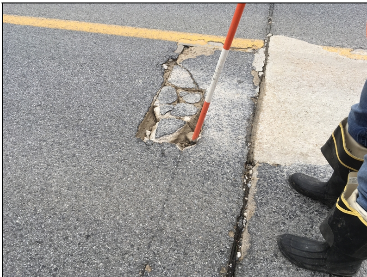
Span #8 Failed patched area in the approach span.
