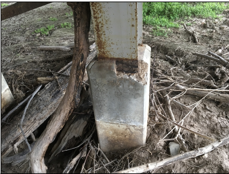
The reinforced concrete is spalling and cracking at the base of the steel piles
