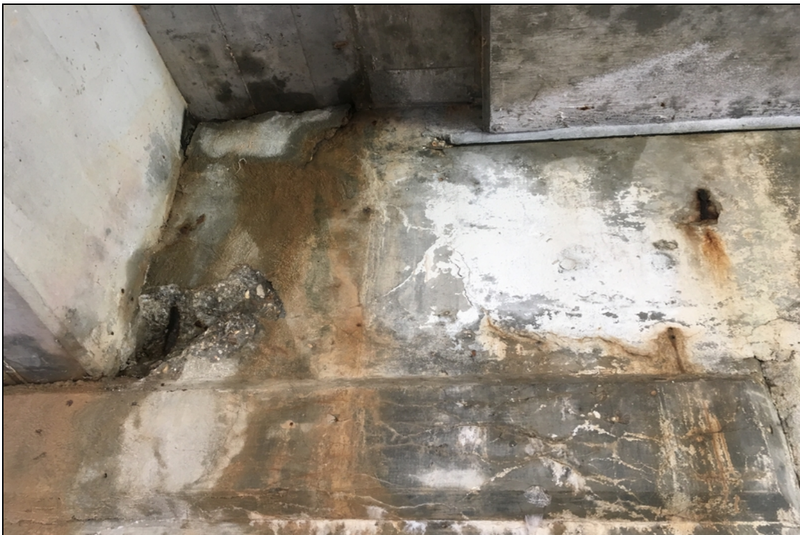
Centerline of abutment 2 breastwall has spalling with exposed reinforcing steel with initial section loss.
