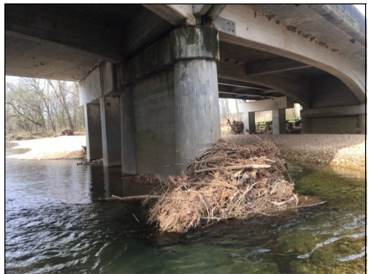
Pier 2 has drift accumulation
