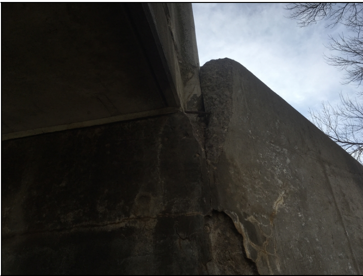
Abutment 2 right wingwall juncture has spalling that exposes the reinforcing steel with initial section loss.
