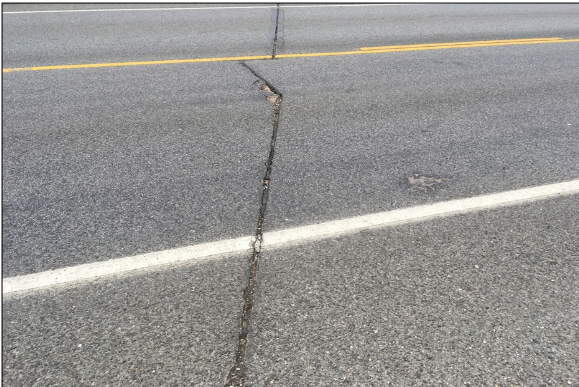
Adhesion failure
