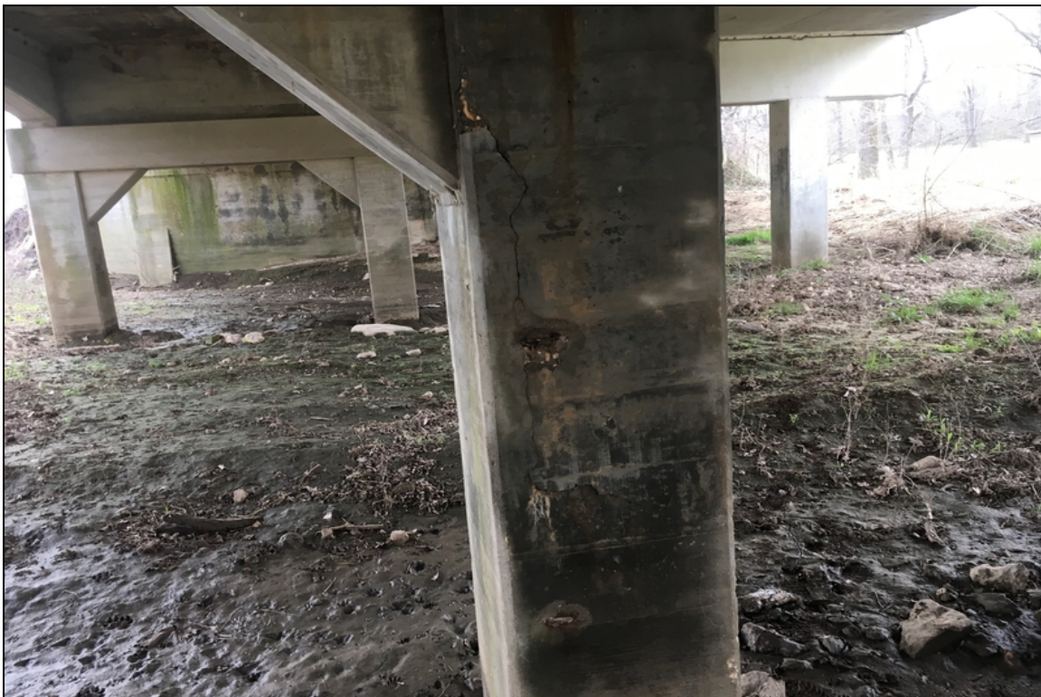
Bent 9 column 2 have spalling with exposed reinforcing steel.
