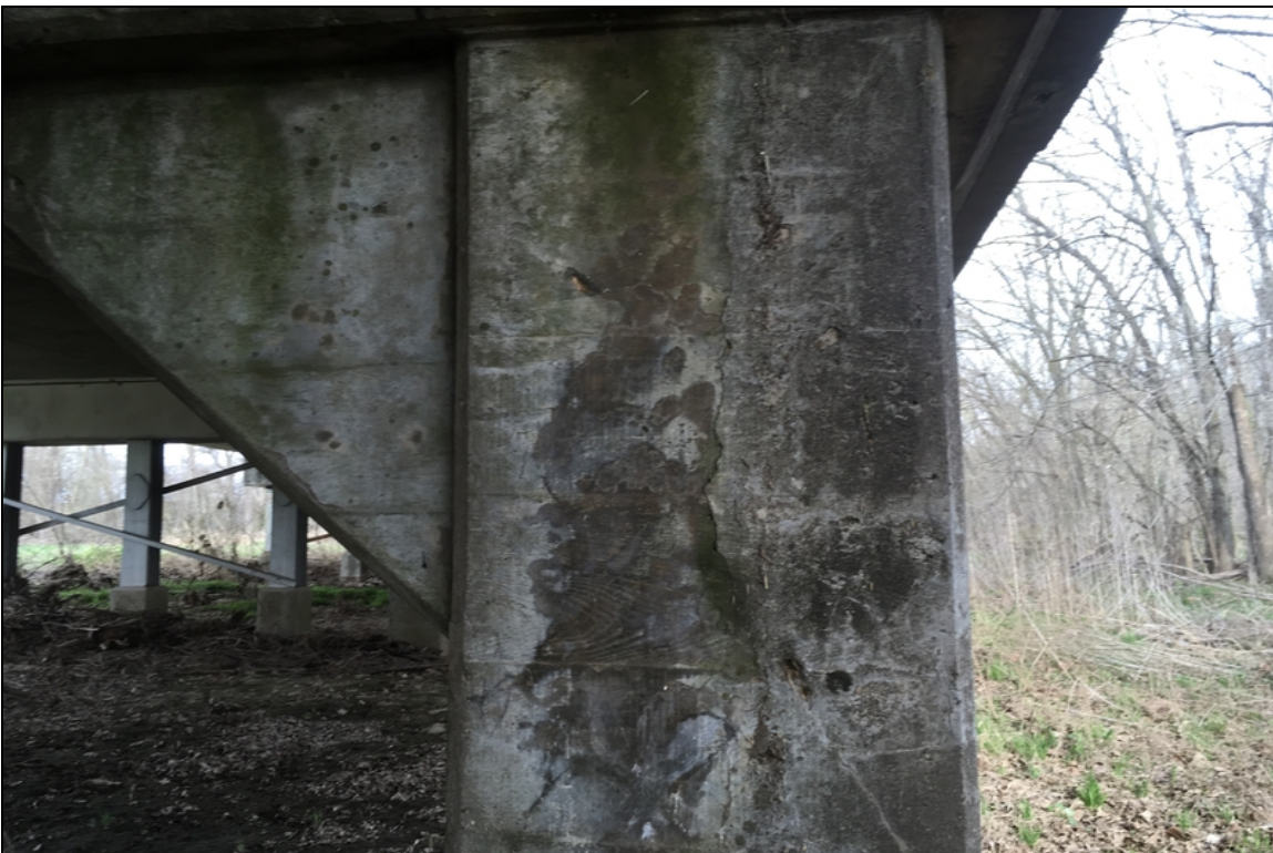
Typical cracking in the columns
