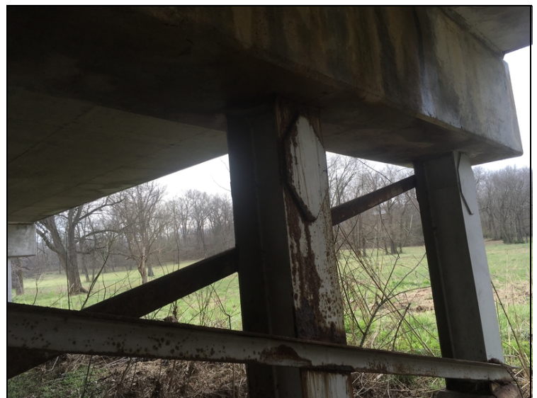
Steel piles have active corrosion with section loss
