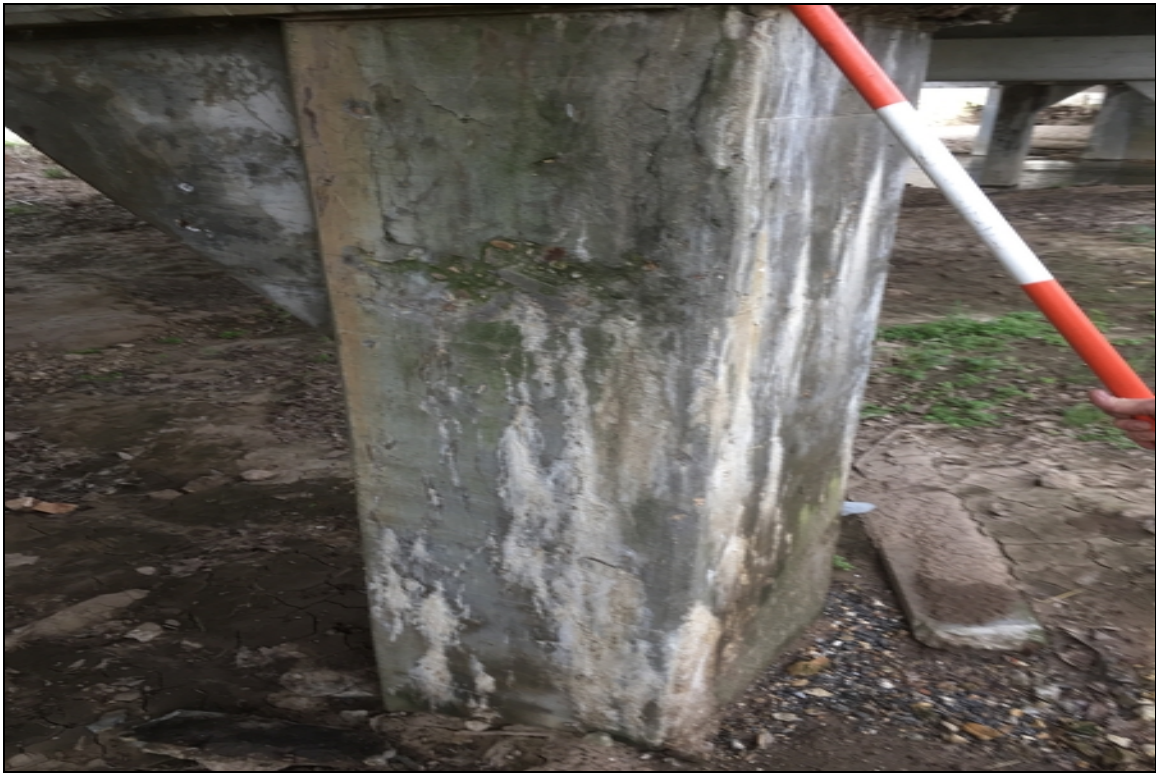
Bent 5 column 1 have cracking with efflorescence
