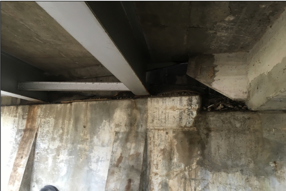
Debris accumulation on abutment 1
