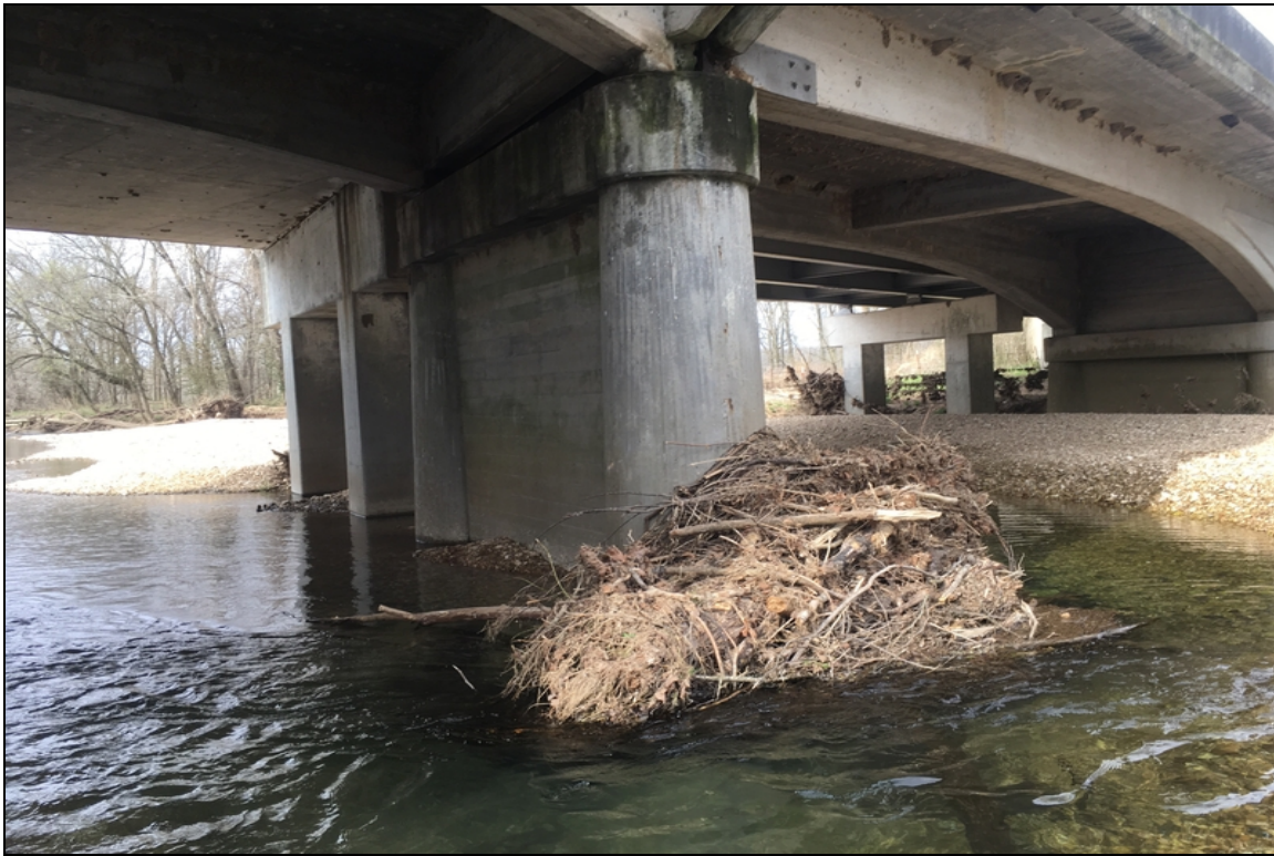
Pier 2 has drift accumulation
