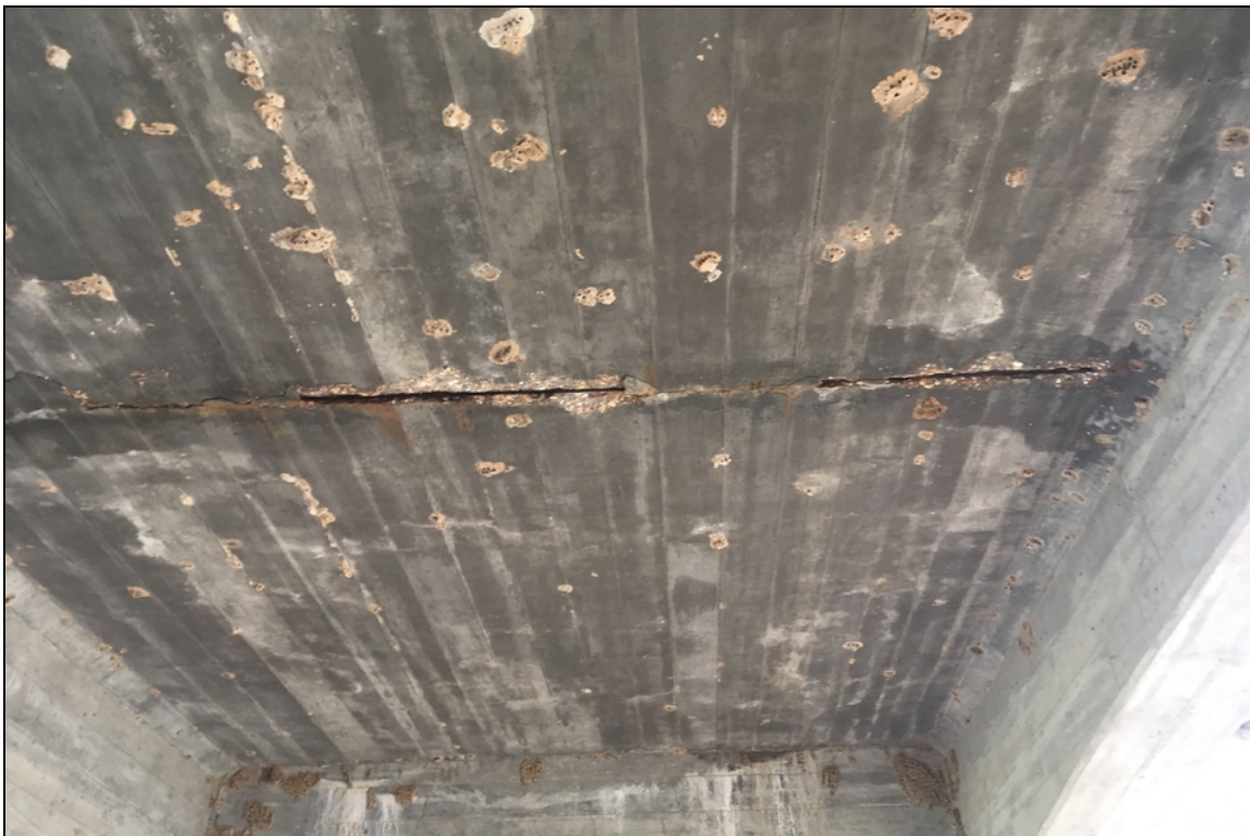
Spalling with exposed reinforcing steel in span 9
