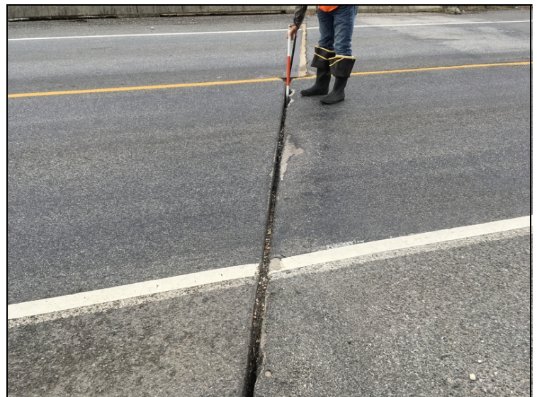
Abutment 1 pourable joint Seal is missing allowing dirt and debris on top of bridge seat
