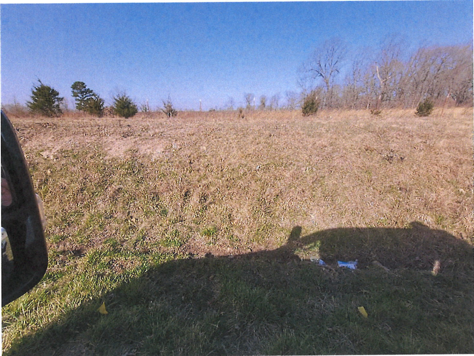
Existing cut slope near Station 138+00 north side of road.
