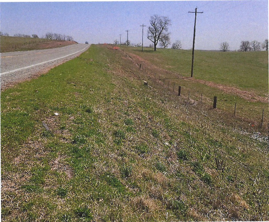
Existing embankment slope near Station 118+00 looking east.
