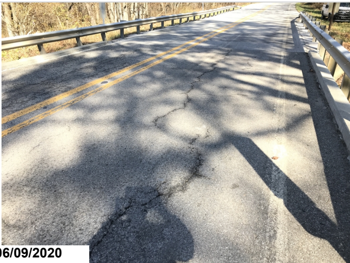
Cracking in the north bound lanes wearing surface
