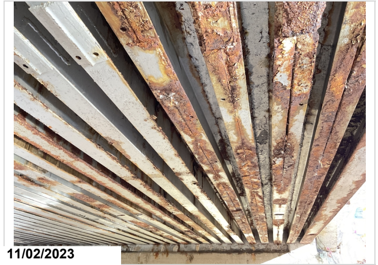
Flaking rust and section loss to girders on east side of bridge
