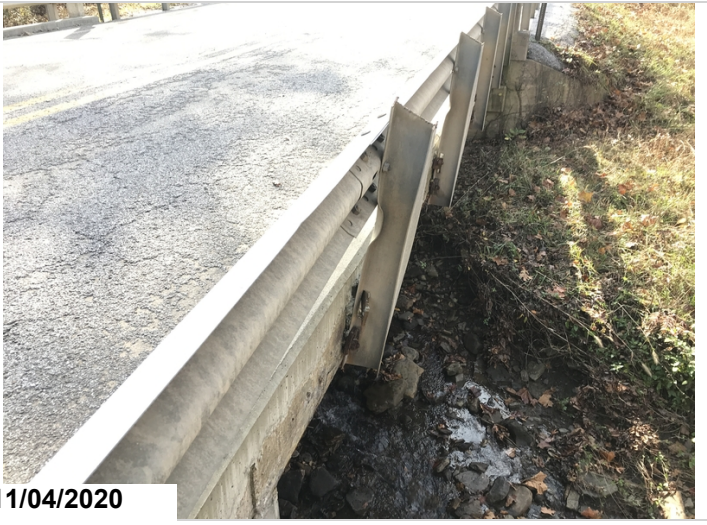
Railing left adjacent abutment #2 minor collision damage.
