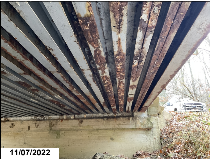
View of girders with flaking rust
