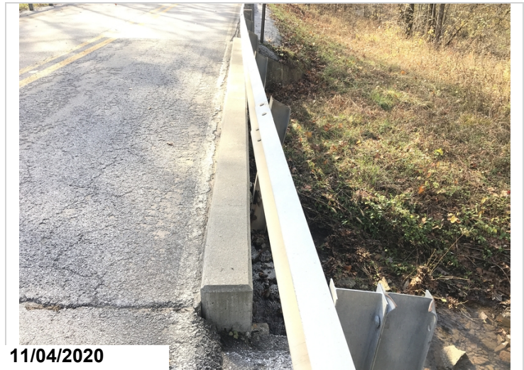
Railing left adjacent abutment #2 minor collision damage.
