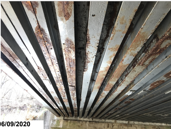
View of active corrosion to girders typical for right side of structure
