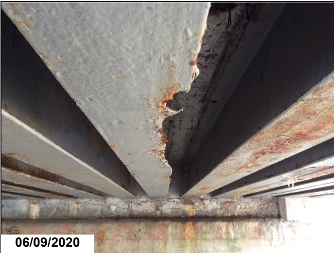
Girder #28-Section loss to bottom flange.
