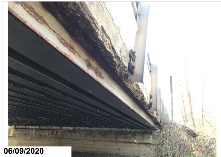
Left side of deck in overhang area spalling that exposes the top flange of girder.
