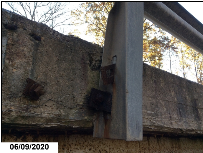
Bent 2 left - bridge rail anchorage is loose.
