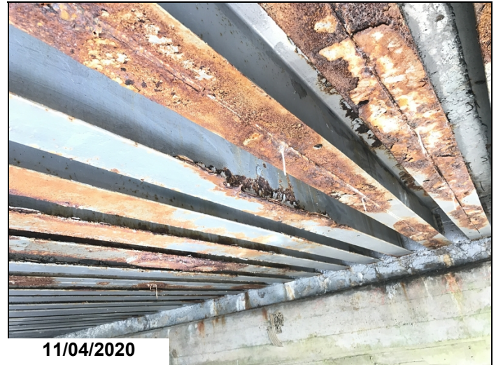
Girder #28 has significant section loss to the bottom flange
