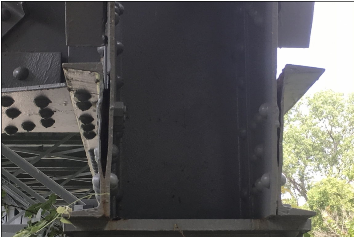
Truss end connection at L 21 left truss showing distortion. Typical of all 4 lower locations at the beginning and end of the trusses.
