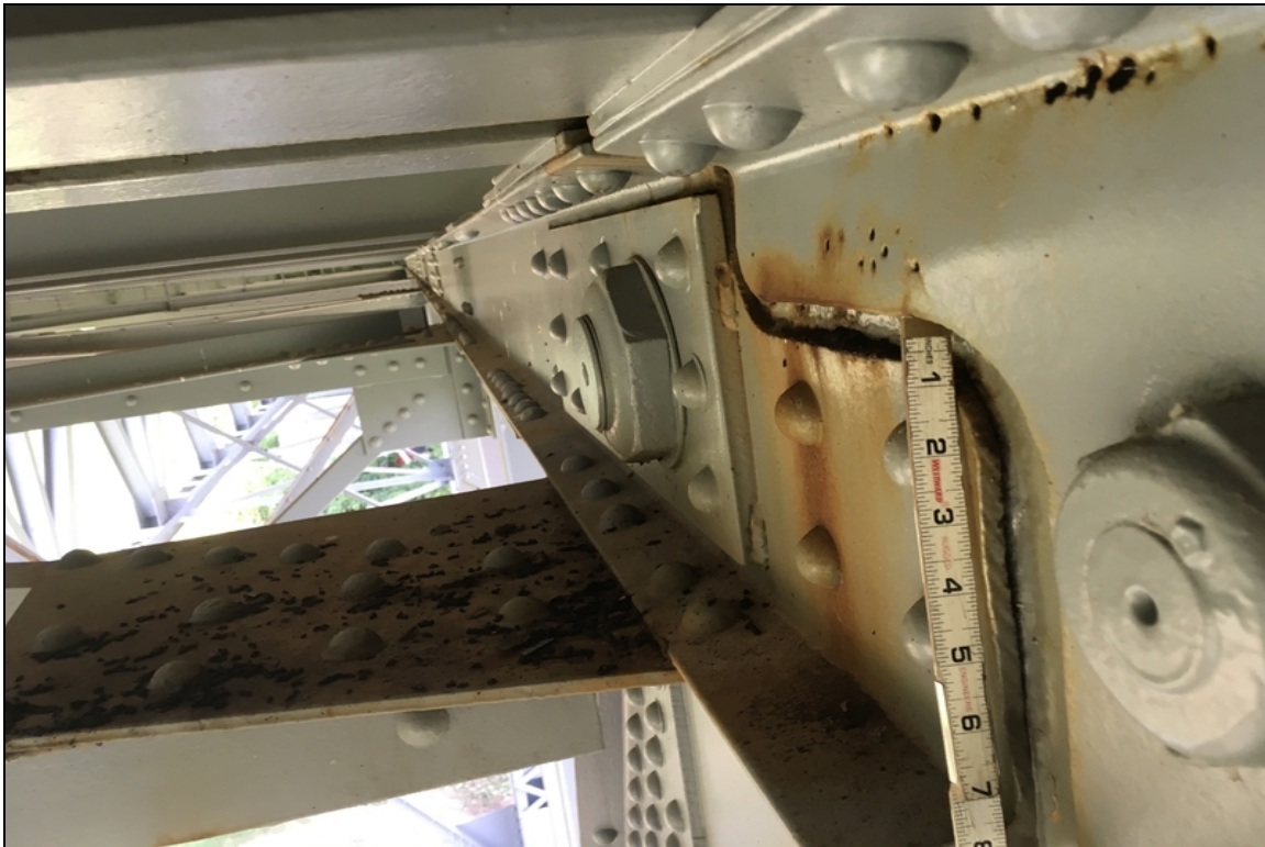
U16 connection on the interior left truss is distorted and bulging due to pack rust. The web has rust holes at this location on the interior and exterior top chord connection.
