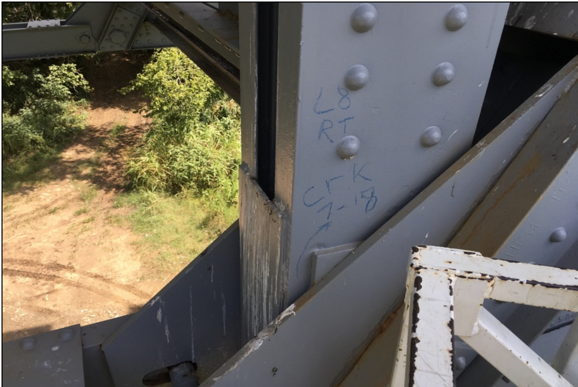
Crack location L8 right truss.
