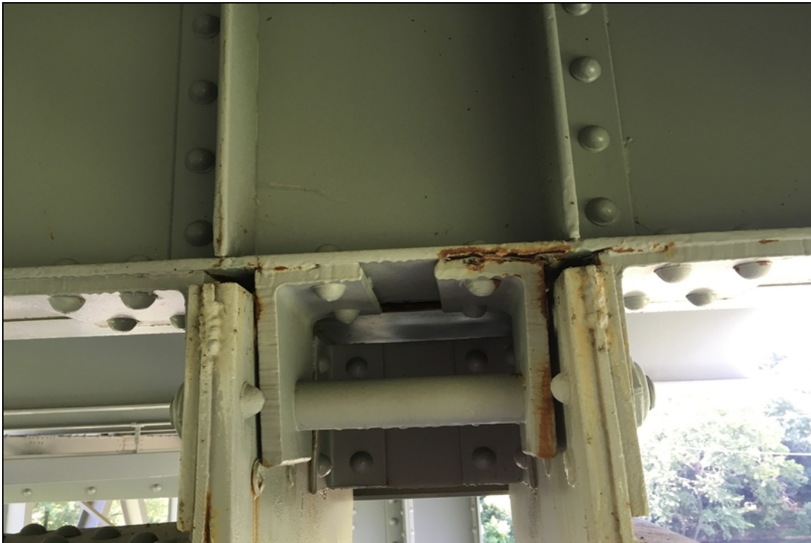
Right truss upper beginning pin condition.
