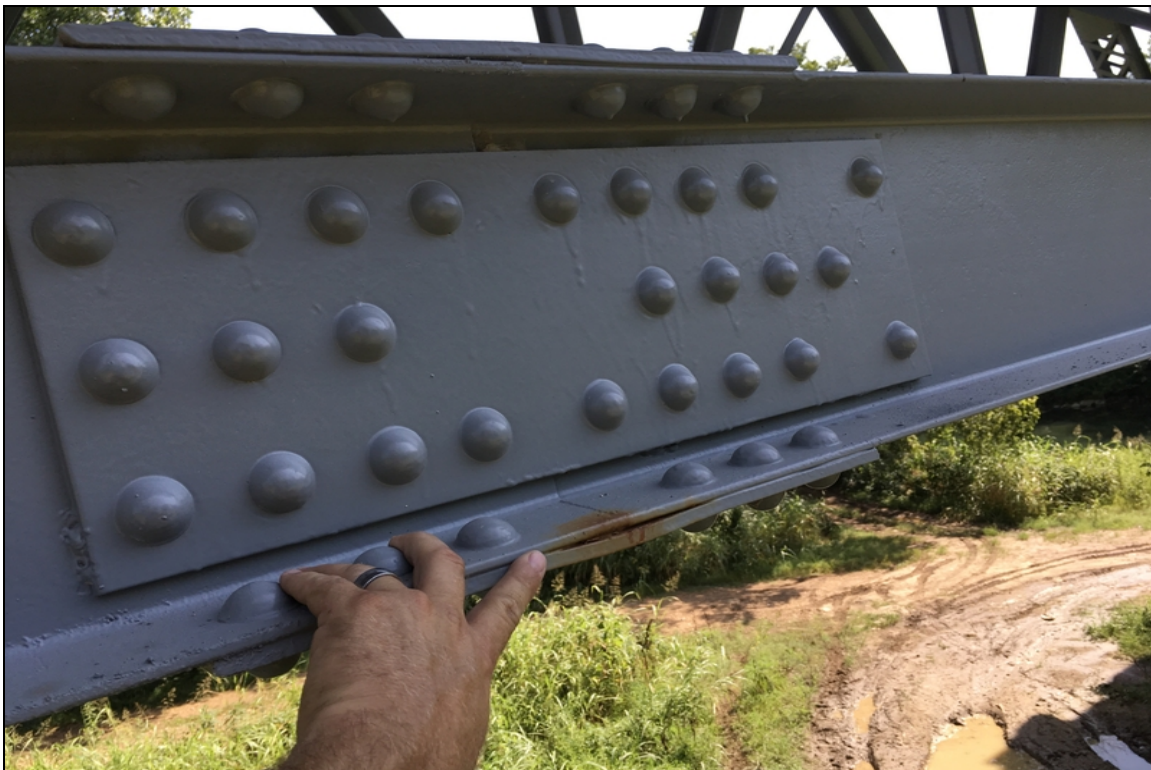
Corrosion with 3/16" distortion on the bottom batten plate of the right truss at L3 right truss.
