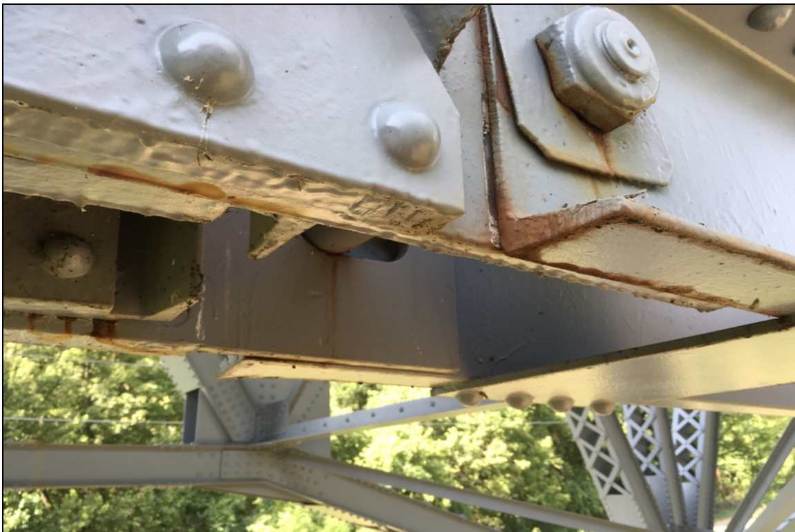
Lower pin area condition at L8 left truss.
