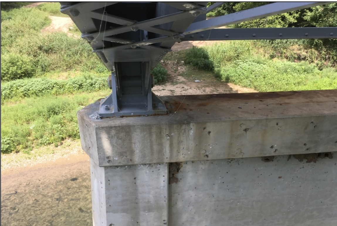
Bearing condition at pier #3 typical of both at this location.
