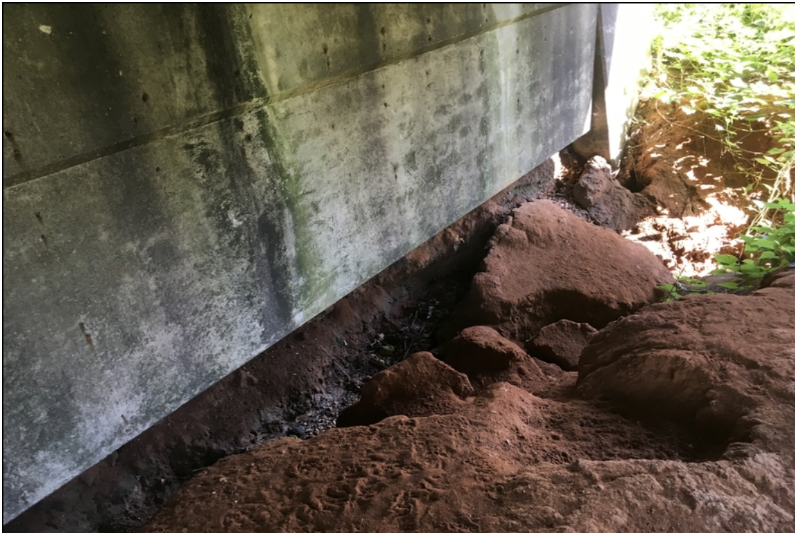
Embankment erosion at abutment #1 that extends under the web wall of the abutment.
