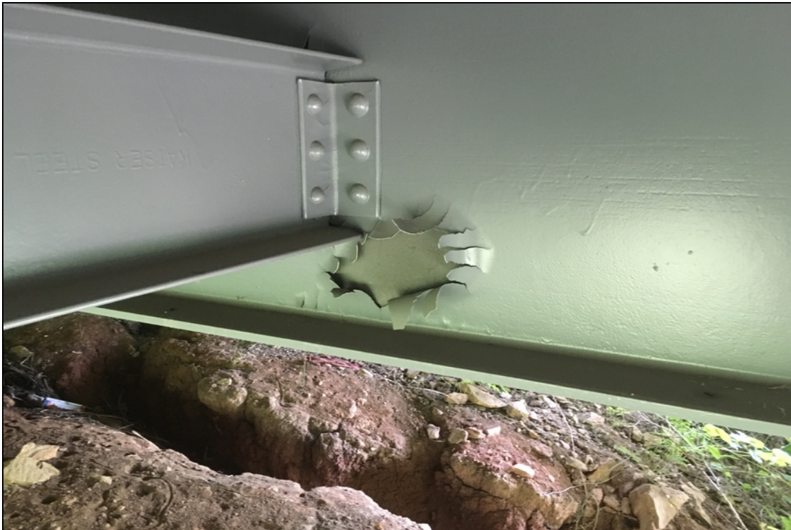
Paint has lost adhesion in span #6 on all 5 beams in the same location near mid span.
