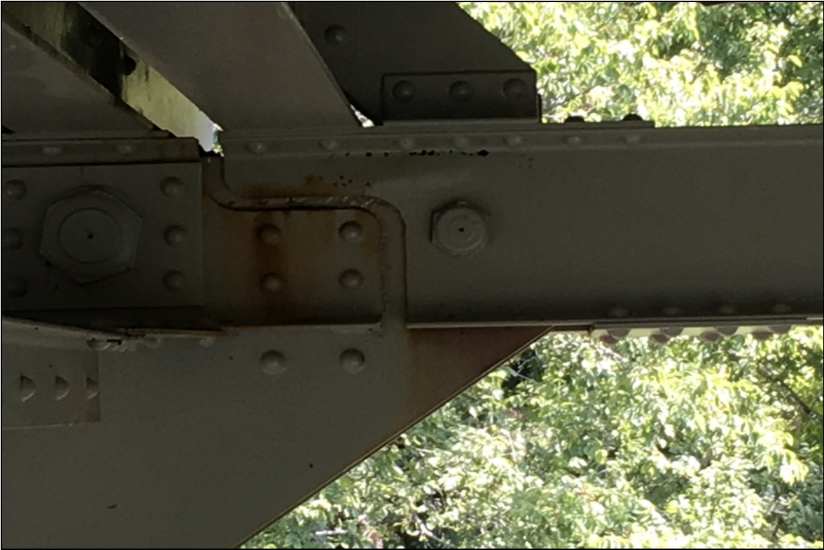
Rust holes on the interior top chord connection at U16 left truss.
