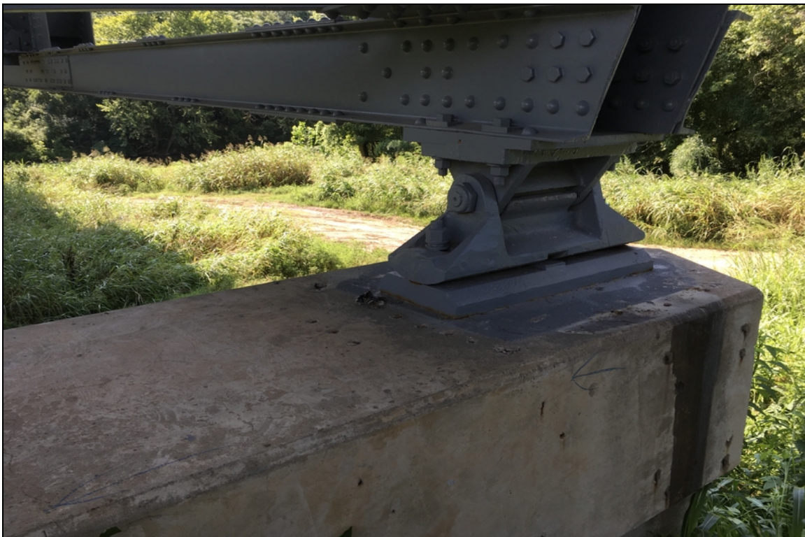
Pier #1 bearing condition typical of both at this location.
