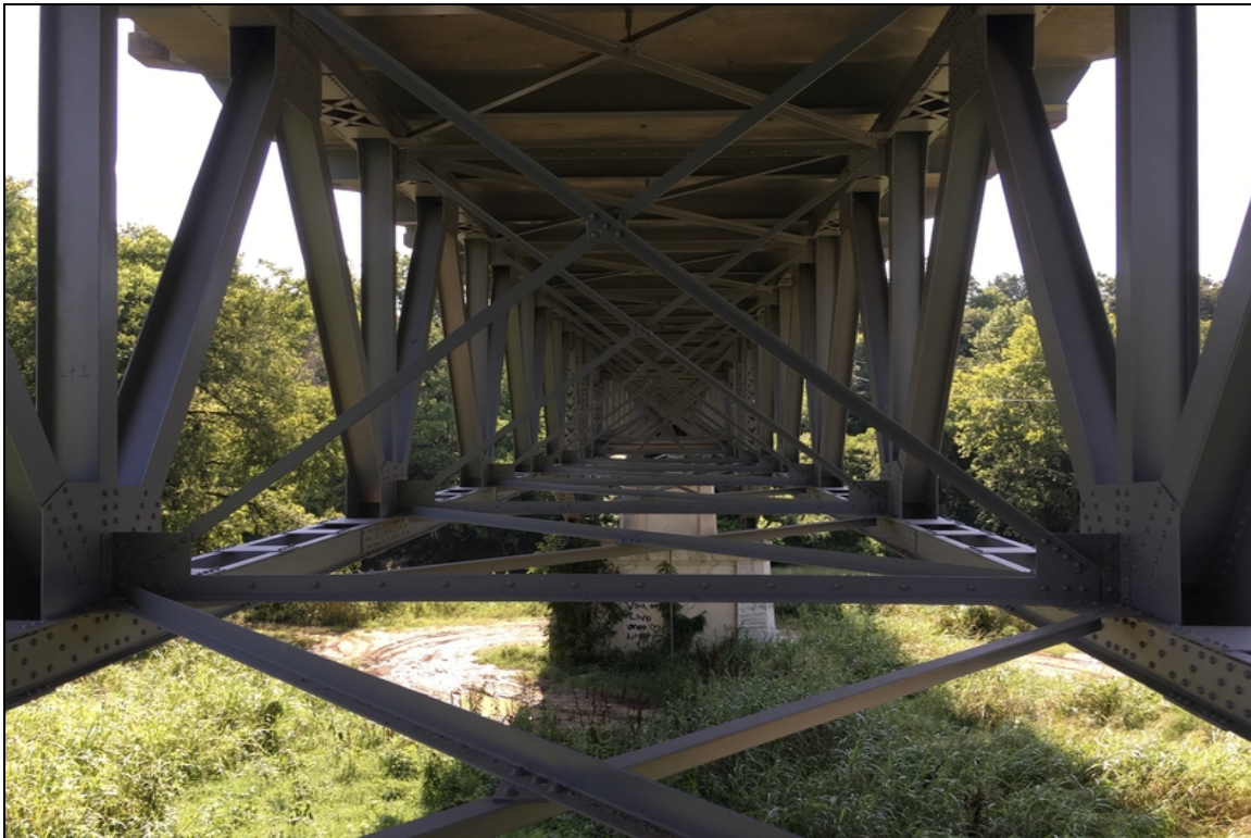
View of the paint condition of the truss spans. Typical.
