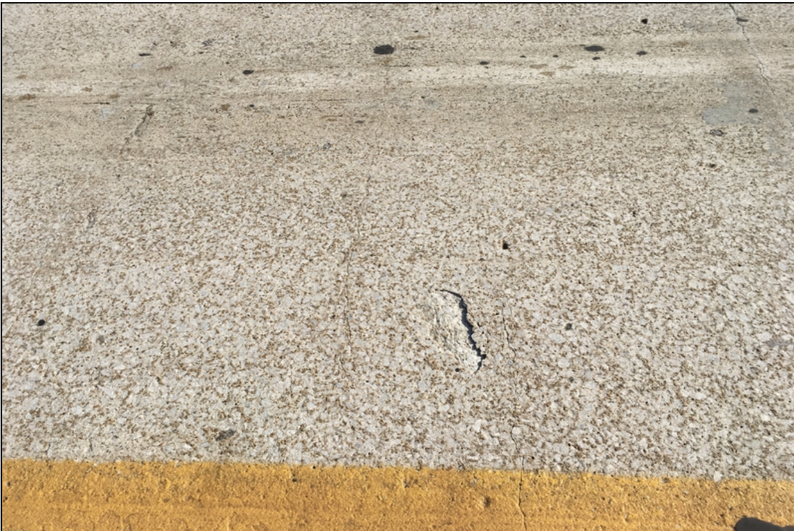
Driving surface showing delamination and cracking.
