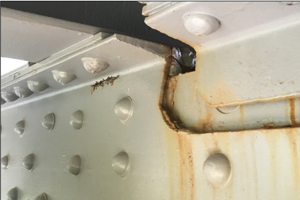
3" long rust hole on the web of the interior upper chord connection at U26 right truss.
