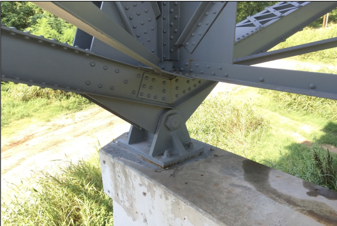
Bearing condition at pier #2. Typical of both at this location.
