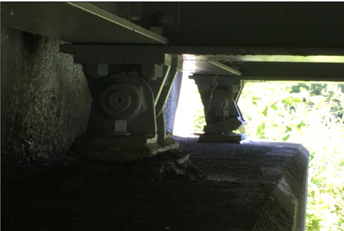
Excessive tilt of bearing #1 at abutment #1. One anchor bolt is missing.
