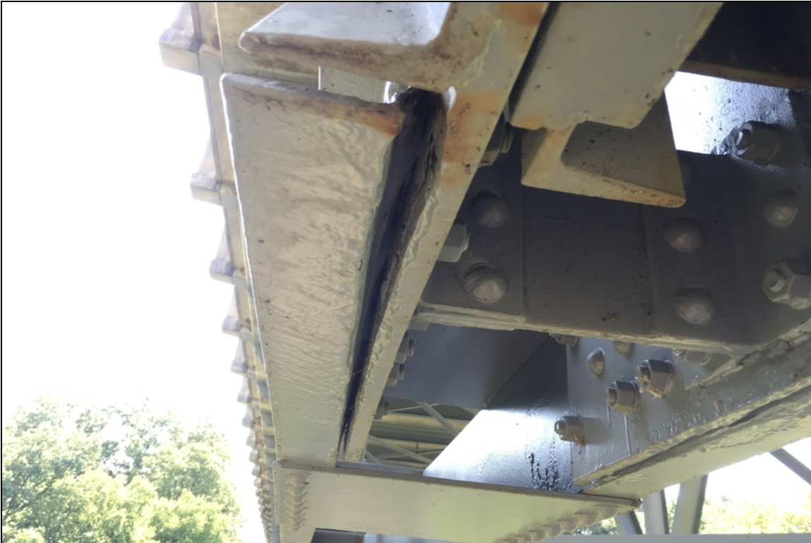
Pack rust with 1" of distortion on the bottom chord at L8 left truss on the exterior connection. This condition is also typical of the right bottom chord at the same location.
