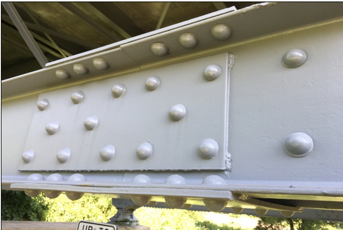
Numerous Tack welds on the splice plate at L1. Typical of the left and right sides.
