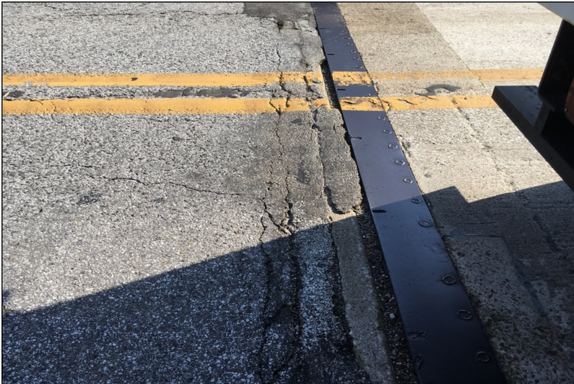
Sliding plate condition at abutment #1.
