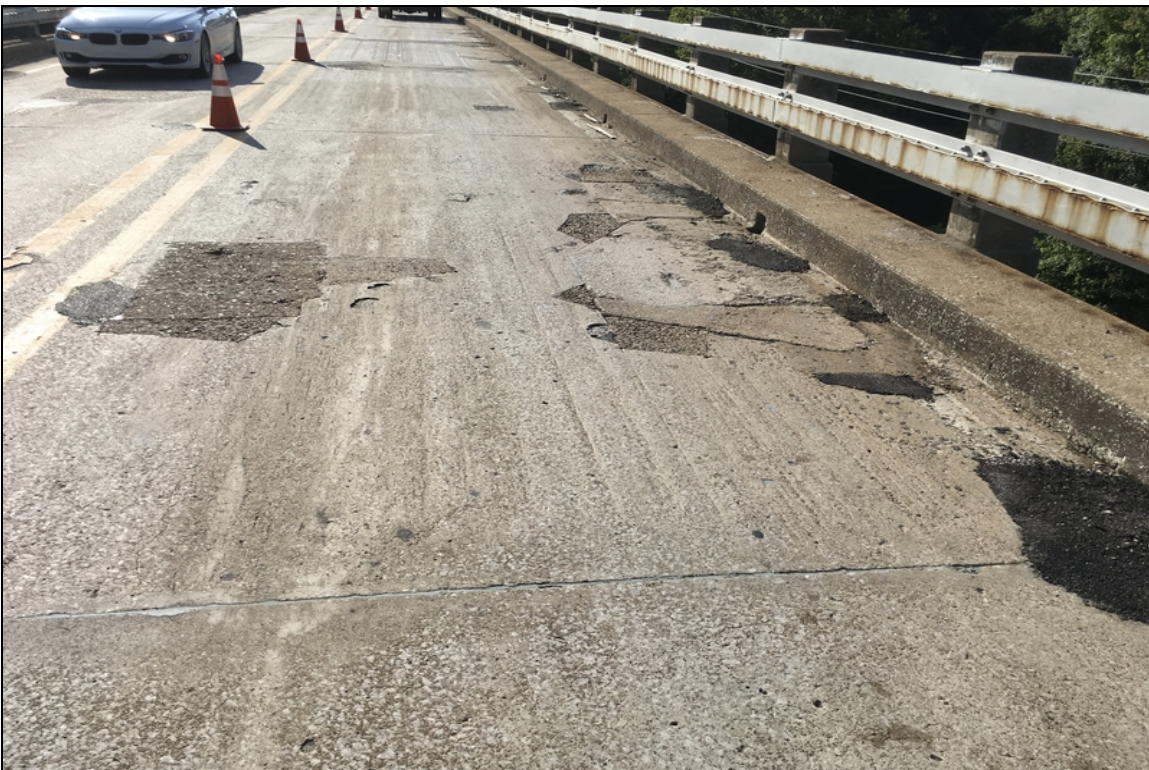
Driving surface showing patched areas in the gutter lines.
