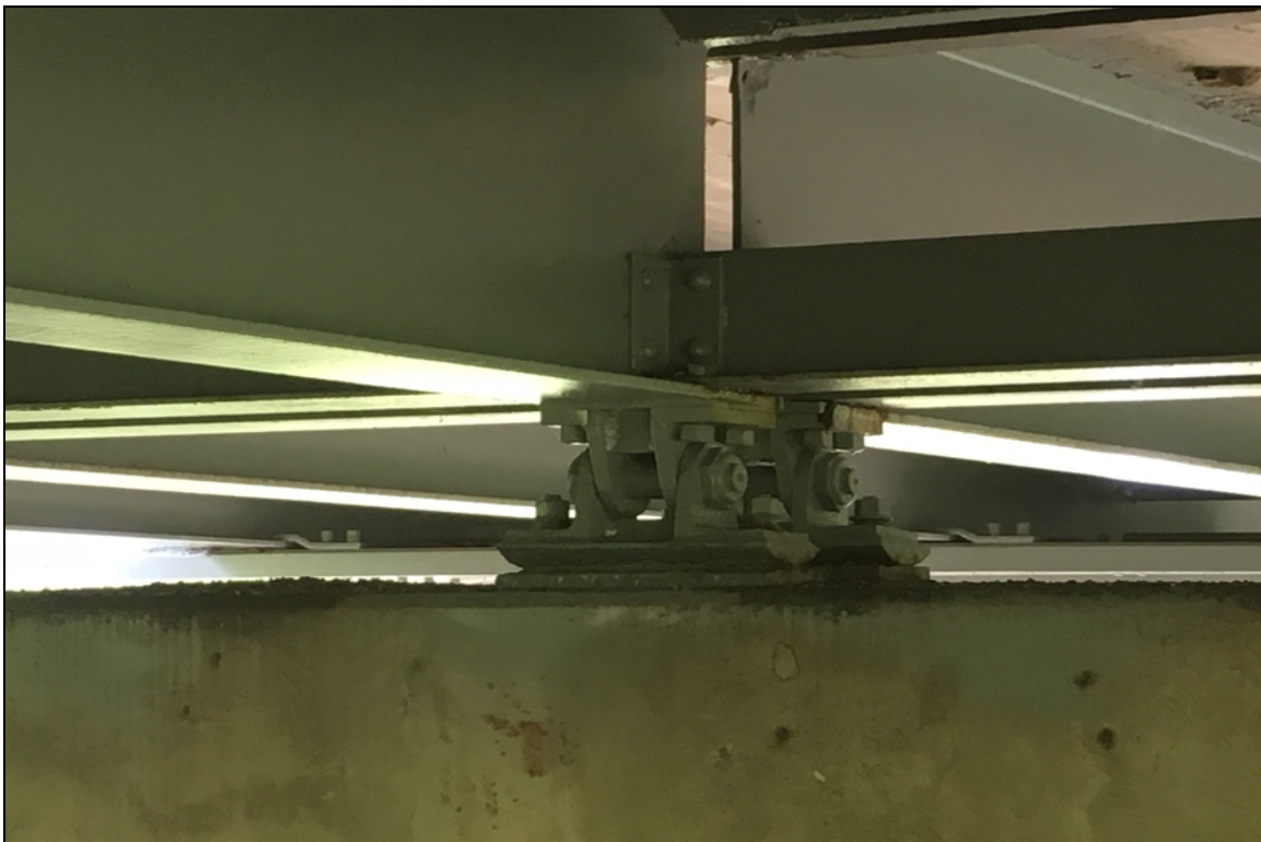
Bearing condition at pier #5. Typical of all 10 at this location.
