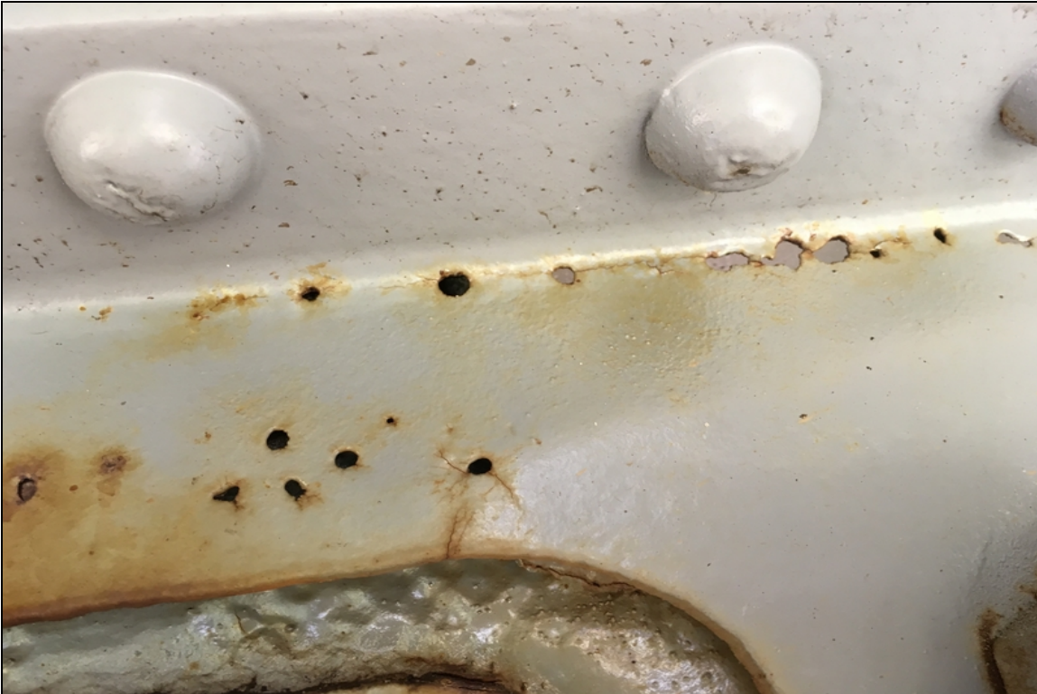
U16 left truss interior top chord connection has rust holes that appear to be cracking. This area is next to the upper pin location.
