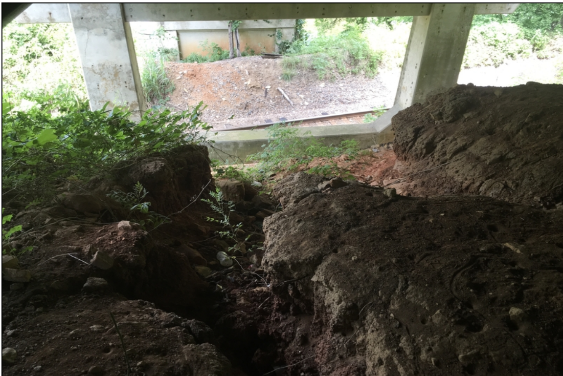
The abutment #2 embankment has erosion.
