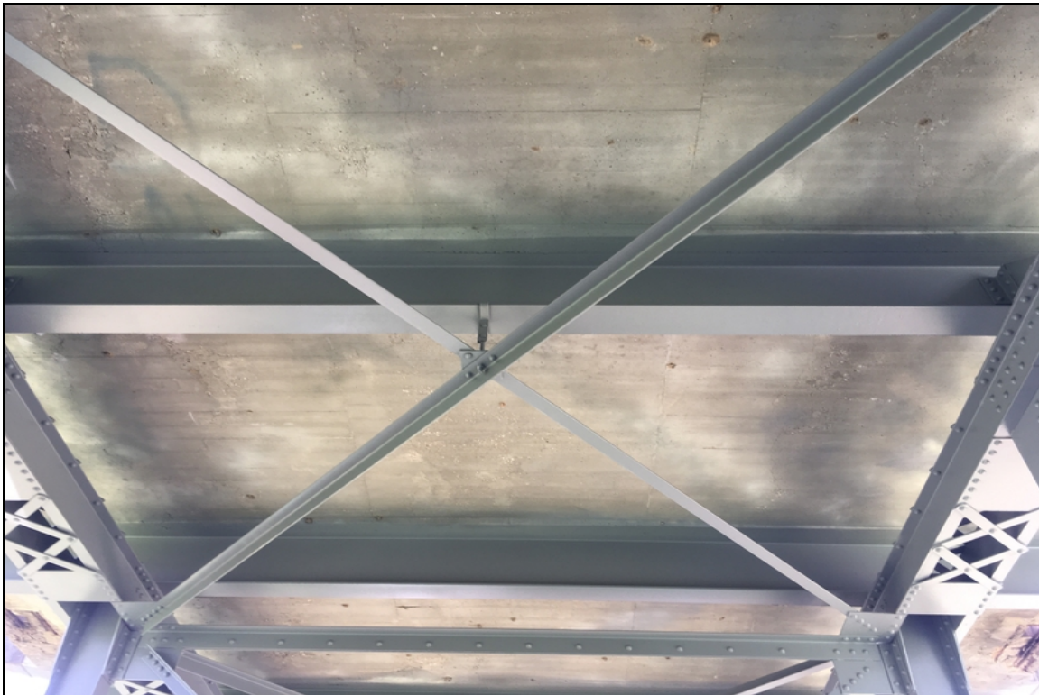
Undersurface condition in the truss spans.
