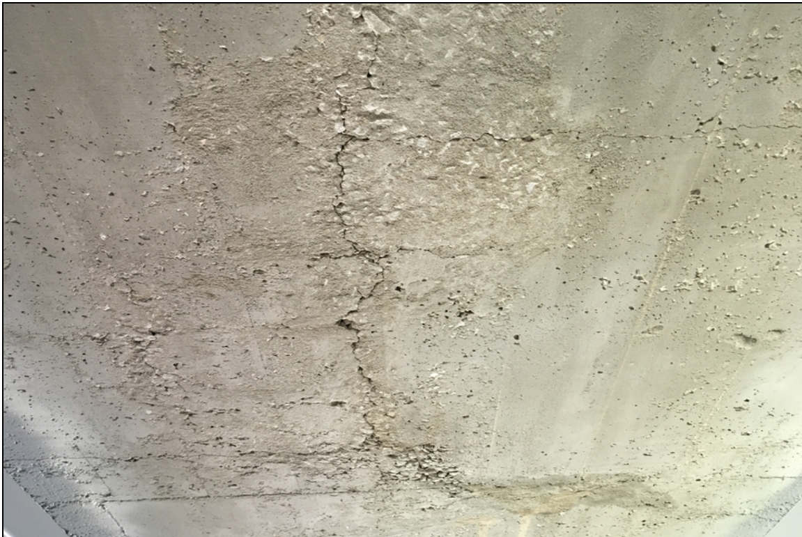
Deck undersurface condition showing cracking. Typical.
