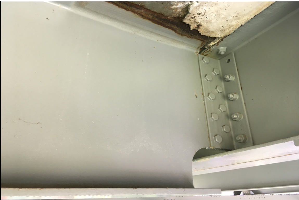
Bolt missing at beam #4 connection at the end of span #1. Typical of beams 2,3,4 at the same location.
