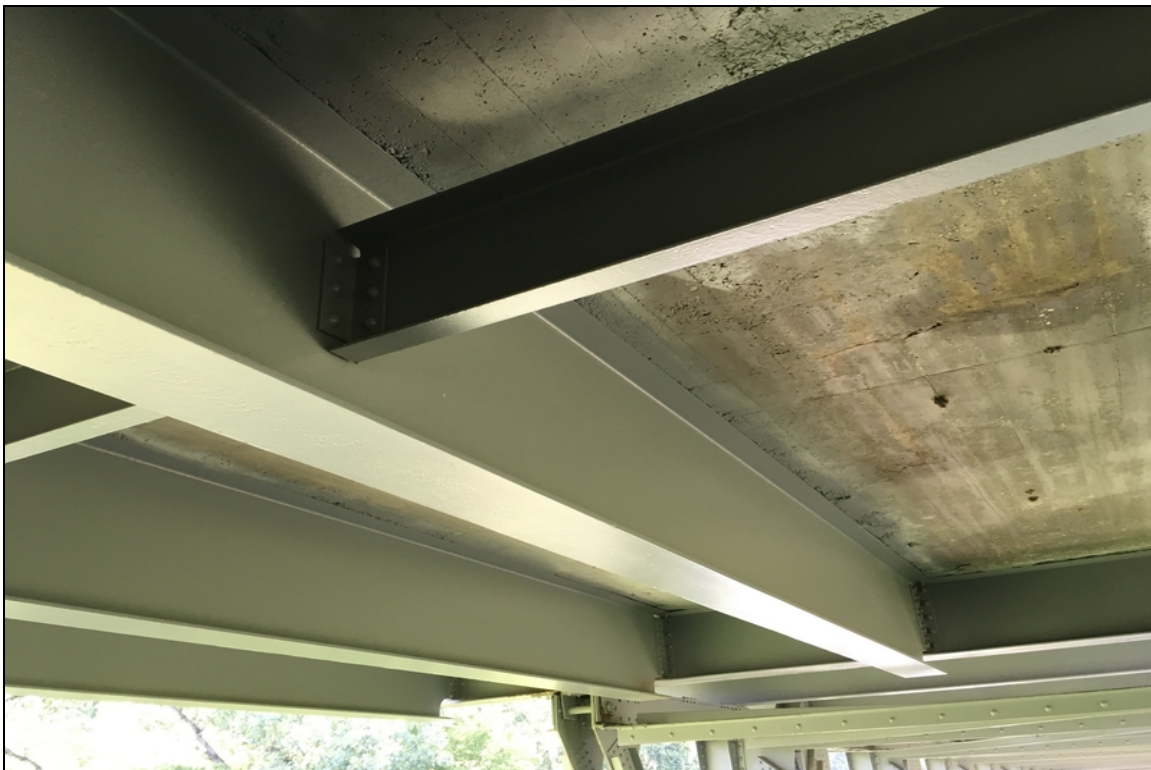
Typical paint condition of the multi beam spans.
