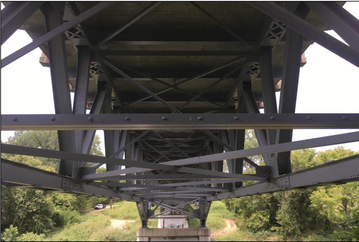
View of the fracture critical elements.
