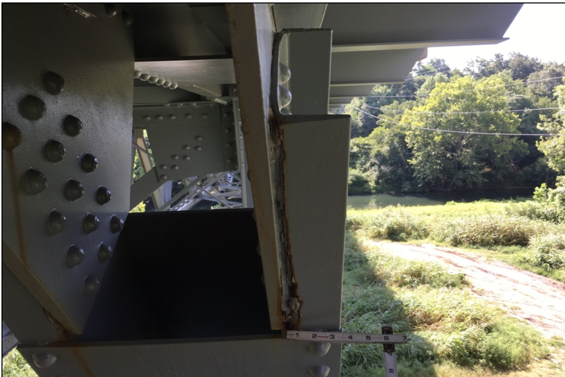
The upper connection of the exterior diagonal member at the beginning of the right truss. Showing pack rust with 1/2" of distortion.
