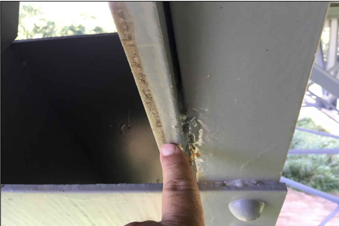
Cracked tack weld at the upper end of the beginning diagonal of the left truss. Typical of the left and right side of the left truss. This is typical is several locations throughout the structure, the cracking is not affecting the base metal.
