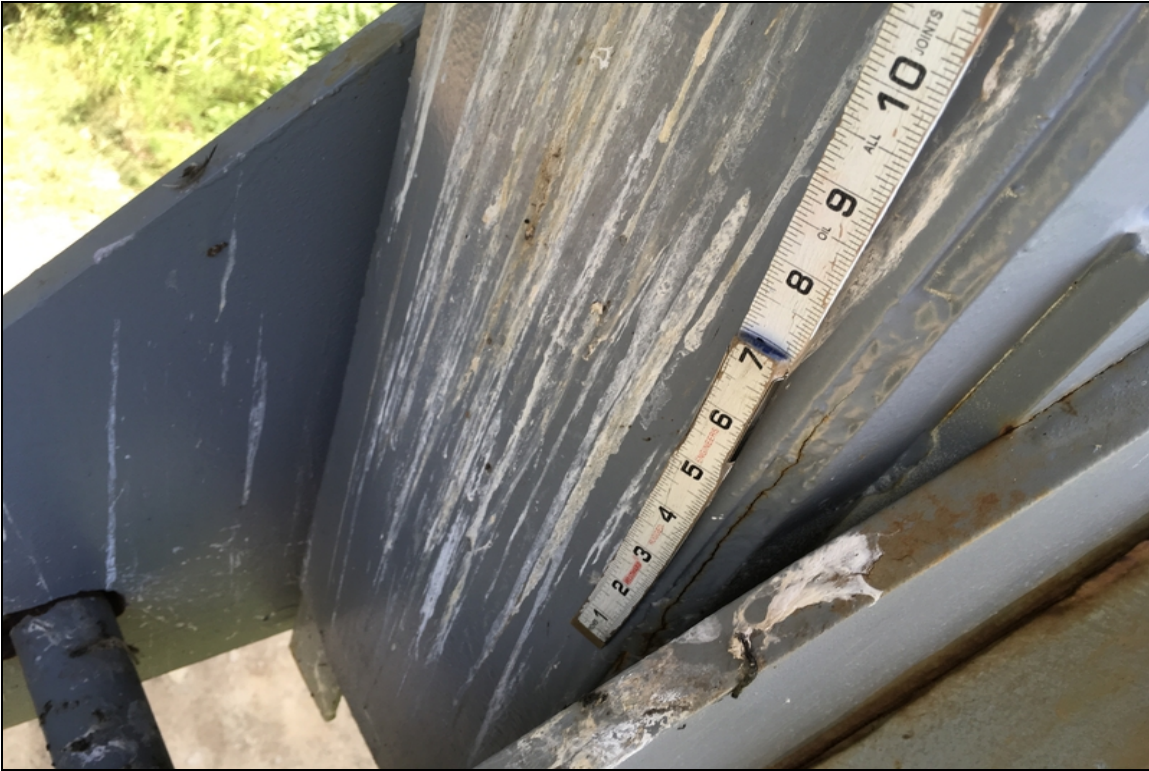
8" long vertical crack in the weld at the L 8 vertical member in the batten plate. This crack could extend into the vertical member.
