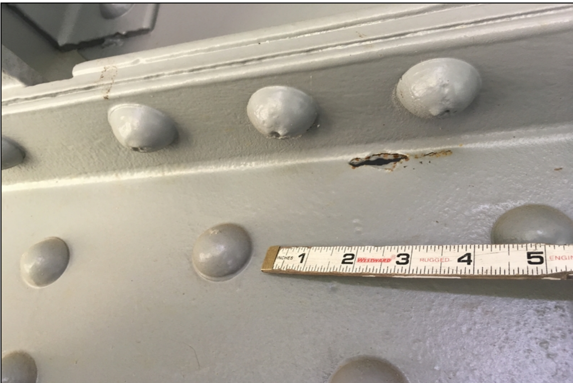
2 " long rust hole at the top of the web of the top chord on the interior connection at U26 left truss.
