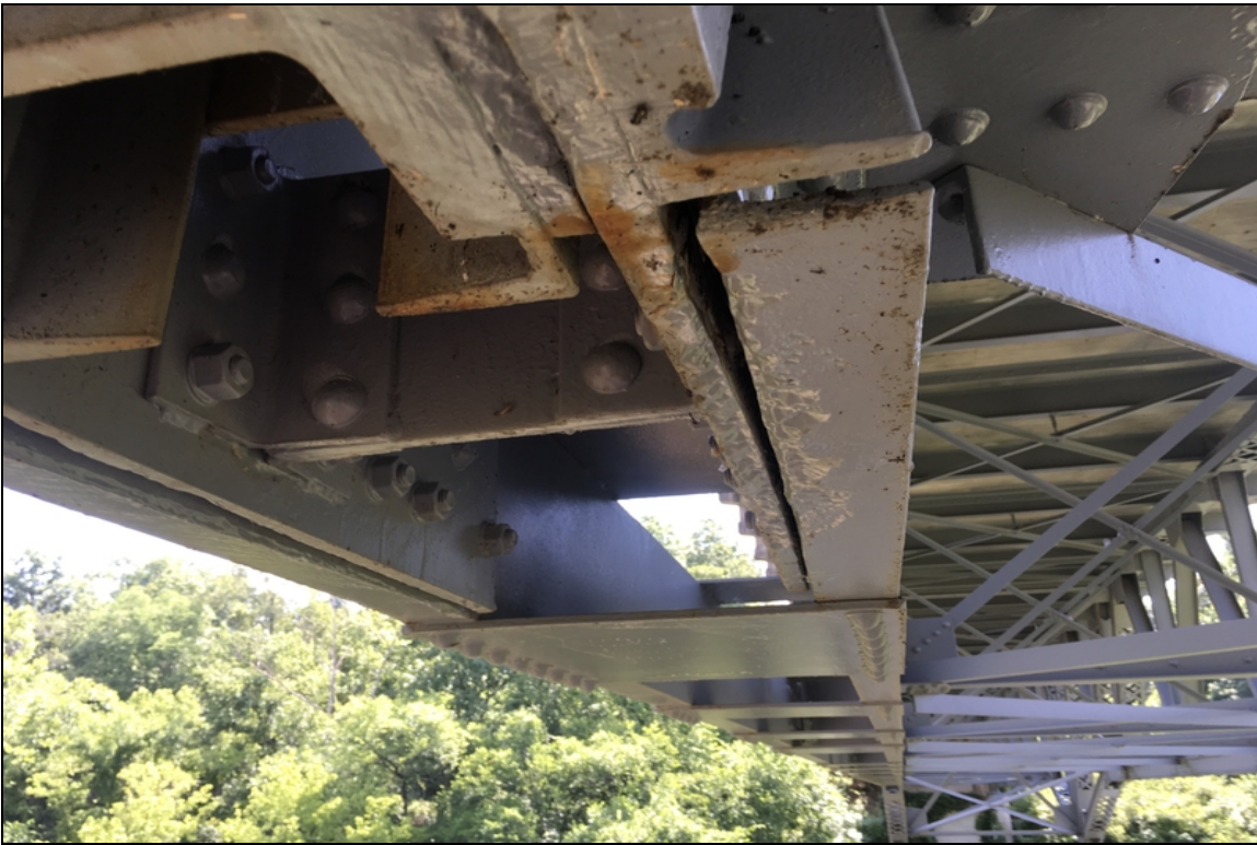
Pack rust with 1/2" of distortion on the interior lower chord connection at L8 It truss.
