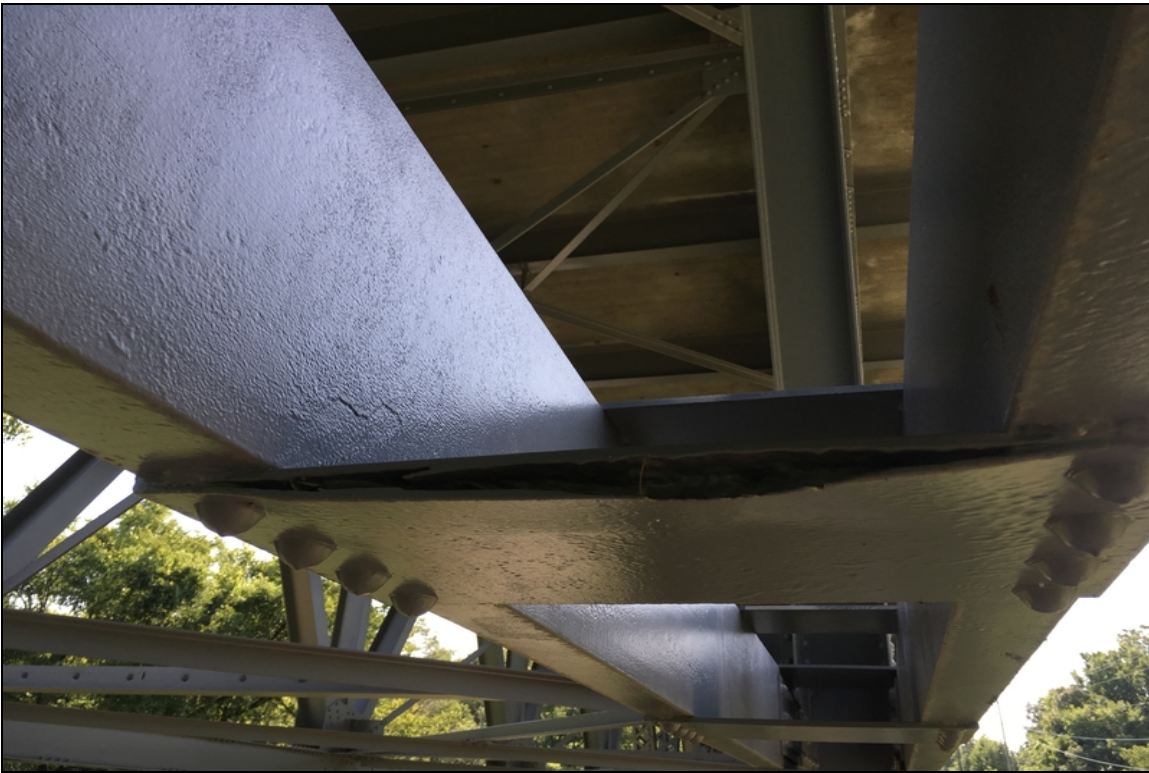
Laminar separation between a single plate just in front of L1 right truss bottom chord.
