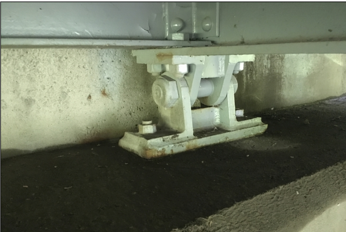
Bearing condition at abutment #2. Typical of all 5 at this location.
