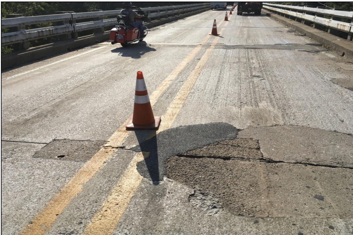
Driving surface showing patched areas at the joints.
