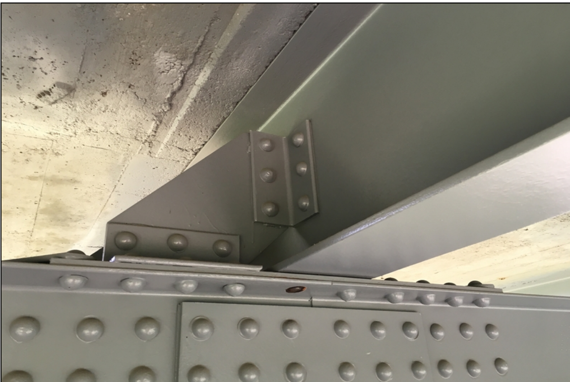
Sheared rivet at U6 left truss. The floor beam has an 1/8 gap between the bottom flange and top left chord.
