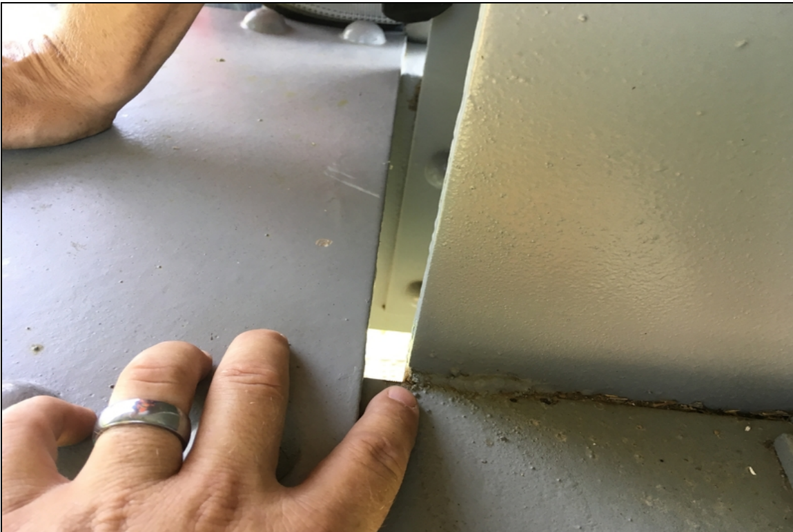
Cracked tack weld on the top of the bottom chord at L3 left truss.
