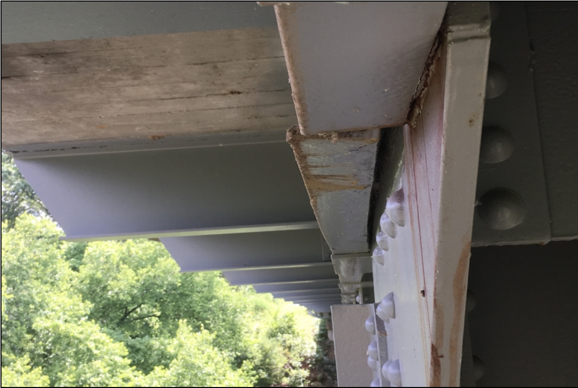
Exterior top chord connection at U 25 left truss showing pack rust with distortion on the bottom flange of the top chord.
