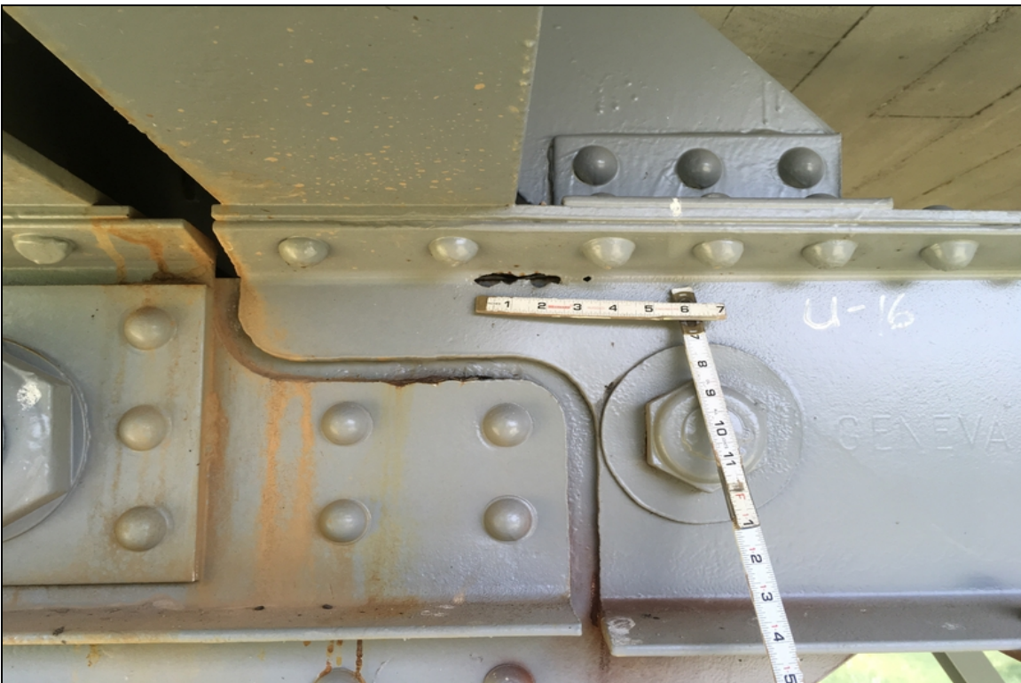
Rust holes in the web of the top chord at U16 right truss. 1/2" x 3" exterior connection. This is typical also of the interior connection at the same location.
