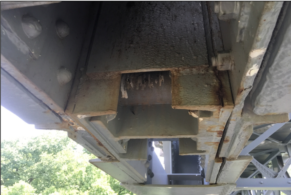
Lower pin area condition at L13 left truss.
