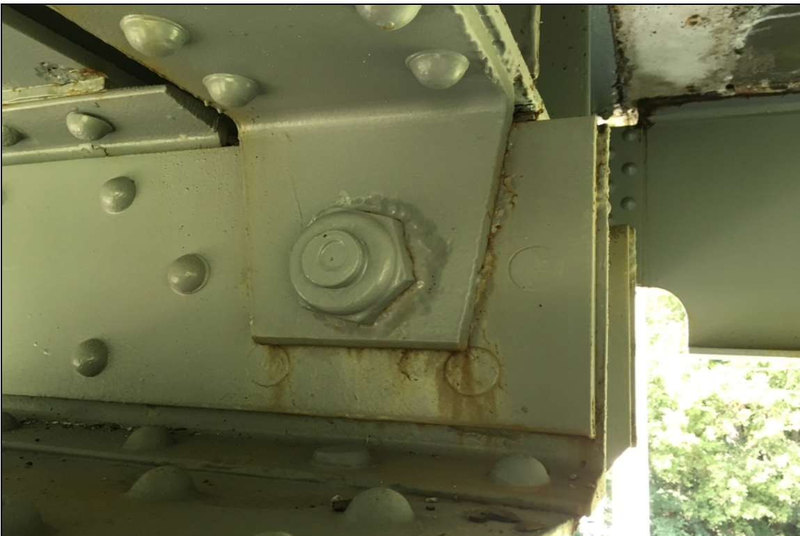
Plug welds at the upper pin location of both trusses at the beginning of the trusses.
