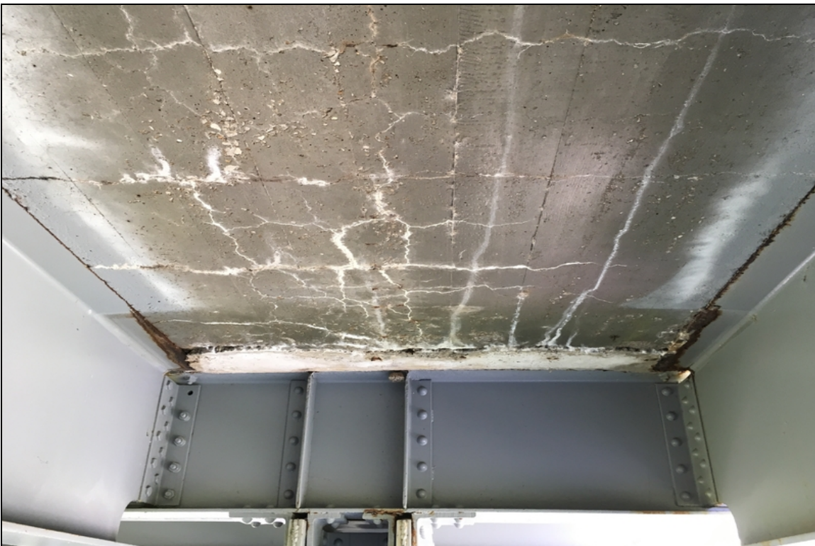
Efflorescence map cracking in bay #4 at the end of span #1. This area sounds dead under hammer blows.
