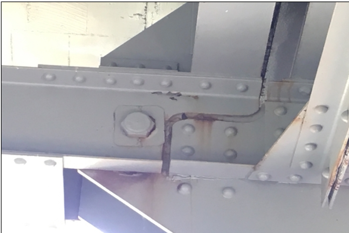
Interior connection at U16 on the right truss. Showing rust holes in the upper web.
