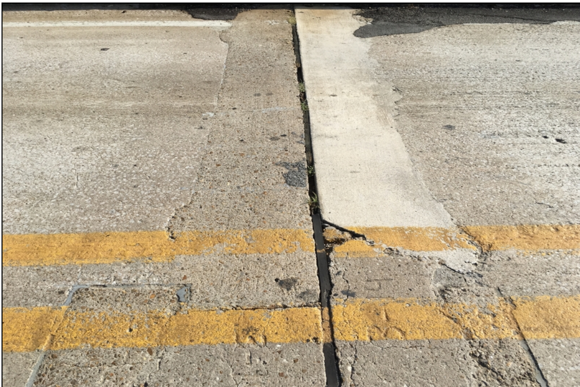
Typical joint seal condition.
