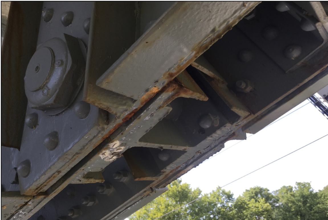
Lower pin connection area at L 13 right truss.
