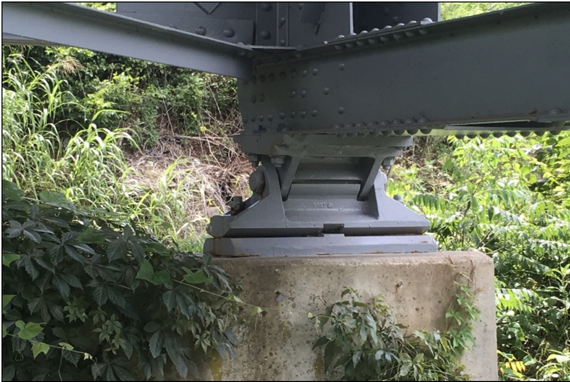
Bearing condition at pier #4. Typical of both at this location.
