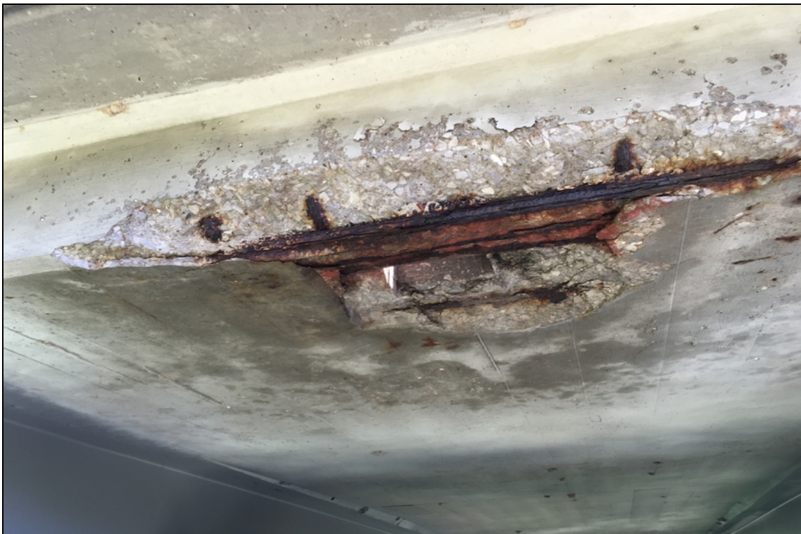
Spalls with exposed rebar at the drain areas. Typical.
