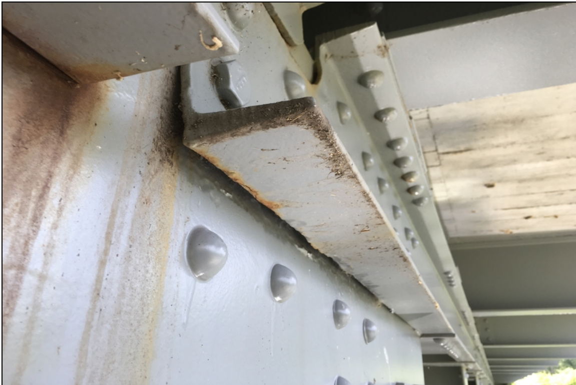
1/2" of distortion on the bottom flange of the exterior top chord connection at U26 right truss.
