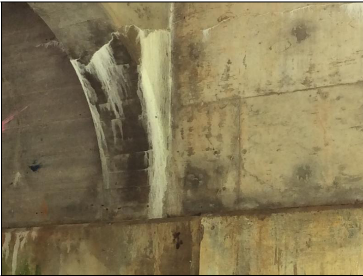
Span #1 over bent #2 efflorescence to haunch of girder #3
