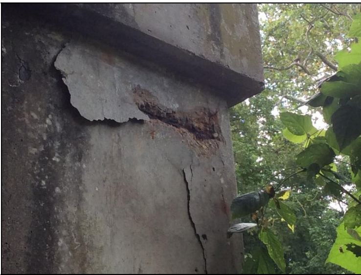
Exposed rebar to right column of bent #5
