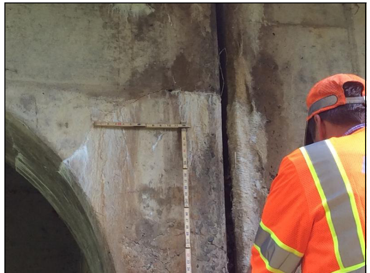
Cracking to haunch of girder #4 over bent #1
