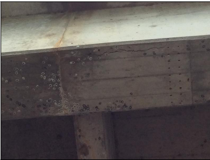
Midspan crack in girder #4 of span #3
