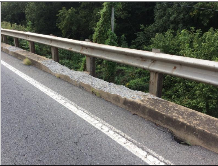
15' exposed rebar to right curb section in span #4
