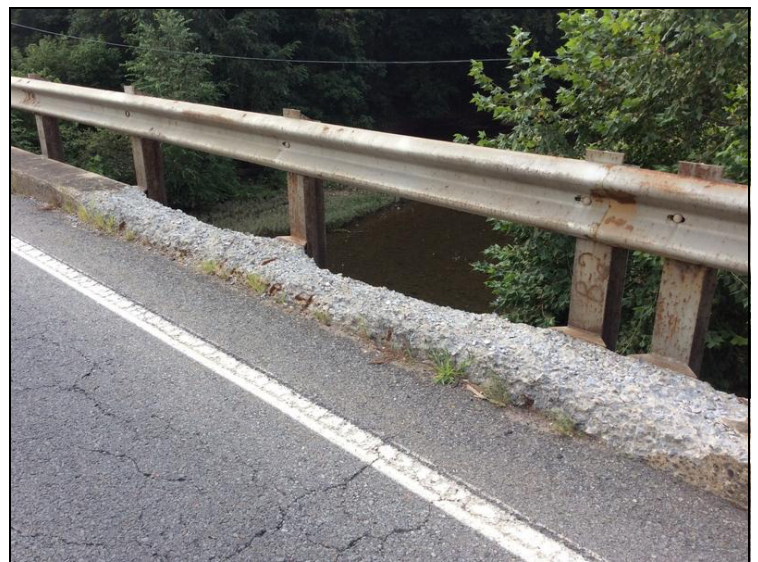
20' exposed rebar to right curb section of span #3
