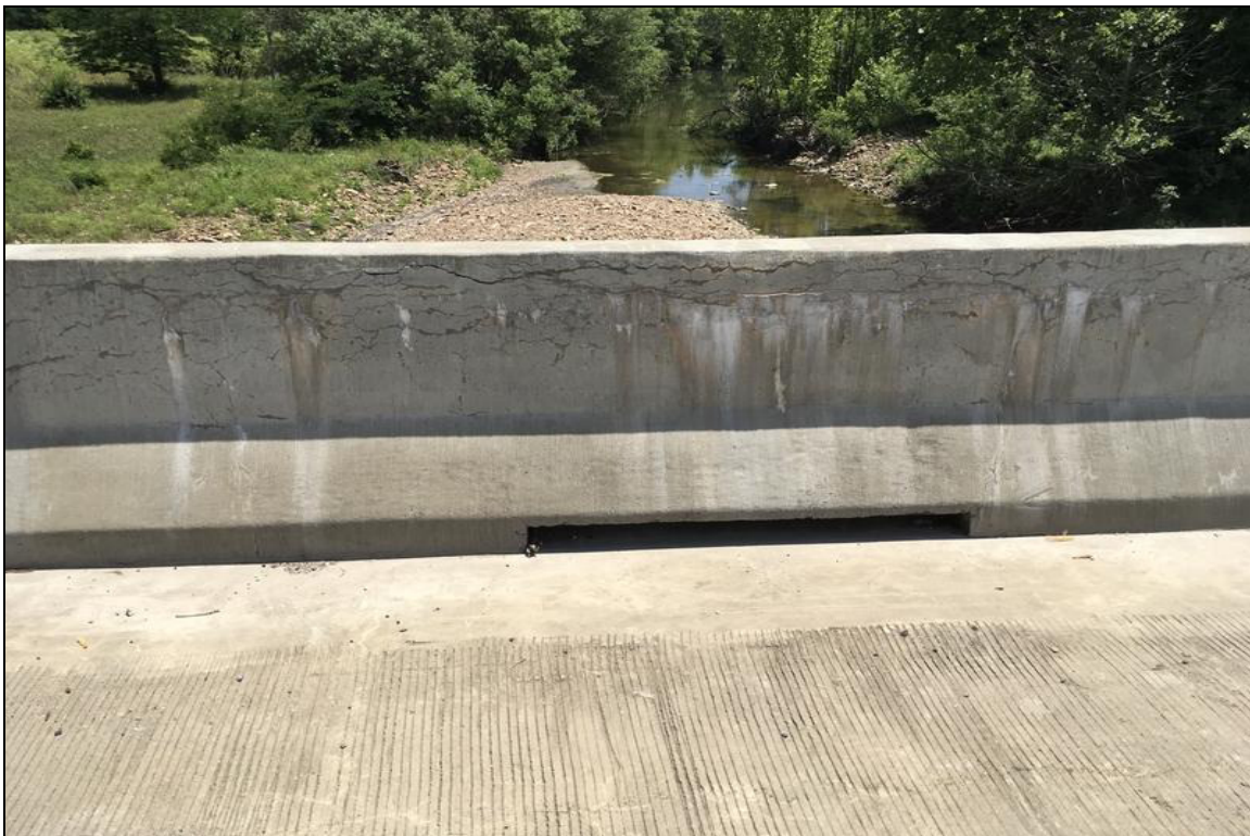
Several parapet sections on the right side have map cracking. Worst case condition.
