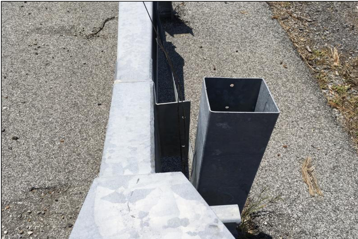
The Right beginning end treatment is not connected to the post Typical also of the Left ending end treatment is not connected to the post.
