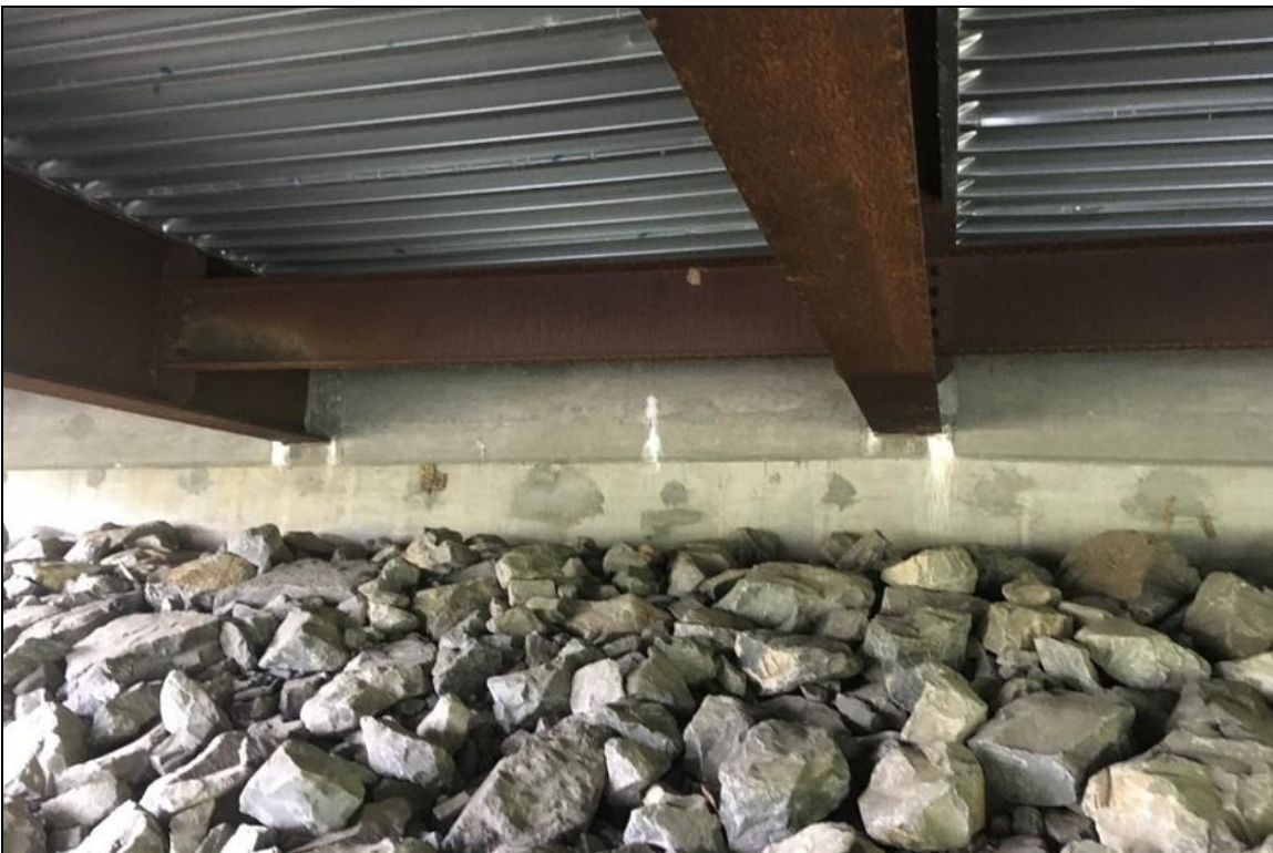
Efflorescence at the beam corners of abutment 2.
