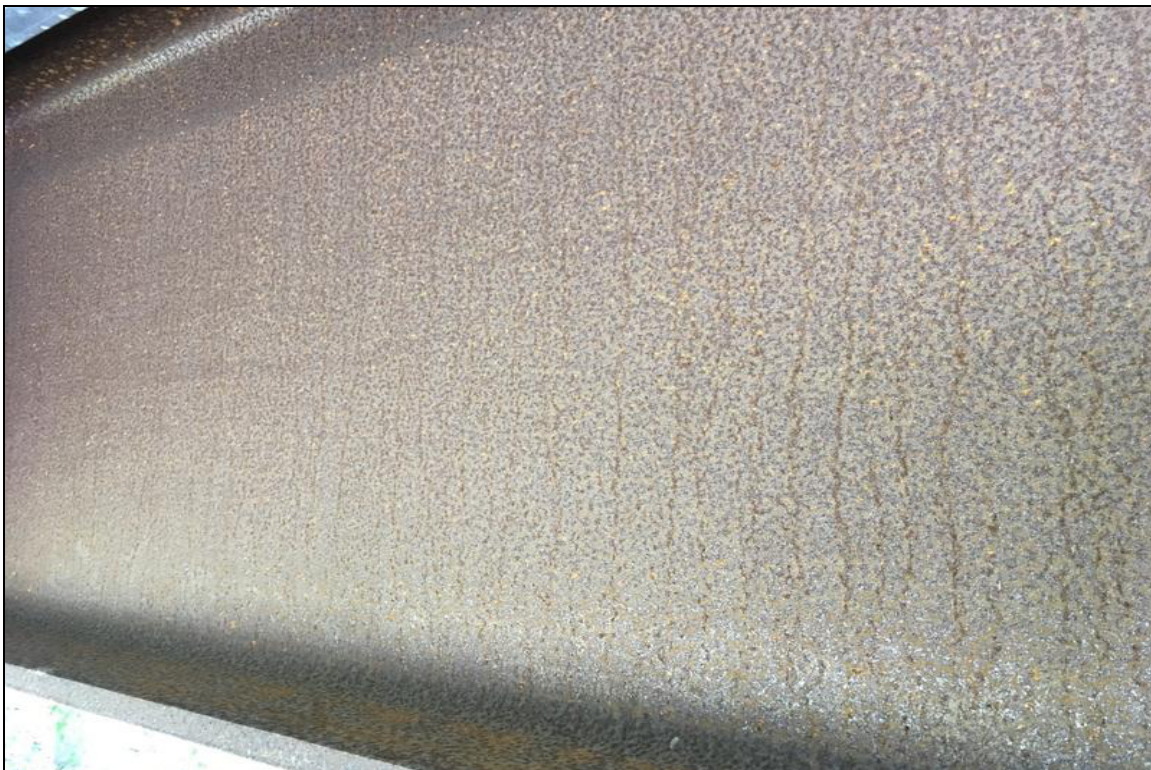
Typical condition of the weathering steel protective coating.
