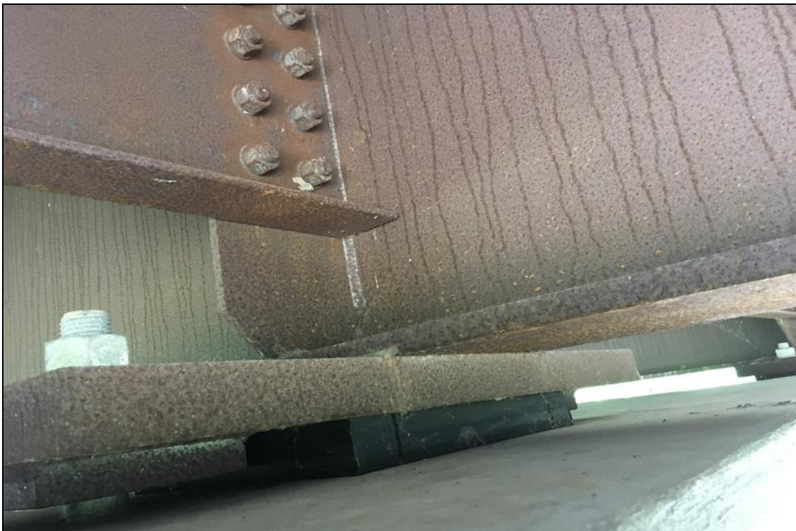
View of the bearing condition at bent #2. Typical of all 5 at this location.
