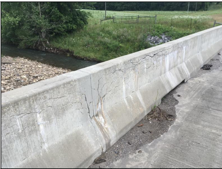
Map cracking with efflorescence in the left parapet wall in span 2.
