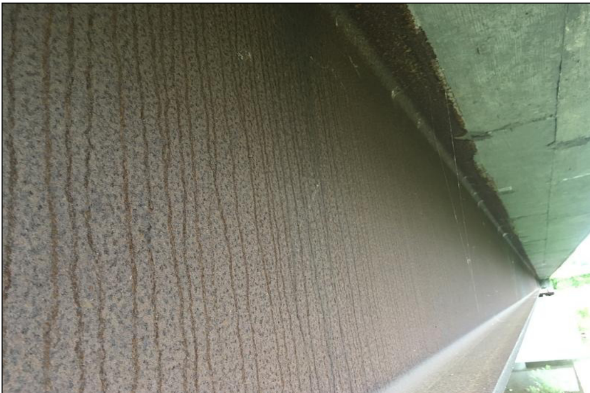
Typical view of the weathering steel protective coating condition.
