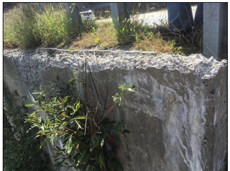
The top edge of the left retaining wall at abutment #1. Showing deterioration with no rebar exposed for 14'
