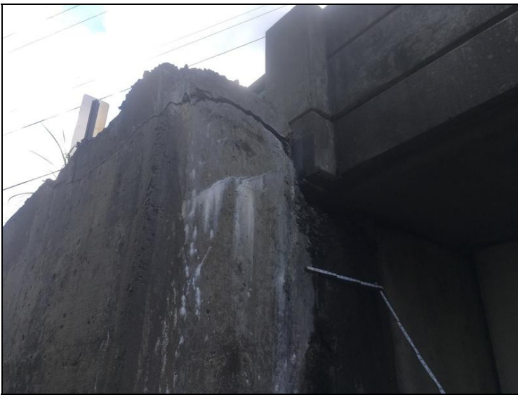
The left corner of abutment #2 has 13' of spalling, deterioration, and efflorescence cracking
