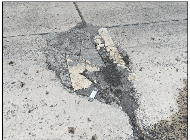
Unsound patched area in the right lane. Typical of several locations.
