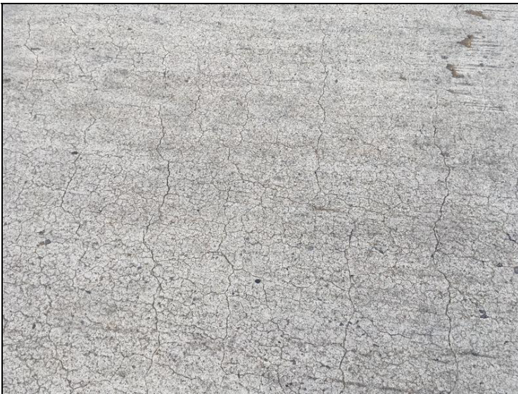
Map cracking in the deck driving surface. Typical of the entire deck.
