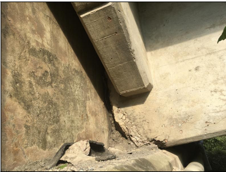
View of the exterior bearing area of beam #2 over abutment #1. Showing deterioration and crushing. The bottom edge of the tee is nearly in contact with the top face of the abutment
