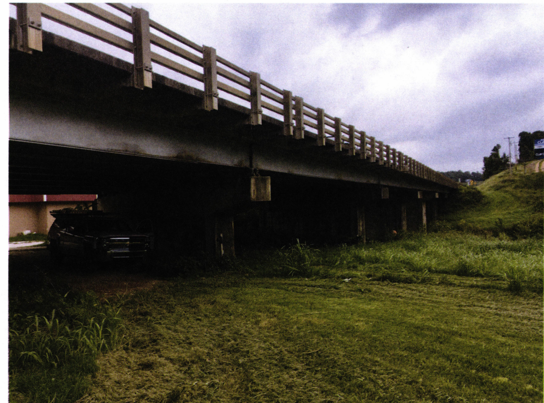
SITE NO. 2 - BRIDGE NO. 05330
