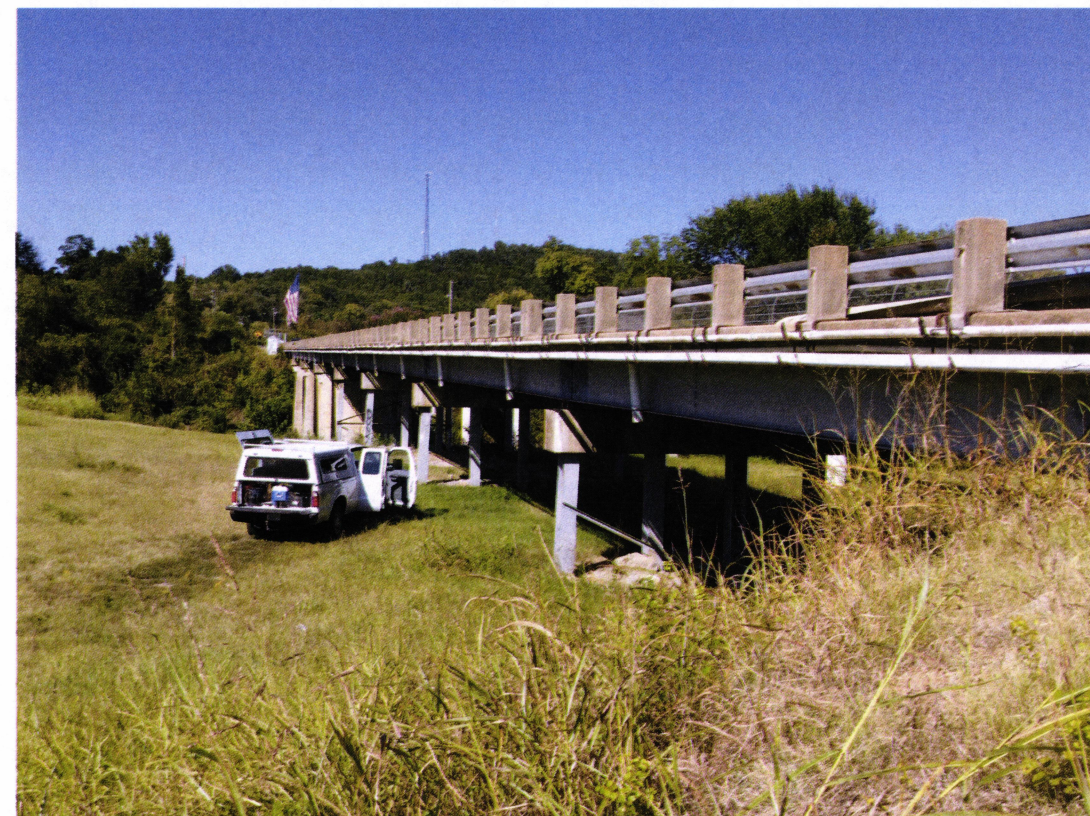
SITE NO. 3 - BRIDGE NO. 00338
