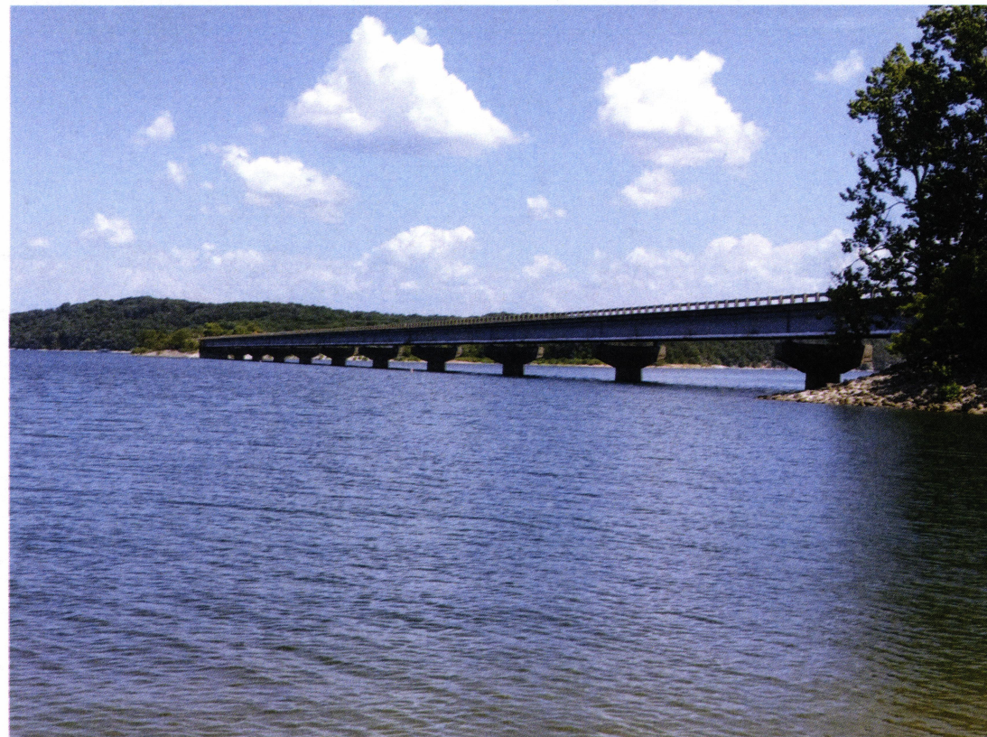
SITE NO. 1 - BRIDGE NO. 03636
