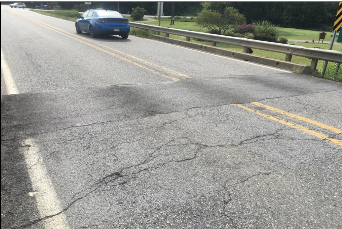
Repaired road way settlement at abutment #1
