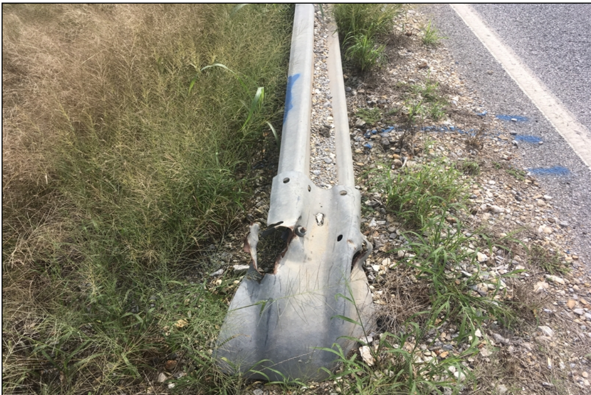
Torn end treatments at the abutment #1 end of the approach railing.
