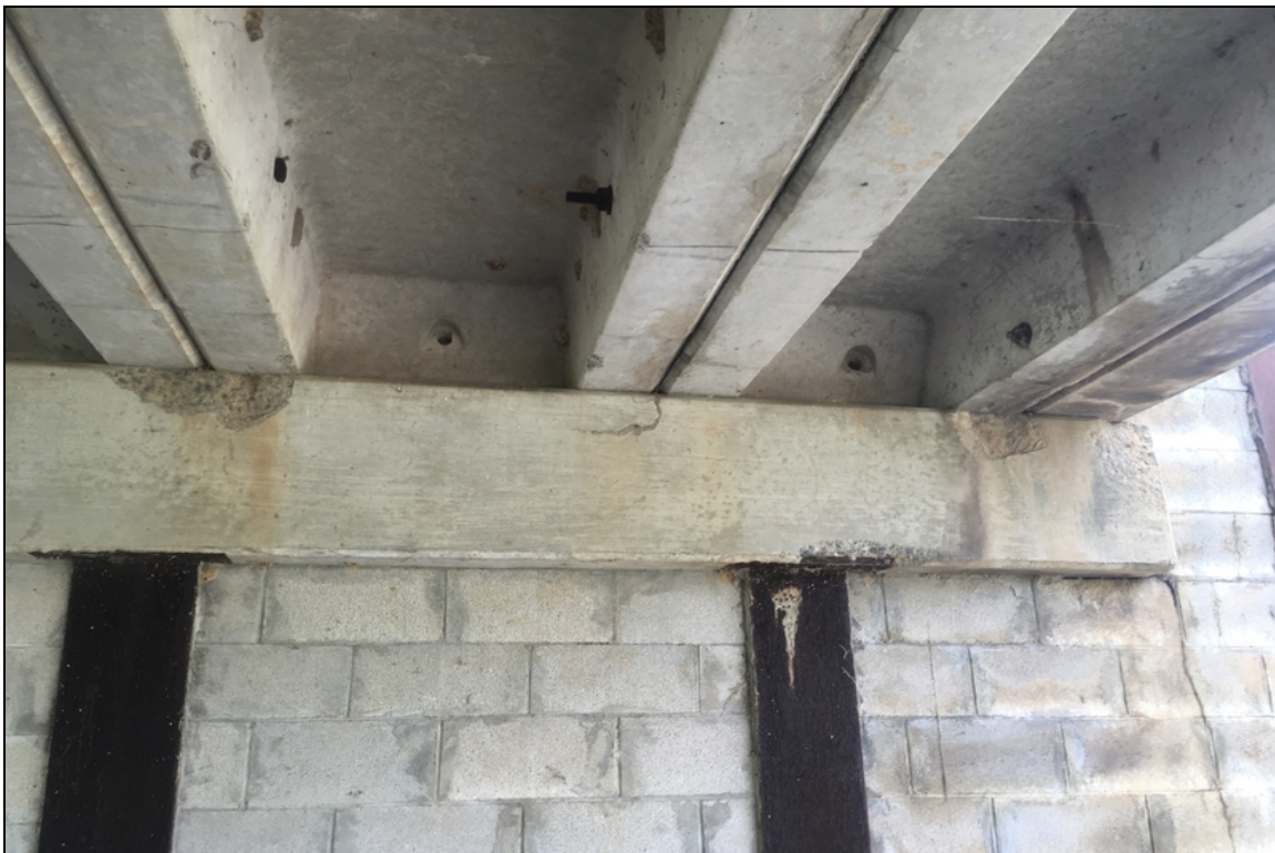
Spalling and delamination at the right end of pier cap #2.
