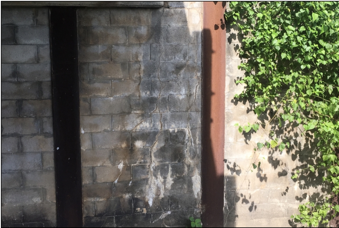
Vertical cracking with efflorescence on the left side of abutment #1.
