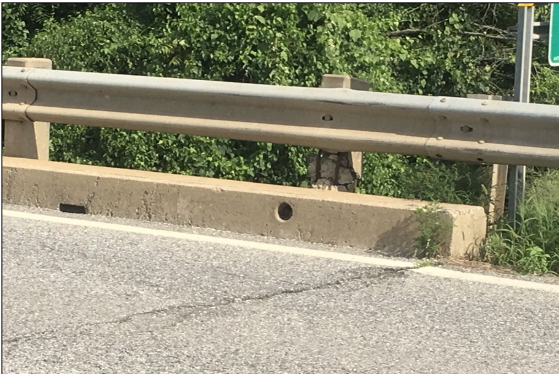
Post #5 along the left side of the structure is damaged.
