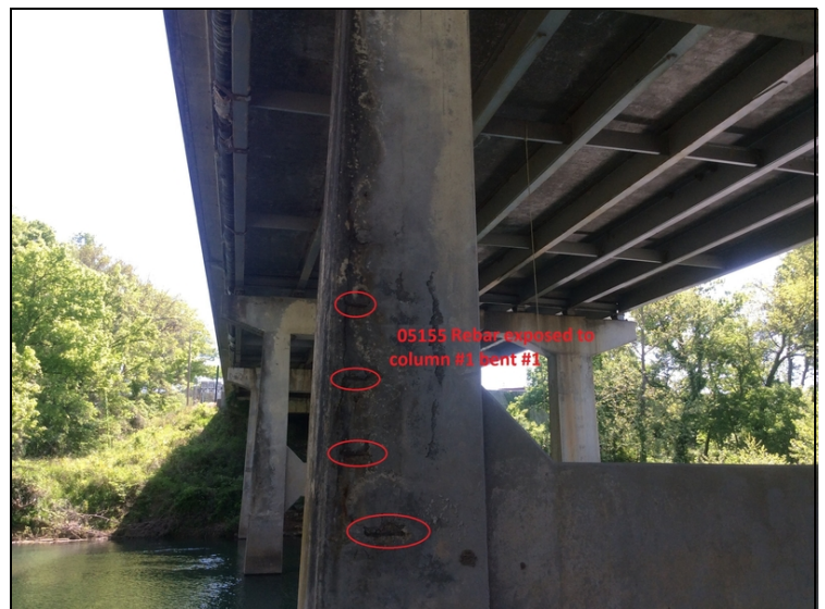
Bent #1 column #1 behind side spalling with steel exposed.
