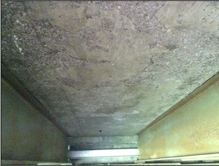
Scaling in undersurface typical.
