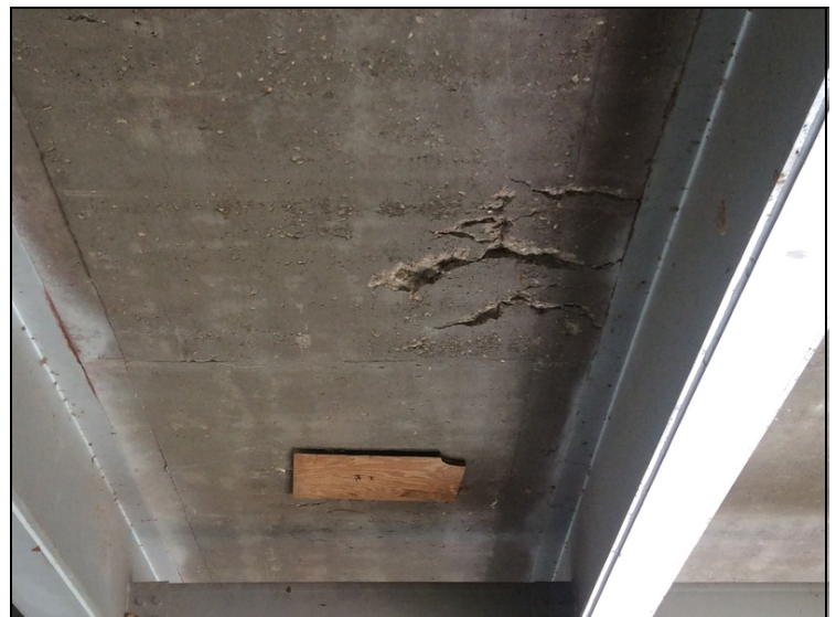
Span #1, bay #6-spalling in undersurface.
