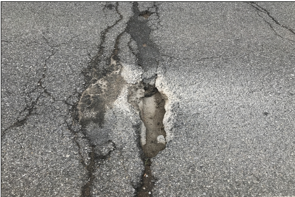
West approach roadway adjacent left side of abutment #1 pothole has formed.
