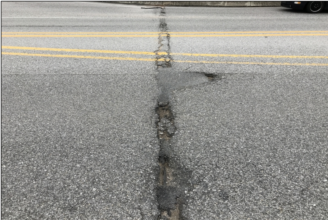
View of bent #4 joint displacement of asphalt overlay material.
