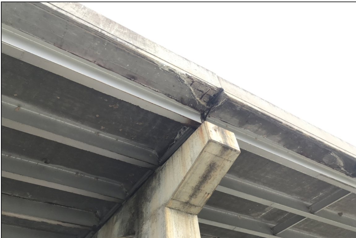
Right side of span #1 above bent #1 right spalling with reinforcing steel exposed.
