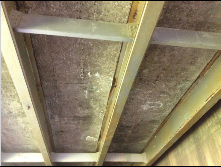
Span #5 bays #3 and #4 delaminated areas.
