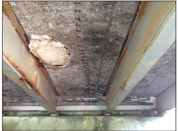
Span 1 bay 2 adjacent abutment 1 concrete patch.
