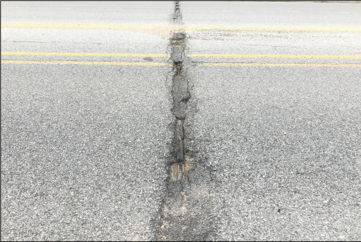
Condition of joint material & wearing surface at bent #1 joint.
