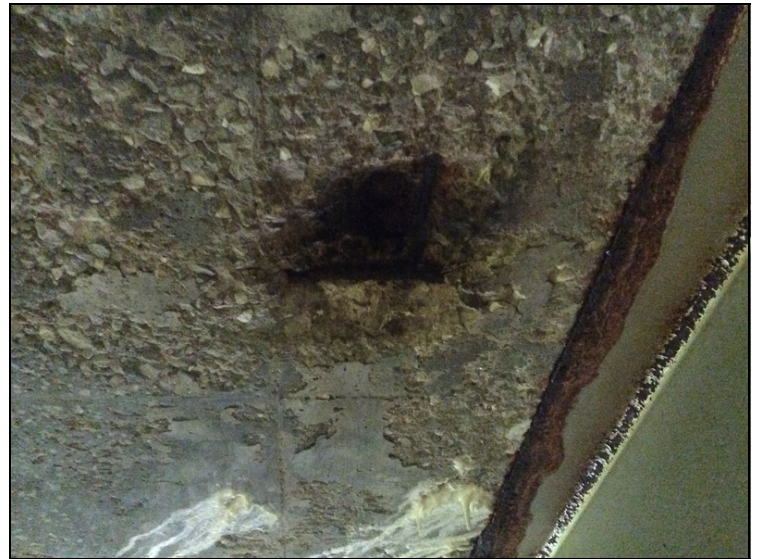
Span #5, bay #4-Spalling with exposed reinforcing steel.
