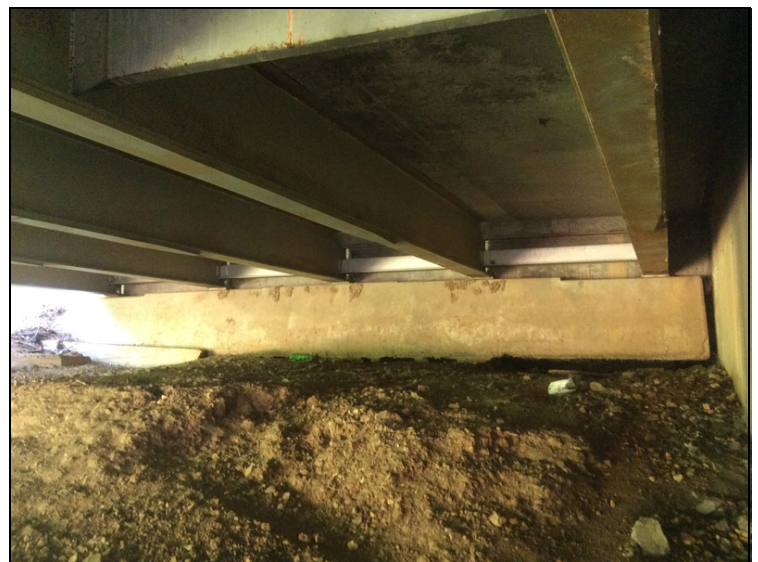
Abutment 2 left - settlement of end slope
