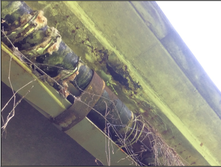
Span #5, Left side-Spalling around deck drains.
