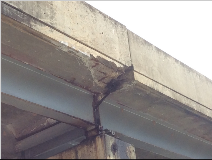
Span #1, right side over bent #1-Spalling with exposed reinforcing steel.
