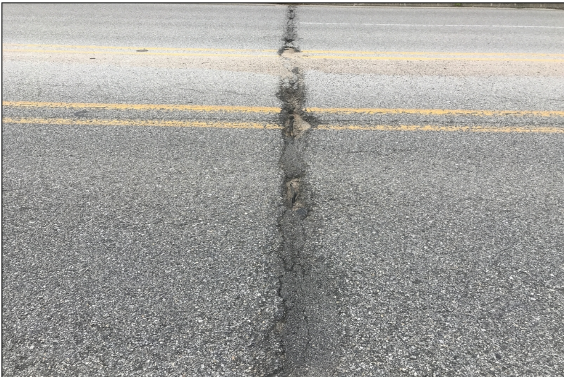
Condition of joint material & wearing surface at bent #3 joint
