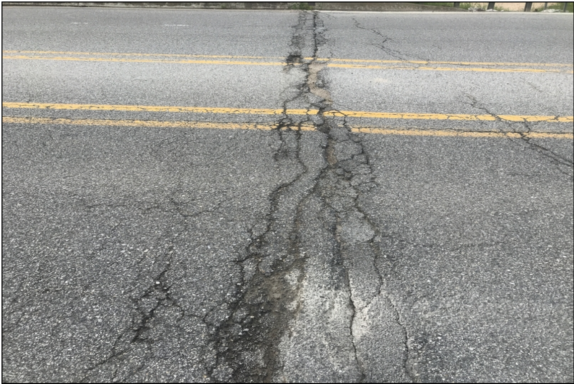
Condition of abutment #1 joint
