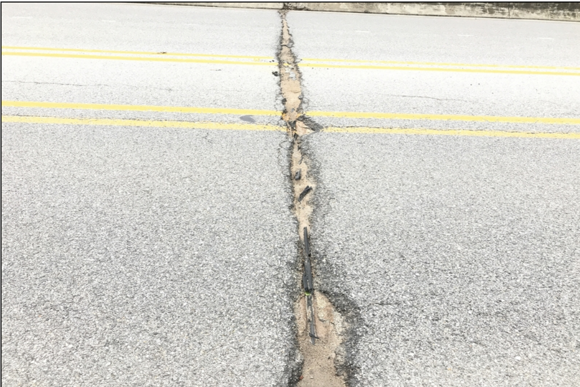
View of bent #1 joint displacement of asphalt overlay material.
