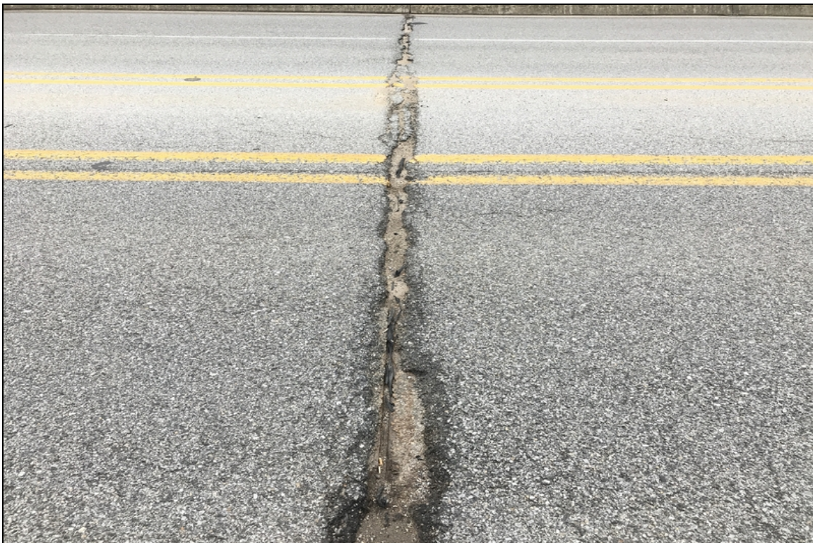
View of bent #3 joint displacement of asphalt overlay material.
