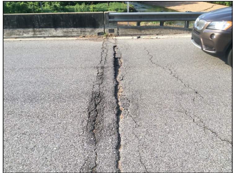
Abutment 1 right lanes approach roadway potholes.
