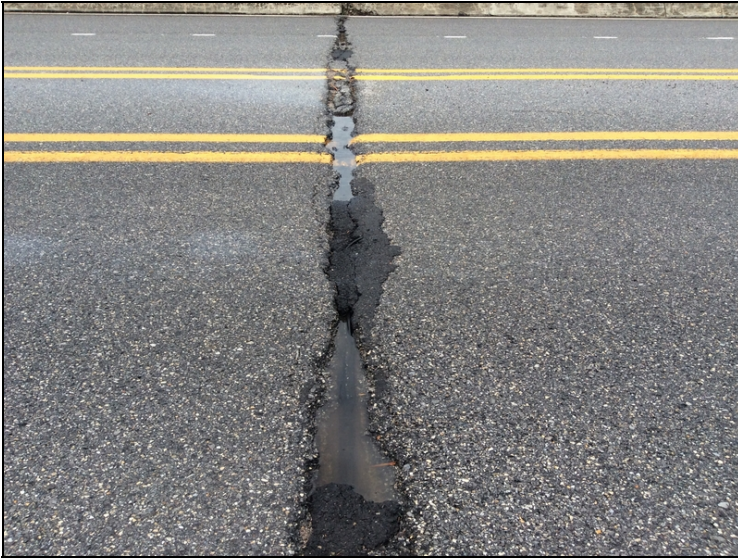
Bent #1-Potholes in ACHM driving surface.
