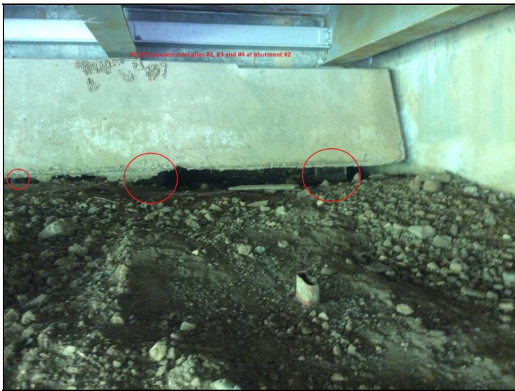
Exposed steel pile #2, #3, & #4 at abutment #2
