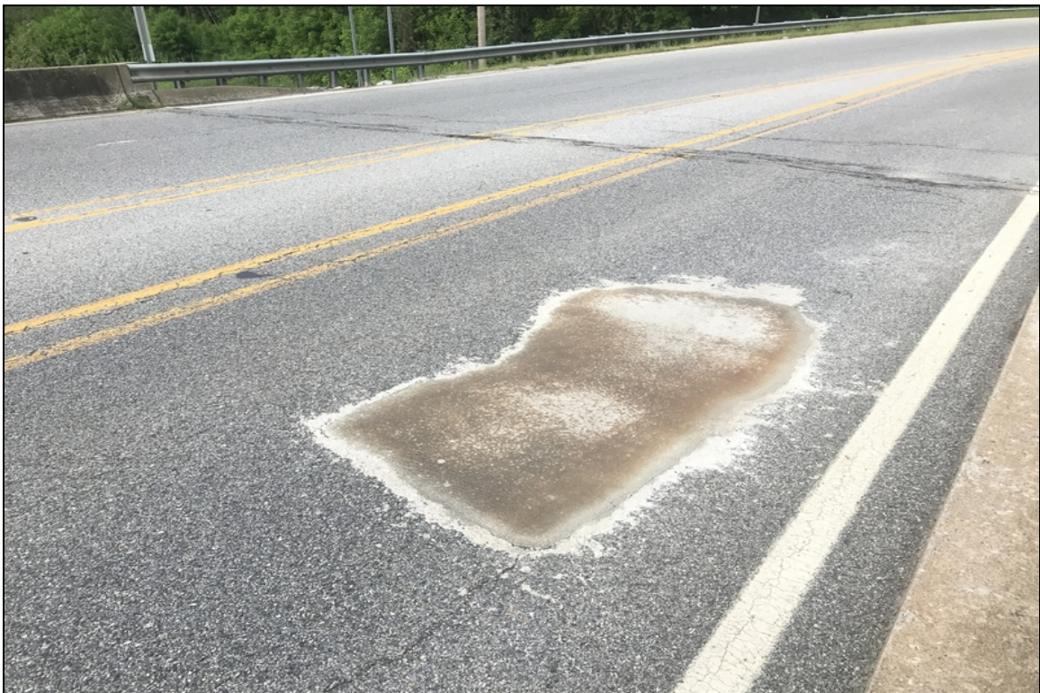
Large concrete patch span #1 left lane.
