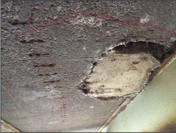
Span #1, bay #2-Delaminated area around repair.
