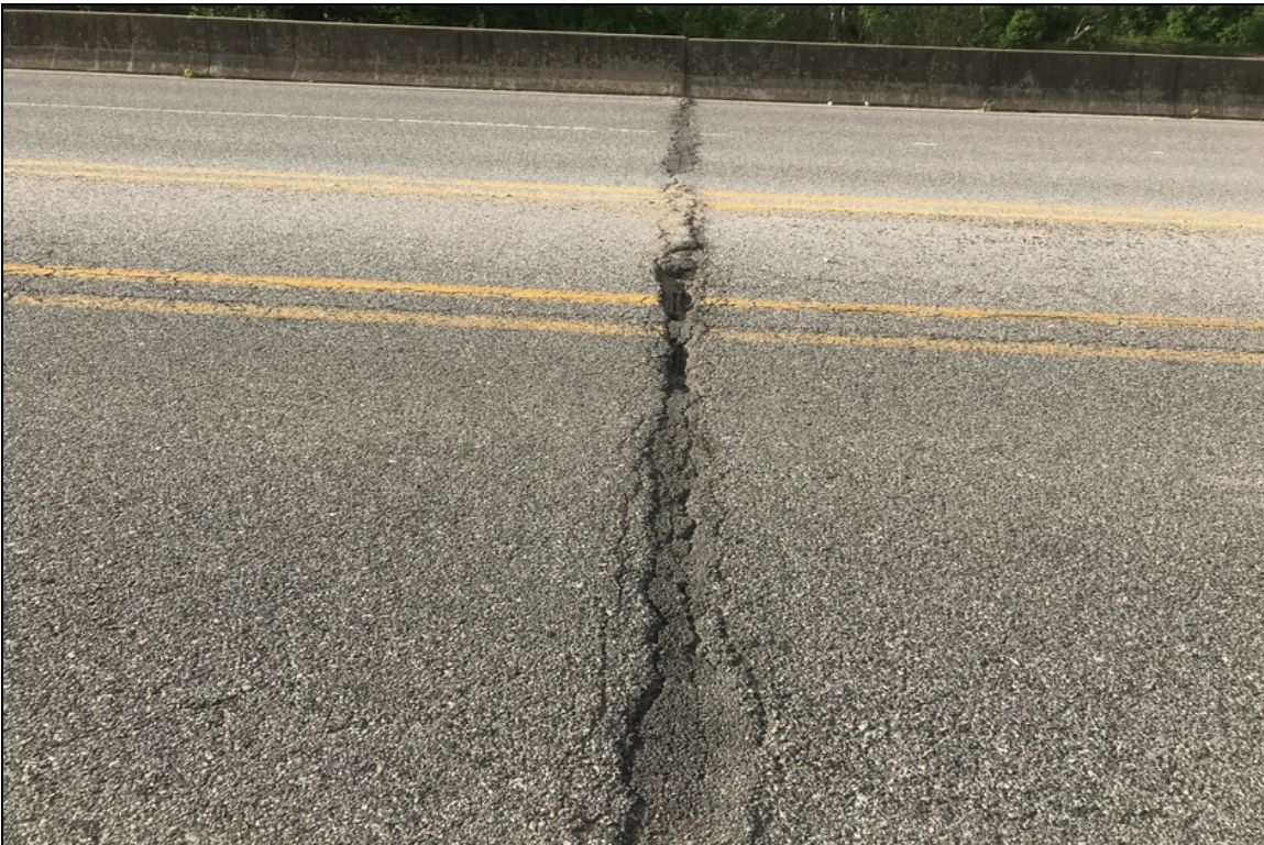
Condition of joint material & wearing surface at bent #2 joint
