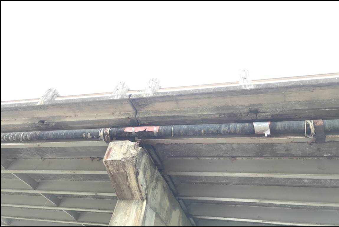
Typical exposed reinforcing steel around deck drains.
