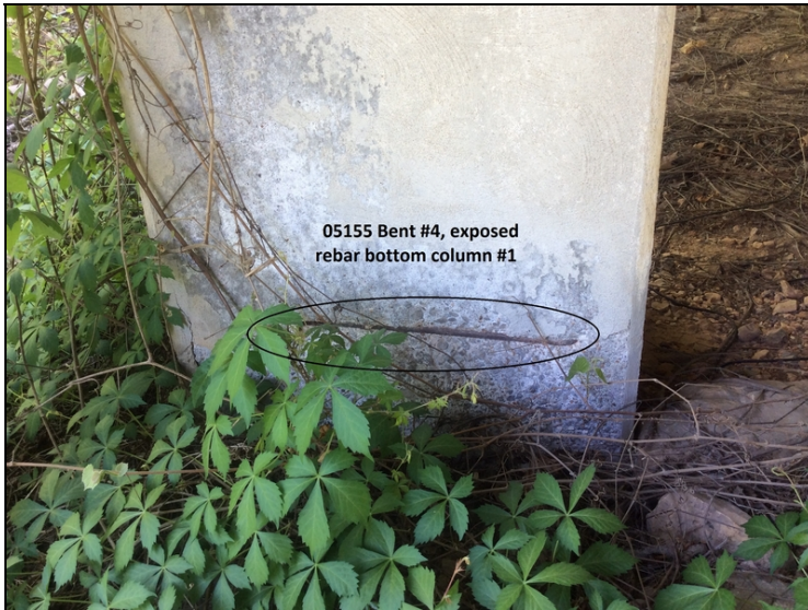
Bent #4 column #1 base of column shallow rebar exposed.
