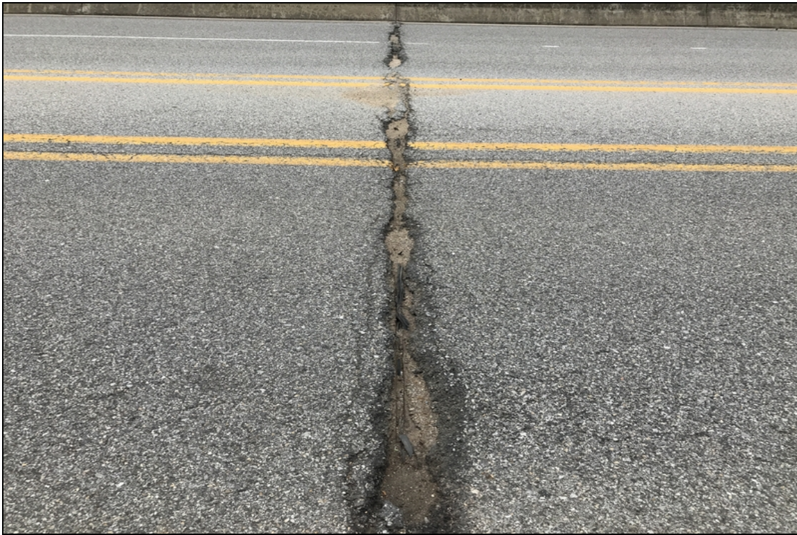
View of bent #2 joint displacement of asphalt overlay material.
