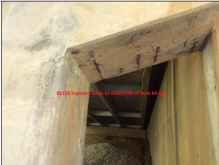
Bent #4 cap right undersurface has exposed rebar
