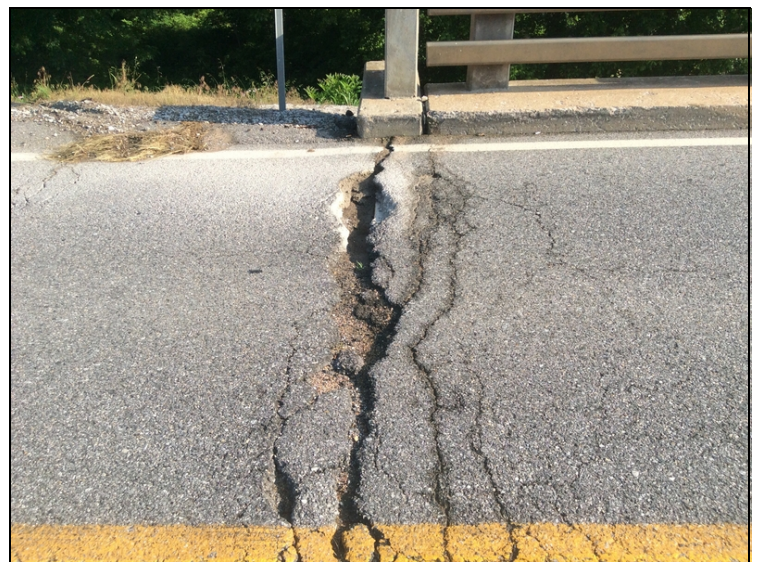
Abutment 2 left lanes approach roadway potholes.
