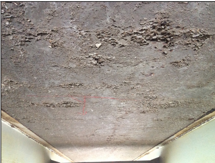
Span #1, bay #3-medium scaling with large delaminated area.
