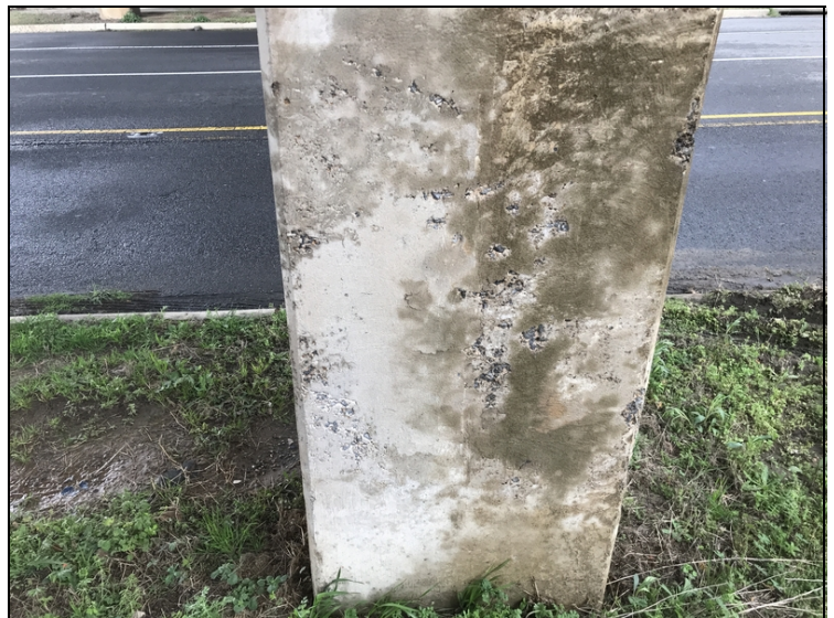
Typ Scale in Column 2 at Pier 2 & Column 1 at Pier 3.
