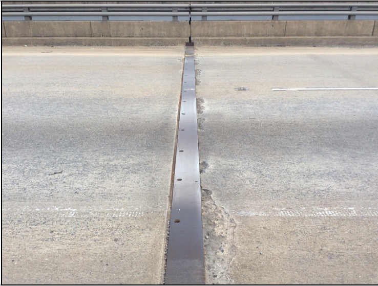
Joint #3, span #3 - minor and moderate spalls along slide plate
