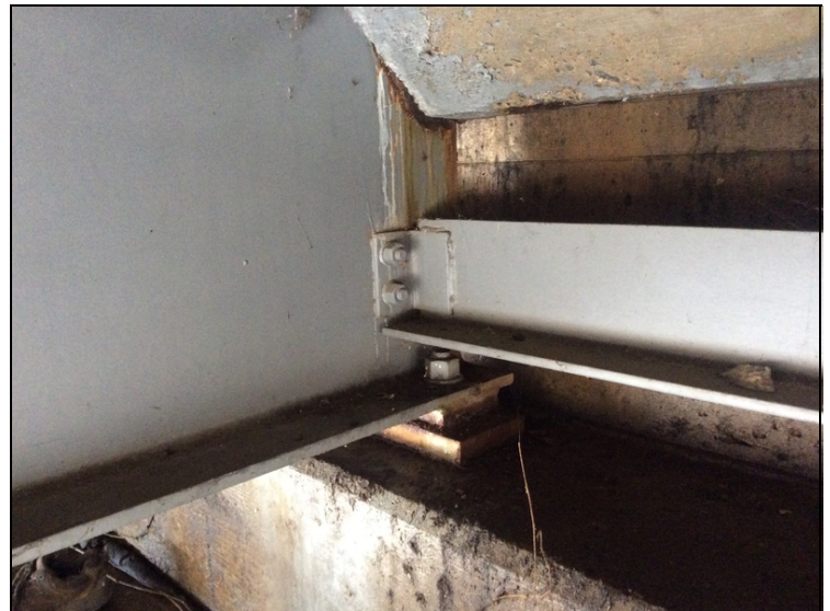
Abut #1, beam #4 - minor section loss in web. Beam #5 typical. Bearings 2 - 5 minor pack rust. B1, B6 & B7 minor rust.
