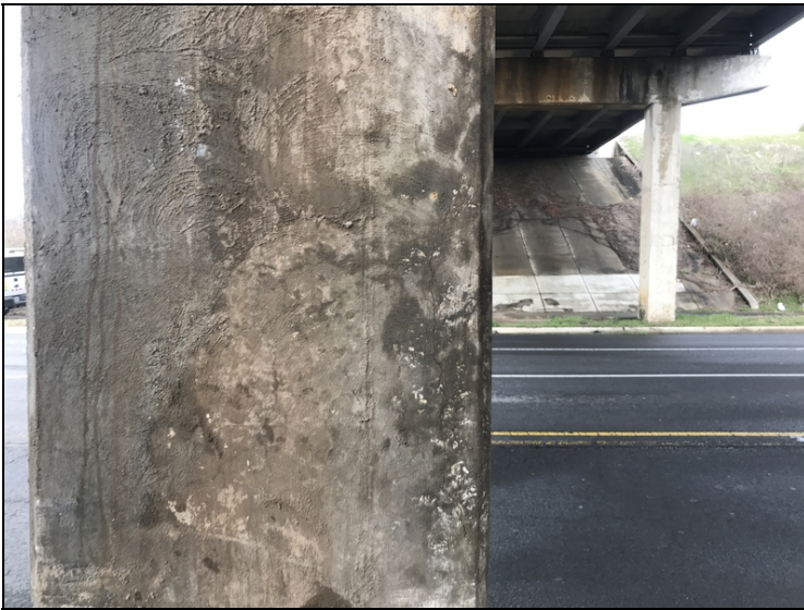
Typ. Cracking in Column 1 at Pier 2 & Column 2 at Pier 3.
