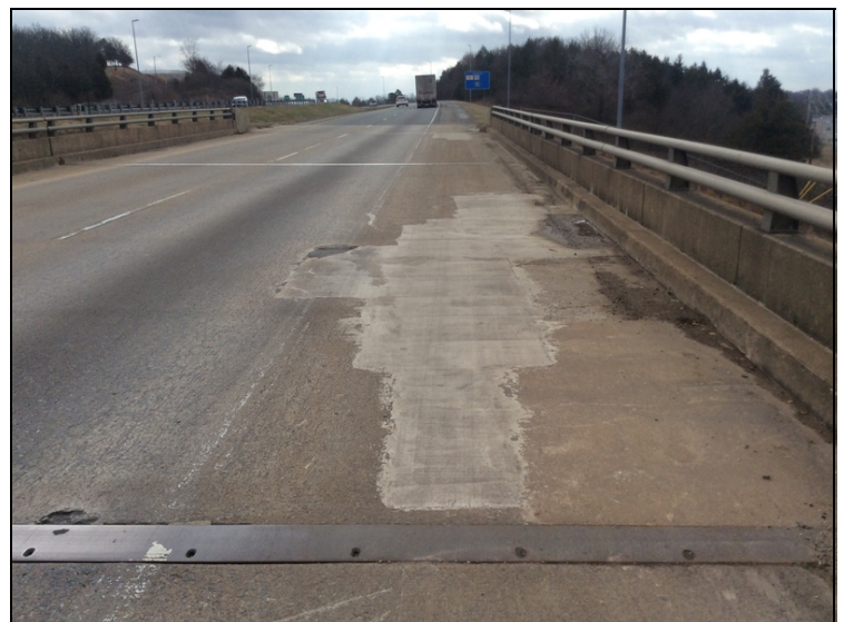
Span #2, right side - minor spalls around patch area and next to curb.
