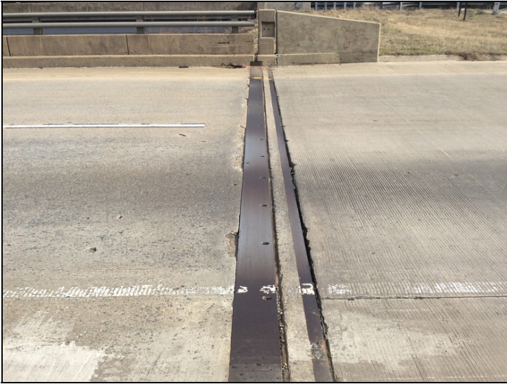
Joint #4 - minor to moderate spalls along the back side of slide plate.
