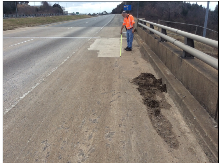
Span #3, right shoulder - moderate spall.
