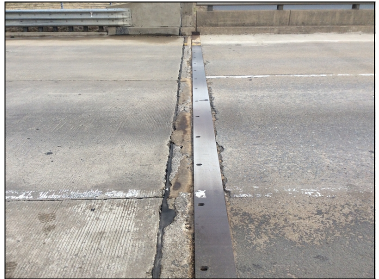
Joint #1 - minor spalls in deck and head wall along slide plate.
