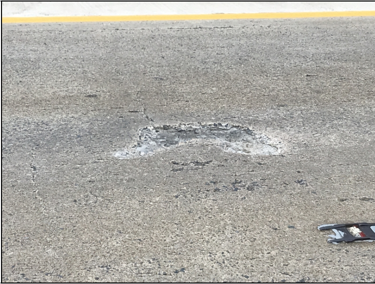
Minor Spalling in Span 1.
