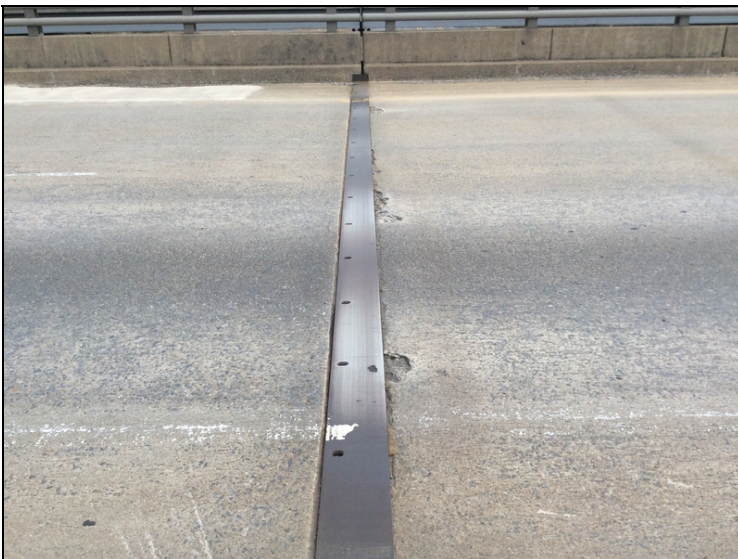
Joint #2, span #2 - minor spalls along ahead side of slide plate
