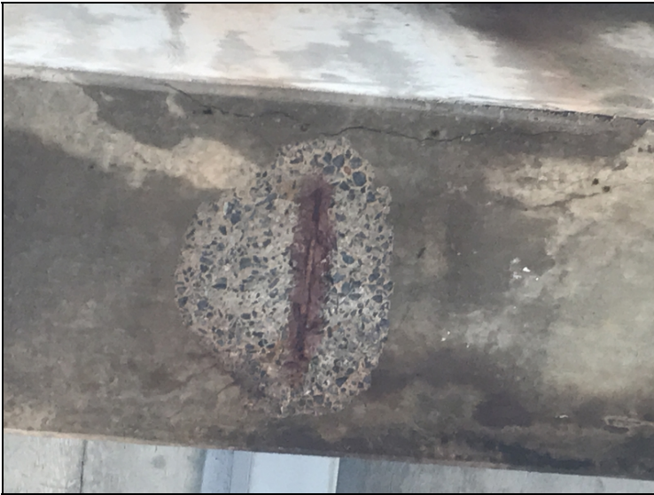
Delam, Cracking & Spalling W / Rebar Exposed in Bt Face of Cap 3.
