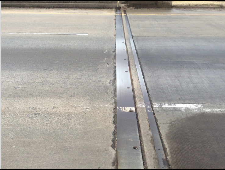
Joint #1 - minor spalls along the ahead side of slide plate. Typical at all joints
