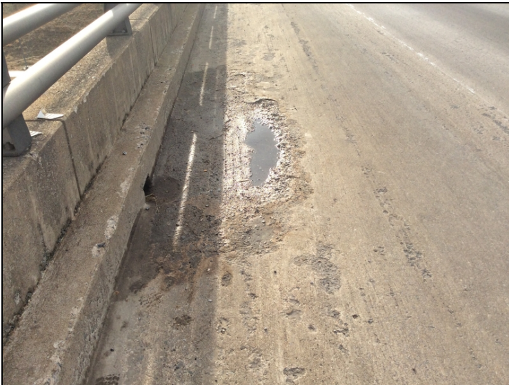
Span #1, left side - spall and scale
