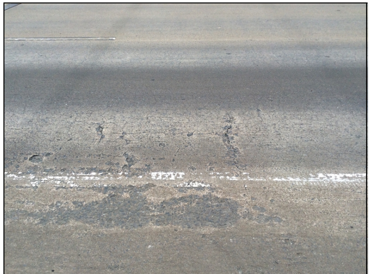
Moderate and major unsealed cracks. Map cracking in outside lane and moderate scale.
