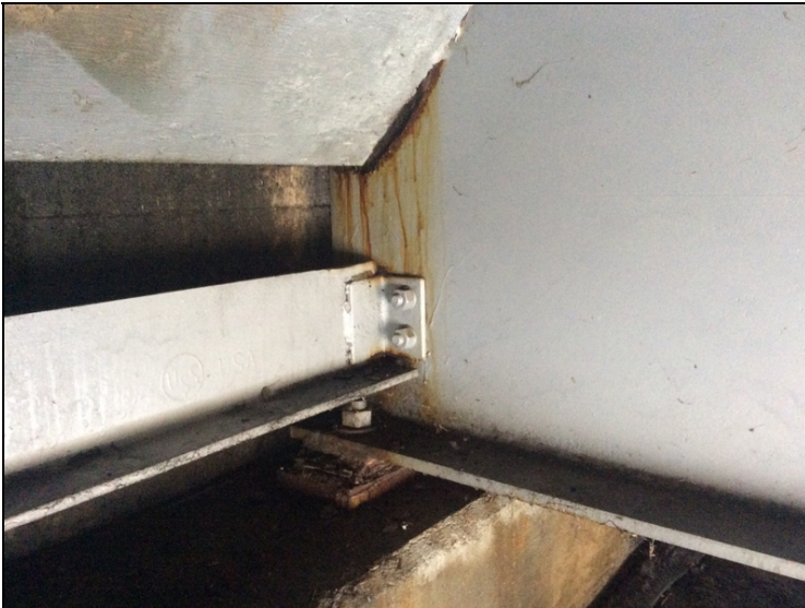
Abut #4, Beam #4 - moderate section loss in web below concrete haunch.
