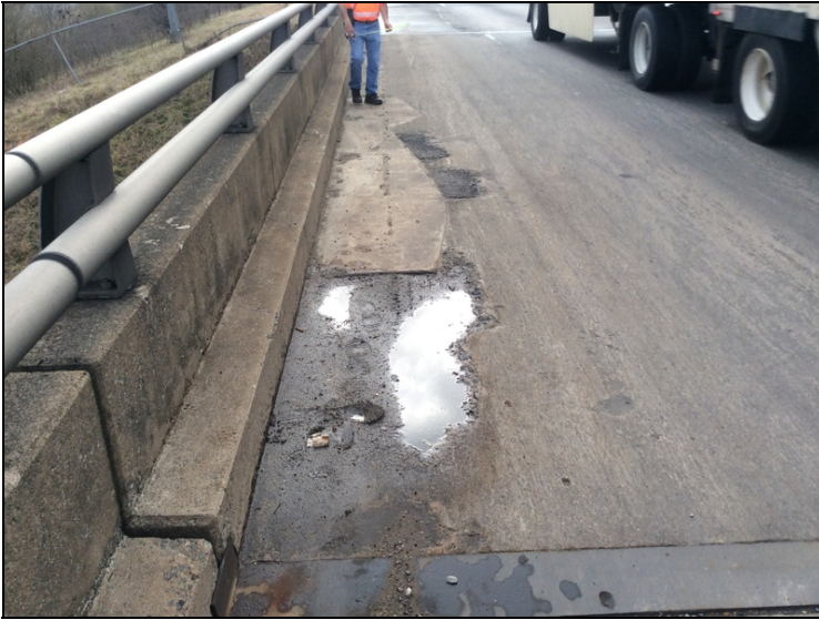
Span #3, left side - moderate spalls
