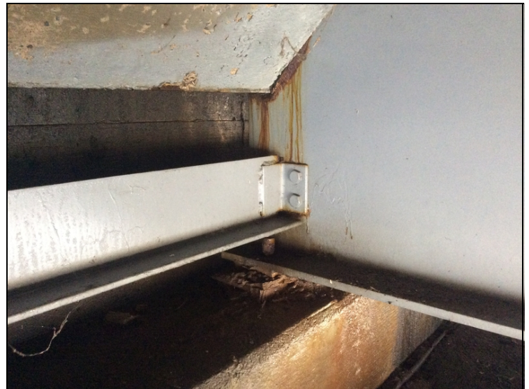
Abut #4, beam #3 - heavy pack rust on bearing, Bearing B1 & B2 minor pack rust.
