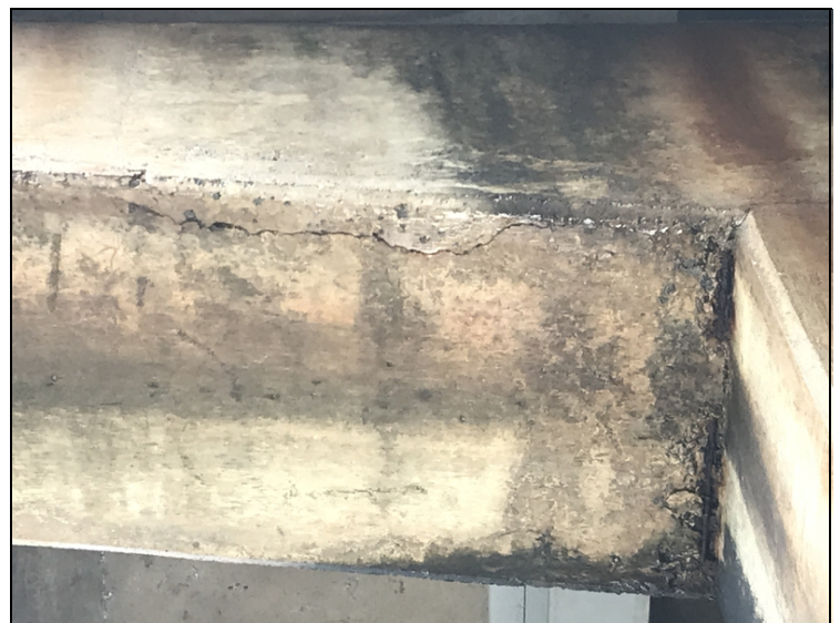
Typ. Cracking in Bt Face of Cap 3.
