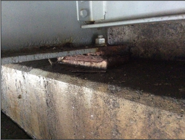
Abut #1, bearing #3 - heavy pack rust.
