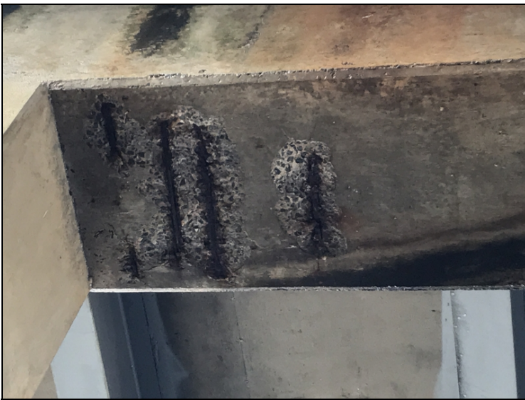
Delam, & Spalling W / Rebar Exposed in Bt Face of Cap 3.
