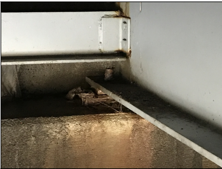
Anchor Bolt Nut Missing on Beam 3 at Abutment 4.
