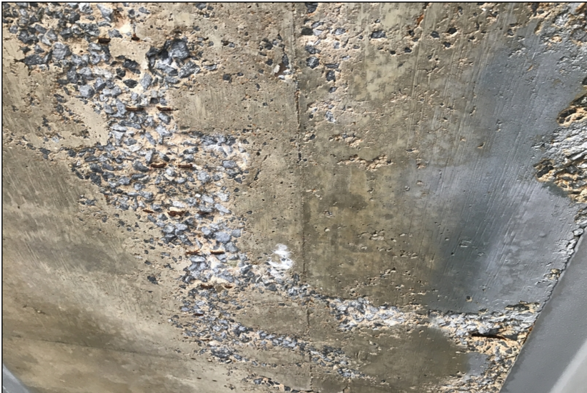
Typ. Scale in Soffit.
