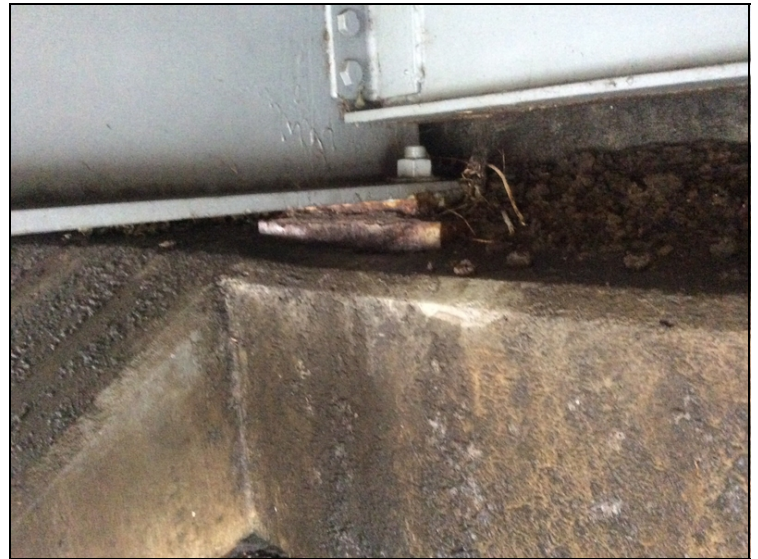
Abut #1, bearing #2 - moderate pack rust. B5 & B6 typical, B1 & B7 minor rust.
