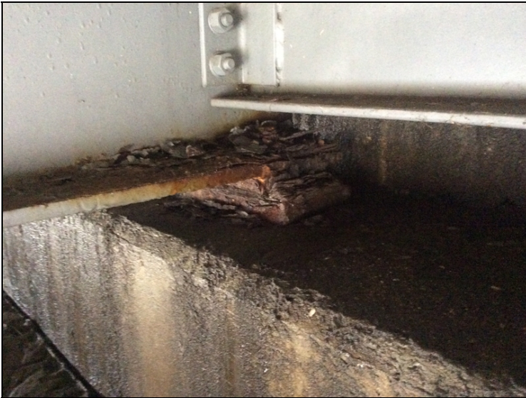
Abut #1, bearing #4 - heavy pack rust.
