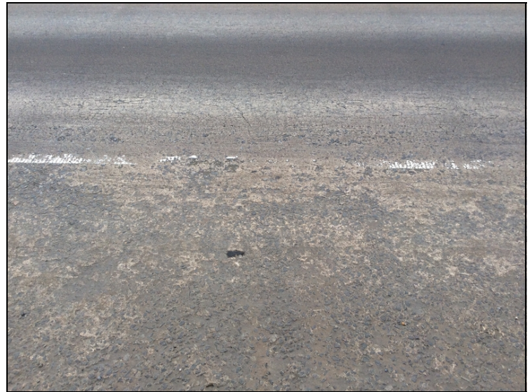
Map cracking mostly in outside lane.
