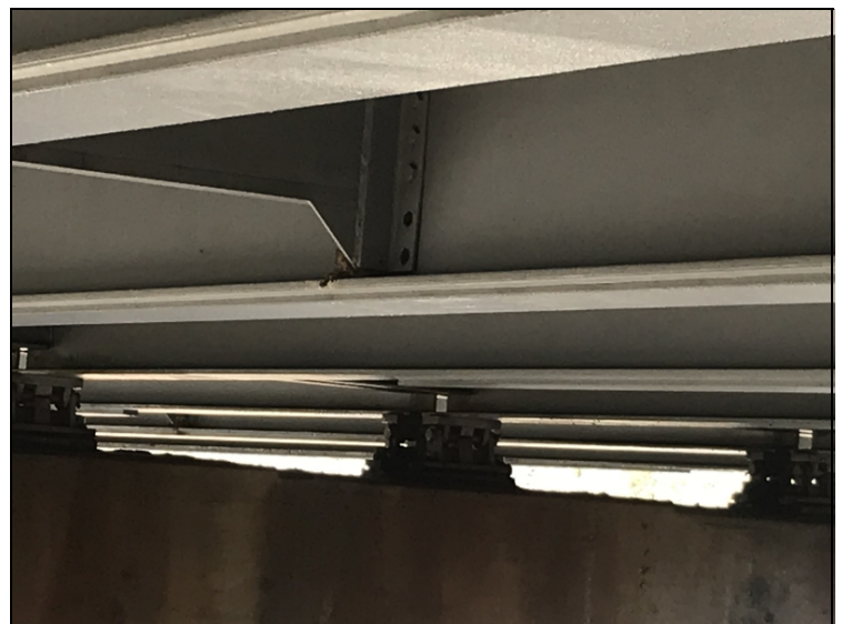
Bolts Missing on Beam 5 Span 3.
