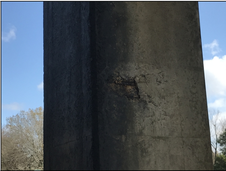
Delam & Spalling W / Rebar Exposed in Column 1 Rt. Side at Pier 2.
