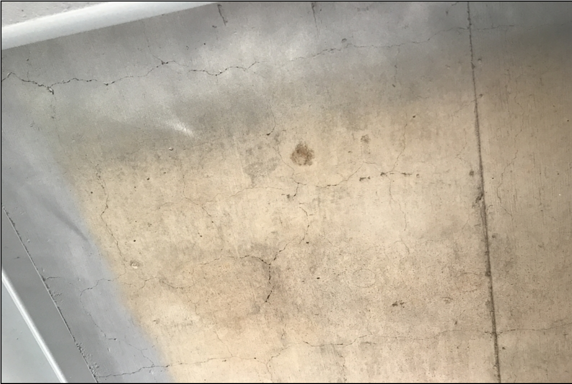
Span 1 bay 4, typical cracking of soffits.
