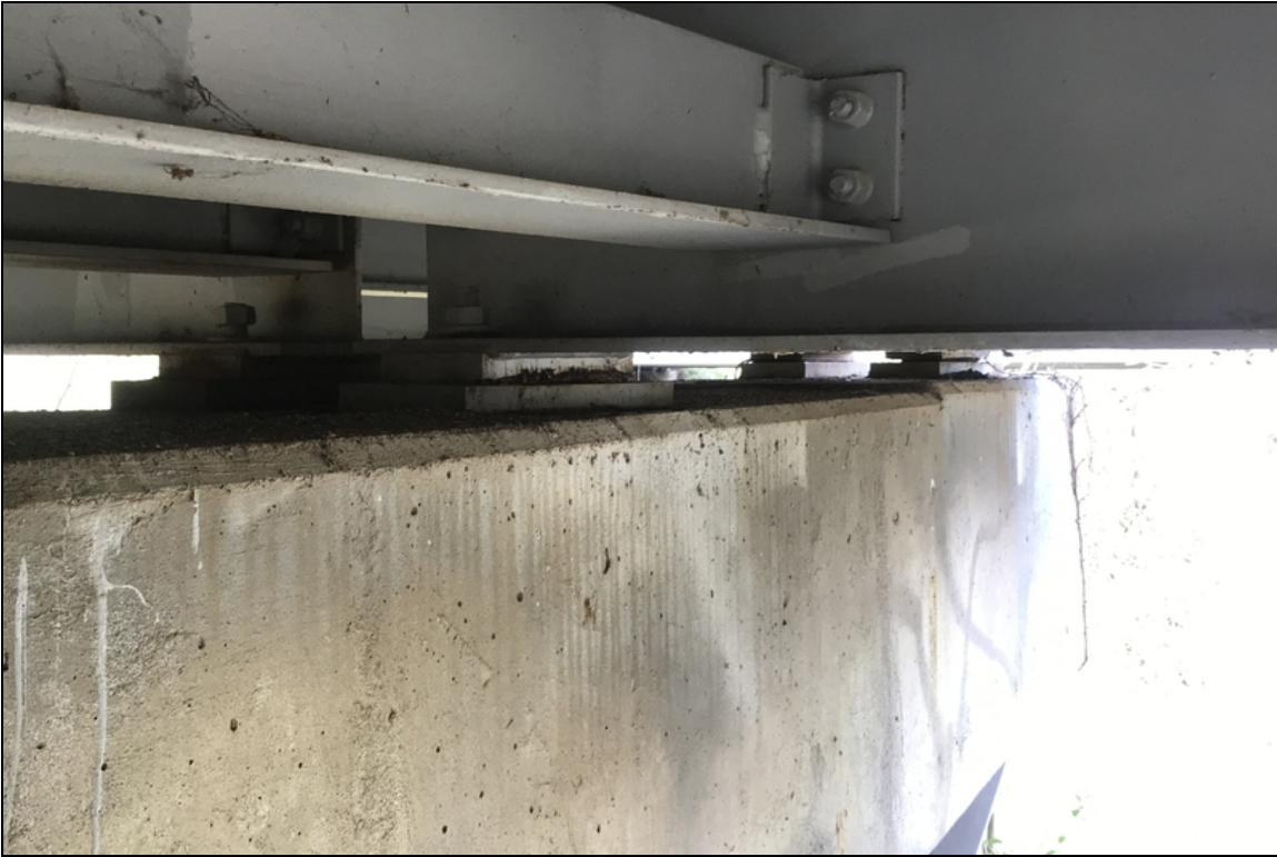
Bent 2 G2 bearing 2 has pack rust, this is typical at G 3, 4, 5.
