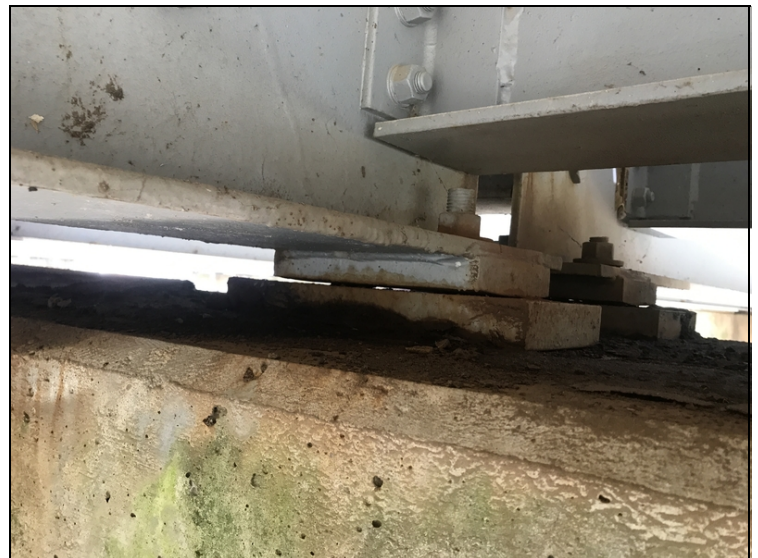
Moveable bearings at bent 3 have corrosion and some having pack rust. Bearings 4 back side and bearings 3 and 4 ahead side are floating.
