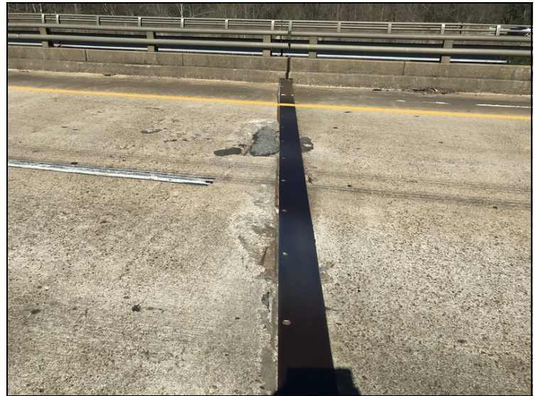
Span 4 large spalls in both lanes with exposed reinforcing steel.
