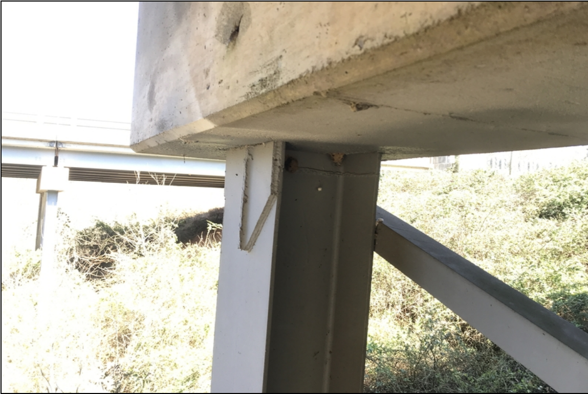
Bent 5 pile 1 has been repaired.
