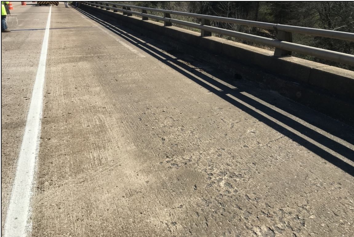
Abrasion along right shoulder this is typical.
