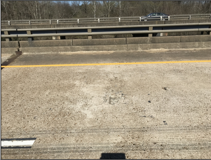
Span 3 left lane spall with exposed reinforcing steel.
