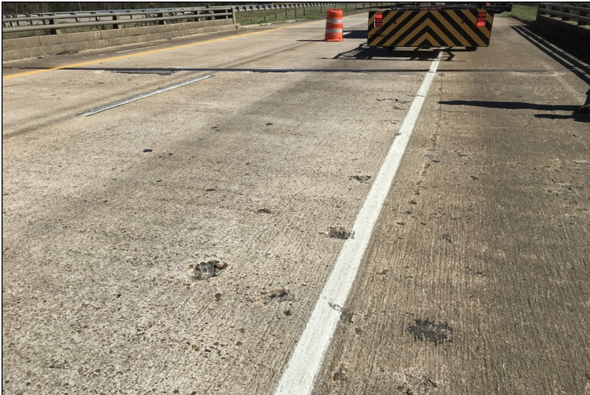
Span 4 shallow spalls in right lane.
