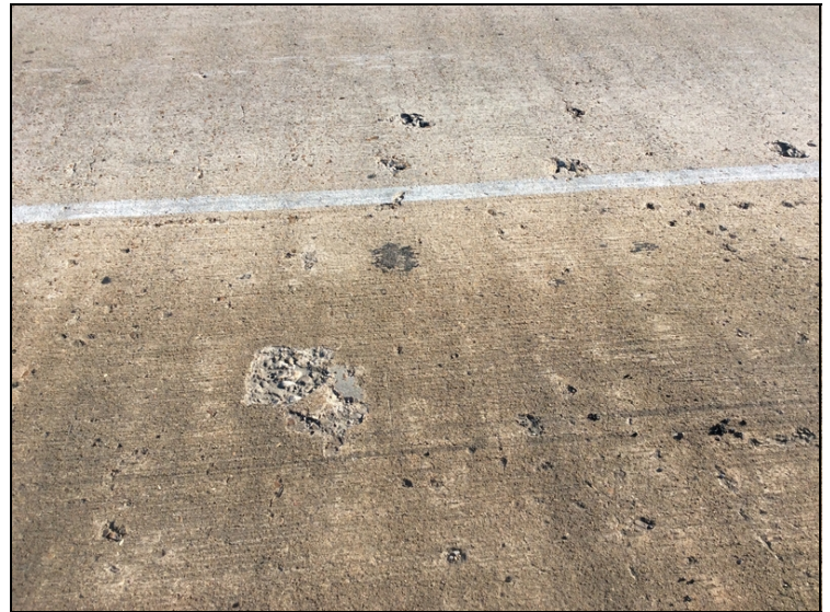
Typ. Delam, Cracking, Scaling & Spalling in Deck.
