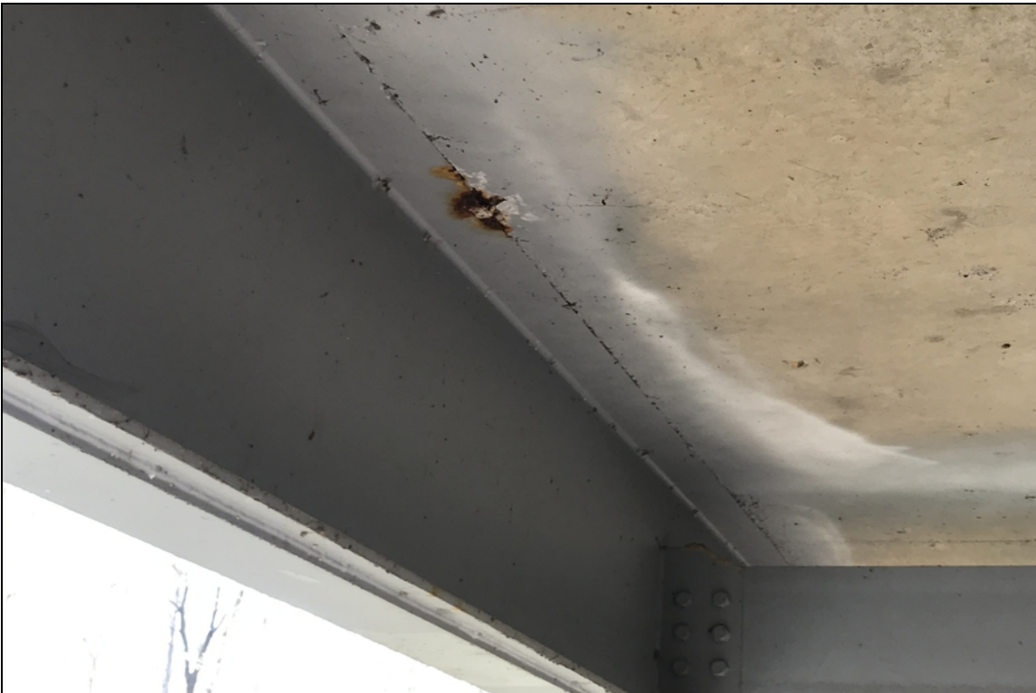
Span 2 girder 7 has corrosion on top flange between diaphragm 2 and 3.
