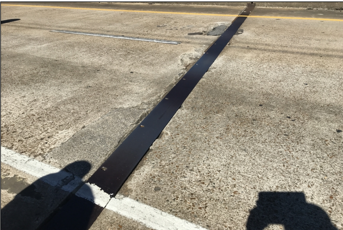
Bent 5 right lane has approximately 5' of loose joint armor.
