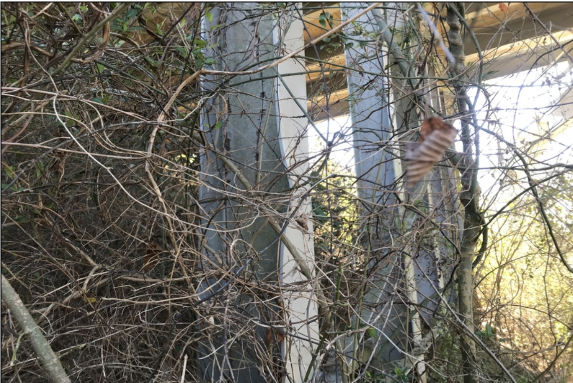
Bent 5 pile 1 has a bend in the flange approximately 5' above ground level.
