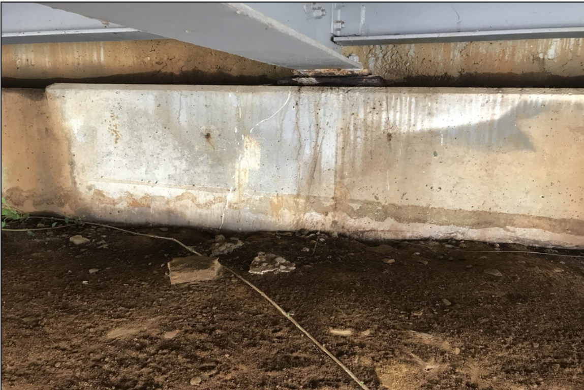
Bent 1 has a few vertical cracks.
