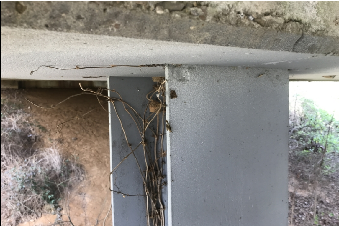
Bent 2 piles 5 and 7 has section loss at the top of piles.
