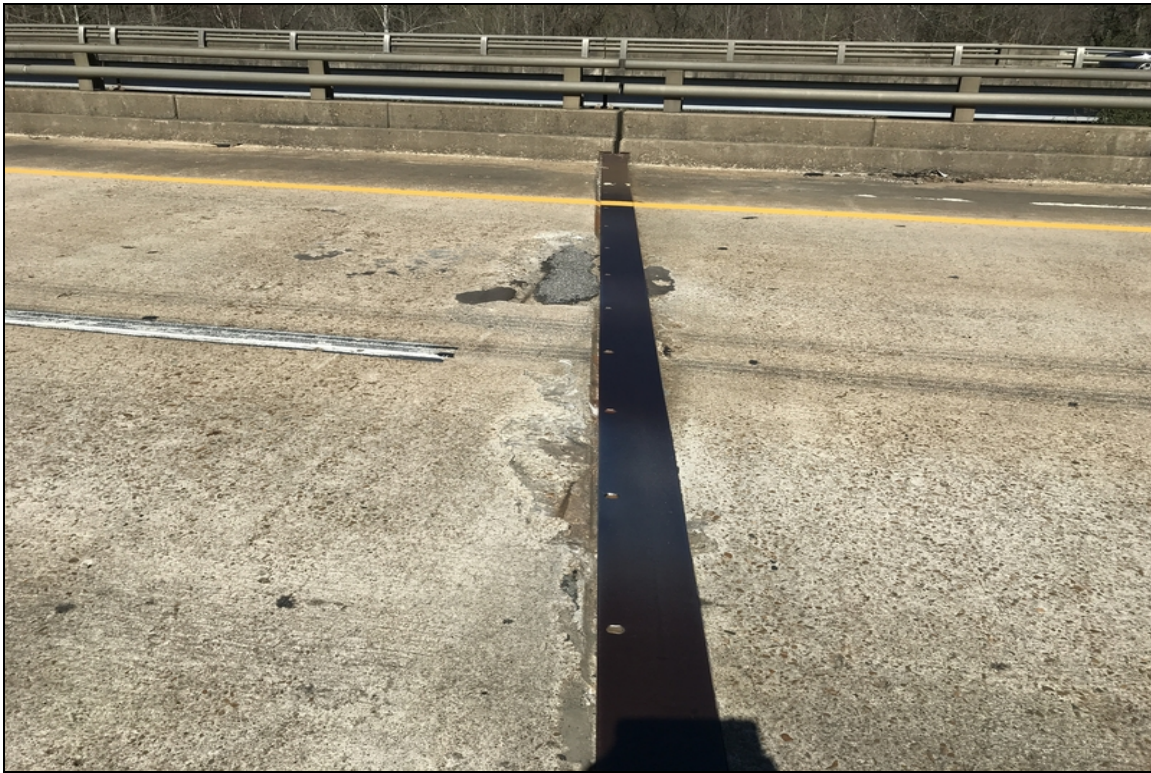
Span 4 large spalls in both lanes with exposed reinforcing steel.
