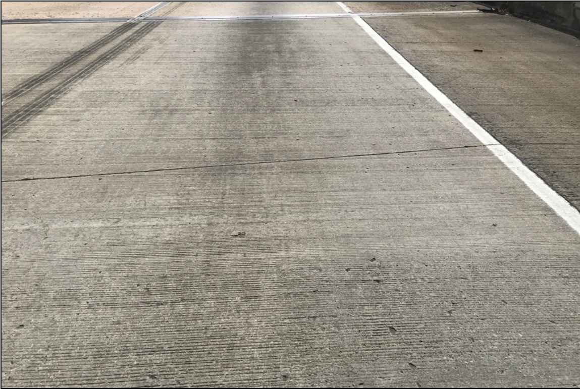
West approach has longitude cracking.
