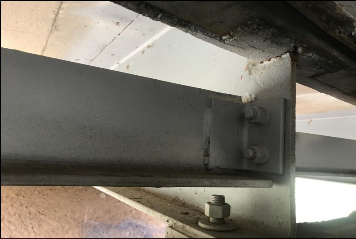
Bent 2 top of girders have section loss in the haunch area at the follow locations. Girders 2 thru 7 back side and girders 3 thru 5 on the head side.
