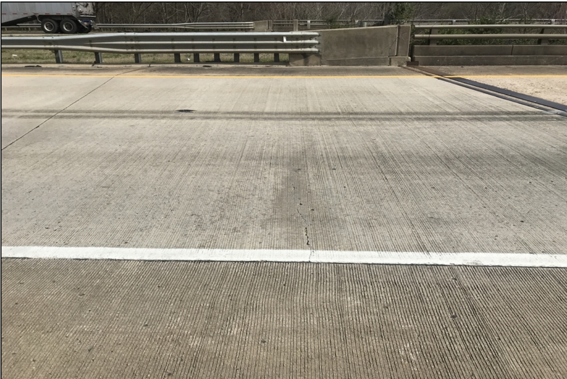
West approach right lane, large transverse crack.
