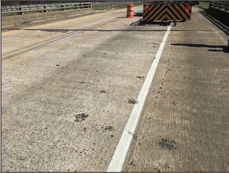
Span 4 shallow spalls in right lane.
