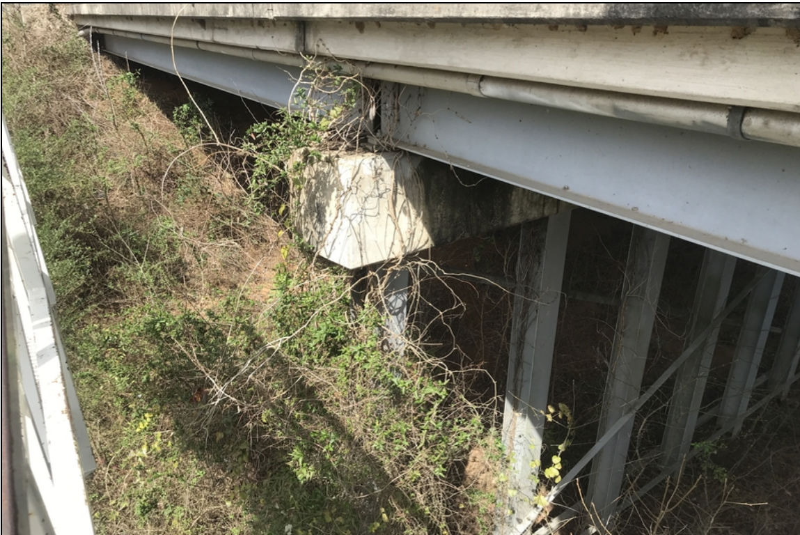
Bent 2 right vegetation up on cap and piles.
