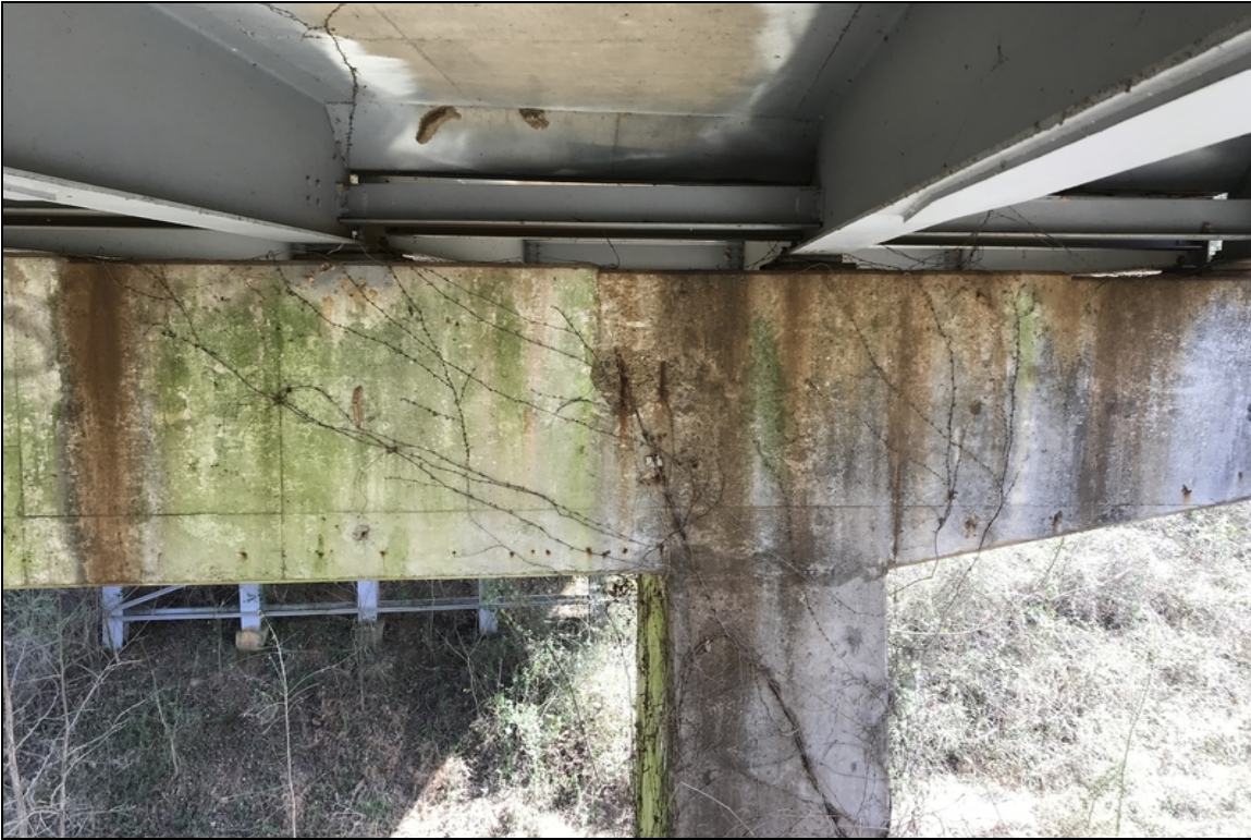
Bent 4 back side 2' spall with exposed reinforcing steel with section loss.
