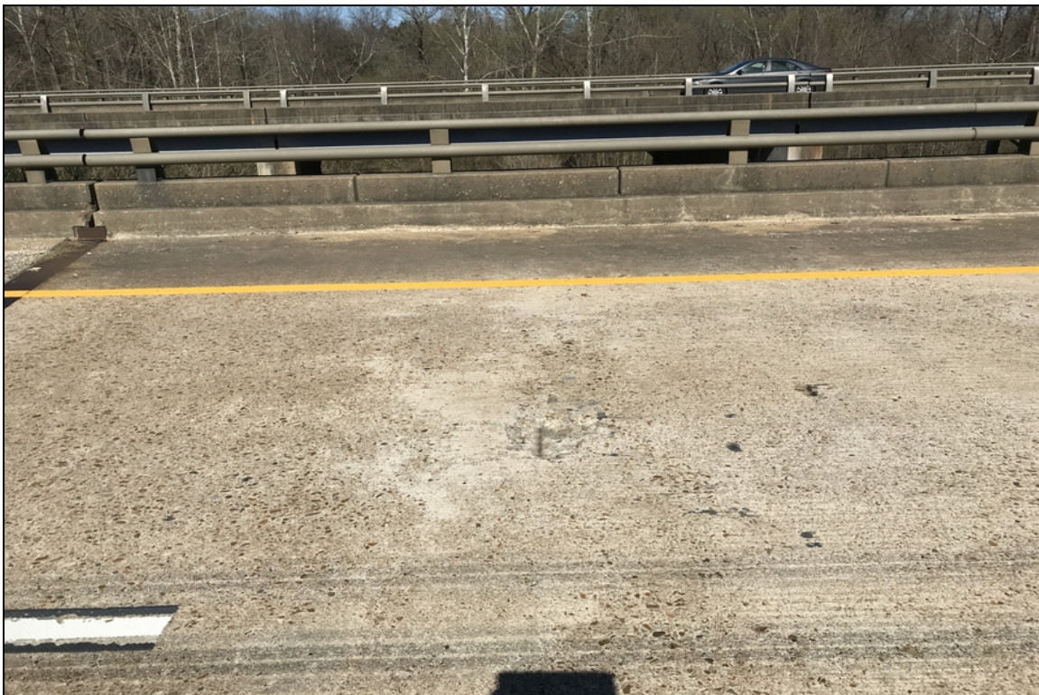
Span 3 left lane spall with exposed reinforcing steel.
