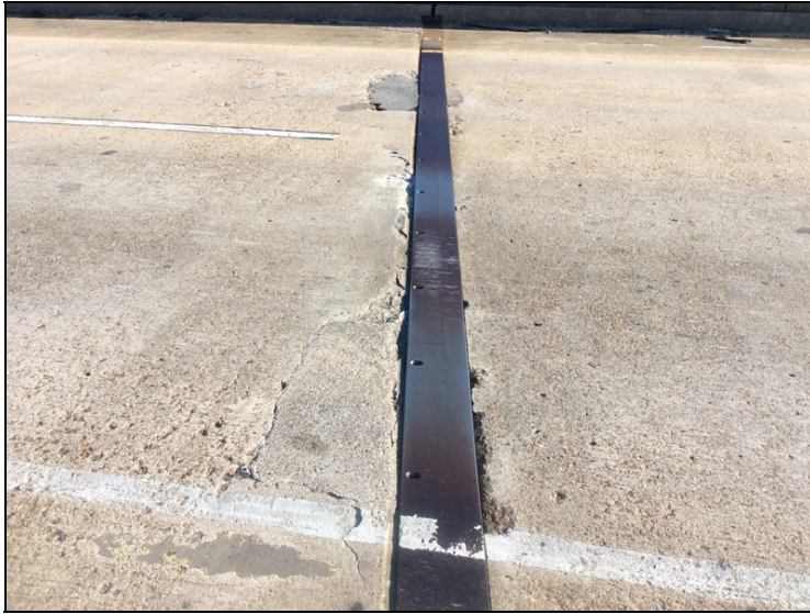
Typ. Delam, Cracking, Scaling & Spalling at Joints.
