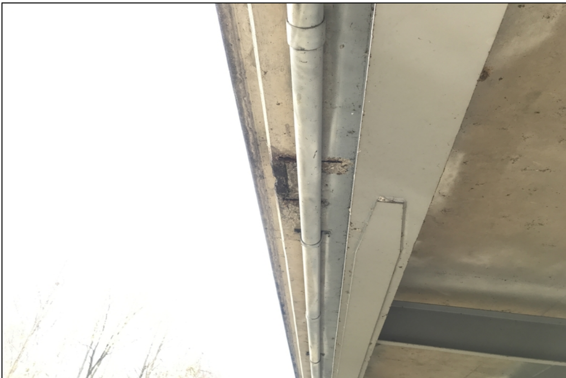
Span 2 has 2 spalls with exposed reinforcing steel in the soffits on the right side at the drains.
