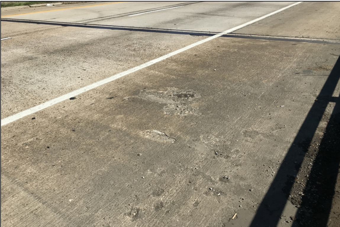
Span 5 deep abrasion in right lane.
