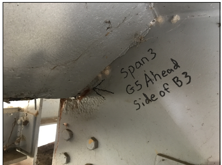
Span 3 Girder 5 ahead of bent 3 there is a crack in haunch area about an 1" long.
