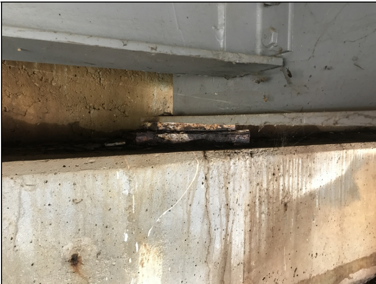
Bent 1 bearings 2 thru 4 are floating, making contact under load.
