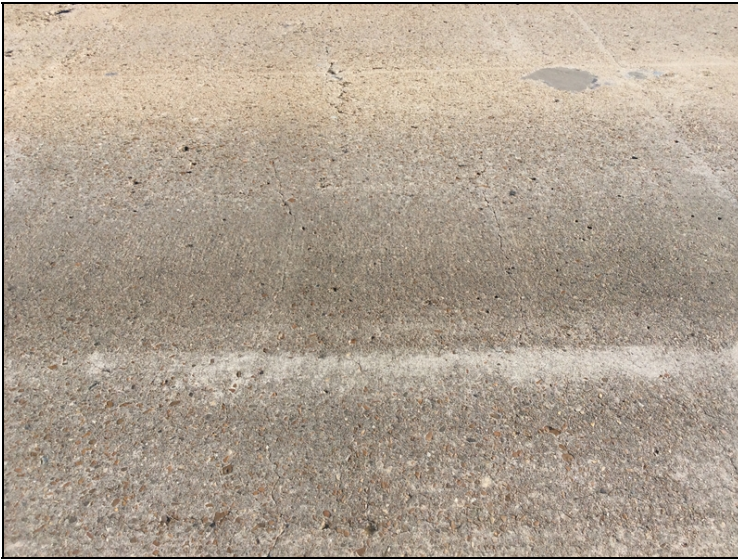
Typ. Cracking in Deck.
