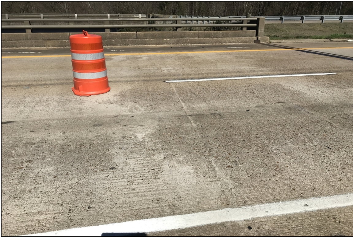
Span 5 large transverse cracks.
