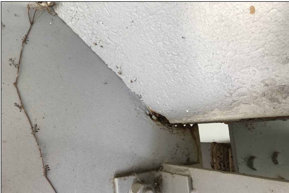
Bent 5 girder 6 has a hole in the haunch area. Girder 3 is the same on back side.
