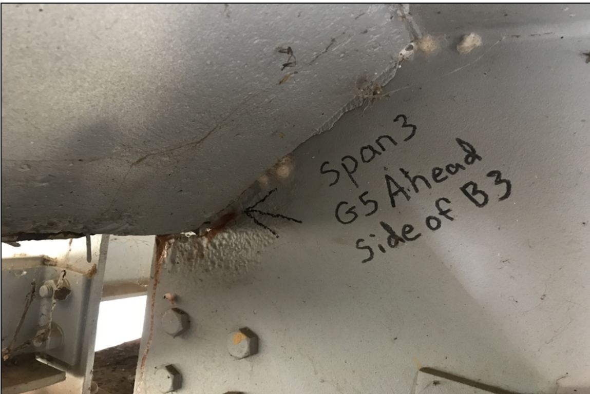
Span 3 Girder 5 ahead of bent 3 there is a crack in haunch area about an 1" long.
