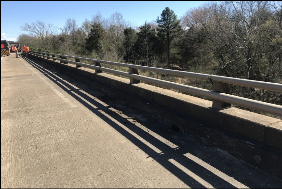
Typical condition of metal bridge rail.
