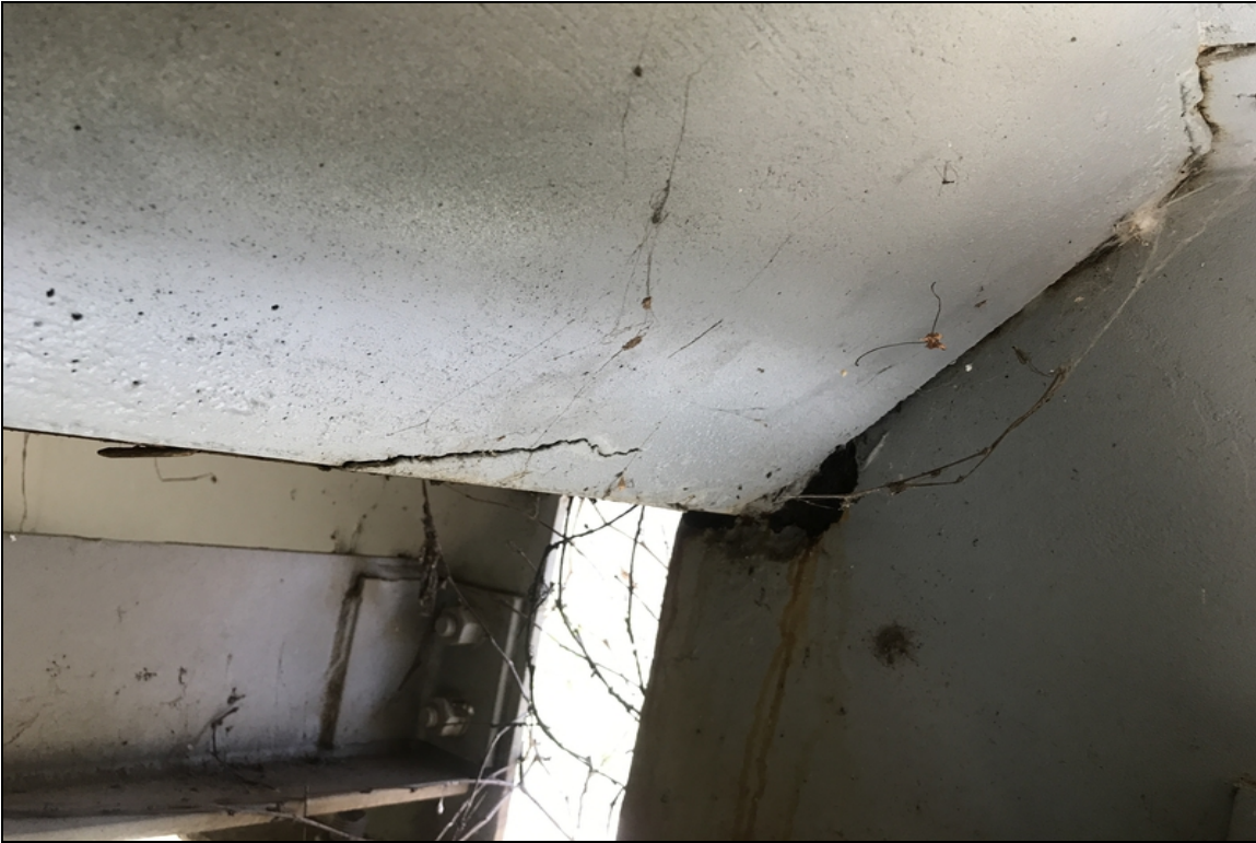
Bent 5 girder 7 has approximately 1/4" section loss in top of web in the haunch area. Girders 4 and 5 area the same. Back side.
