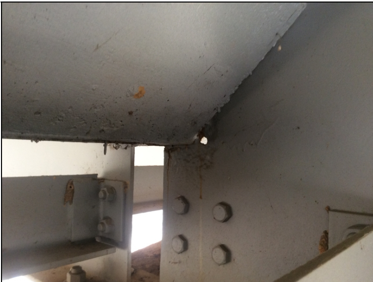
Pier #4, backside, beam #4, hole rusted through web at haunch area.
