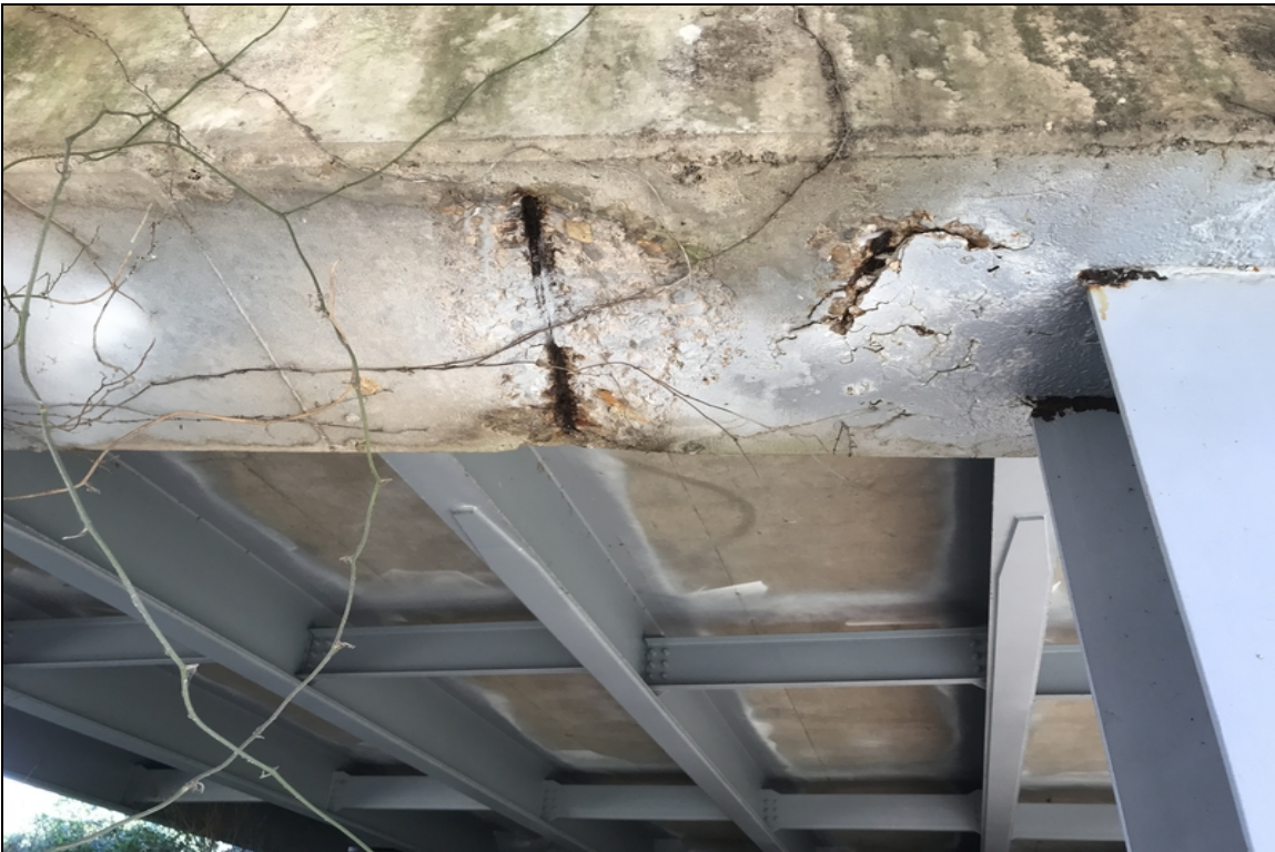
Bent 5 between piles 4 and 5 bottom of cap has a spall with exposed reinforcing steel.
