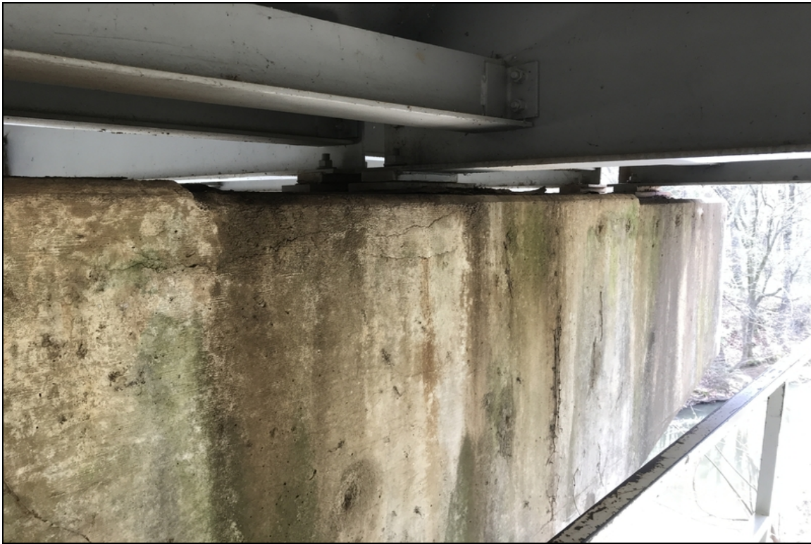
Bent 3 has horizontal cracking between girders 6 and 7. This is typical on back side of cap.
