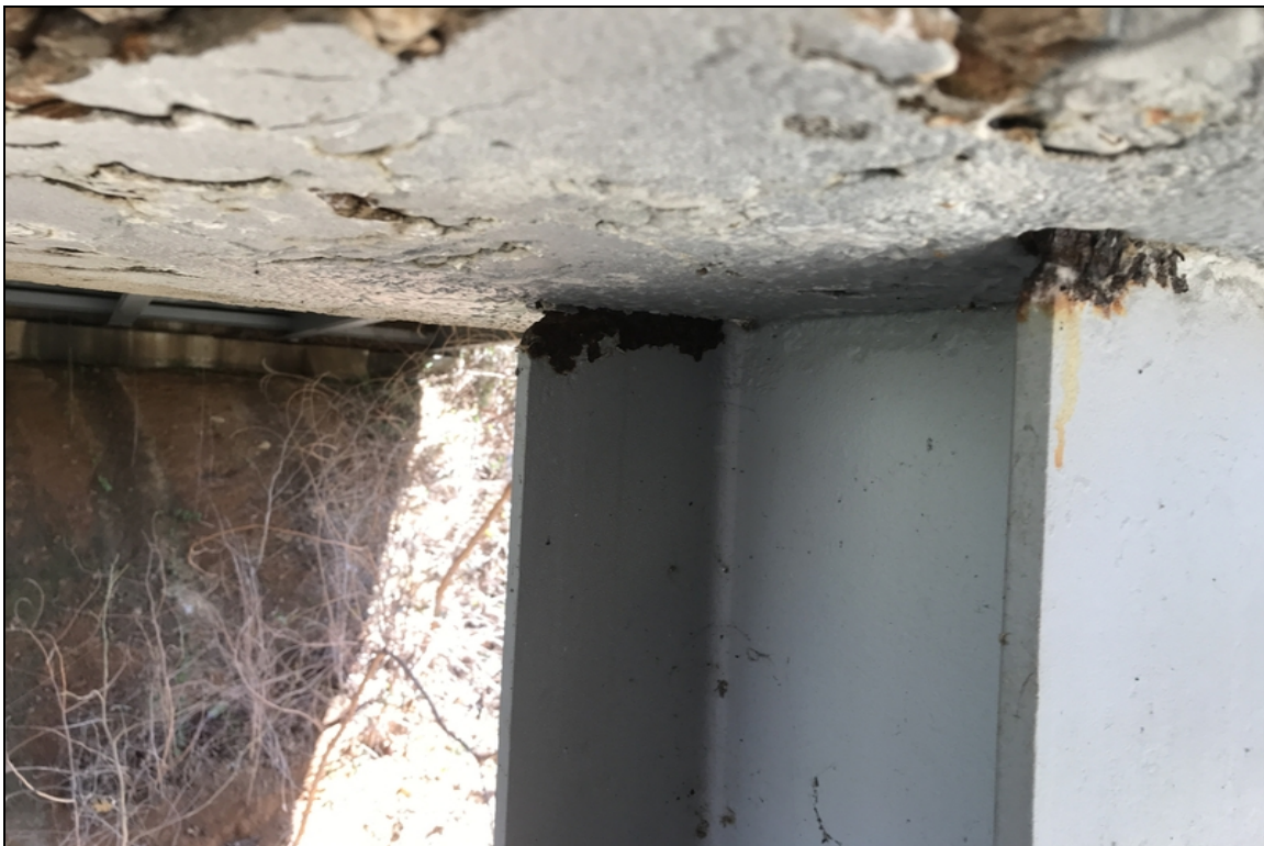
Bent 5 top of pile has section loss some up to knife edge.
