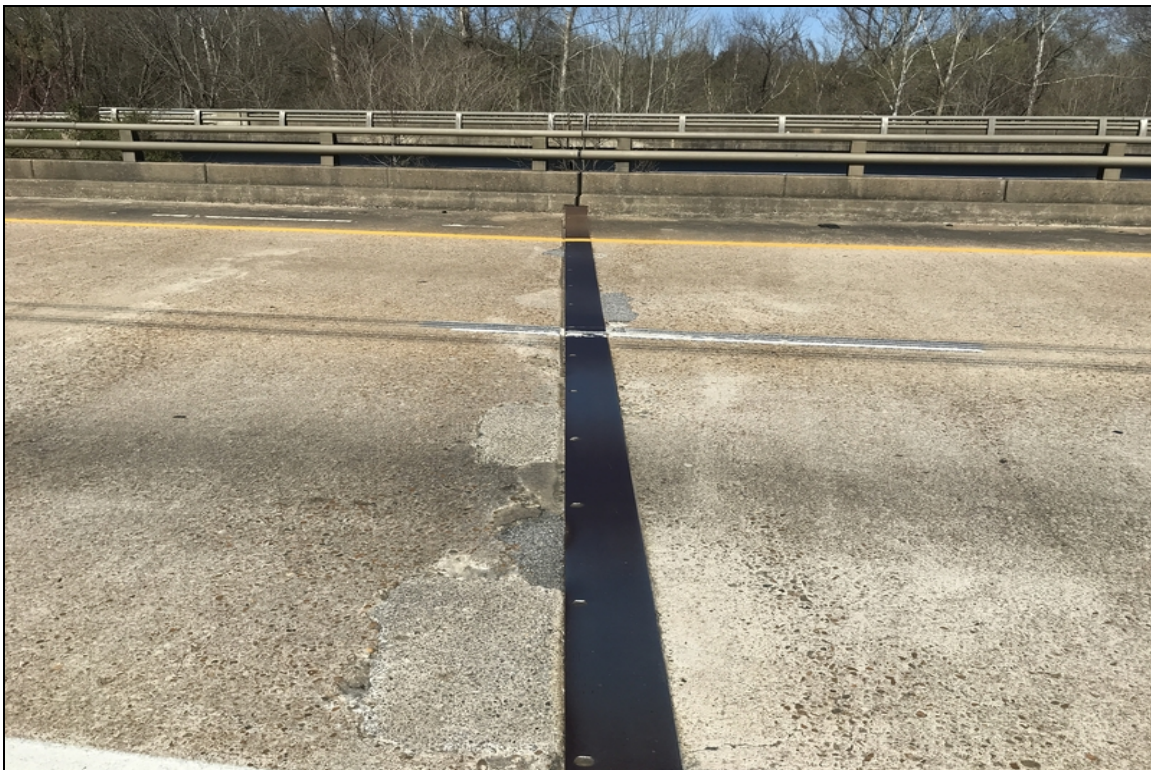
Bent 2 sound and unsound at assembly joint.
