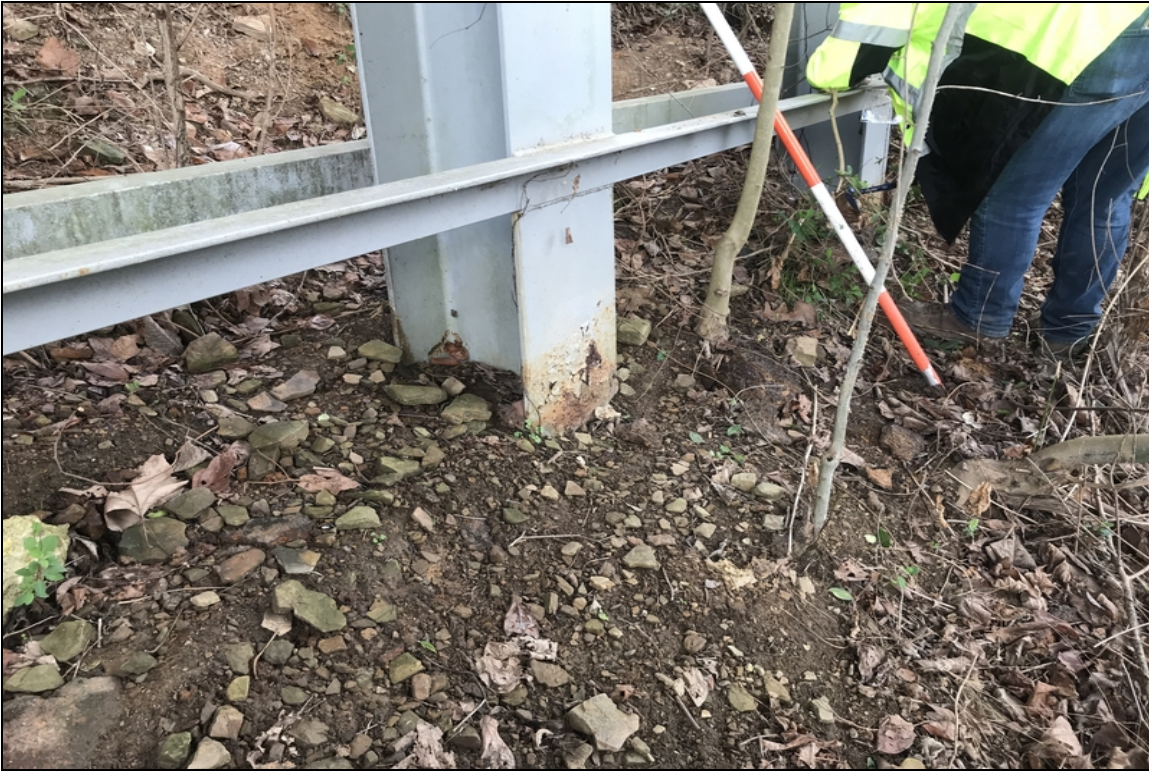
Bent 2 all steel piles have corrosion at ground level. Piles 2, 3, 5 and 7 have up to 1/8" section loss at ground level.
