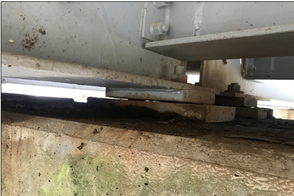
Moveable bearings at bent 3 have corrosion and some having pack rust. Bearings 4 back side and bearings 3 and 4 ahead side are floating.
