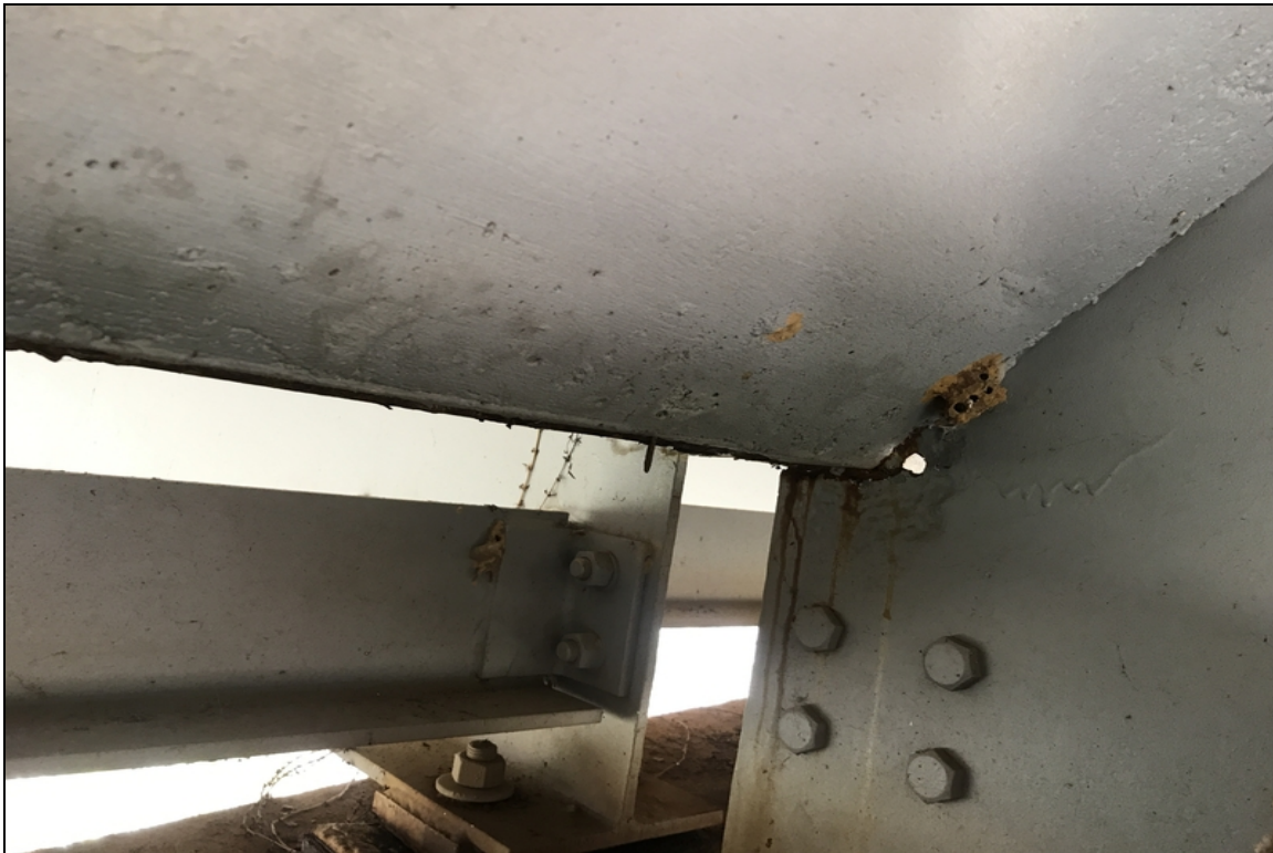
Bent 4 girders 3 and 4 on back side has holes in top of web in the haunch area.
