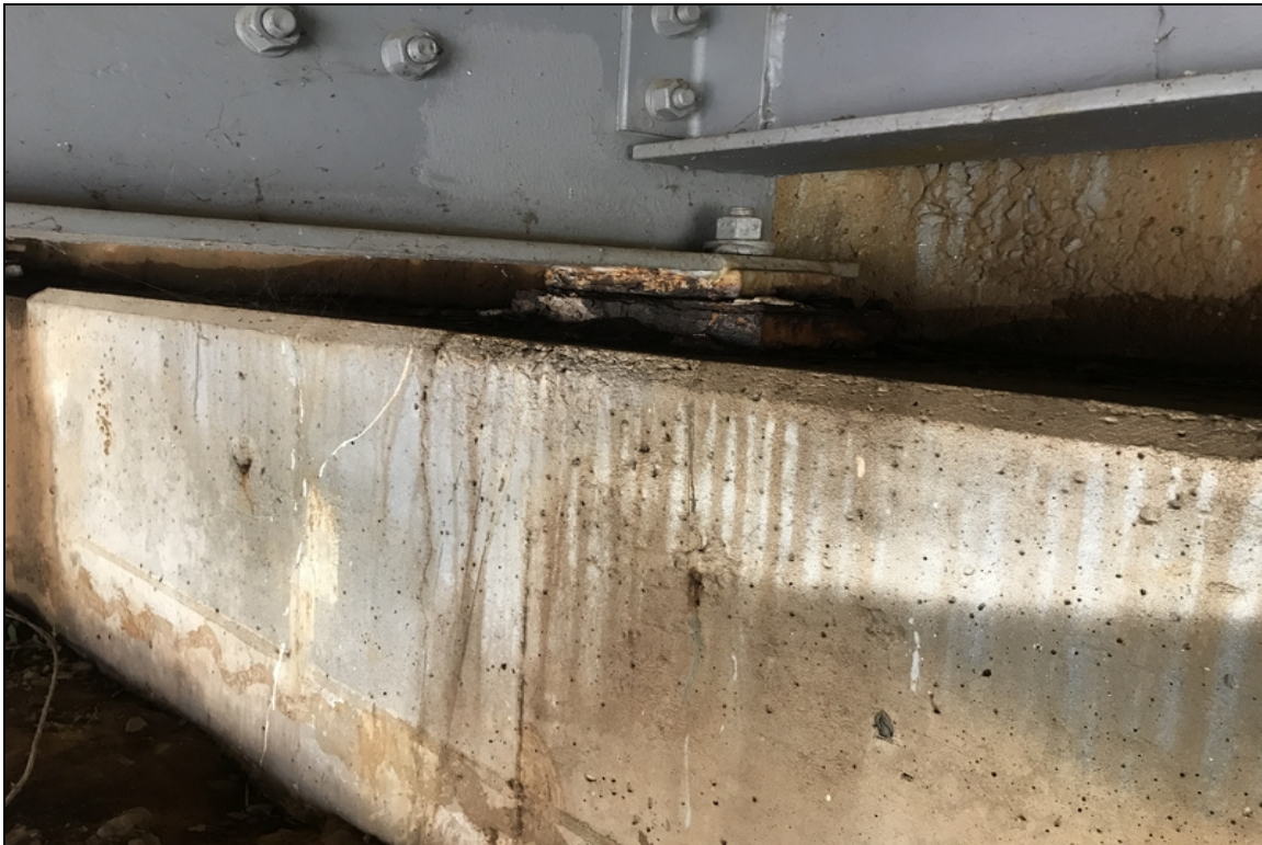
Bent 1 girder 4, bearing has corrosion with pack rust.
