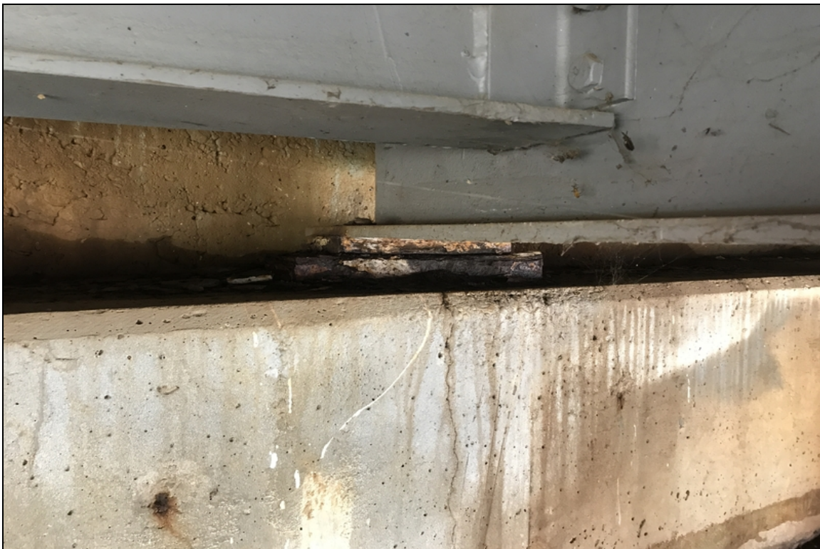
Bent 1 bearings 2 thru 4 are floating, making contact under load.
