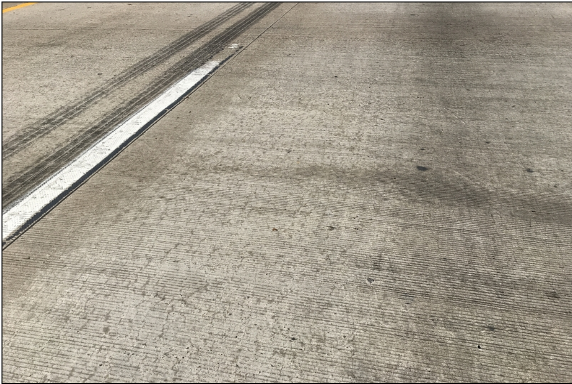
Typical map cracking in right lane in east approach.
