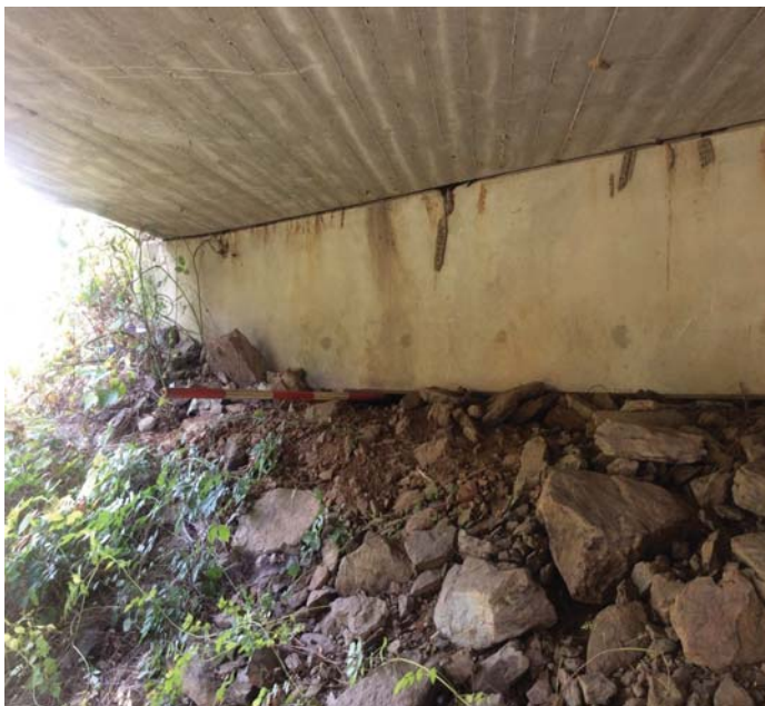
PHOTO 1 Description Undermining of cap. 2' behind face
