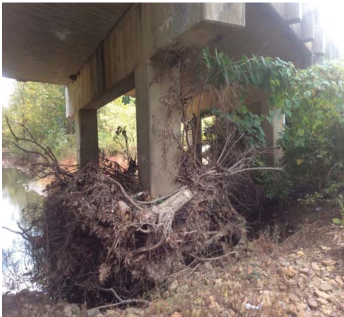
PHOTO 1 Description Drift on pier 2 upstream face
