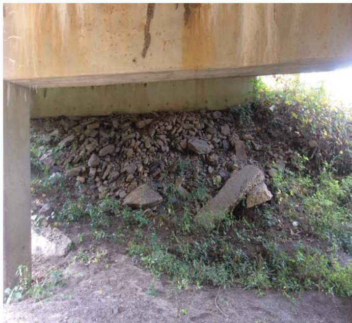
PHOTO 3 Description Riprap abutment 1
