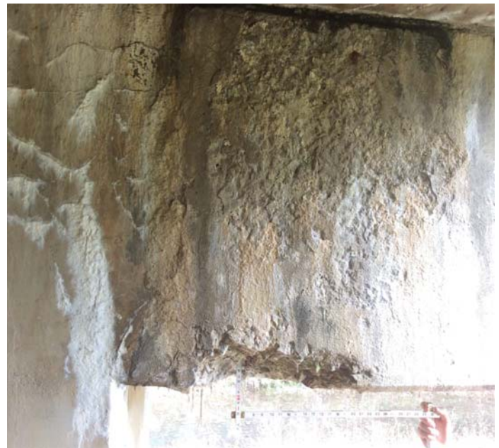
PHOTO 2 Description Spall pier 1 span 1 downstream
