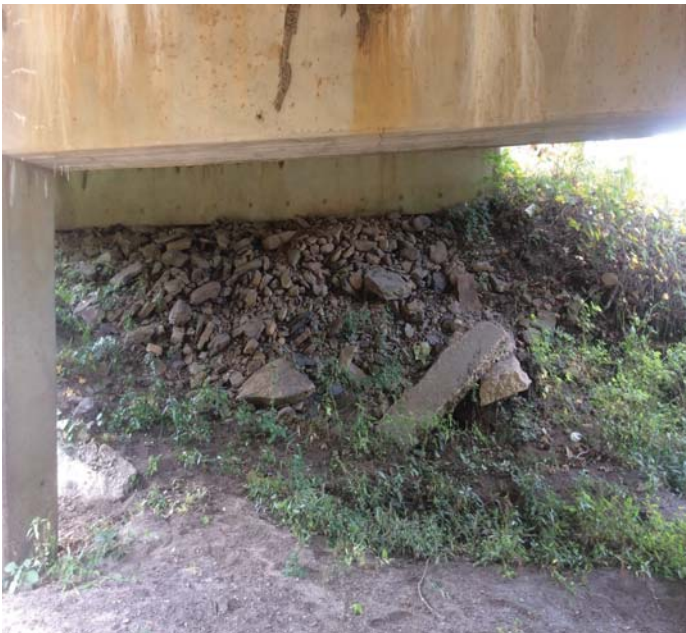
PHOTO 3 Description Riprap abutment 1
