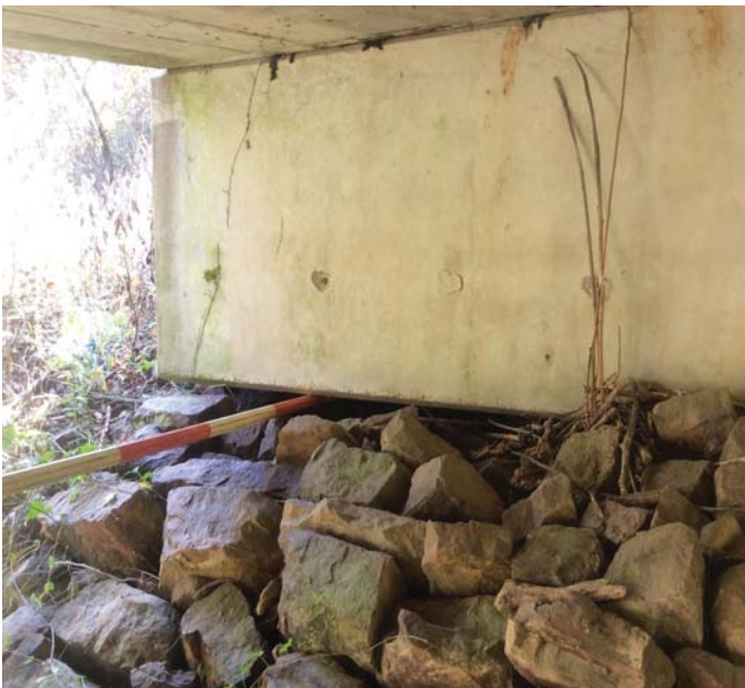
PHOTO 1 Description Ends of abutment undermined 2.5 ft back of face at wings for 6 ft.
