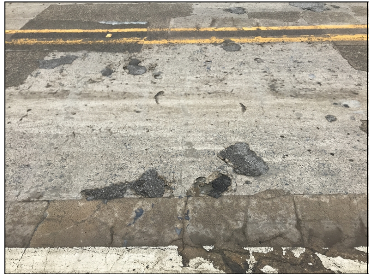
Typ. Delam, Cracking & Spalling in Deck.
