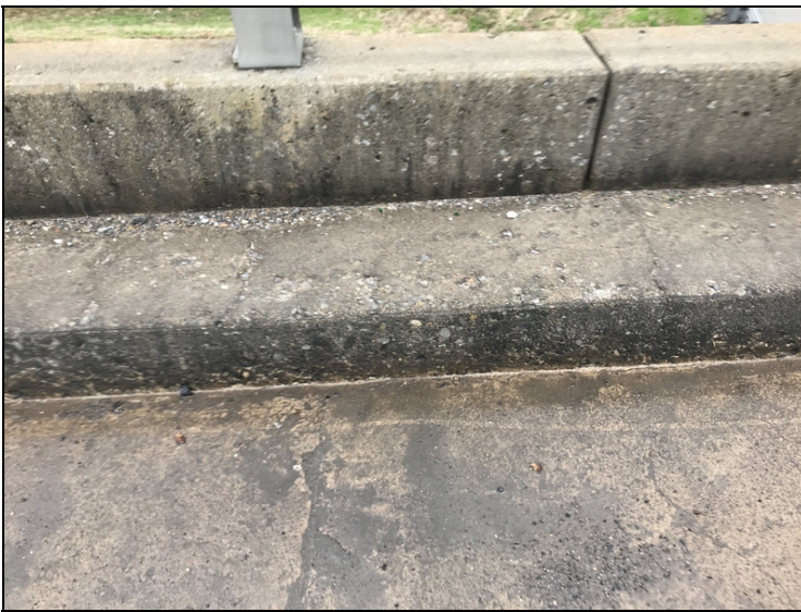
Typ. Cracking & Scale in Curbs under Rail.
