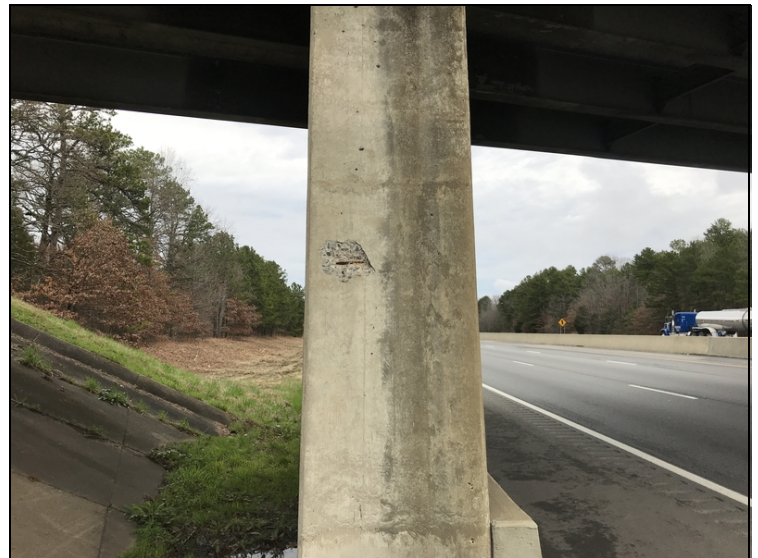
Typ. Delam & Spalling W / Rebar Exposed in Columns.
