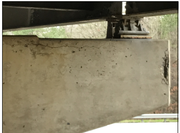
Typ. Cracking & Spalling in Faces of Caps.
