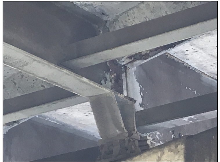
Typ. Rust & Section Loss on End of Beam 3.
