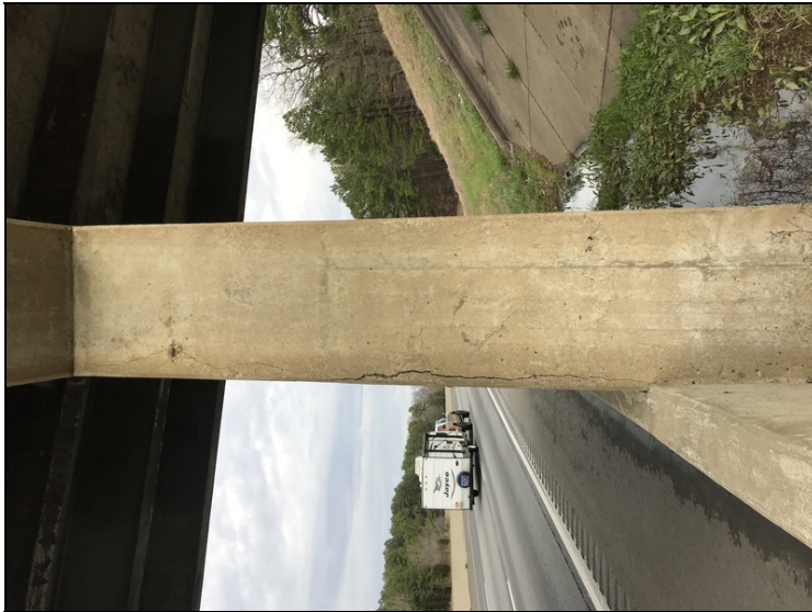
Typ. Cracking in Columns.
