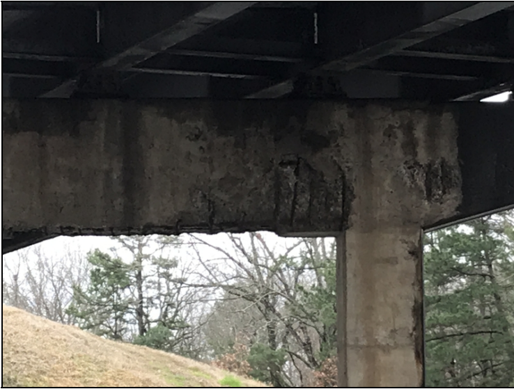
Delam, Cracking & Spalling W / Rebar Exposed in Ahd. Face of Cap 3.
