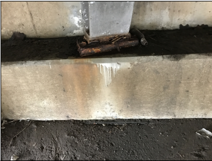
Typ. Rust on Bearings.
