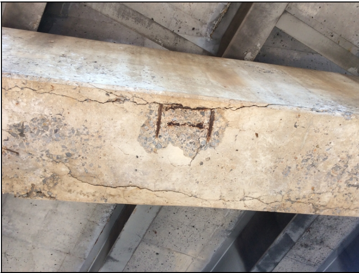
Dealm, Cracking & Spalling W / Rebar Exposed in Bt. Face of Cap 3
