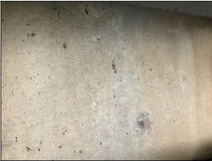
Typ. Cracking in Back Walls.
