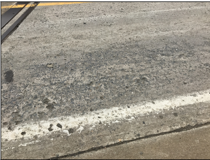
Typ. Condition of Approach Slabs.
