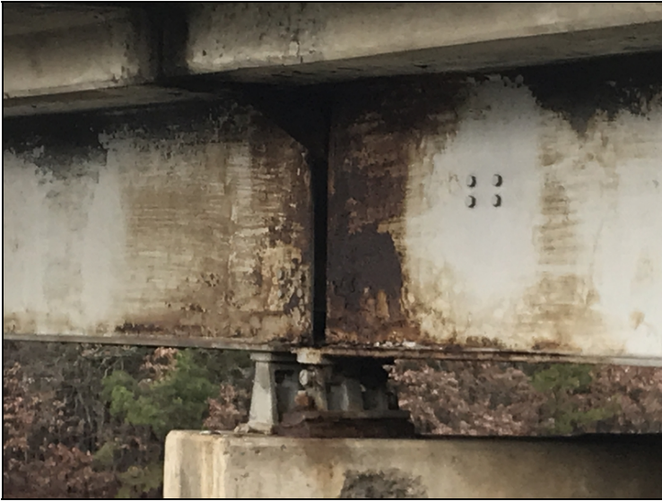
Typ. Rust on Ends of Beams.
