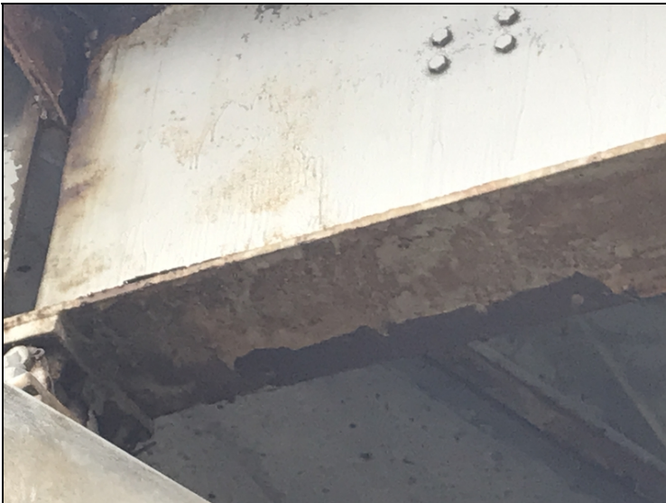
Typ. Rust on Ends of Beams.
