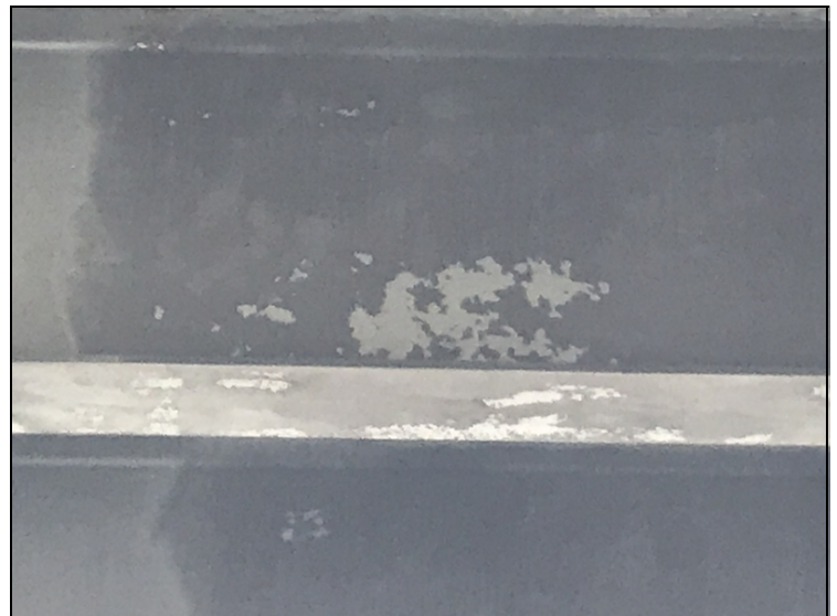
Typ. Chalking & Peeling of Paint on Beams.
