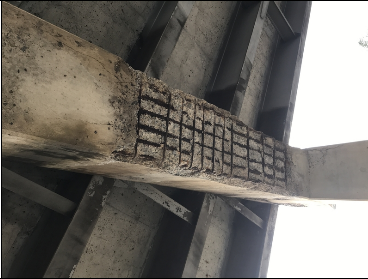
Dealn, Cracking & Spalling W / Rebar Exposed in Bt. Face of Cap 3
