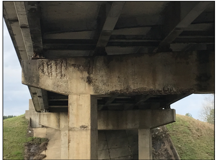
Typ. Condition of Bk. Face of Cap 3.
