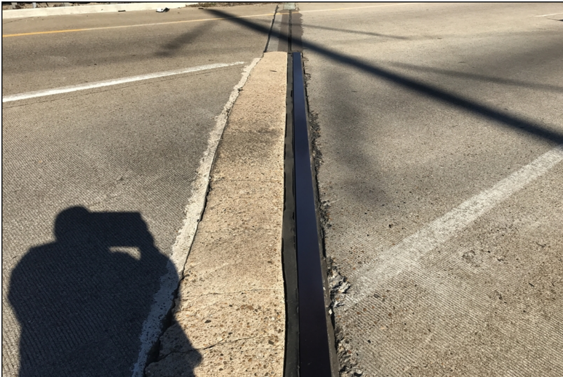
Abutment 1 joint material
