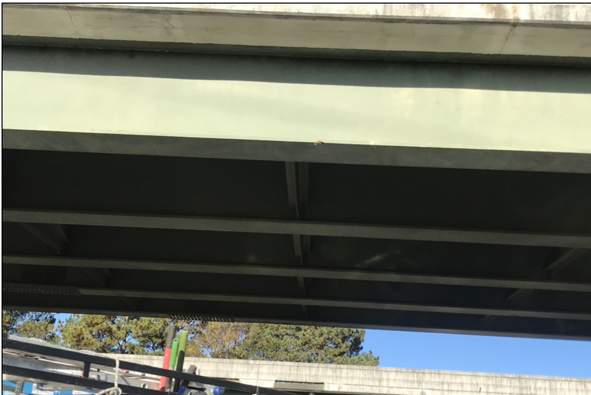
Girder 5 span 2 traffic impact to bottom flange
