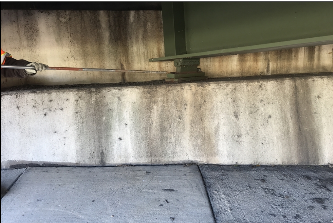
Abutment 2 bearing 2 anchor bolt, broke off and top 1/2 bolt and nut is missing.
