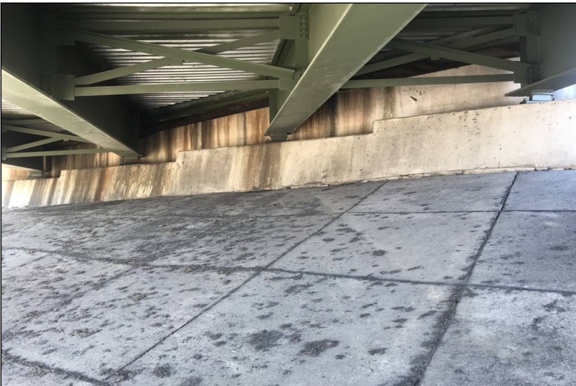
Abutment 1 cap joint leaking
