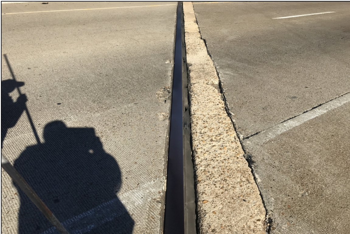
Abutment 2 joint material
