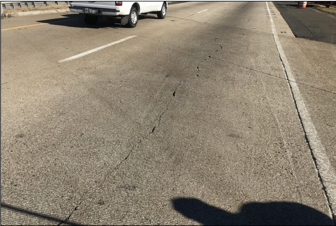
Crack in approach slab
