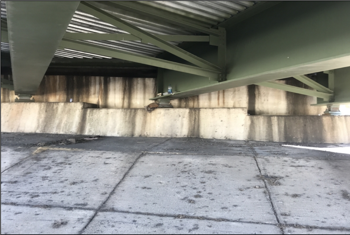
Joint leaking on to cap
