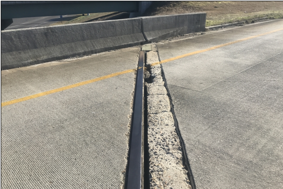
Spall at abutment 1, joint.
