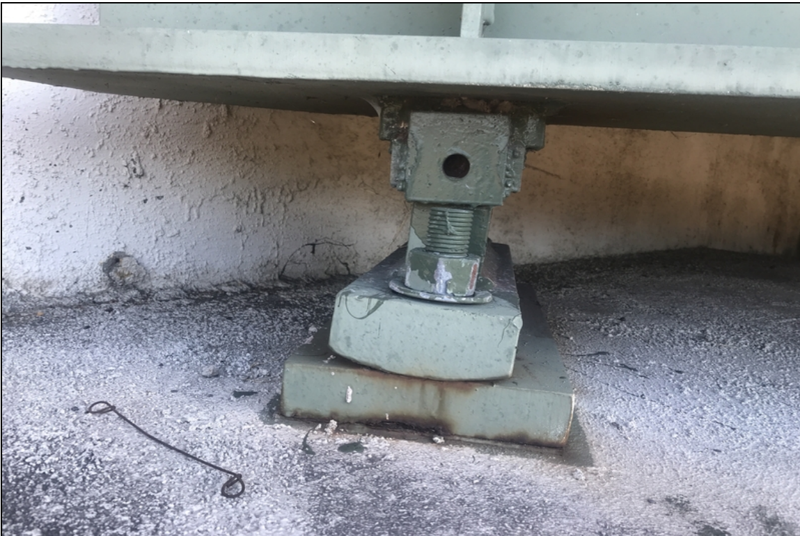
Bolts missing in bearings, abutment 4, 1 and 4. Abutment 1 girder 2 missing bolt also.
