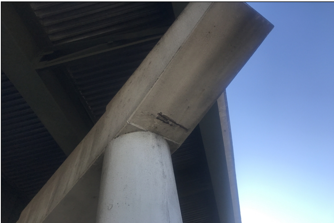
Bent 2 left spall with exposed rebar.
