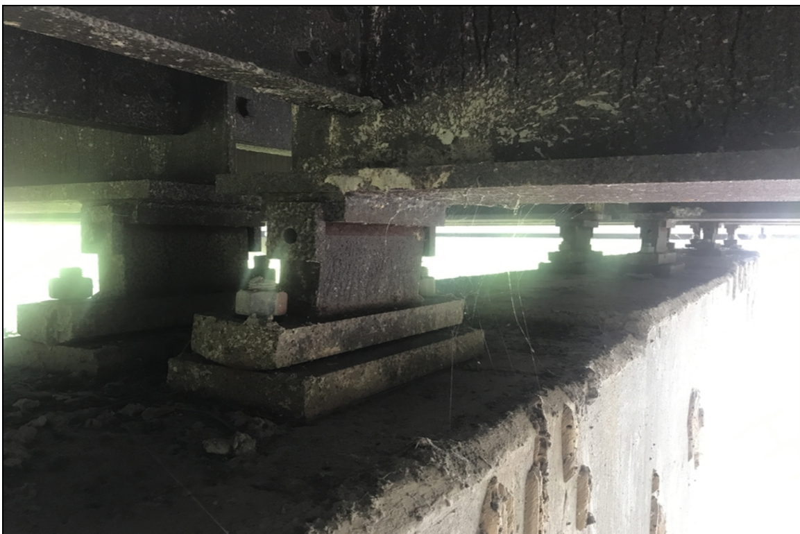
Span 18 bent 19 bearing 3, 4 and 5 missing top bolts on left side
