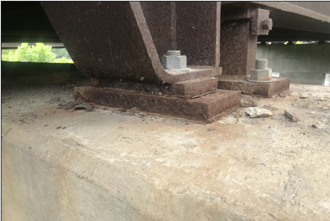
Bent 20, beam 1, light flaking rust on bearings.
