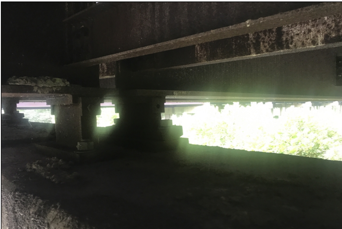
Missing bolt span 17 bent 18 bearing 4 also not pictured also bearing 1
