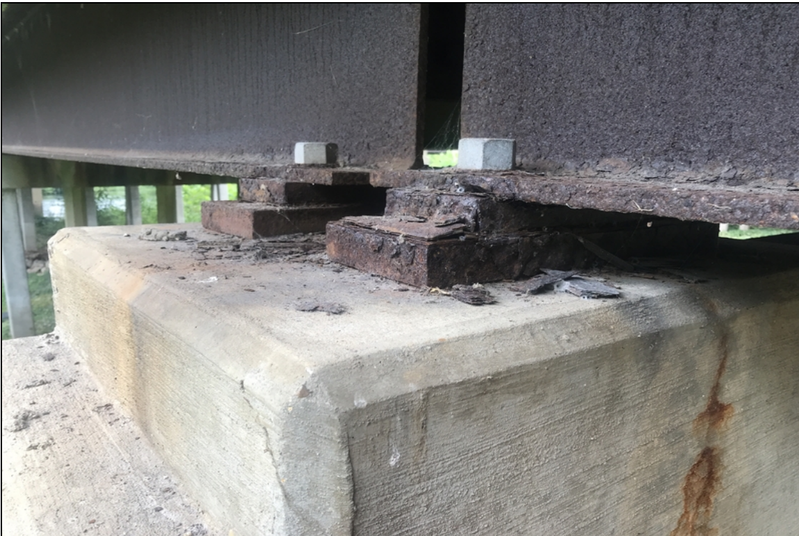
Bent 15 bearing 1 flaking rust
