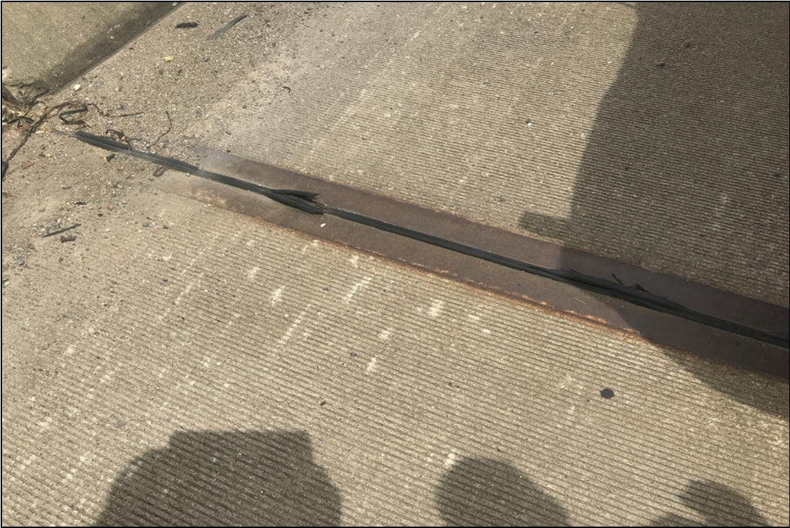
Bent 5 joint seal tore
