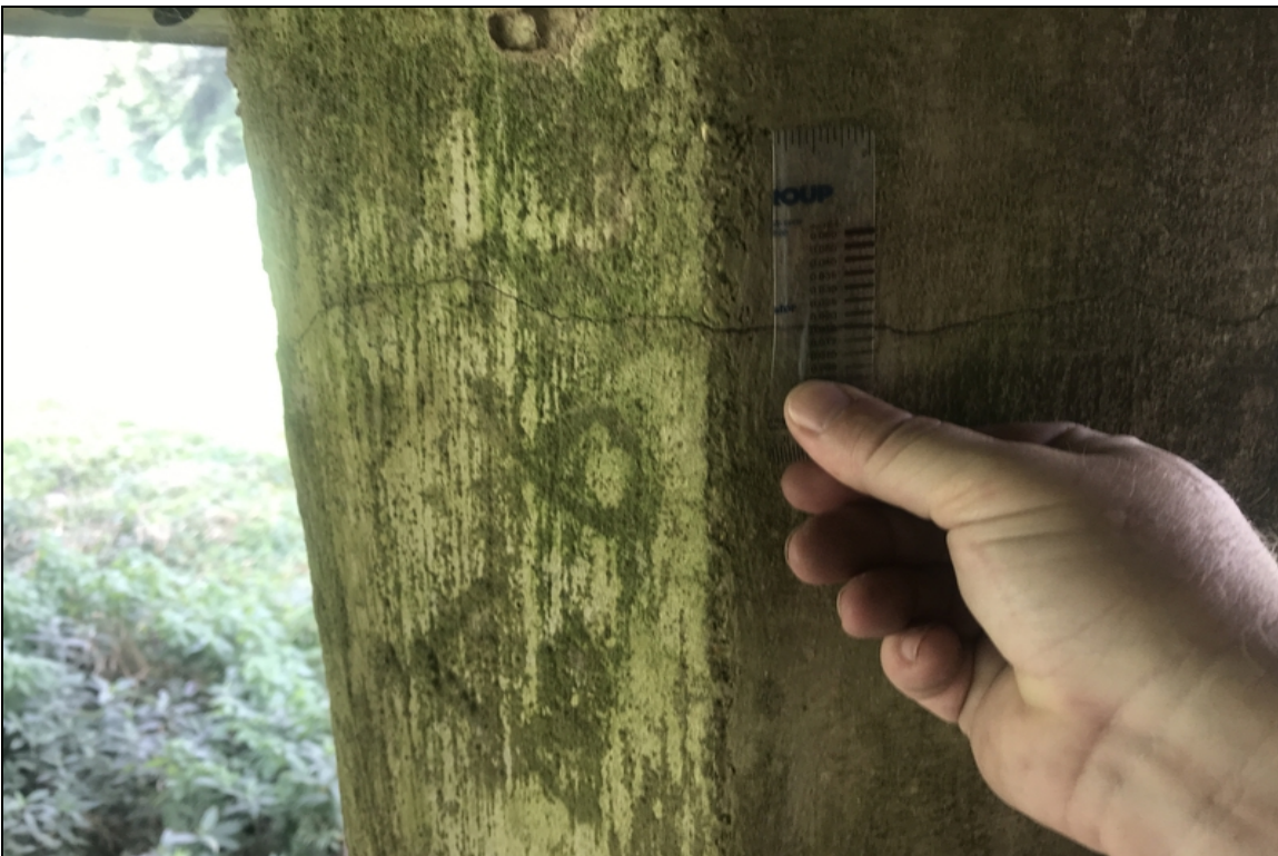
Crack pile 3 bent 14
