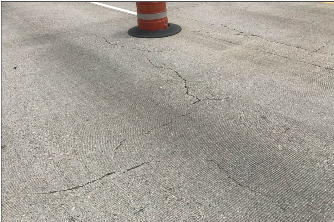
Approach slab cracks
