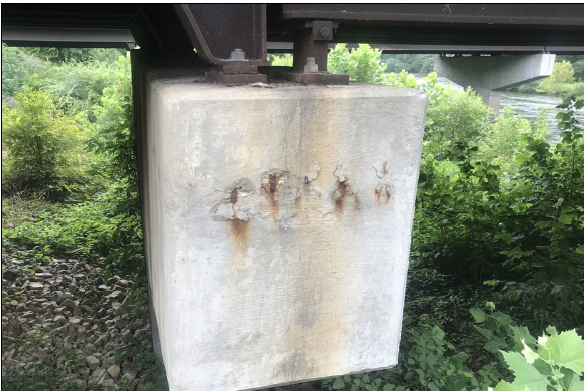
Left end of cap at bent 20, spall with exposed rebar.
