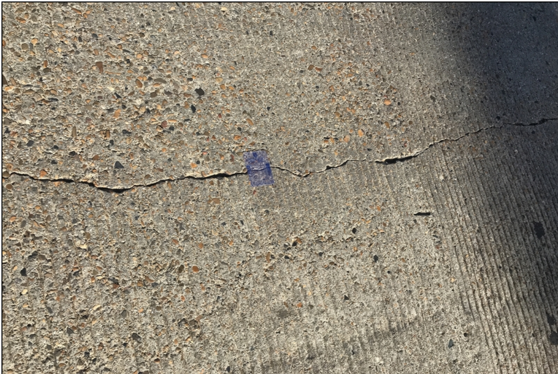
Longitudinal deck cracks, all span, 0.060-0.070
