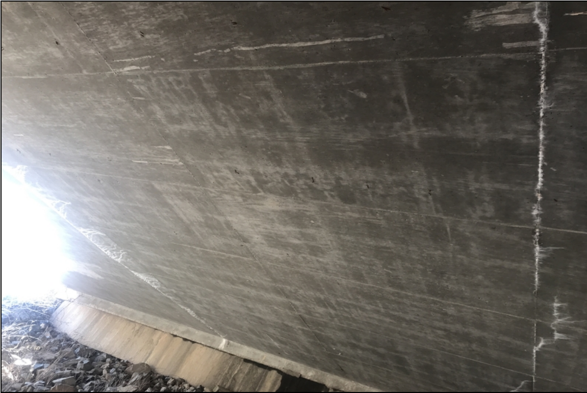
Soffit, cracks with efflorescence.
