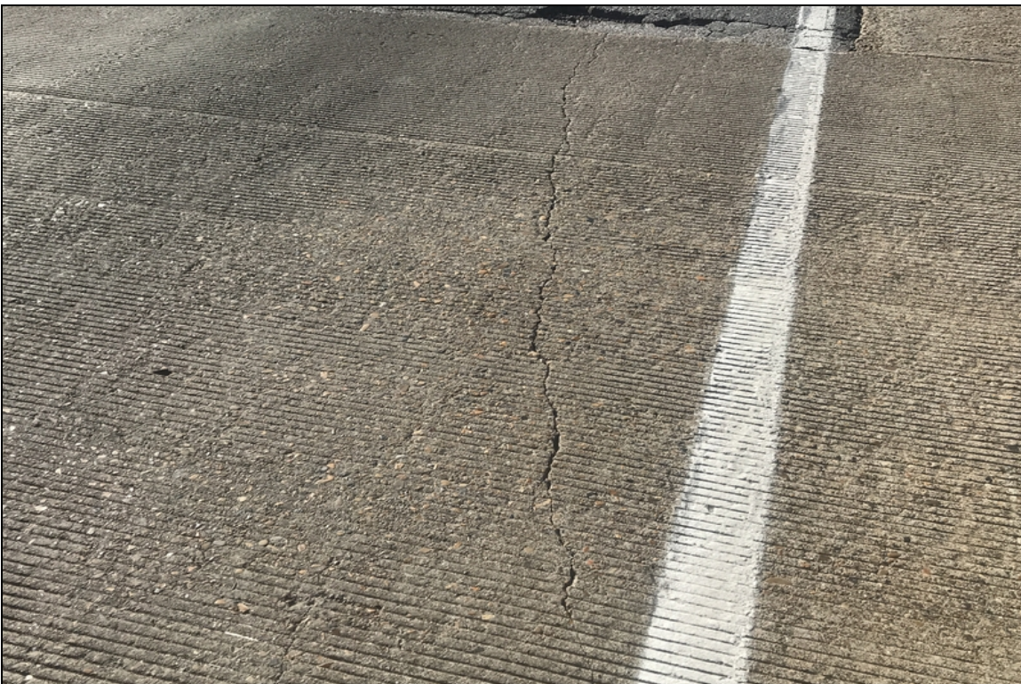
Span 1, deck cracks.
