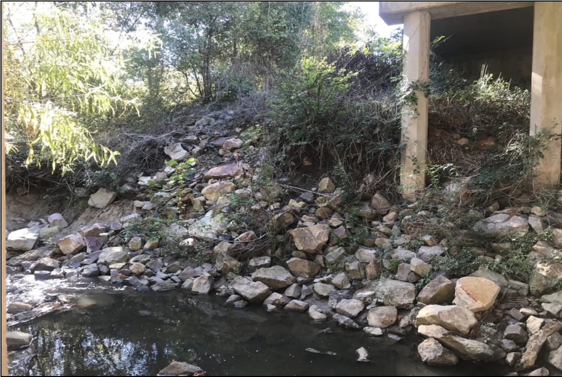
Bent 2, pile 7, erosion around pile and down stream.
