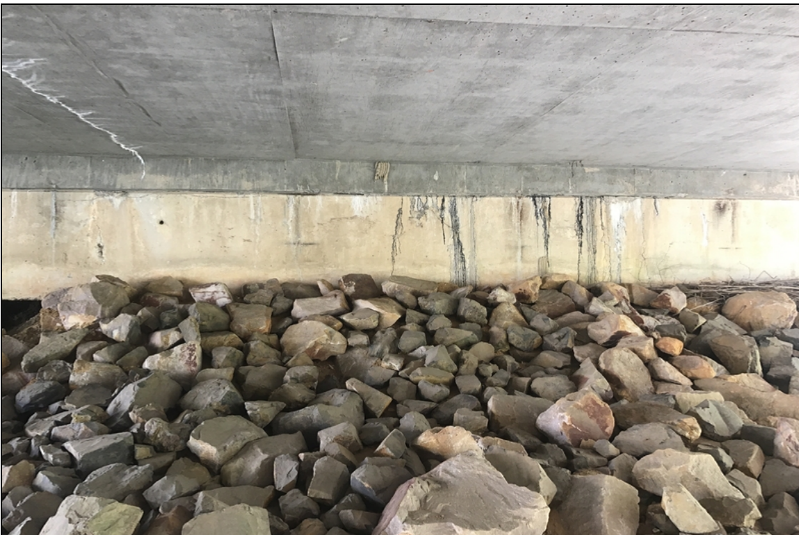
Abutment 5, cracks in back wall
