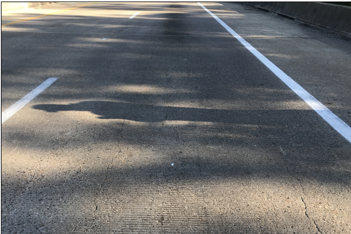
Span 1 longitudinal cracks.
