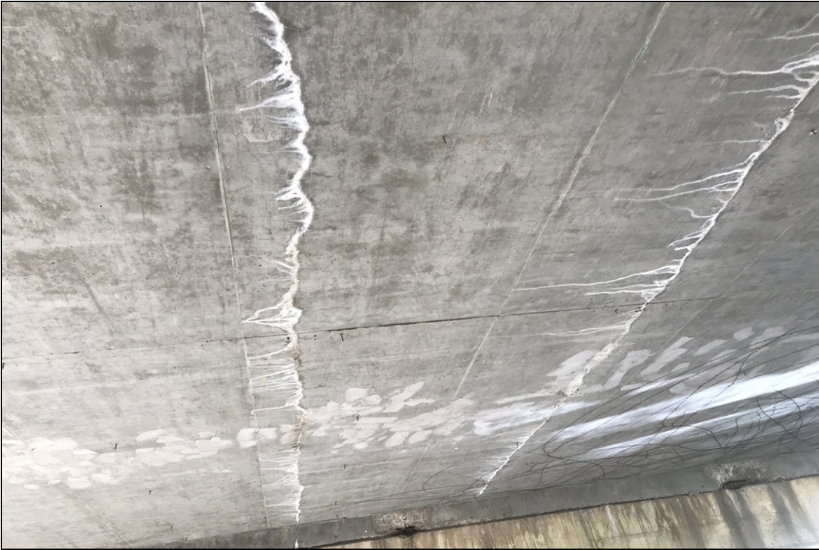
Span 3, soffit cracks with light efflorescence
