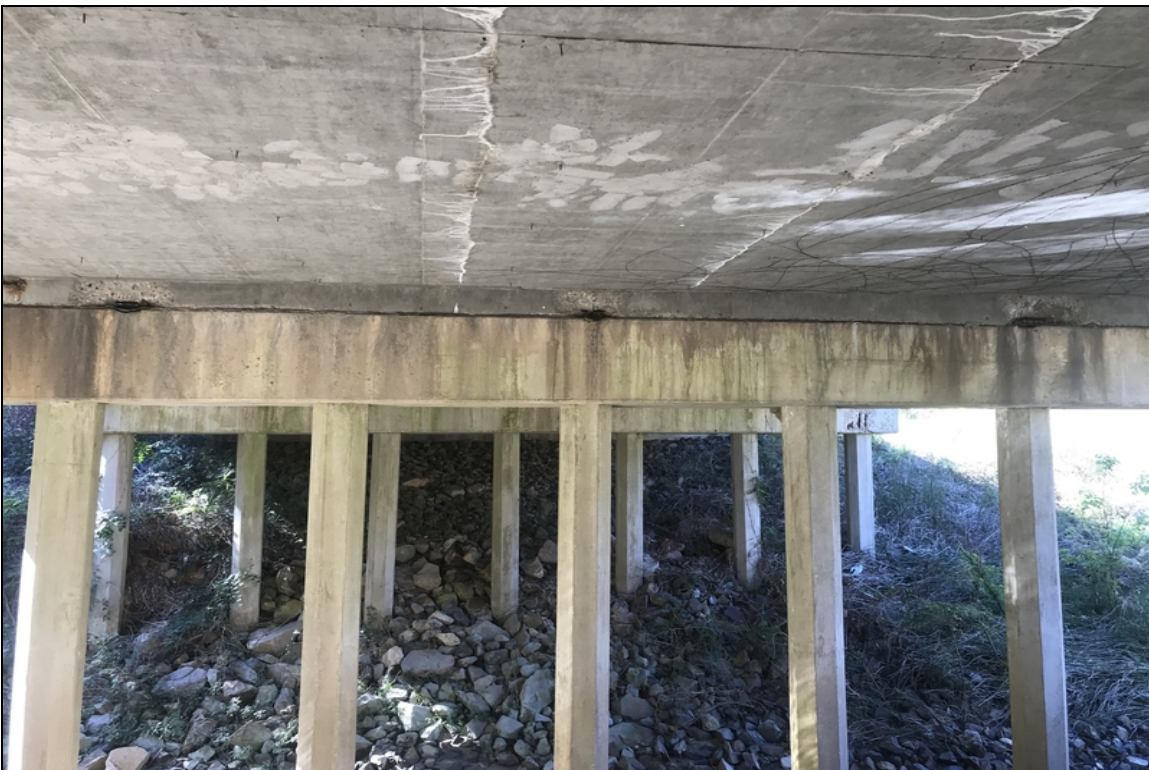
Bent 3, spalls with exposed rebar, ahead side.
