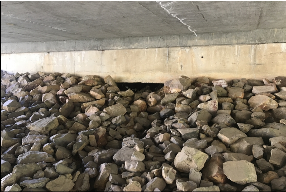
Abutment 5, erosion under cap and down slope.
