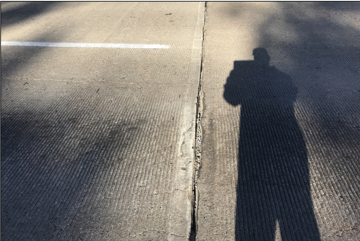
Joint 3, seal missing.
