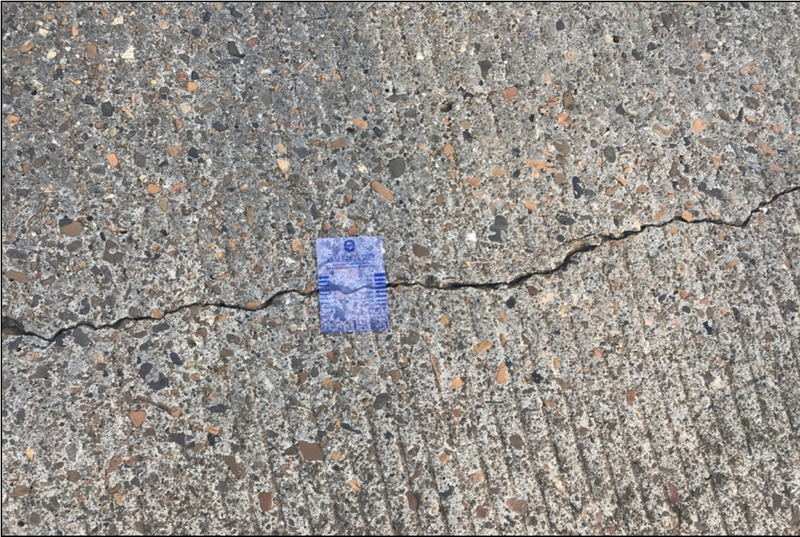
Deck cracks, 0.070
