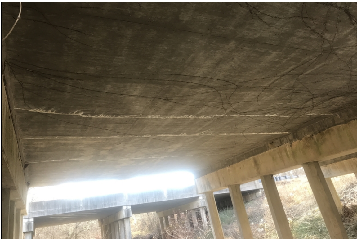
Soffit span 3, cracks with light efflorescence.
