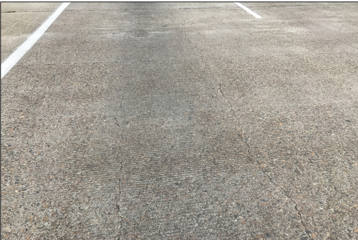
Cracks Span 1.
