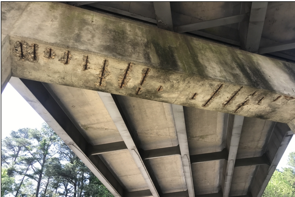
Bent 3, cap with exposed rebar.
