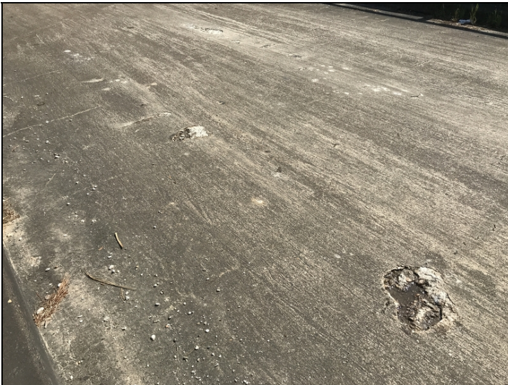
Span 3, deck spalls cracks and exposed rebar
