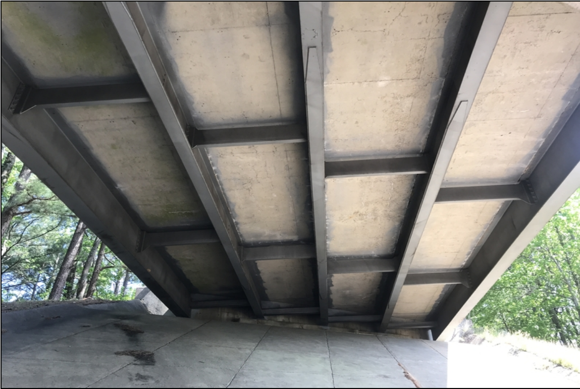
Span 4 soffit, deck cracks with efflorescence
