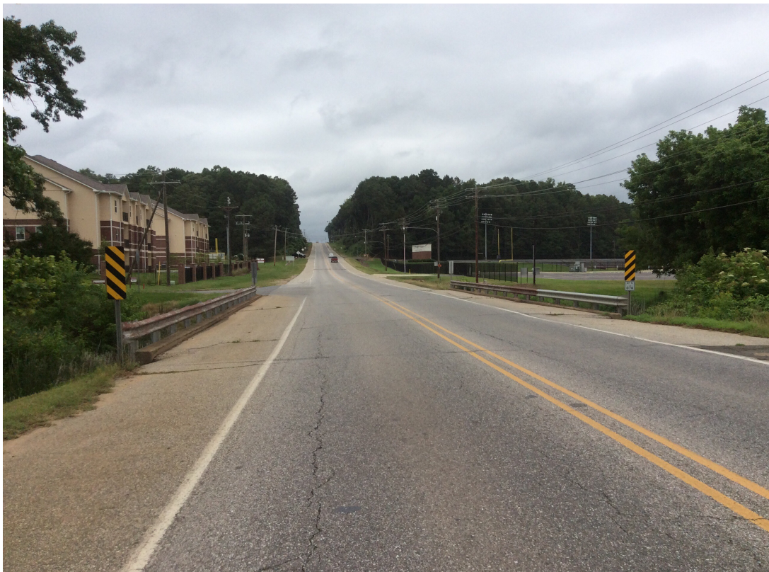
9 inch's of asphalt overlay on bridge deck
