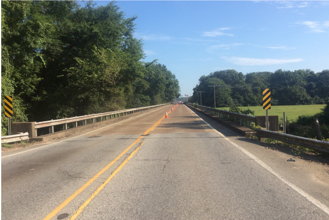
No overlay on bridge deck
