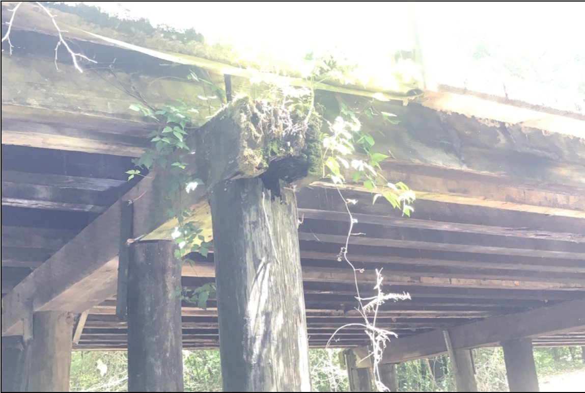
Bent 9 cap right end decayed and top of pile 7
