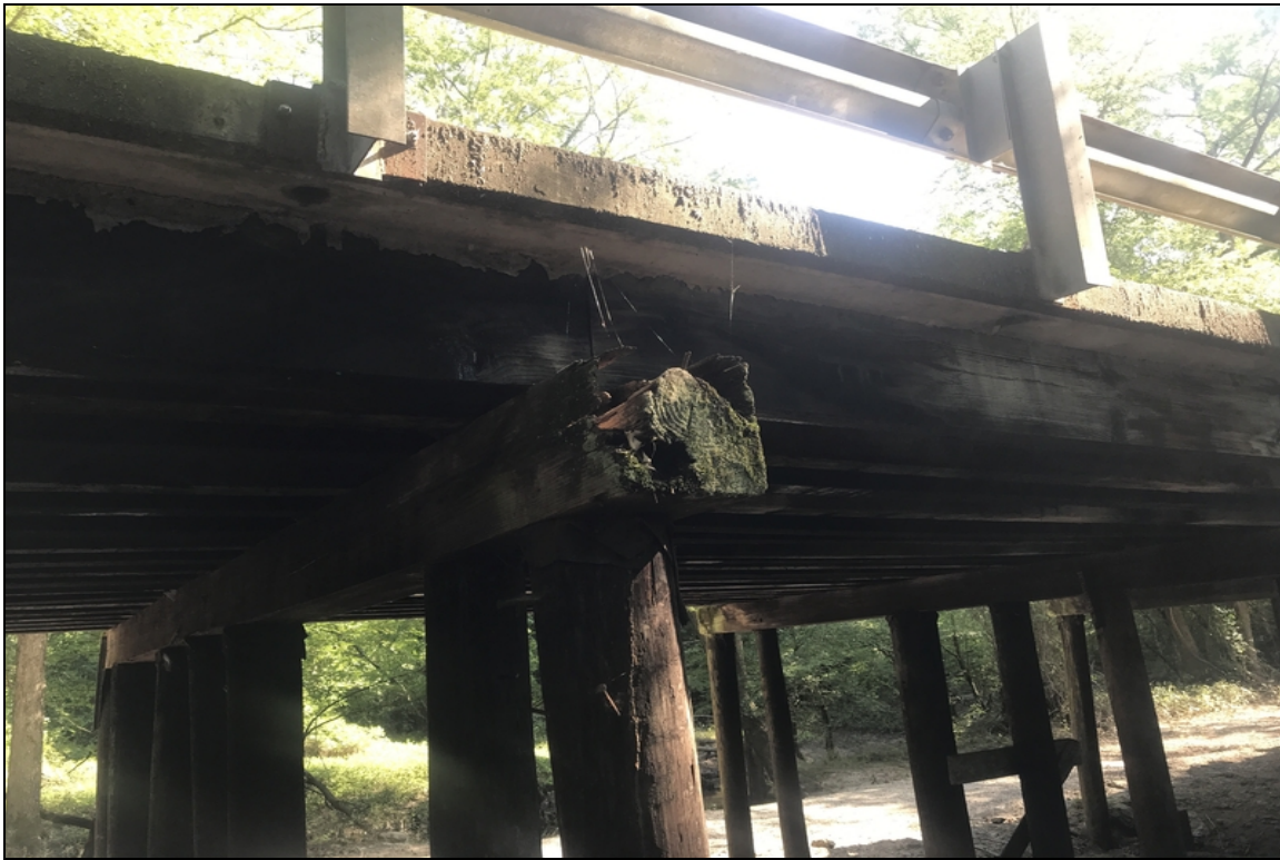
Bt 3 cap right end, decayed.
