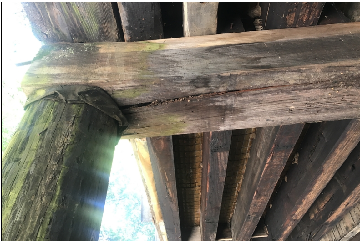
Bent 8, left end of cap crushing over pile 1.
