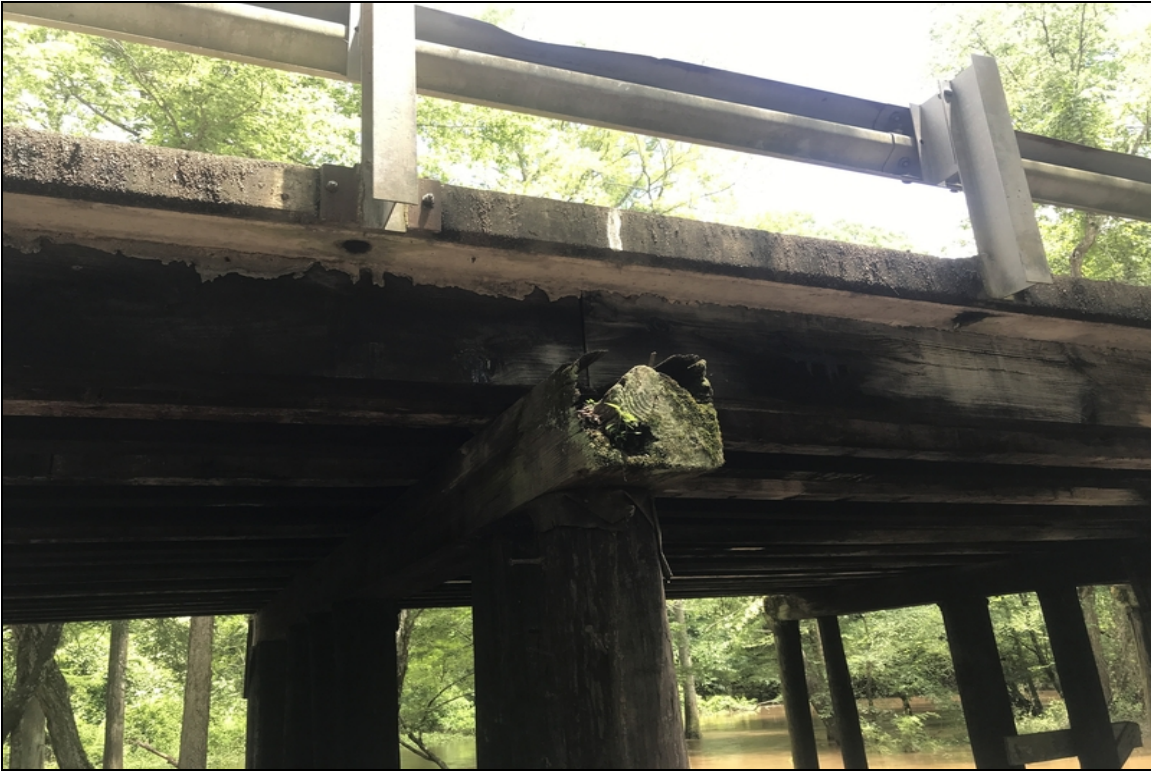
Right end of cap bent 3, decay
