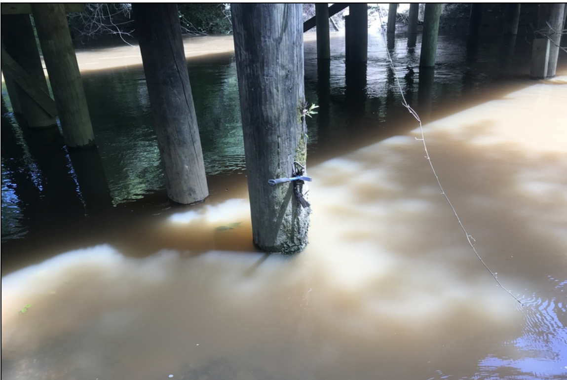
Bent 9 pile 7, decayed at cap and 3 feet from ground line
