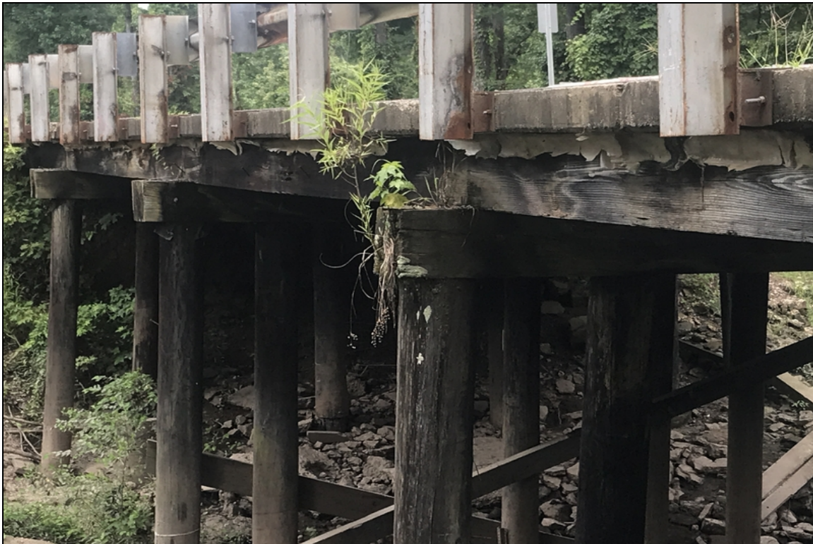
Bent 4 right side cap has decay on outside 1 foot
