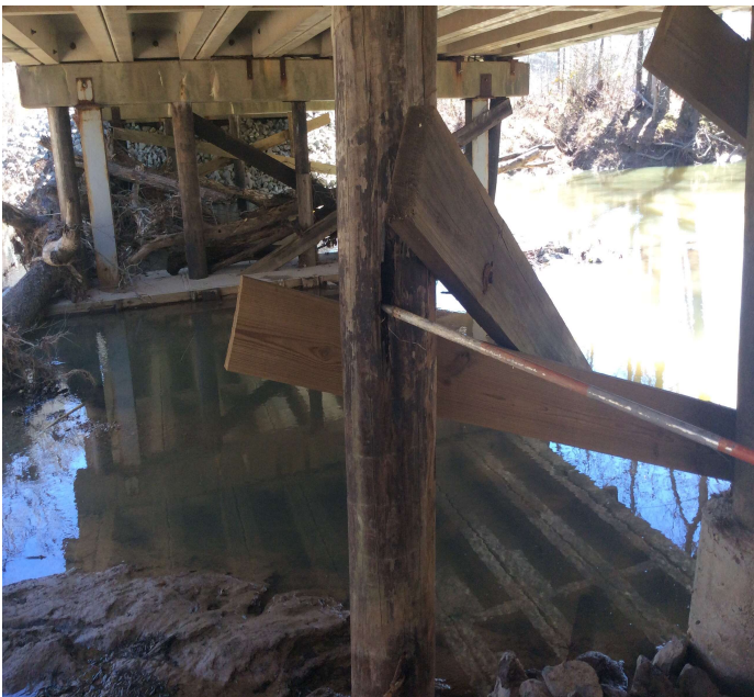
PHOTO 1 Description Bent 2 Pile 2 rotten spot
