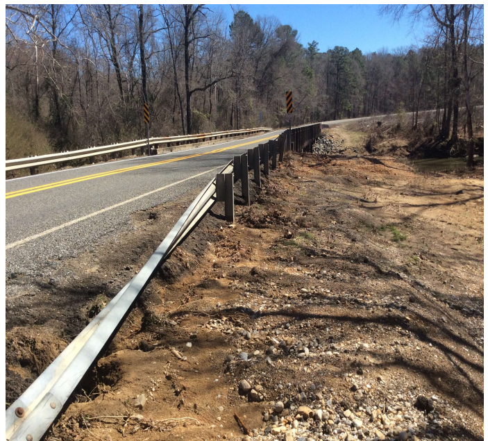
PHOTO 2 Description Erosion right side at abutment 1
