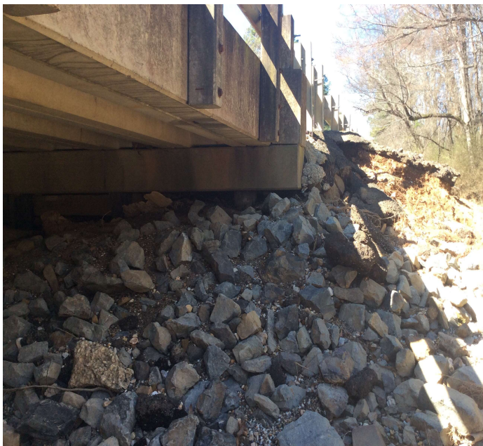
PHOTO 1 Description Scour at abutment 1.
