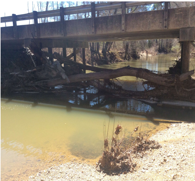
PHOTO 1 Description Drift bents 3 and 4.
