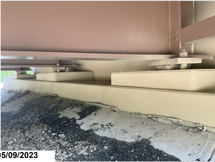
Bent 1 bearings.
