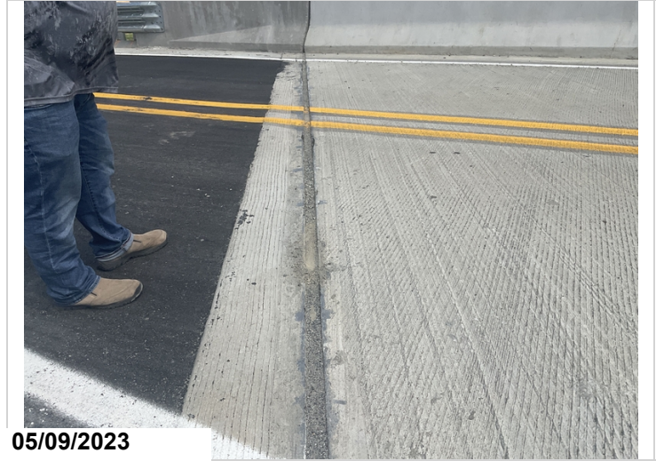
Bent 3 joint full of debris.
