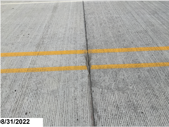
Sawed construction joints full of Debris and missing D -200
