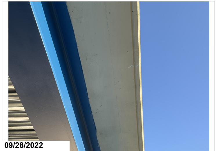
Span 1, right side of overhang has a transverse crack with efflorescence staining. Each span has several similar cracks with efflorescence staining.
