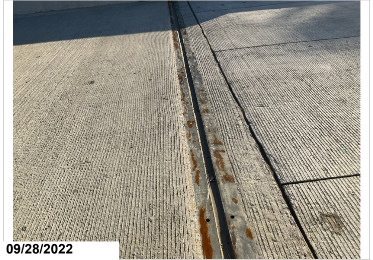
Bent 1: joint seal
