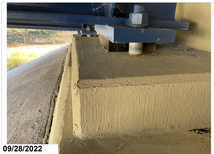
Bent 1, girder 2: elastameric bearing. Common
