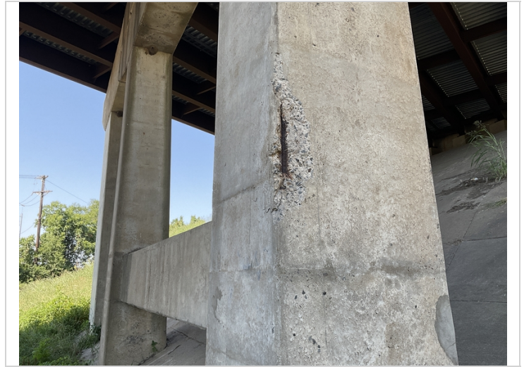
Bent 2 column 2 exposed rebar
