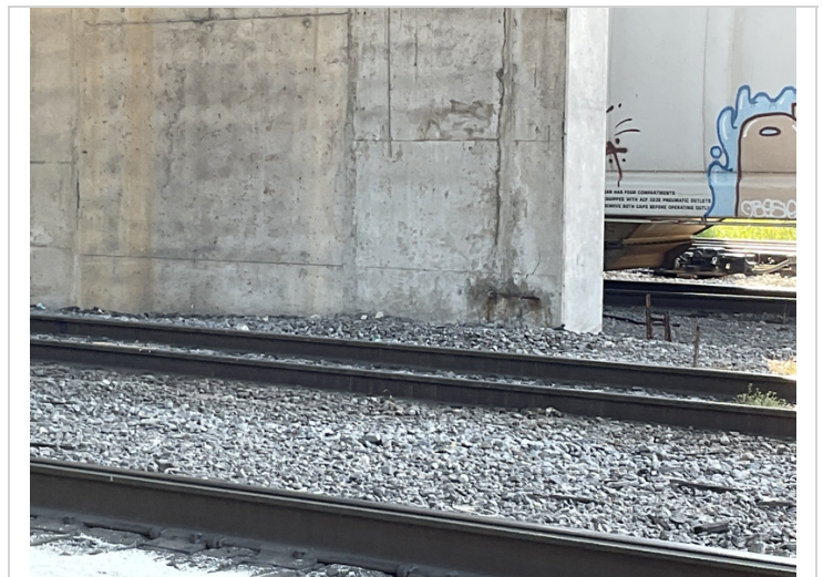
Bent 4 exposed rebar on bottom right side of pier wall
