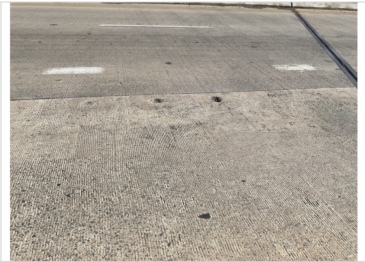
Small spalls in span 4
