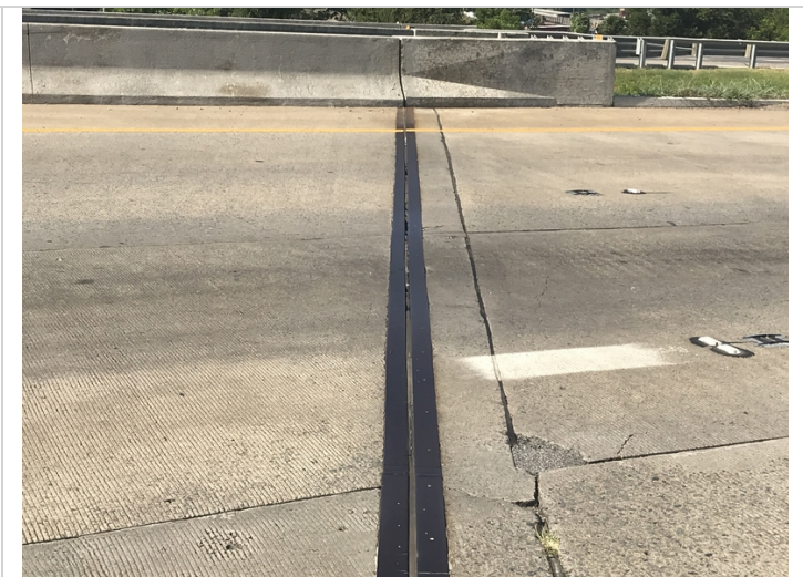
Bent 1: approximately 6 foot of joint seal missing, allowing water to freely flow through
