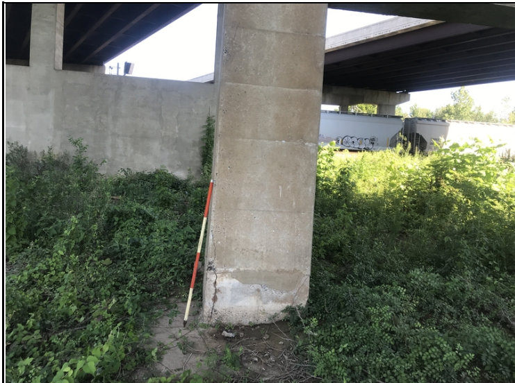
Bent. 6 , column 3: large vertical crack.
