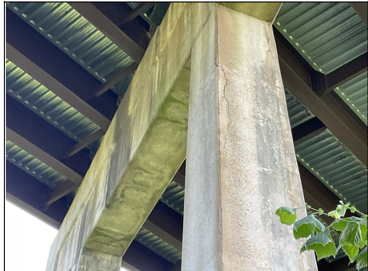
Bent 7 column 3 crack
