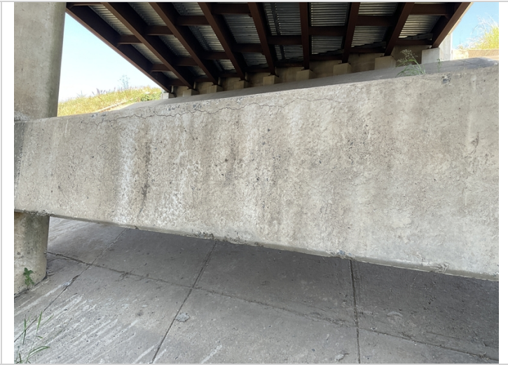
Bent 2 cracks in cross brace (pier wall)
