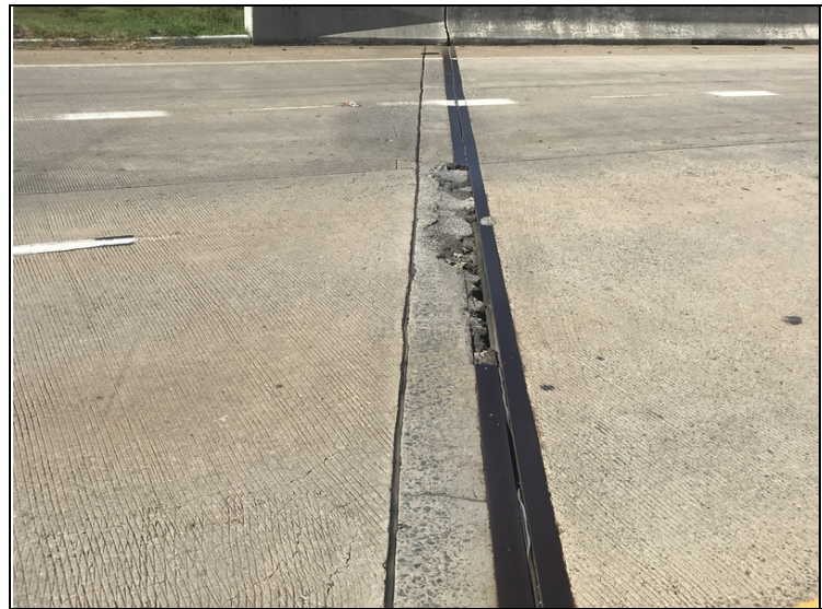
East abutment has spalls at top of back wall.
