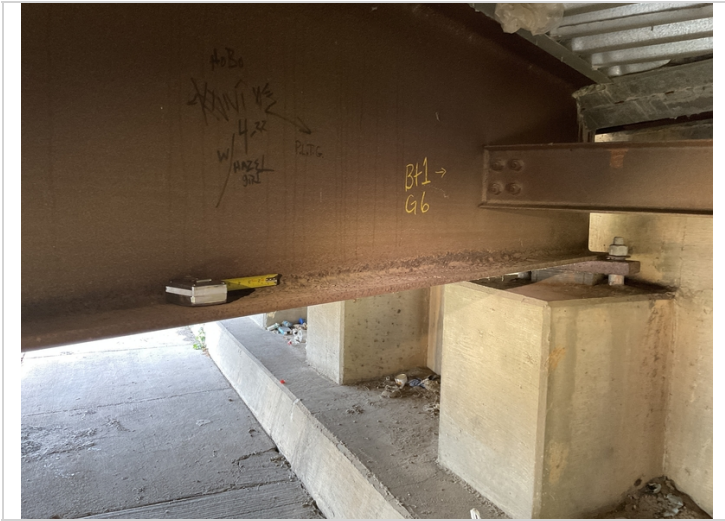
Bent 1, girder 6: laminating rust and active corrosion to the bottom flange and lower web.
