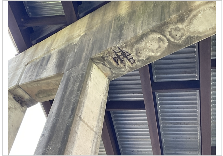
Bent 10 exposed rebar on bottom of cap next to column 2.
