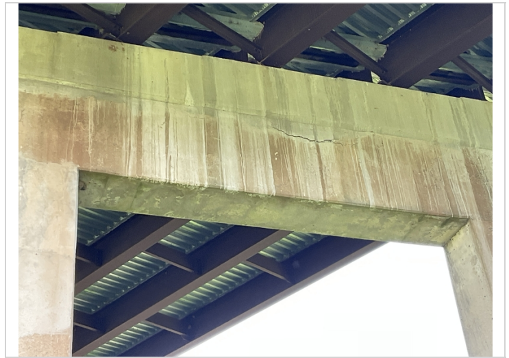
Bent 6 delams on ahead face
