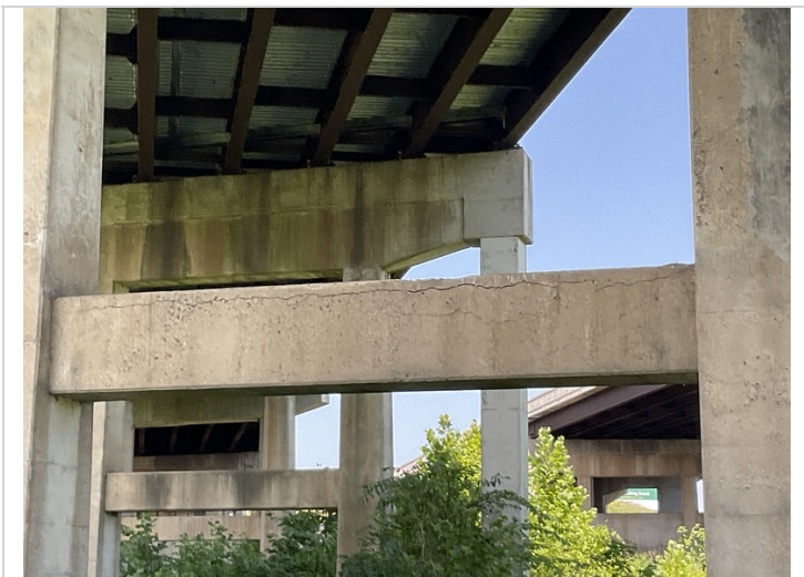
Bent 8 cracks in cross brace
