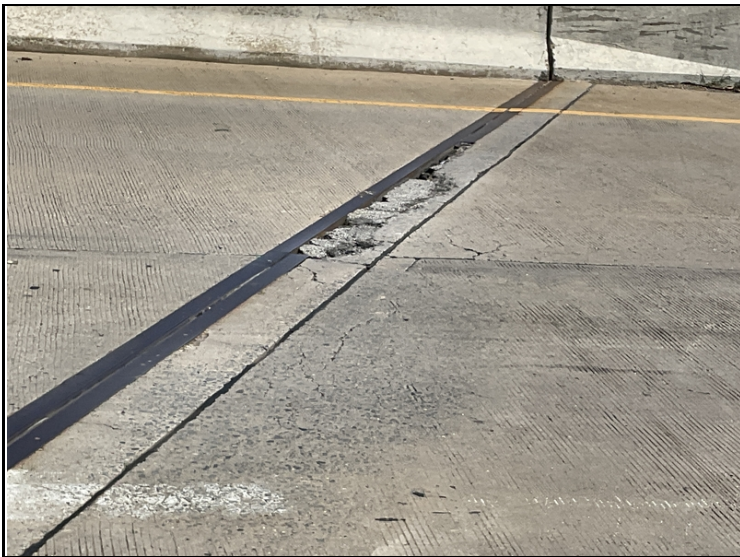
12' of spalls in top of back wall at bent 13
