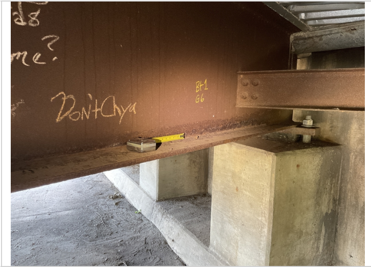
Bent 1, girder 6: laminating rust and active corrosion to the bottom flange and lower web. Common girder 5
