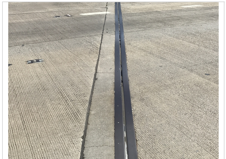
Bent 1: multiple areas of joint seal missing allowing water to flow through to the steel girders.
