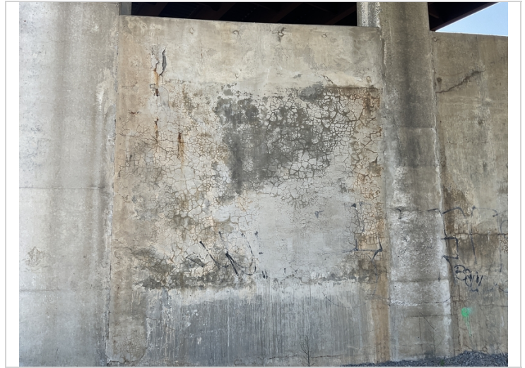
Bent 3 map cracking and exposed rebar in pier wall
