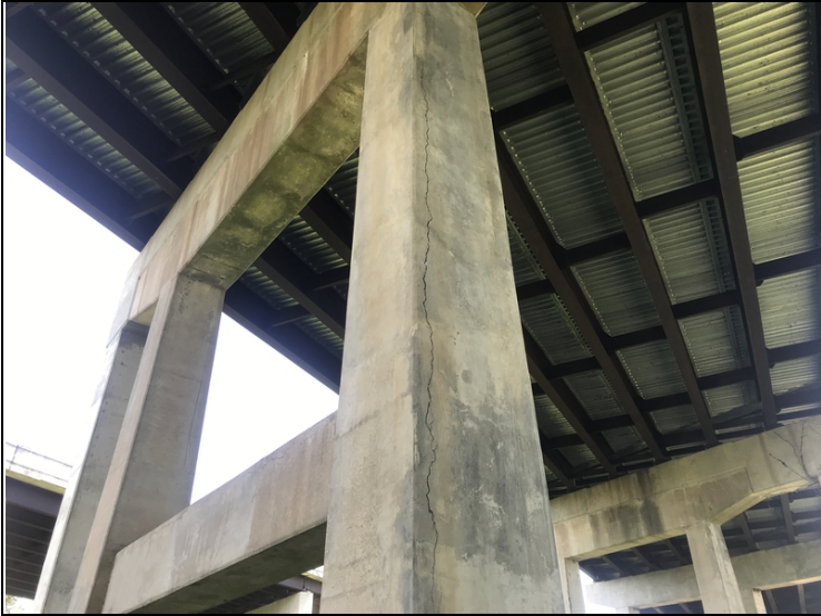
Bent 7, column 2: large vertical crack running the entire length of the column.
