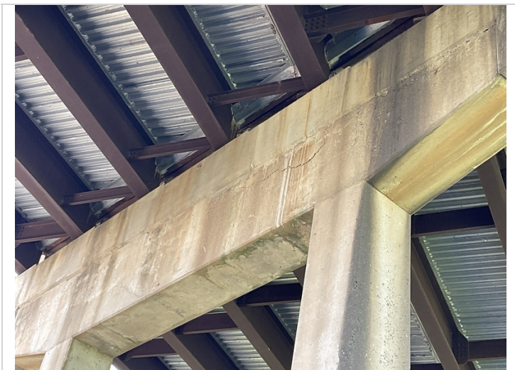
Bent 10 delam on ahead face
