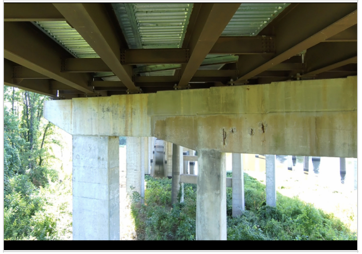
Bent 7 spalls with exposed rebar
