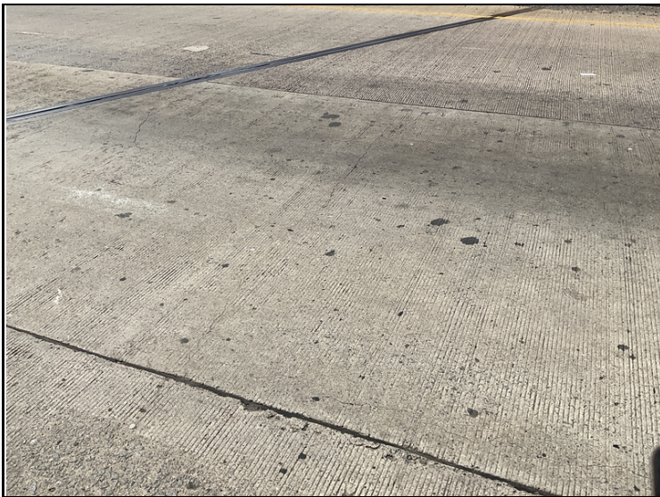
Span 10 typical deck cracking
