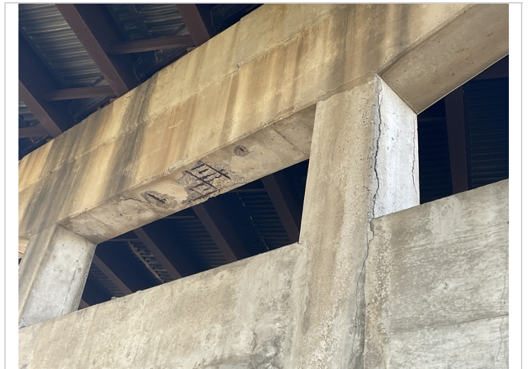
Spalls with exposed rebar on bottom of bent 3. Large cracks in columns 2&3
