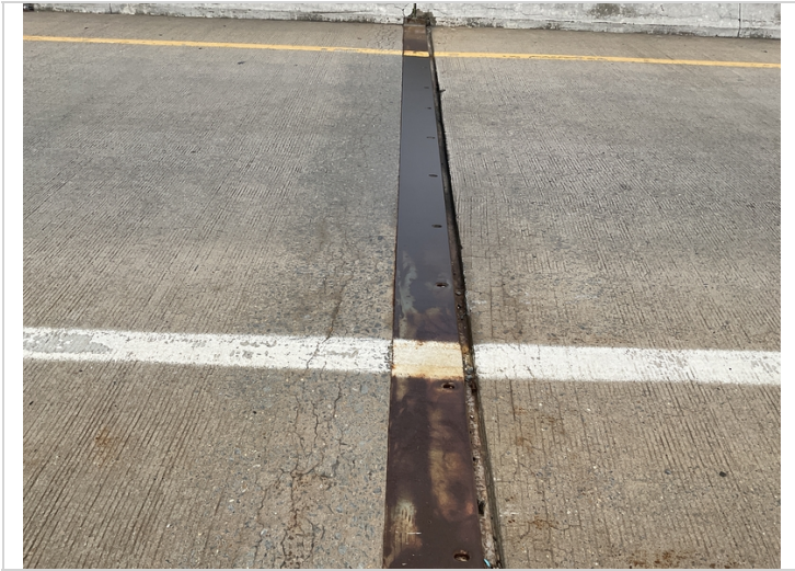
Map cracking around joint at bent 10
