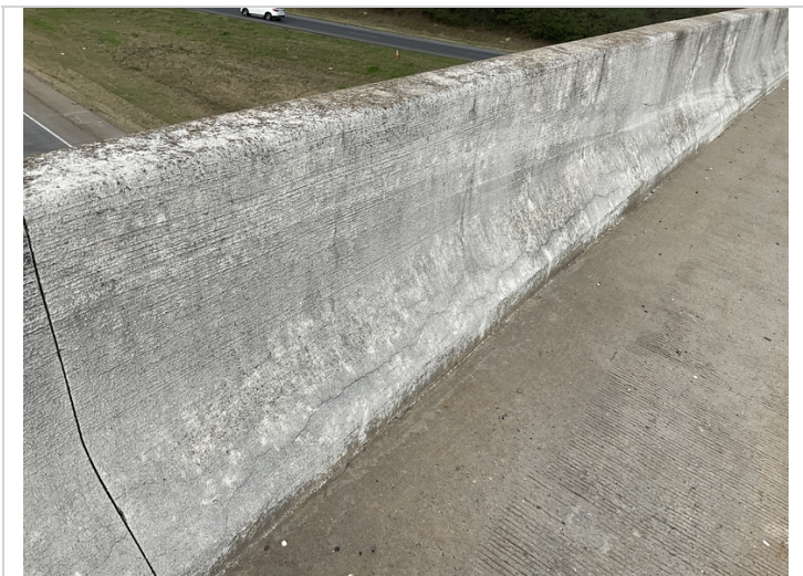
Typical cracks in bridge rail
