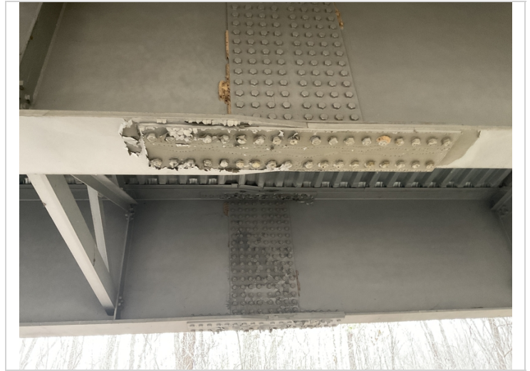
Span 13 peeling paint
