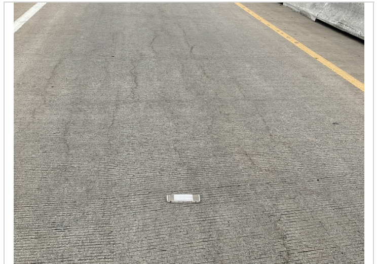
Span 10 deck cracking up to 0.025"
