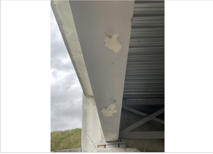
Span 1 girder 4 peeling paint
