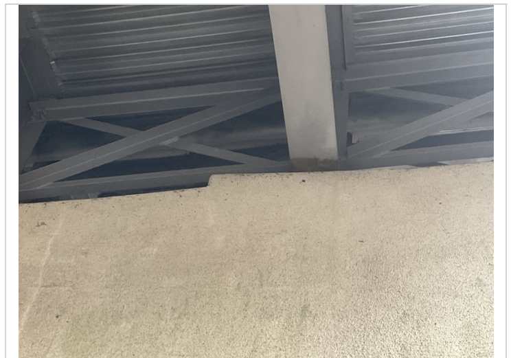
Span 12 at bent 13 girder 3 small area of active corrosion
