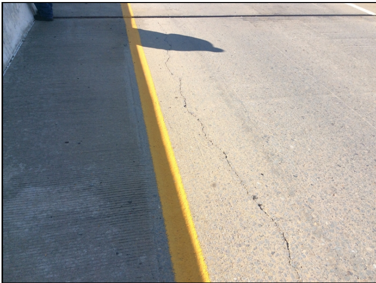
Northeast approach, large unsealed cracks.
