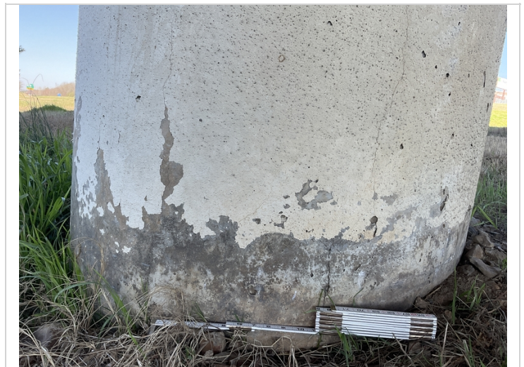
Bent 2, Column 1: has vertical cracks near bottom of column. Similar condition at column 3.
