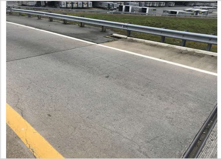
Approach slab at North end of bridge has unsealed longitudinal and transverse cracking.
