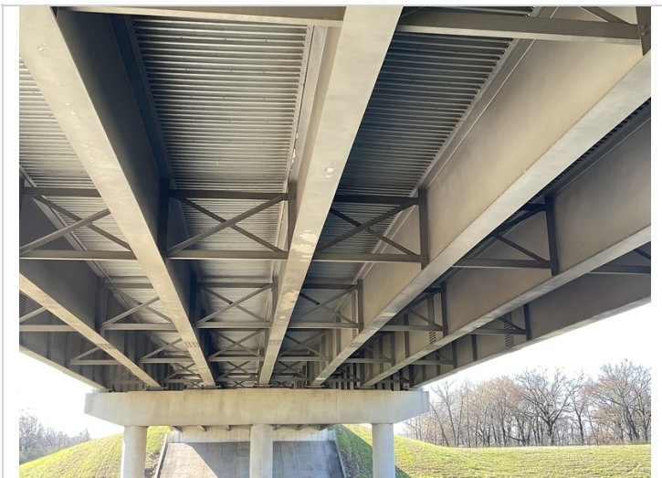
Span 2: girders 3&4 have areas on the bottom flange with peeling paint
