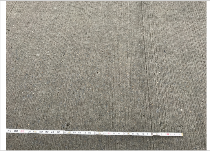
Span 2 deck cracking longitudinal and transverse cracks, common span 1.
