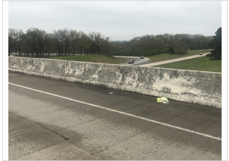
Concrete bridge railing has cracking, both left and right sides.
