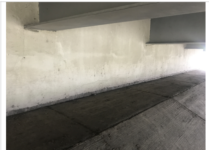
Bent 3 abutment has horizontal cracks under beams 4-6.
