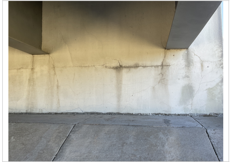
Bent 1: numerous horizontal and diagonal cracking throughout the entire abutment. Bent 3 is in similar condition
