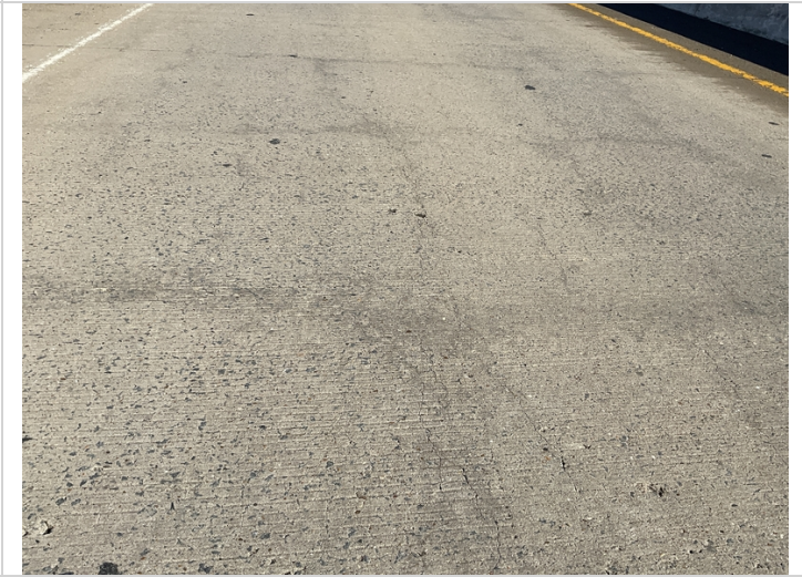
Span 2: multiple longitudinal cracks
