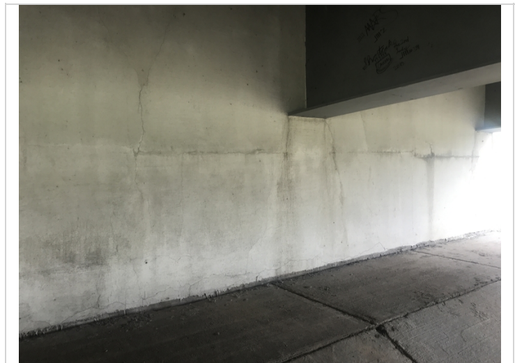
Abutment 1 has horizontal cracking and vertical cracking at beam 2.
