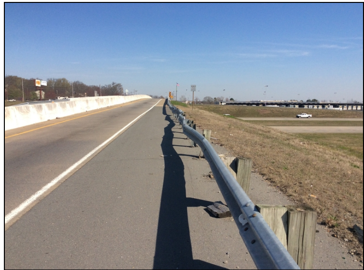
Northbound approach guardrail damaged due to traffic impact.
