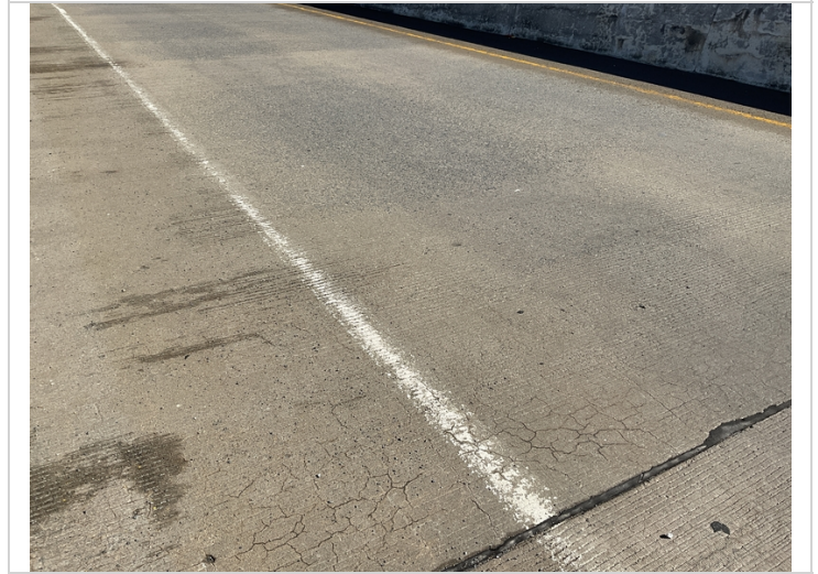
Span 1: map cracking
