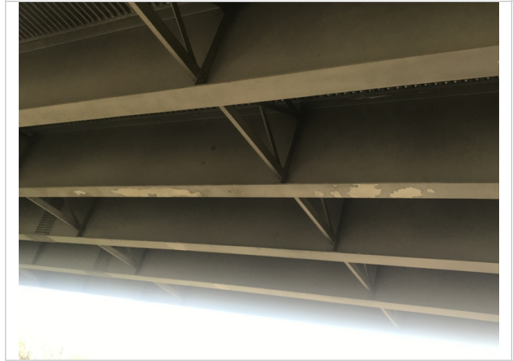
Span 2 beams have peeling paint on bottom flanges.
