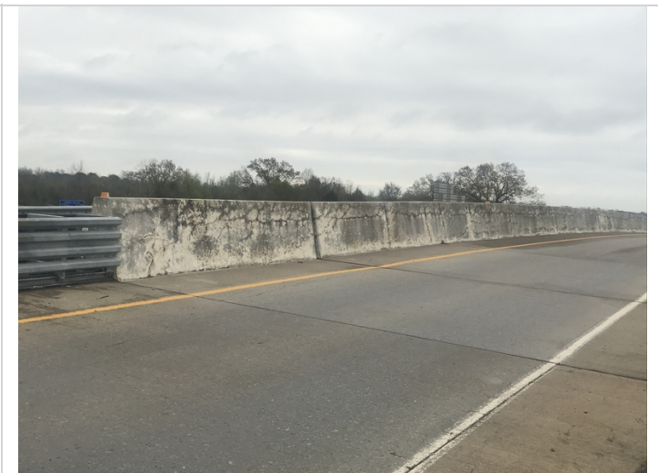
Median concrete barrier wall has cracking.
