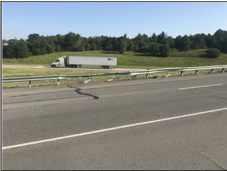
Left approach guard rail damaged due to traffic impact.
