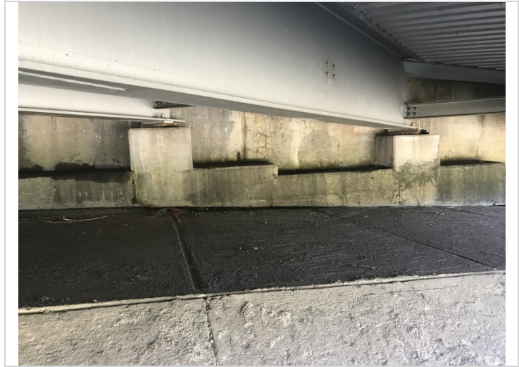
Bent 1: backwall with map cracking between girders 3&4.
