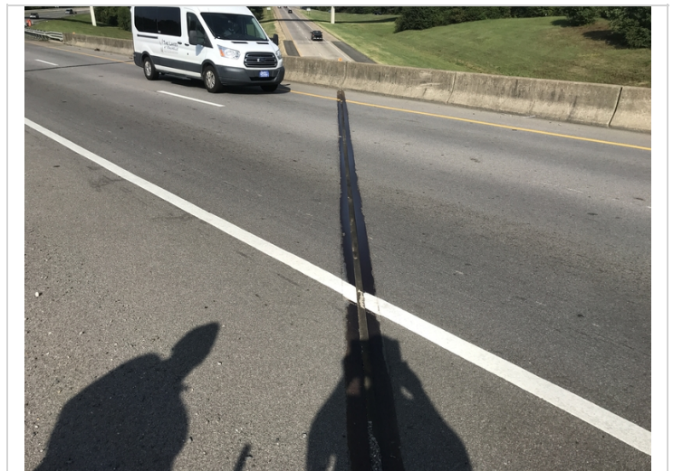
Joint seals have been replaced. 2021
