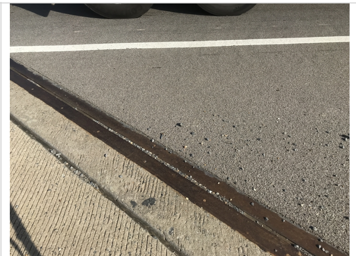
Entire deck surface has had a wearing surface added to it since last inspection
