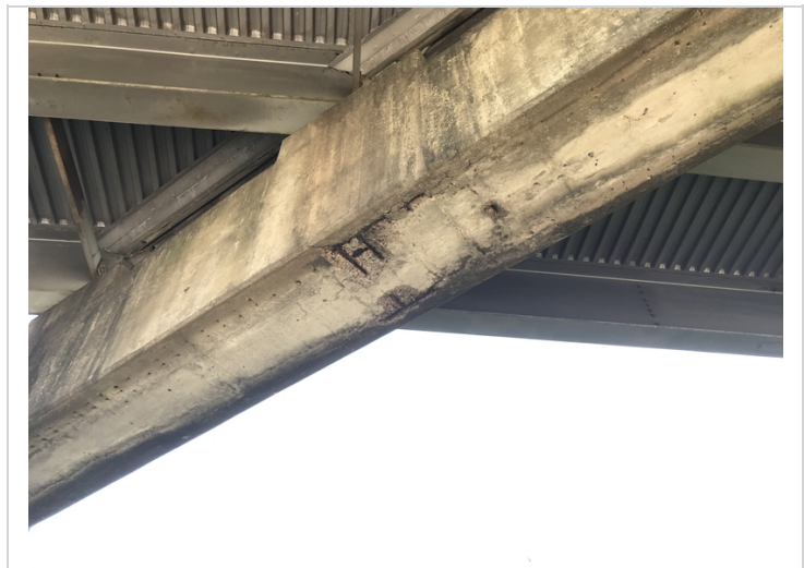
Bent 4 cap: bottom of cap between columns 1&2 has spall with exposed rebar
