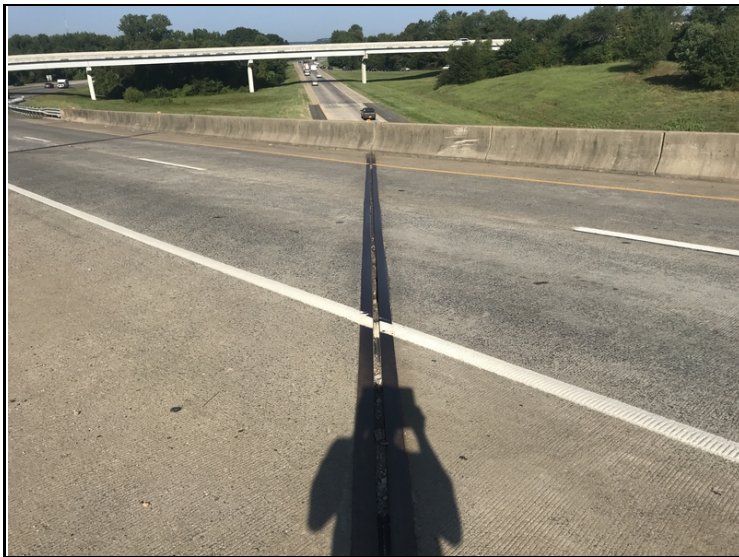
Bent 3 joint seal has lost bond allowing dirt and debris to accumulate. Common bent 6.
