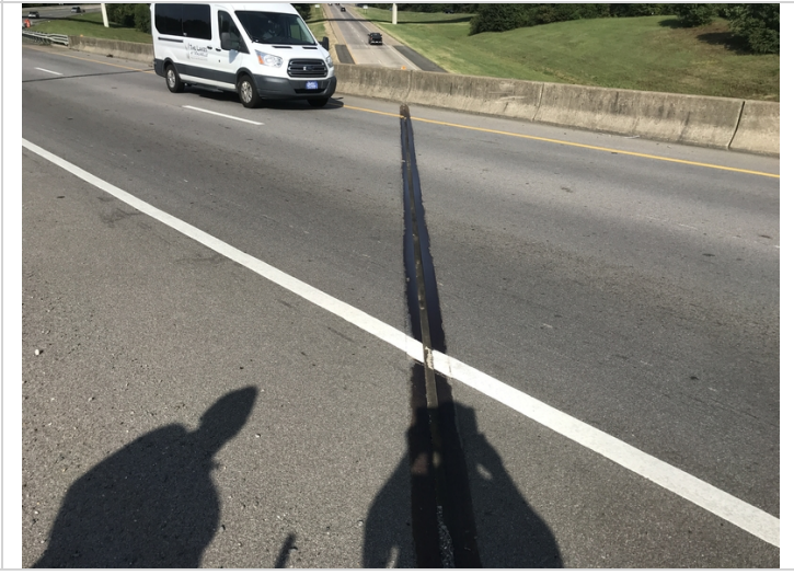
Joint seals have been replaced. 2021
