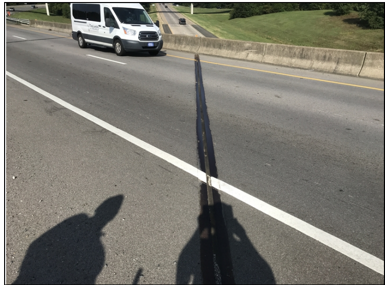
Joint seals have been replaced. 2021
