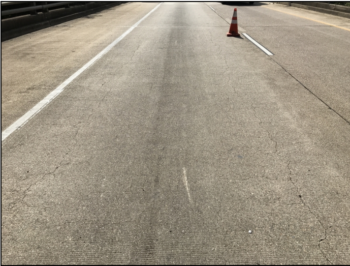
Span 2 large longitudinal cracks.
