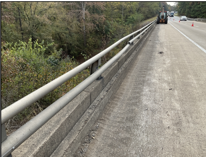
Span 5, right rail damaged due to traffic impact
