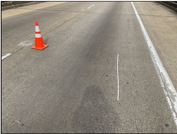
Span 1: multiple unsealed longitudinal cracks
