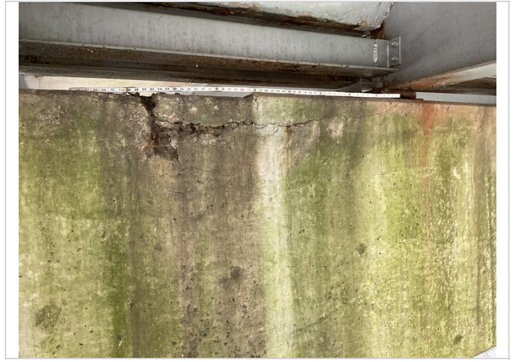
Ahead side of bent 3 between beams 5 and 6: spall and delam approximately 6 feet in length
