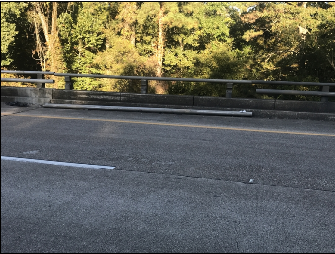
Left bridge rail at span 4 is damaged due to traffic impact.
