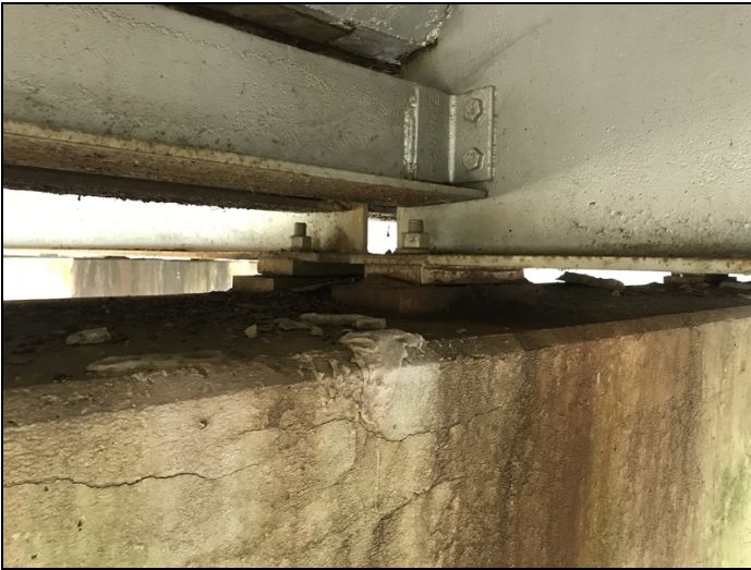
Bent 3 bearings 3 ahead and back have movement.
