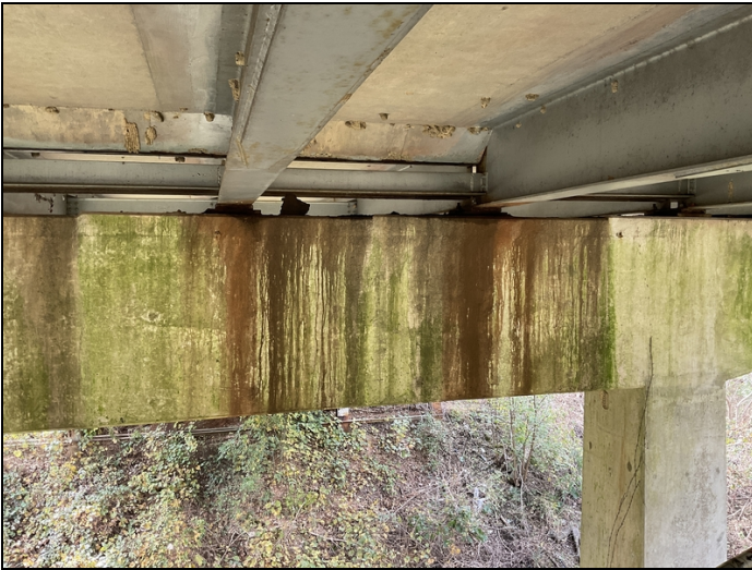
Looking back at bent 3: beams 3&4 the beams are floating causing the bearings to have getting rust
