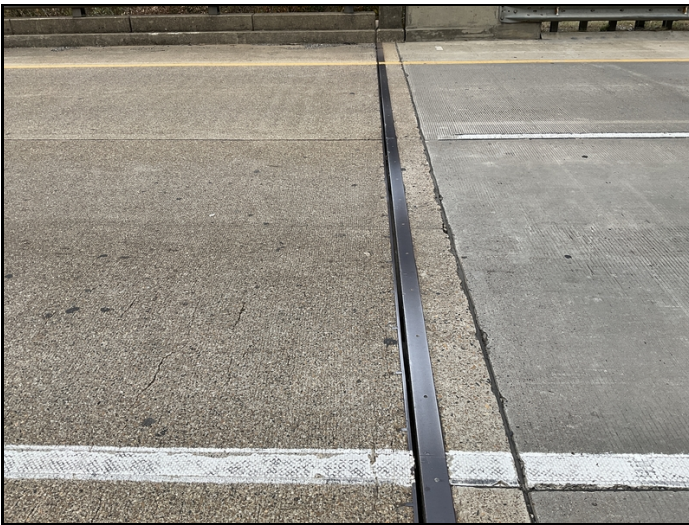
Bent 6: majority of joint seal missing. 2022
