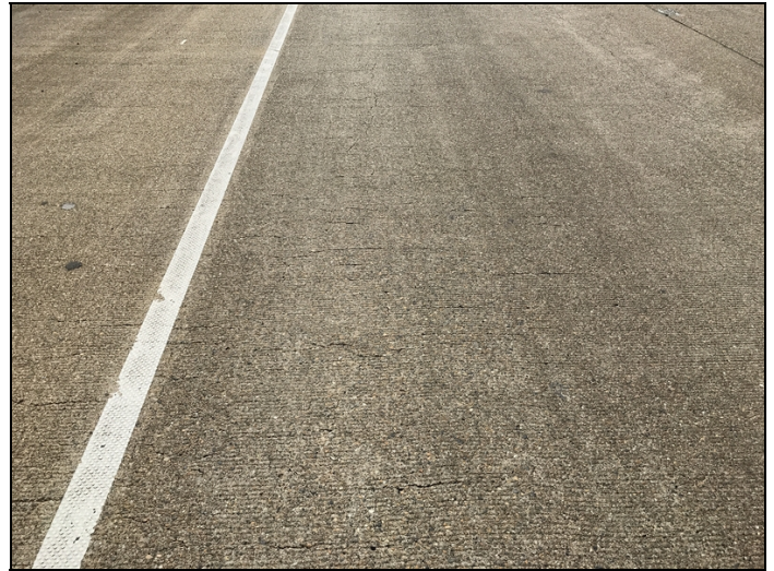
Span 5 longitudinal and transverse cracks.
