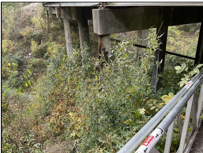
Both sides of bridge has trees and heavy vegetation making it difficult to use the Aspen inspection vehicle.
