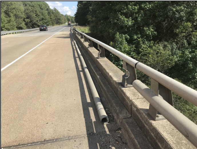
Span 4 collision damage to bridge rail, bottom rail section is missing. Right side
