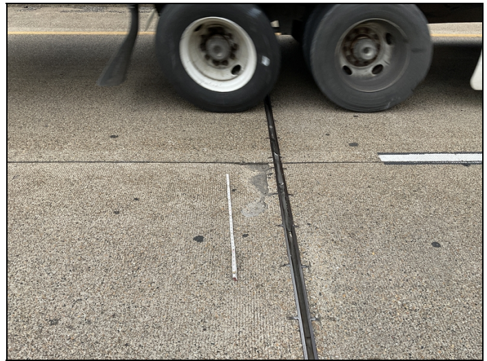
Bent 5: joint seal has lost bond allowing water to leak through. 2022
