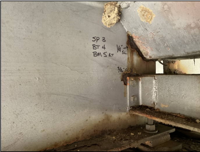
Section loss at the haunch and above diaphragm 2022
