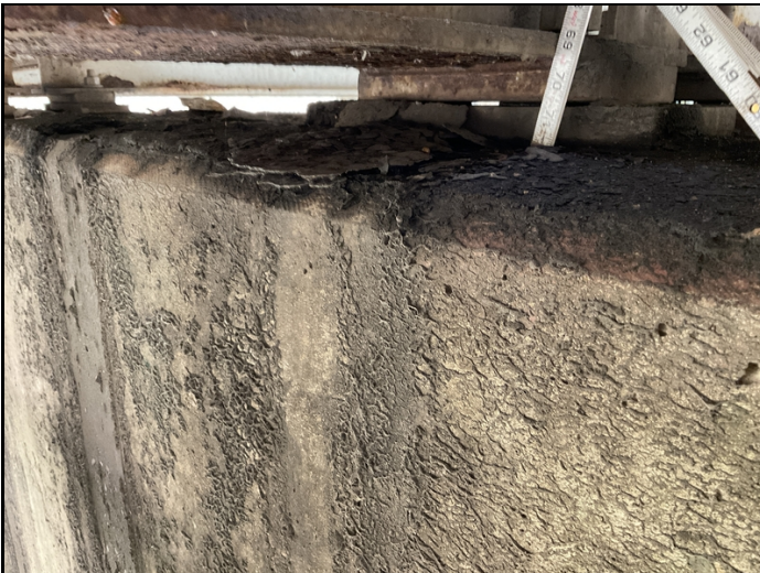
Bent 4, beam 5, span 4: beam floating
