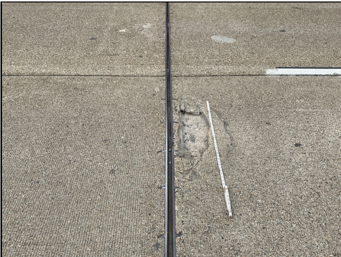
Bent 4: small spall in the lane just right of centerline.
