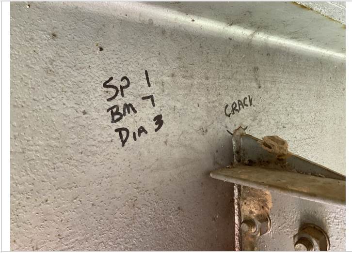
Span 1, beam 7, 3rd dia.: Crack to the weld 2022
