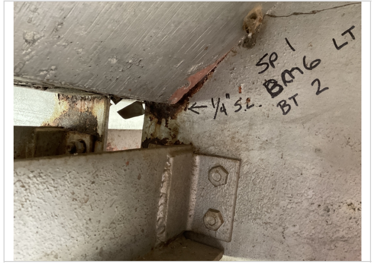
1/4" section loss at the haunch 2022
