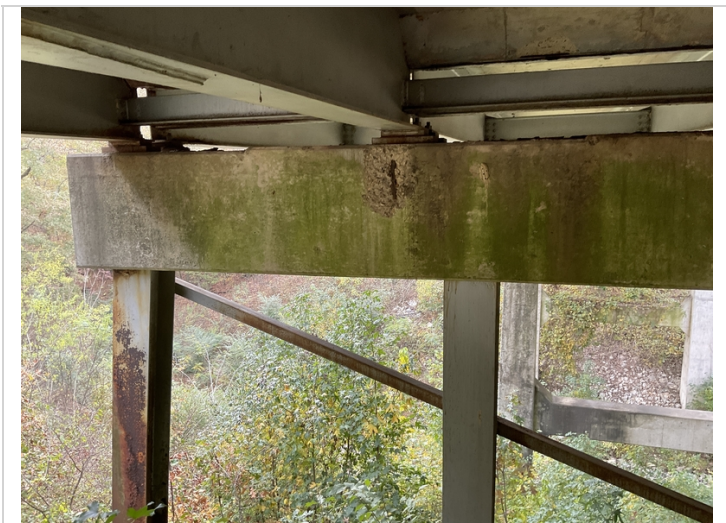
Bent 5 ahead side: spall with exposed rebar under beam 5
