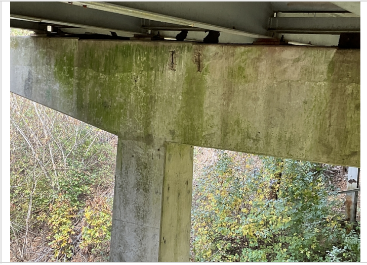
Backside of bent 4 cap has couple spalls with exposed rebar
