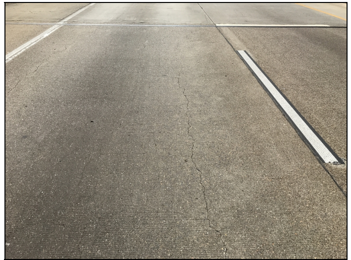
Span 1 longitudinal cracks.
