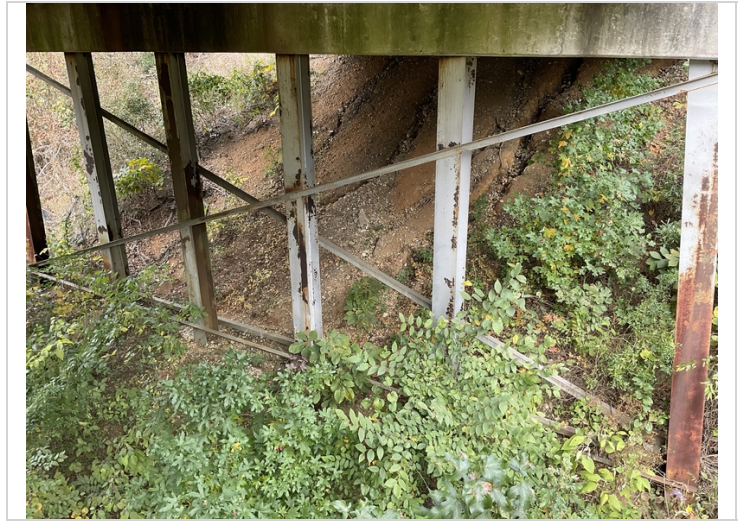
Bent 5: all pile with surface rust
