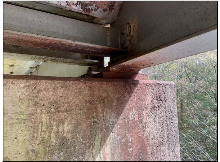
Span 1, bent 2, beam 7: beam is floating.
