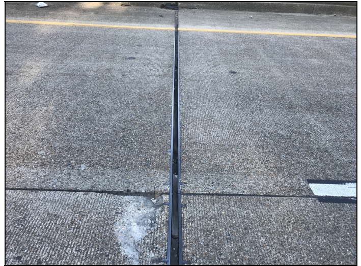
Bent 5 joint seal is damaged and leaking. Common all joints.
