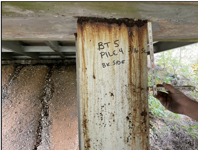
Bent 5, pile 4: top of the pile has up to 3/16" section loss adjacent to the cap. Similar condition at piles 2,3&4.
