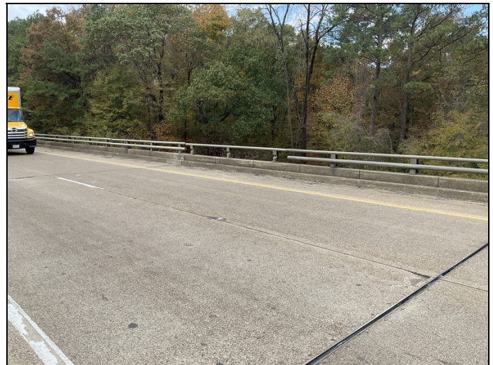
Span 4: left rail is damaged due to traffic impact. 2022
