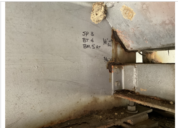
Section loss at the haunch and above diaphragm 2022
