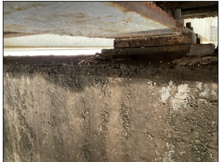
Span 3, bent 4, beam 5: beam is floating and causing a rattling sound
