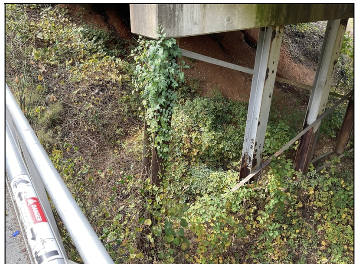
Bent 2: vines climbing onto pile 6
