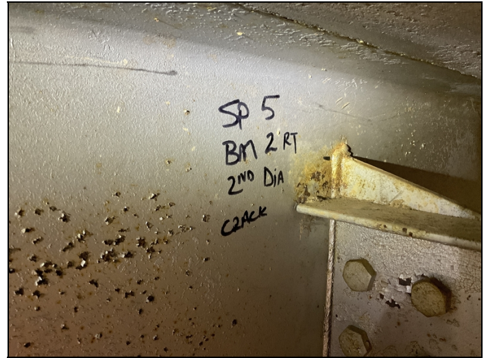
Crack in the weld. 2022
