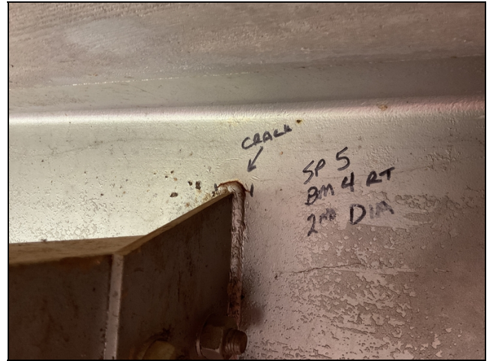
Crack propagates into the web. 2022
