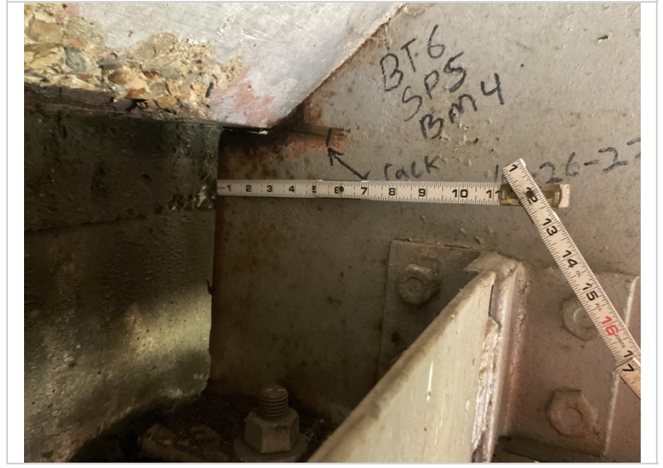
Large crack from the end of the beam into the web.
