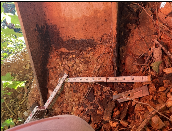
Bent 2, pile 4: at ground line all surfaces with measurable section loss up to 1/8". The right flange in the picture has 1/8" steel remaining.
