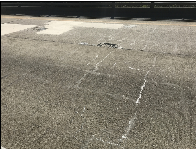
Span 1 spalls and delam in the rigid overlay.
