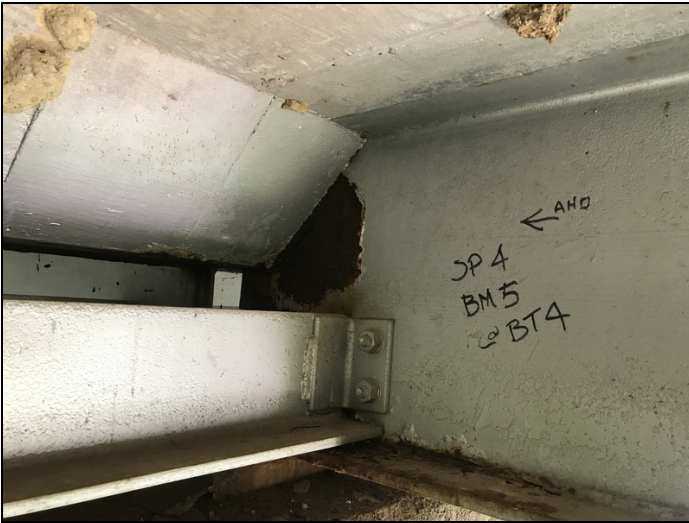
Bent 4 girder 5 back side section loss in web at the haunch area.
