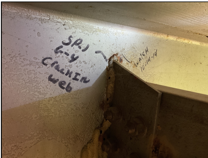
Crack propagates into the web 2022
