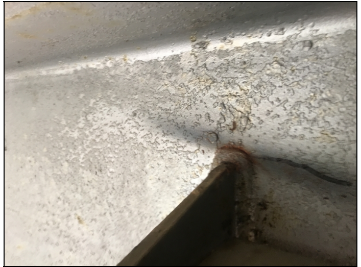
Span 4 beam 4 first diaphragm ahead of bent 2. Crack in the toe of weld at top diaphragm bracket.
