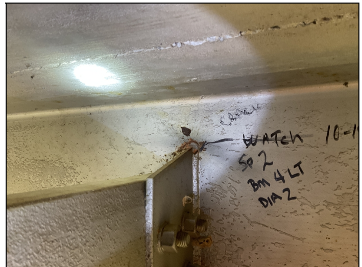
This crack propagates into the web 2022
