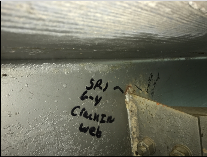
Span 1 girder 4 crack in web at top of diaphragm connection.
