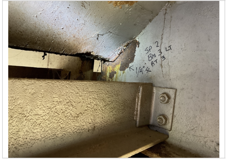
Up to 1/4" section loss at the haunch
