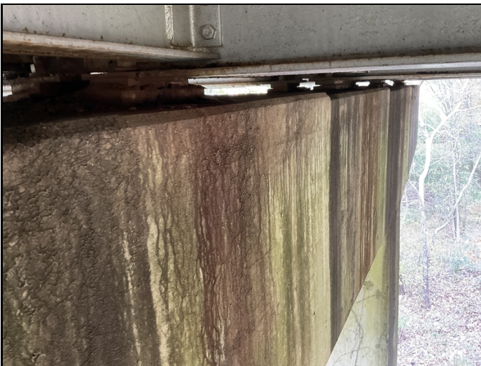
Bent 4: all bearings have large amounts of fretting rust coming from them due to them impacting when loads
