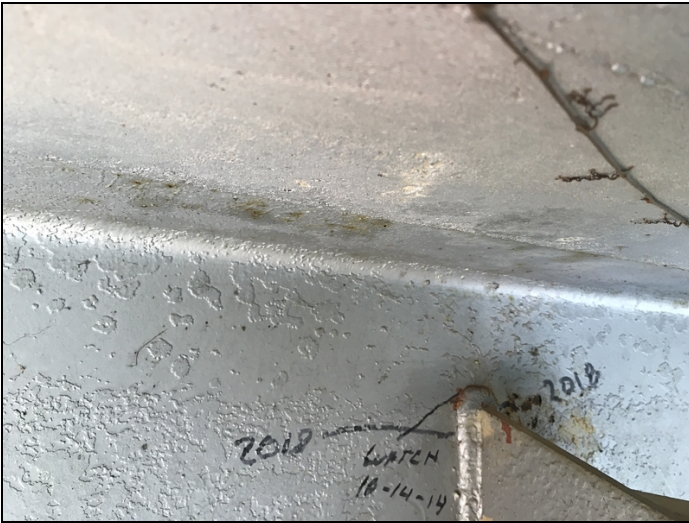
Span 2 girder 4 crack in top of weld in diaphragm connection.
