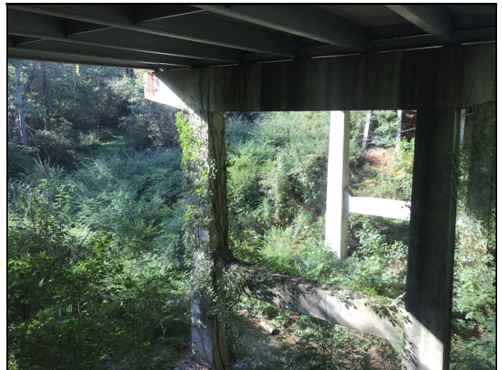
Vines growing on columns at bents 3 and 4.
