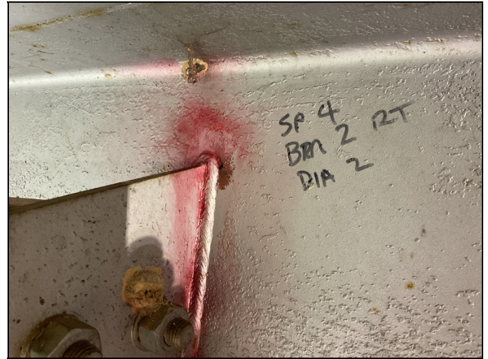
Crack in the toe of the weld. 2022
