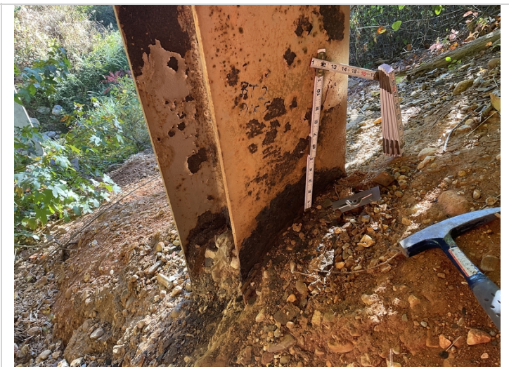
Bent 2, pile 5: up to 1/16" section loss from the ground up 4".
