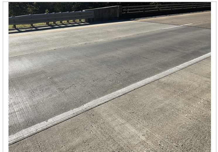
Approach slab with multiple large transverse cracks
