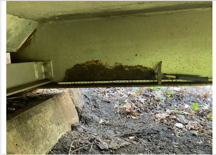
Span 1, girder 1: large area of section loss to the lower web and bottom flange.
