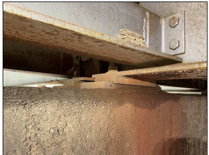
Beam 3, bent 5, span 5: bearing is floating
