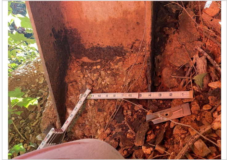
Bent 2, pile 4: at ground line all surfaces with measurable section loss up to 1/8". The right flange in the picture has 1/8" steel remaining.
