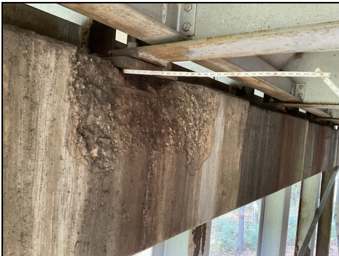
2 3/4" of bearing loss. Bent 5, beam 5, span 5
