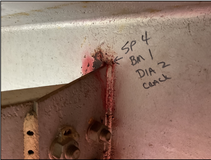
Crack in the toe of the weld. 2022
