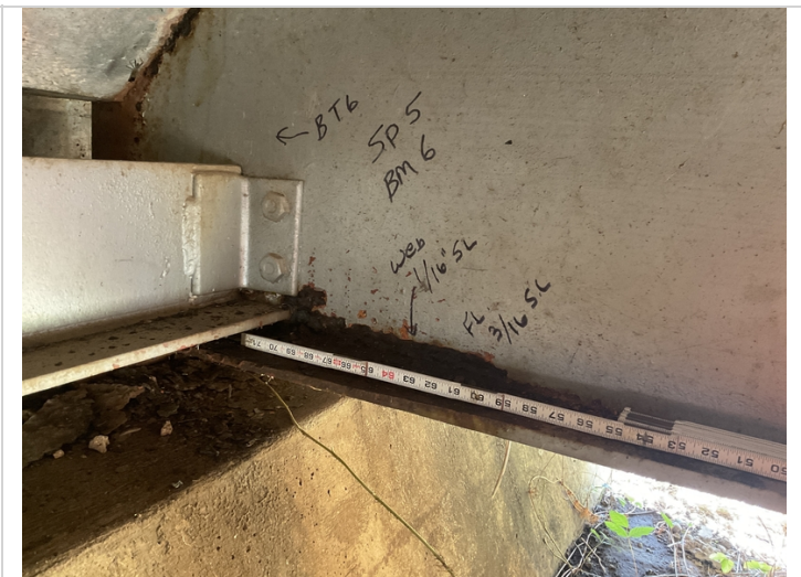
Beam 6, span 5, bent 6: up to 3/16" section loss to the bottom flange and 1/16" section loss to the lower web.
