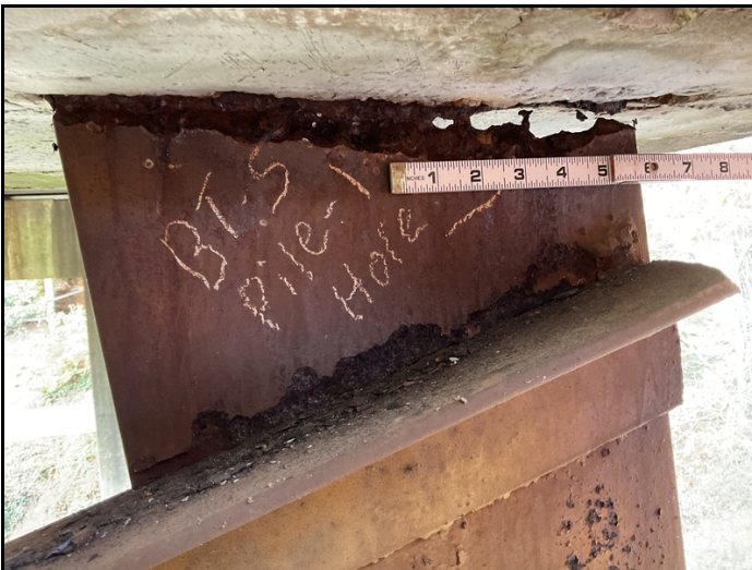
Bent 5 steel pile 1; 5" hole in the pile adjacent to the cap at the ahead side. 2022
