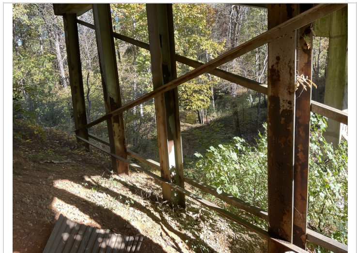
Bent 2: the paint has failed in numerous areas and surface rust and section loss to all piles.
