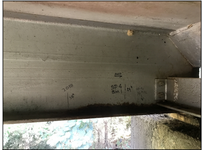
Bent 5 back side girder 1 section loss up to 1/8" on bottom flange.
