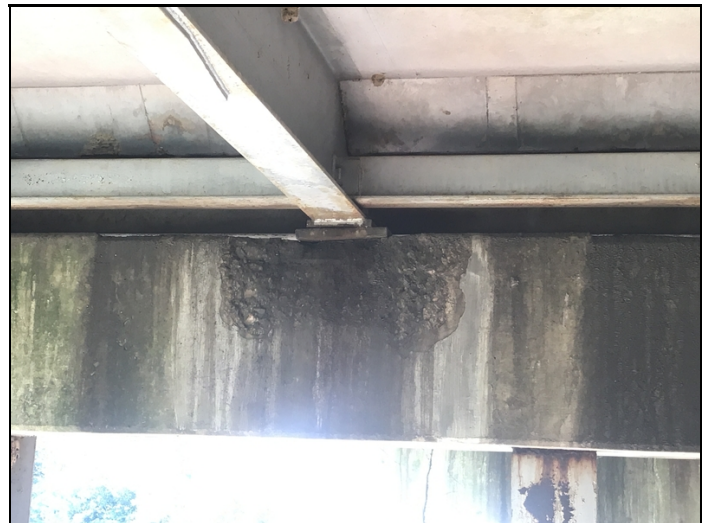
Span 5 bent 5, ahead side, spall on cap below bearing, reducing the bearing surface area. Photo attached.
