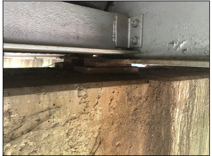
Bent 3 bearing 3 floating under load.
