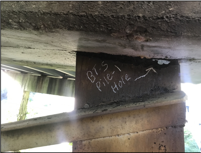
Bent 5 steel pile 1 hole in top of pile and section loss up to 3/16" .
