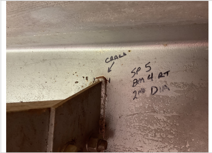
Crack propagates into the web. 2022
