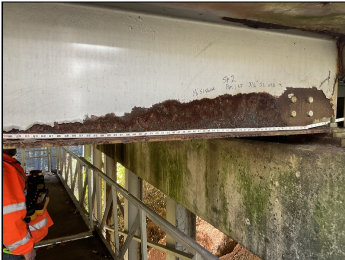
More than 6 feet of the bottom flange and lower web with measurable section loss
