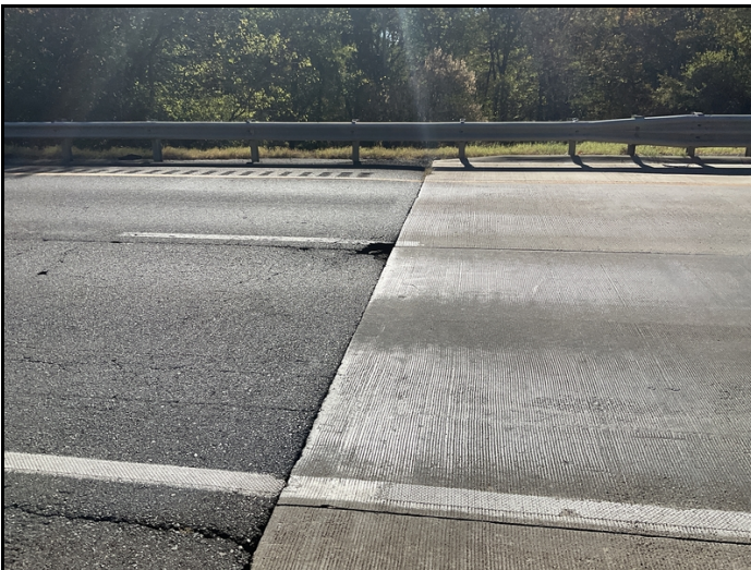
West bound approach roadway with a pothole in the asphalt surface adjacent to the approach slab.
