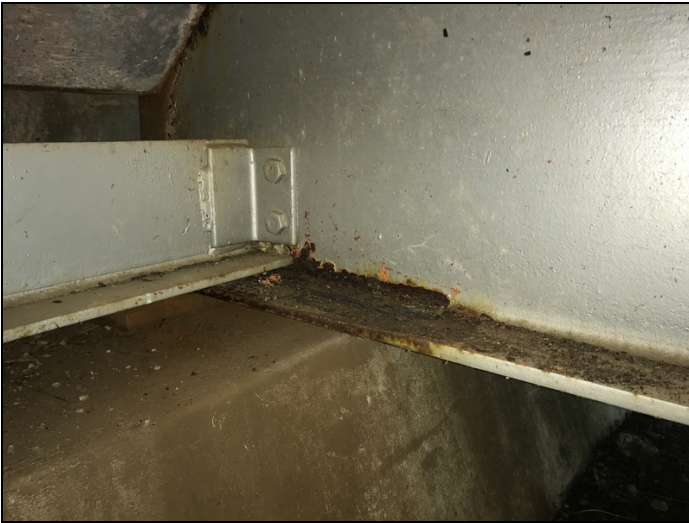
Bent 6 girder 6 section loss to bottom flange.
