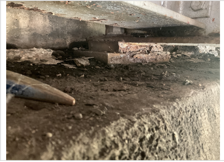
By 6, girder 4: bearing with typical corrosion at this bent.
