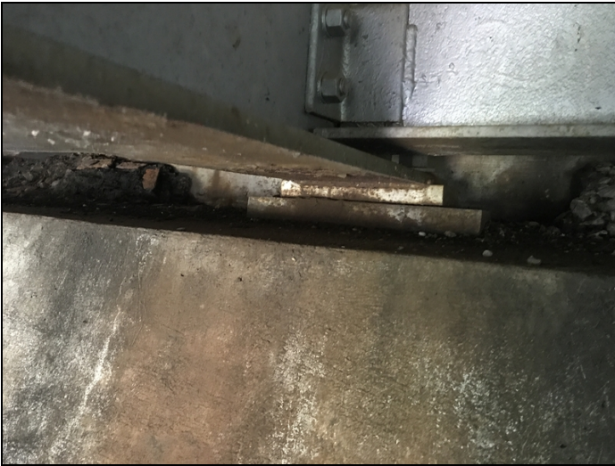
Bent 6 bearings 2, 3, 5 and 6 are floating.
