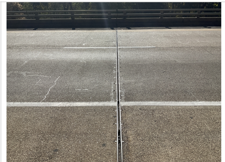
Bent 5: joint seal leaking
