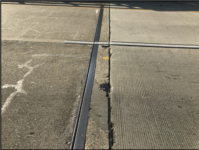
2 spalls in top of back wall at bent 1.
