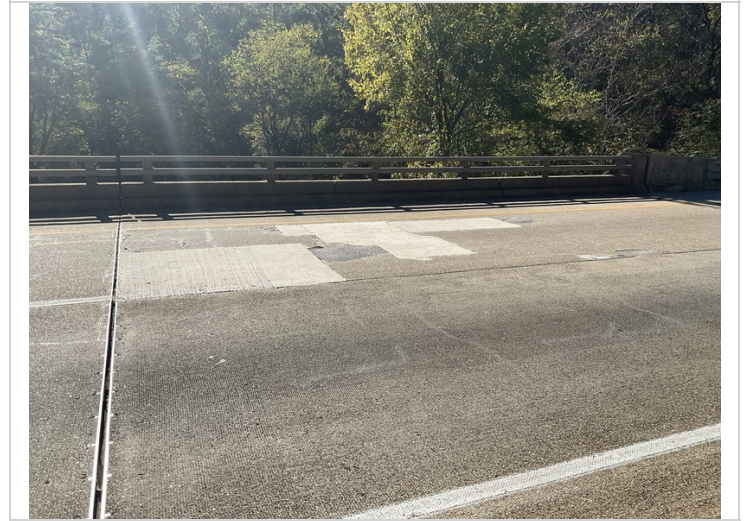
Span 1: multiple concrete patches and asphalt patches in this span.
