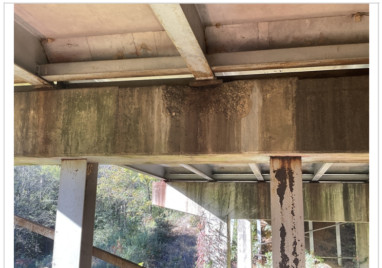
Ahead side of bent 4, girder 5: large spall under girder 5 with some loss to the bearing area
