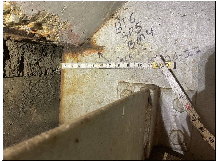
Large crack from the end of the beam into the web.
