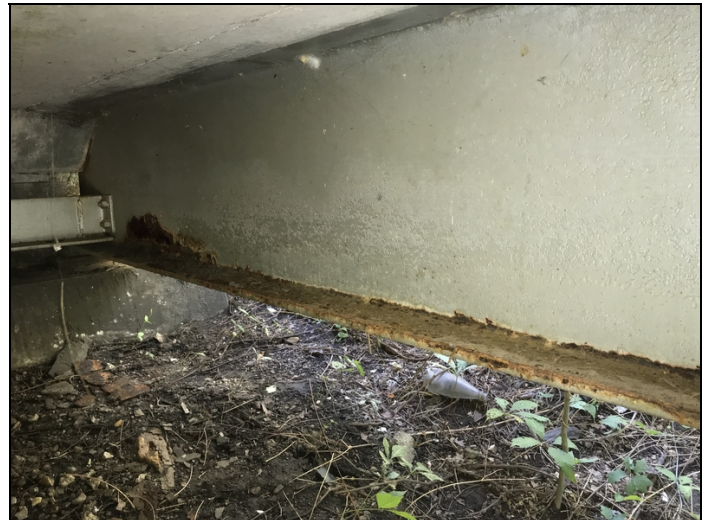
Span 1 girder 1 section loss in web and flange 20' in length.
