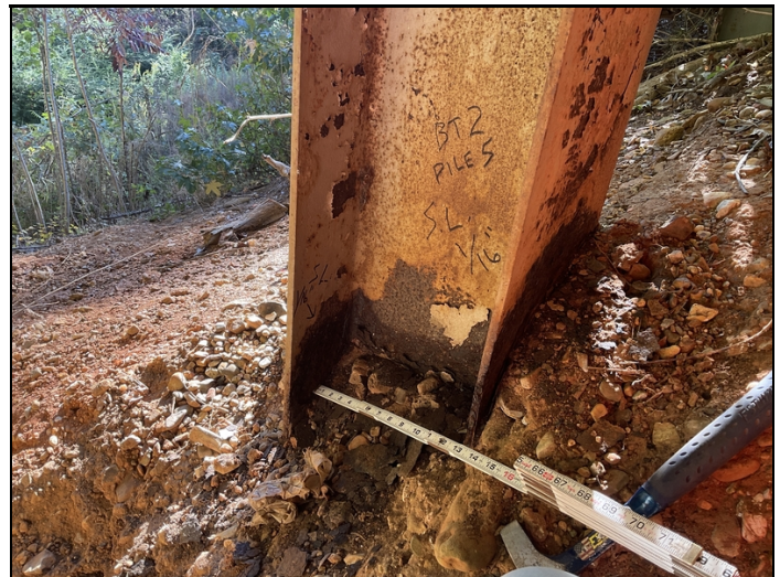
Bent 2, pile 5: at ground line all surfaces with measurable section loss up to 1/16".
