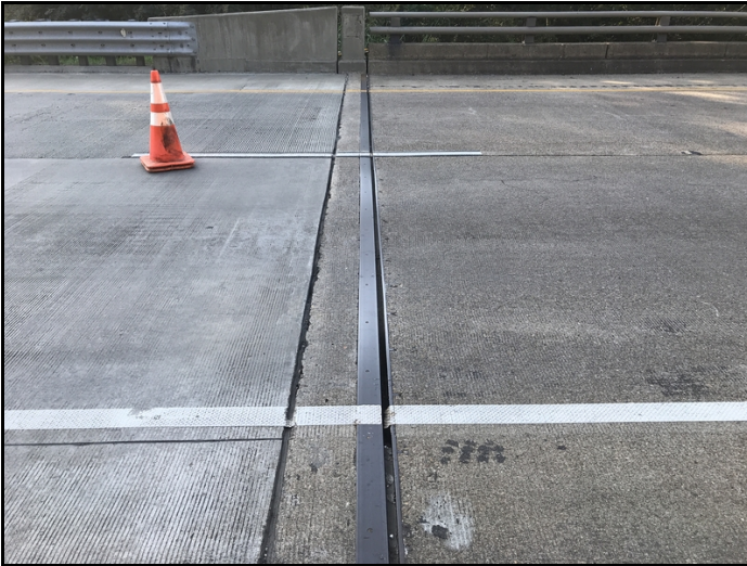
Bent 6 joint is leaking.
