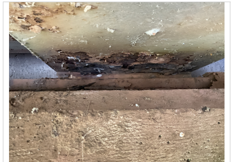
Span 3 girder 4 at pier 1 active corrosion with deep pitting to bottom flange.
