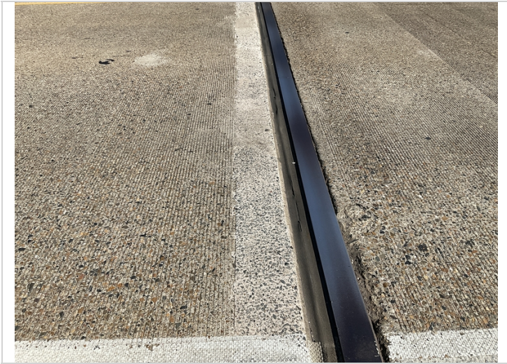
Deck at joint of pier 3 patched area.
