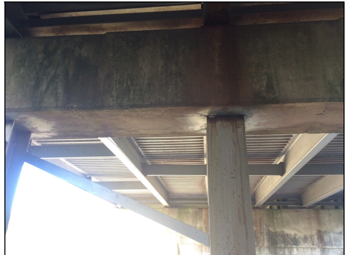
Bent 3 pile 5, hole in flange below cap.
