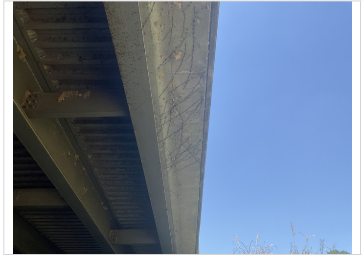
Cracks with efflorescence in the left soffit overhang common right side.
