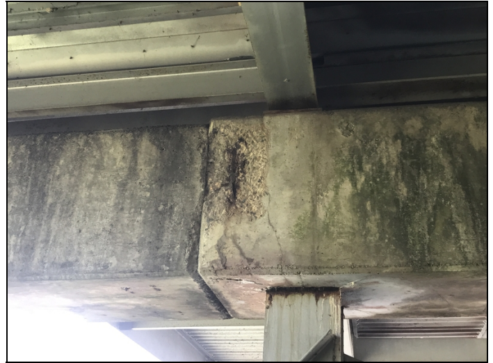
Bent 3, large spall with exposed rebar in the cap.
