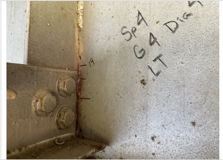
Span 4 girder 4 diaphragm 4 left side back broke welds. Common on right side.
