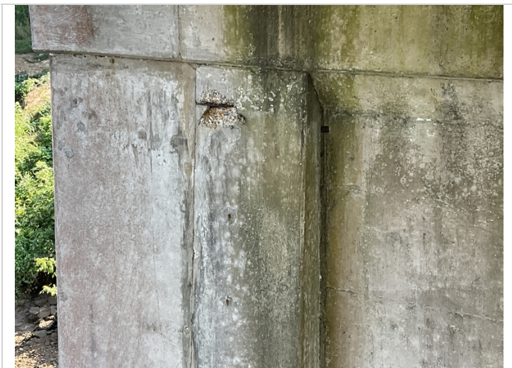
Pier 5 column 1 back spall with exposed rebar.
