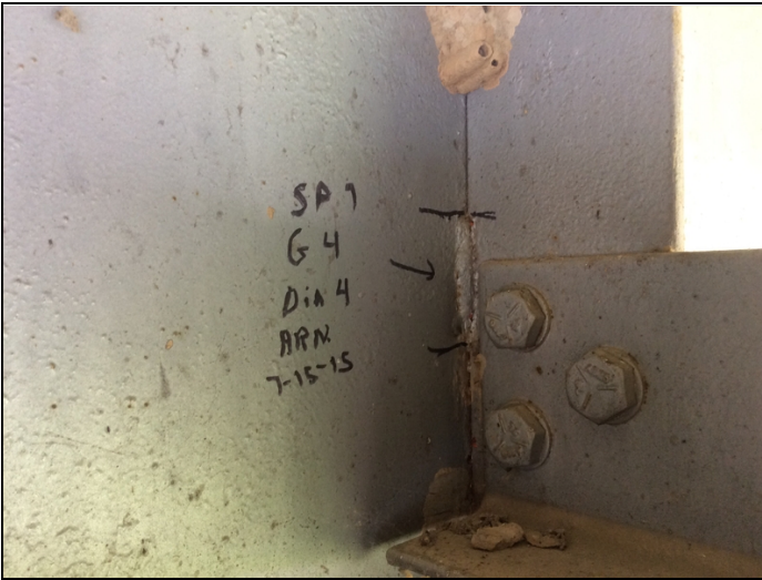
Span 7 girder 4 4th diaphragm has cracked welds.
