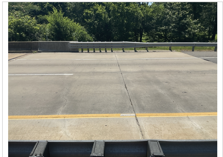
Transverse cracks in west approach slab.
