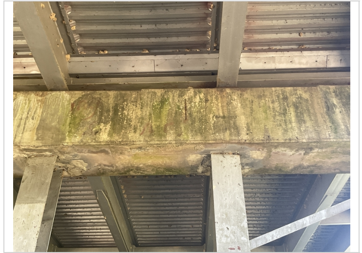
Bent 2 cap ahead spall with exposed rebar above pile 3.
