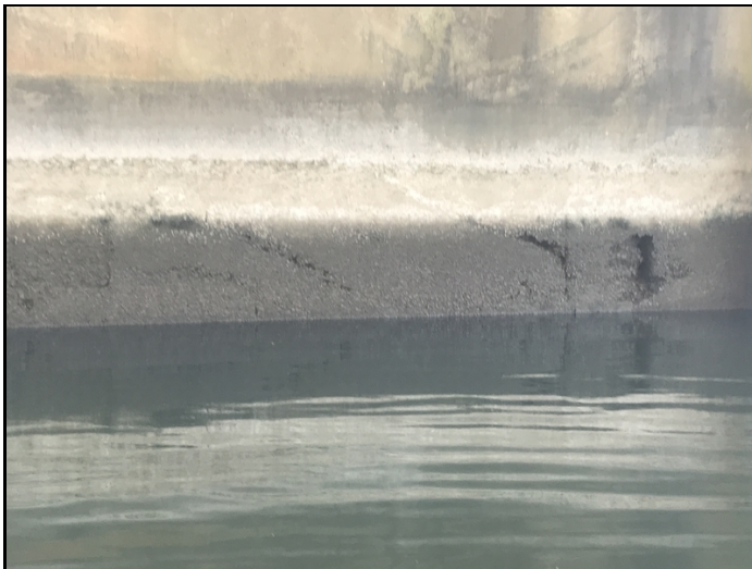
Bent 5 pier wall has areas of severe abrasion at water line.
