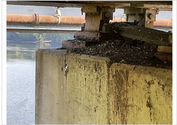
Pier 2 span 3 bearing 1 corrosion.
