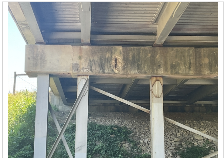
Bent 3 spall with exposed rebar on pier cap back between columns 2 and 3.
