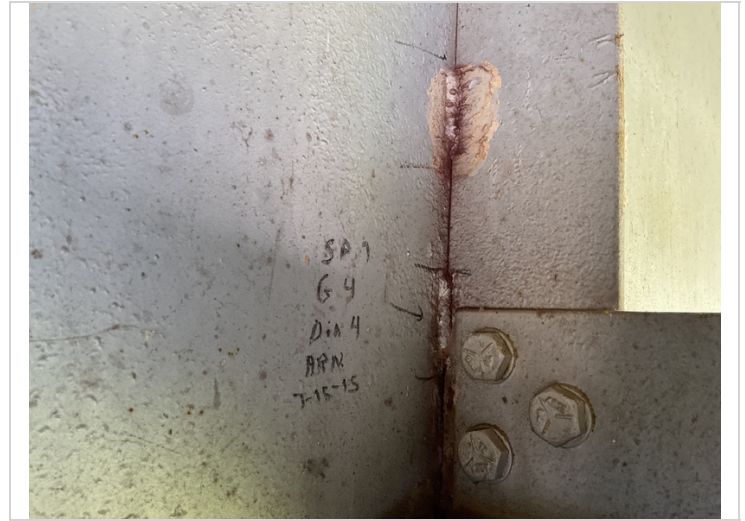
Span 7 girder 4 diaphragm 4 right side back broke welds. Common ahead this location.
