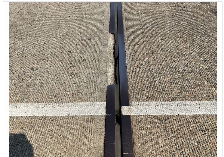
Pier 4 joint armor missing.
