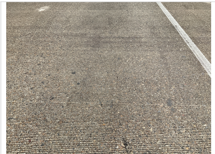
Deck span 2 transverse and longitudinal cracks.
