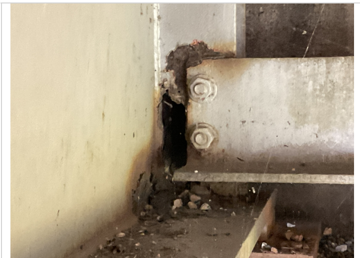
Span 3 girder 4 left side pier 1 girder left side hole in the vertical diaphragm brace and pitting in the lower web.
