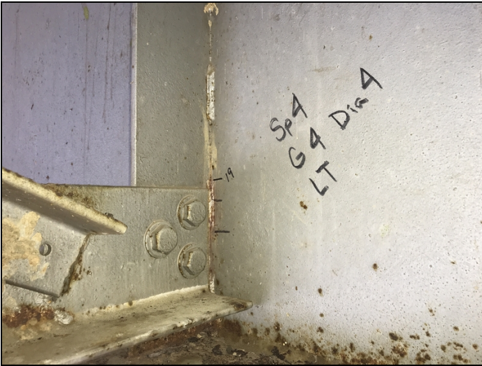
Span 4 g4 d4 left side stiffener has broken welds
