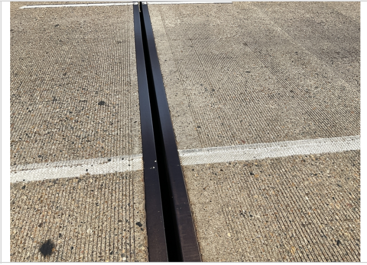
Pier 2 joint seal missing.
