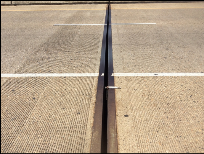
Pier 2, joint seal has fallen through.
