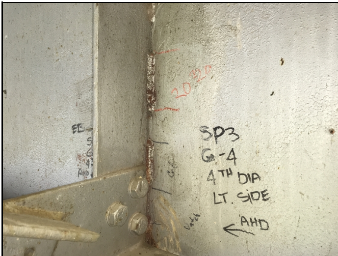
Span 3, girder 4, diaphragm 4, new crack in weld.
