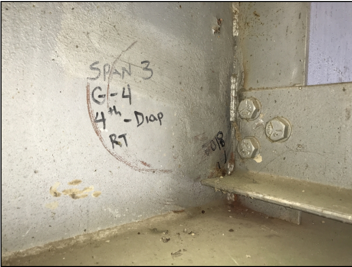
Span 4 g4 d4 rt side has a crack in the web that has grown 3/4" since 2018 inspection
