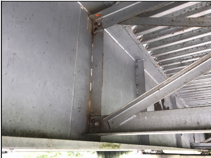
Span 6 g3 d5 diaphragm bolt holes have become misaligned and diaphragm has been welded in place
