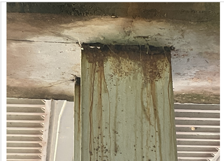
Bent 3 steel pile 5 has deep pitting and small holes in the flange at cap.
