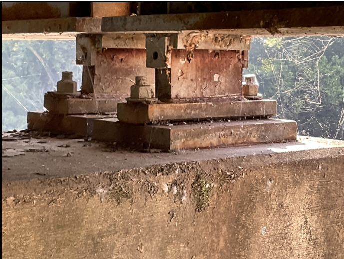
Pier 3 span 4 bearing 6 missing top bolt.
