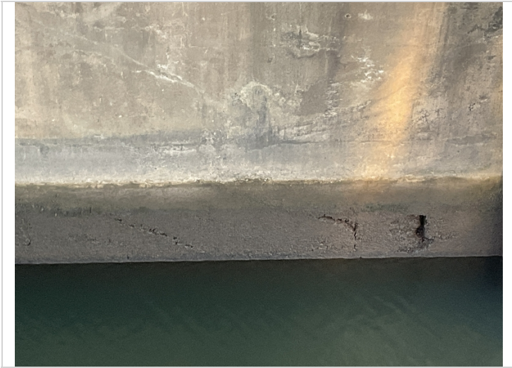
Pier wall 3 back severe abrasion.
