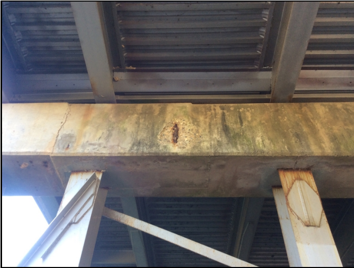
Bent 3 backside, spall with exposed rebar.
