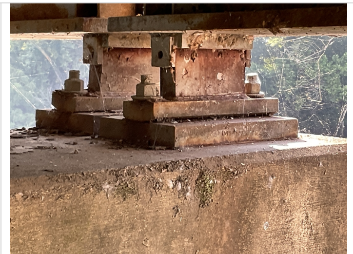
Pier 3 span 4 bearing 6 missing top bolt.
