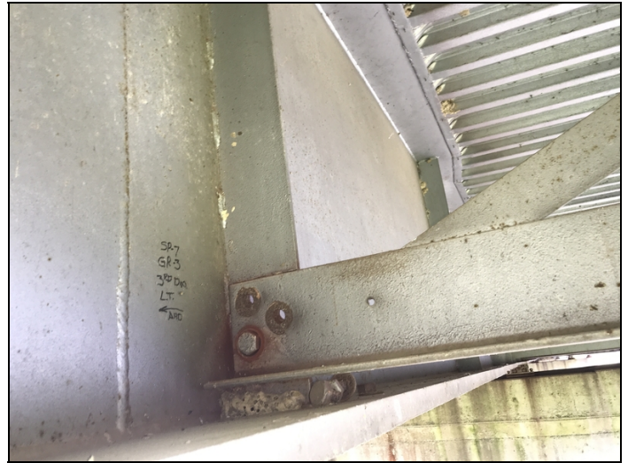
Span 7 g4 d3 have Loose and missing bolts
