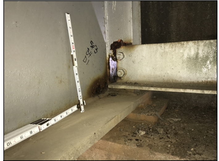
span 3 g4 dia1 diaphragm clip/stiffener has a 2"x4" hole at bottom connection and the web at girder 4 has up to 1/4" deep section loss
