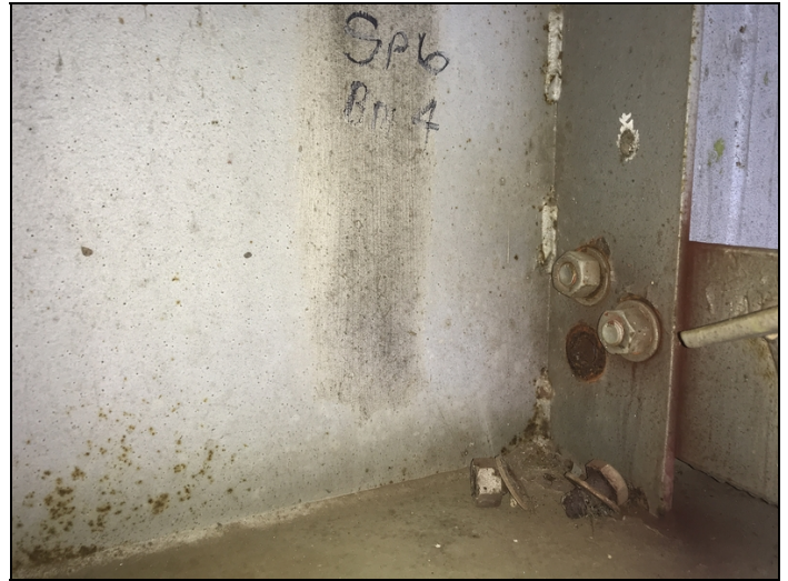
Span 6 girder 4, sheered bolt at diaphragm 4
