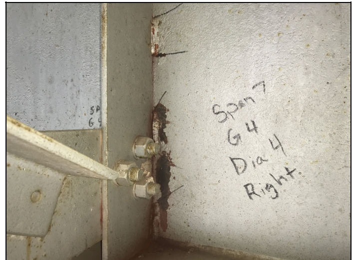
Span 7, girder 4, diaphragm 4, cracks in welds.
