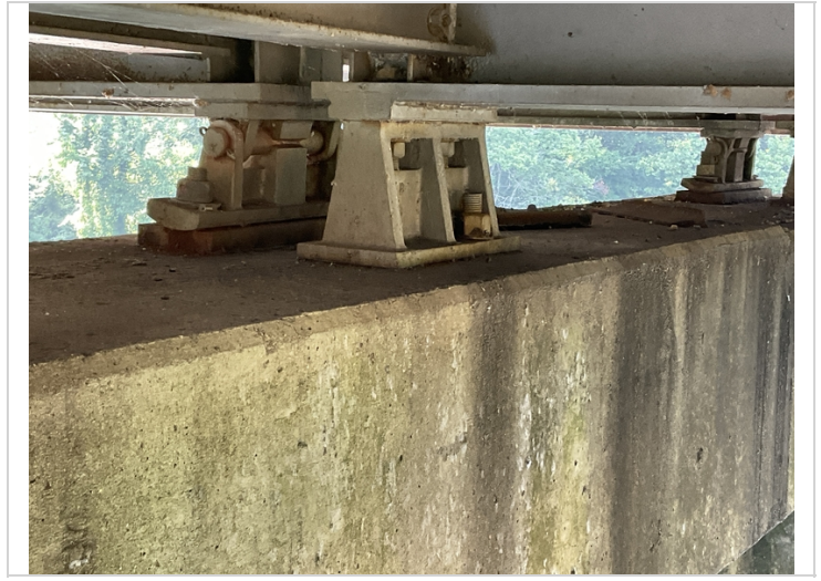
Pier 4 movable bearing are rotated back.
