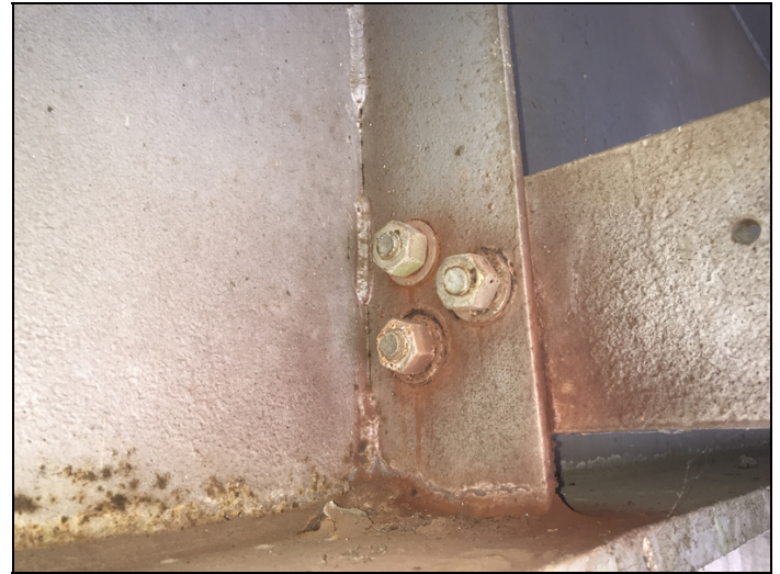
Span 4 girder 5, diaphragm 2, loose bolts.
