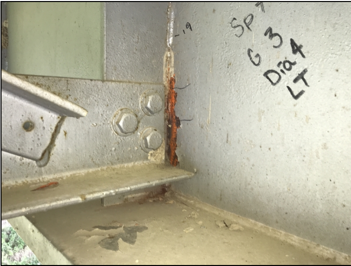
Span 7 g3 d4 cracks in welds have grown into next stitch weld
