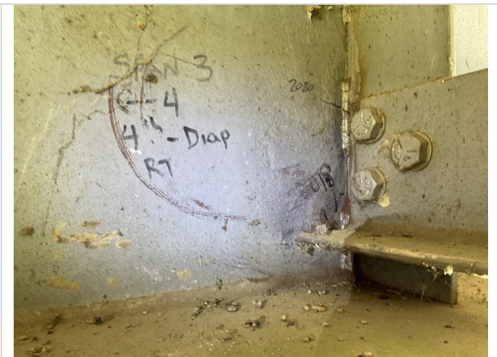
Span 3 girder 4 diaphragm 4 right side back has broke welds crack has propagated into the web.
