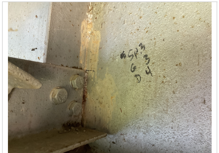
Span 3 girder 3 diaphragm 4 left side back has broke weld.
