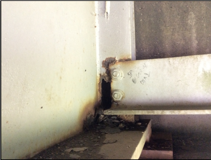
Hole in the diaphragm bracket at span 3 girder 4 diaphragm 1 at pier 1.
