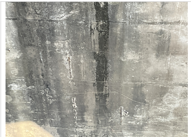
Pier wall 2 ahead spall with exposed rebar.
