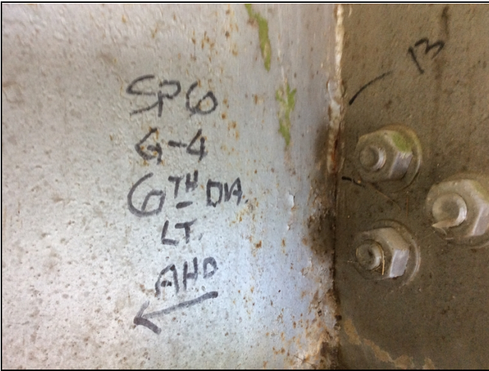
Span 6 girder 4 6th diaphragm has cracked welds.
