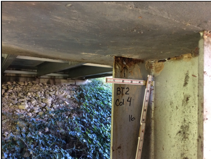
Measurable section loss to the flanges below the cap. Also small hole in the flange at this location. Worst case at this bent.
