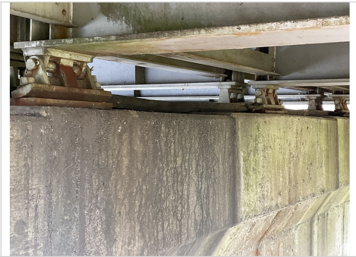
Pier 5 span 7 movable bearing are rotated back.
