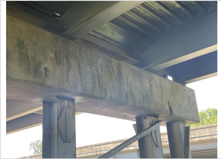
Bent 3 cap ahead spalls with exposed rebar.
