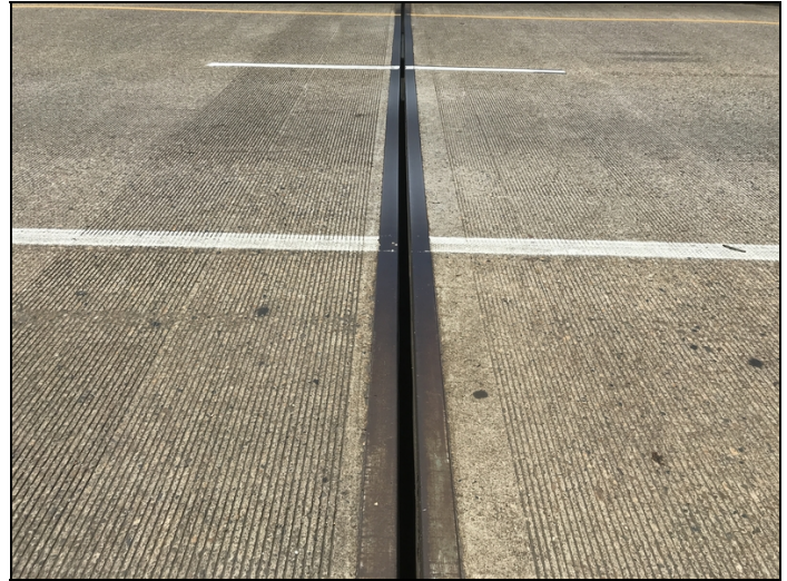
Pier 2, joint missing.
