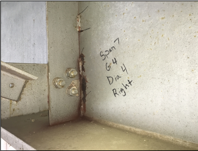
Span 7 g4 d4 the broken welds in stiffener have No change
