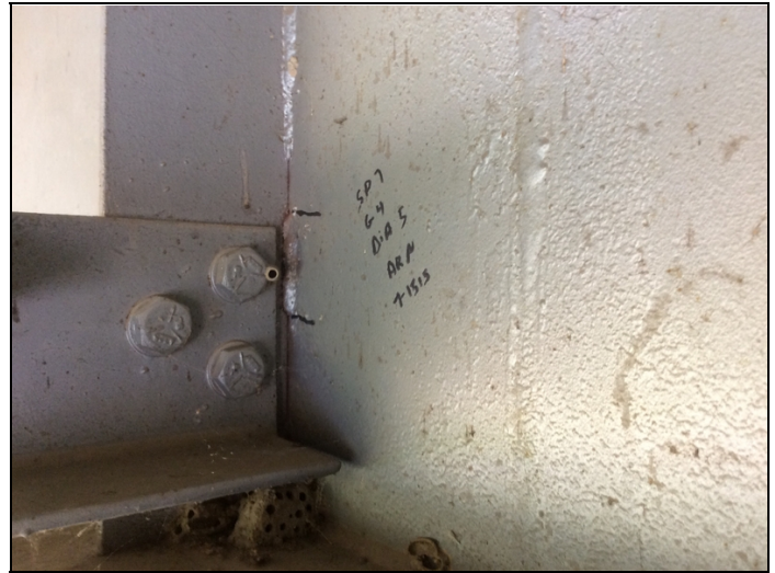
Span 7 girder 4 5th diaphragm has cracked welds.
