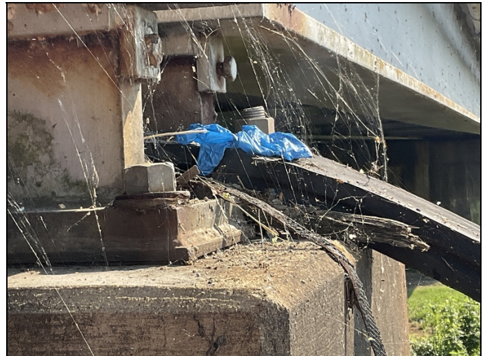
Pier 5 span 7 bearing 6 loose top bolt
