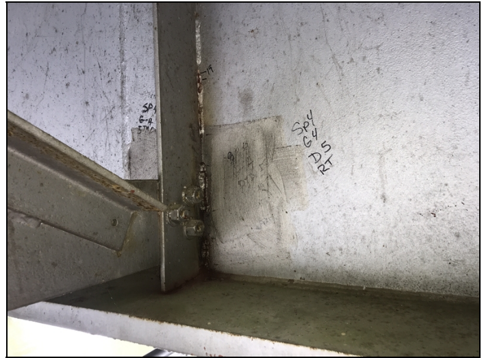
Span 4 g4 d5 diaphragm has Cracked welds
