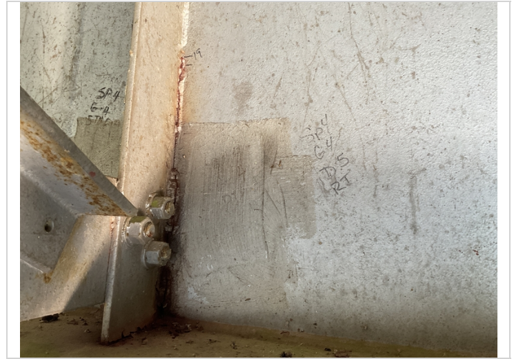
Span 4 girder 4 diaphragm 5 right side broke welds on diaphragm
