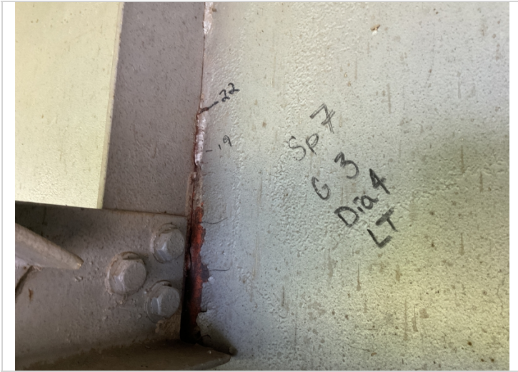
Span 7 girder 3 diaphragm 4 left side back broke welds.
