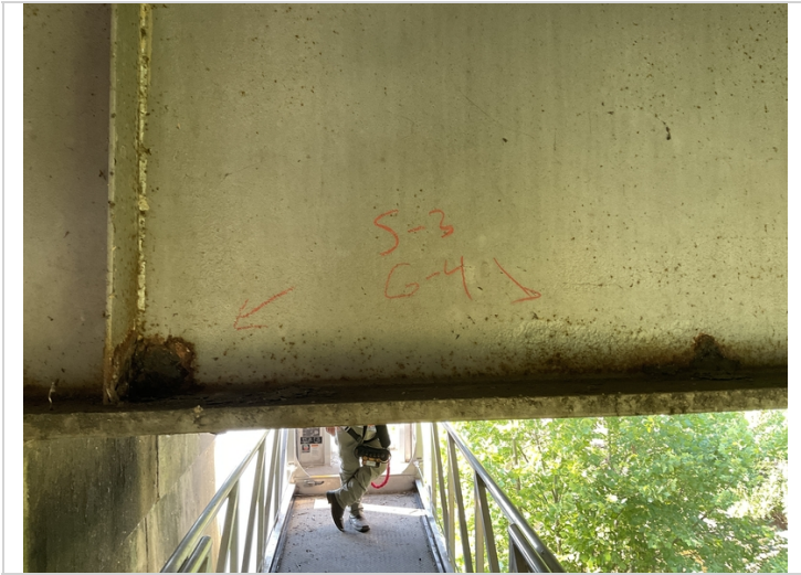
Span 3 girder 4 active corrosion with moderate pitting to lower web.
