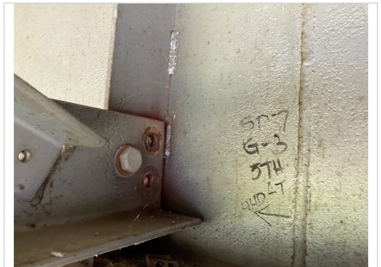
Span 7 girder 3 diaphragm 5 left side missing bolts.
